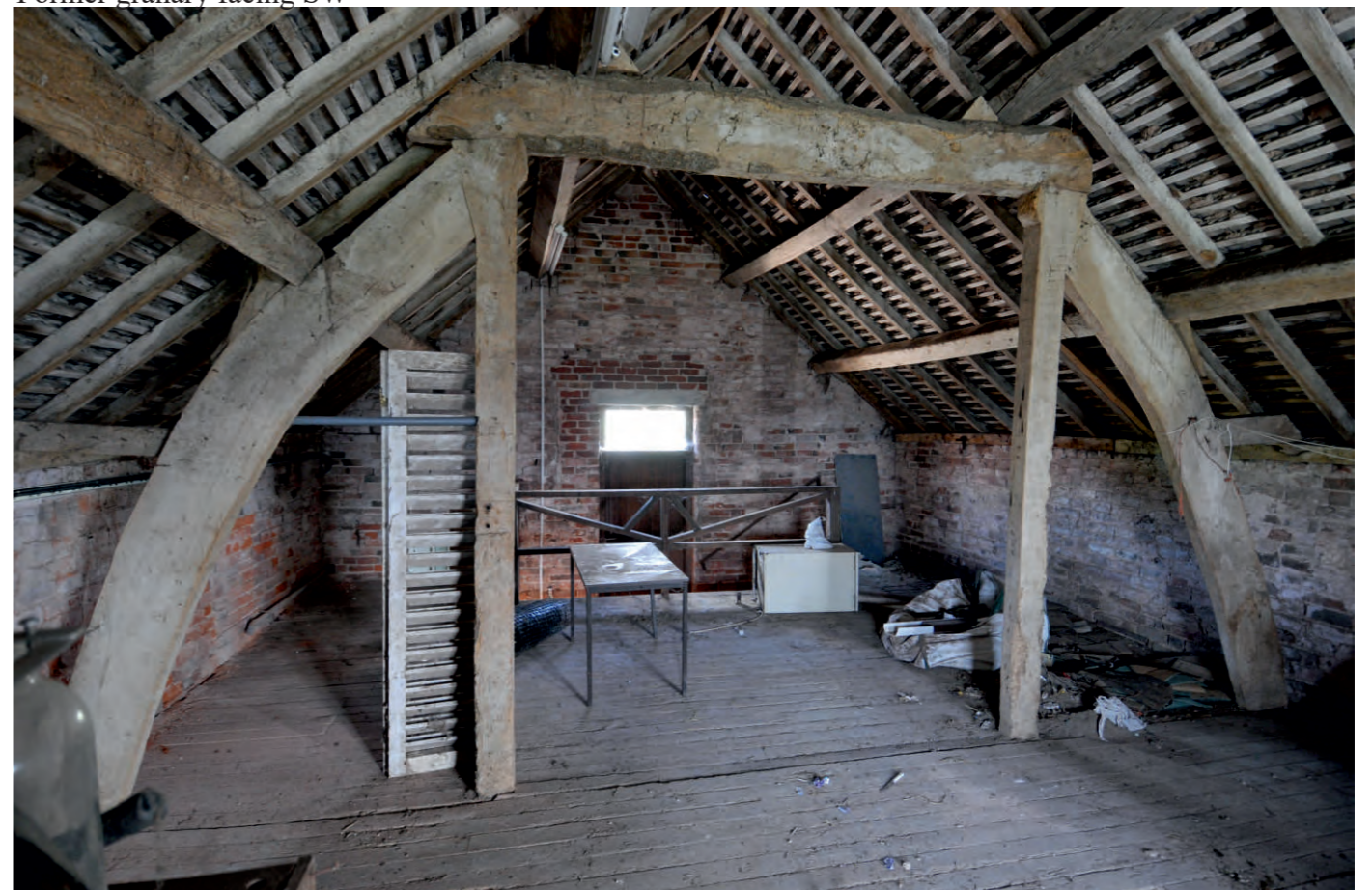
Former granary facing SW
