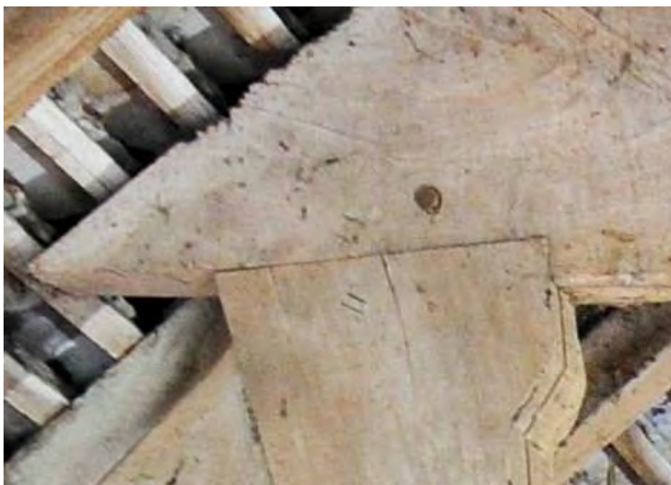
Enlarged detail of queen-post/collar joint showing small diameter pegging
