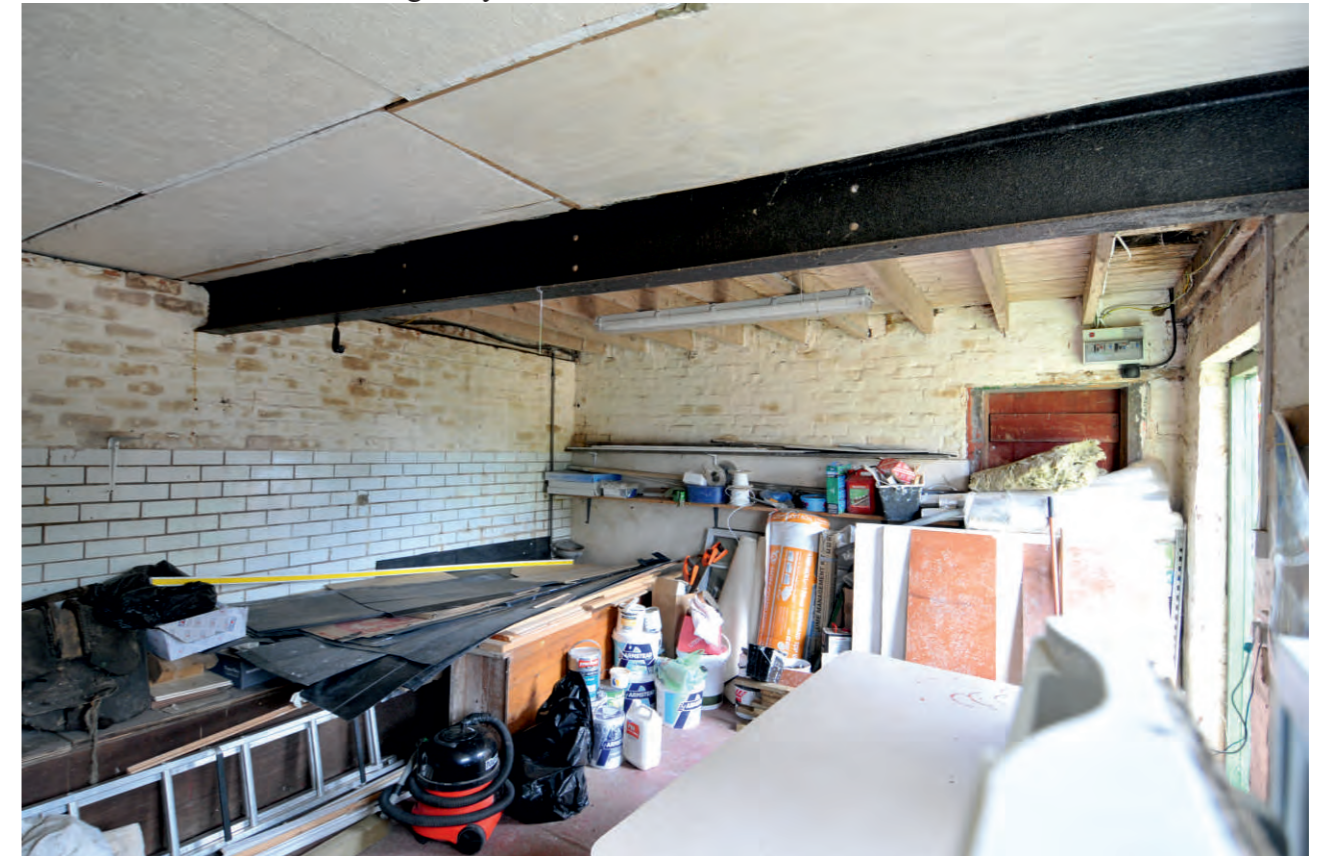
Middle ground floor room created by removal of stable partitions - note relatively recent RSJ on former wall line
