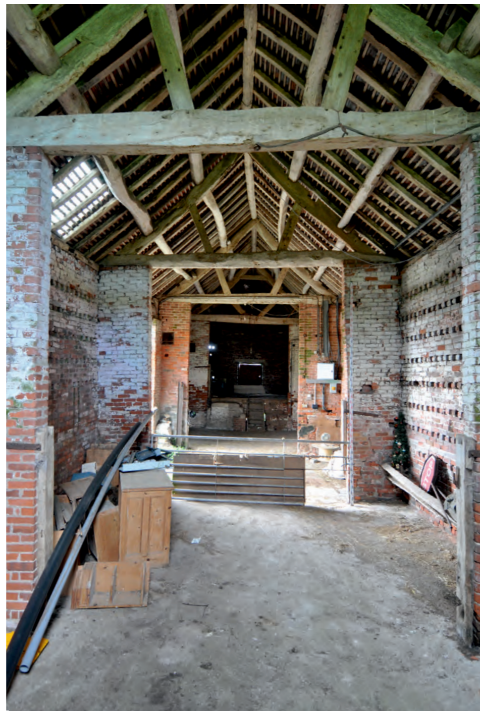
View from easternmost bay towards west
