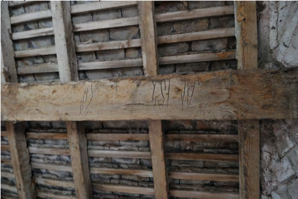
Baltic timber merchant's marks on purlin
