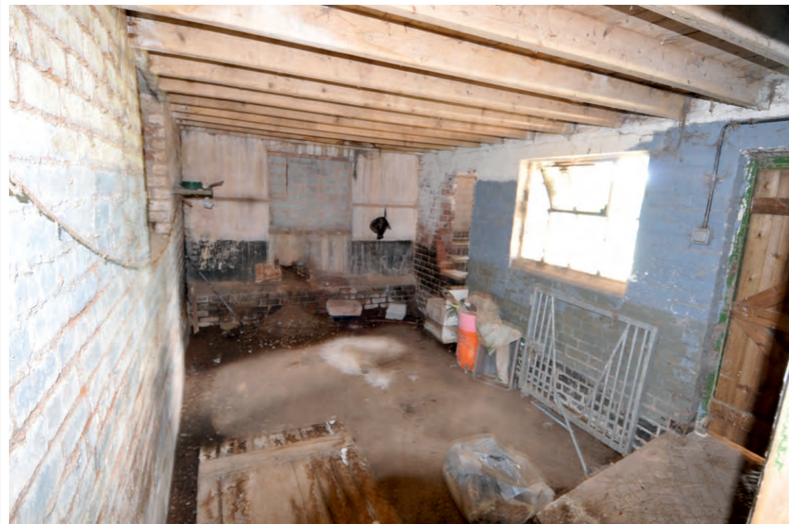
Former loading bay
