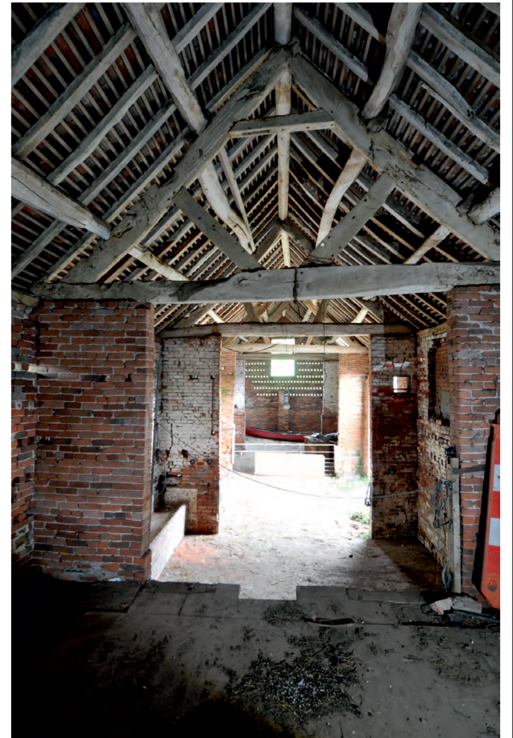
View facing east
