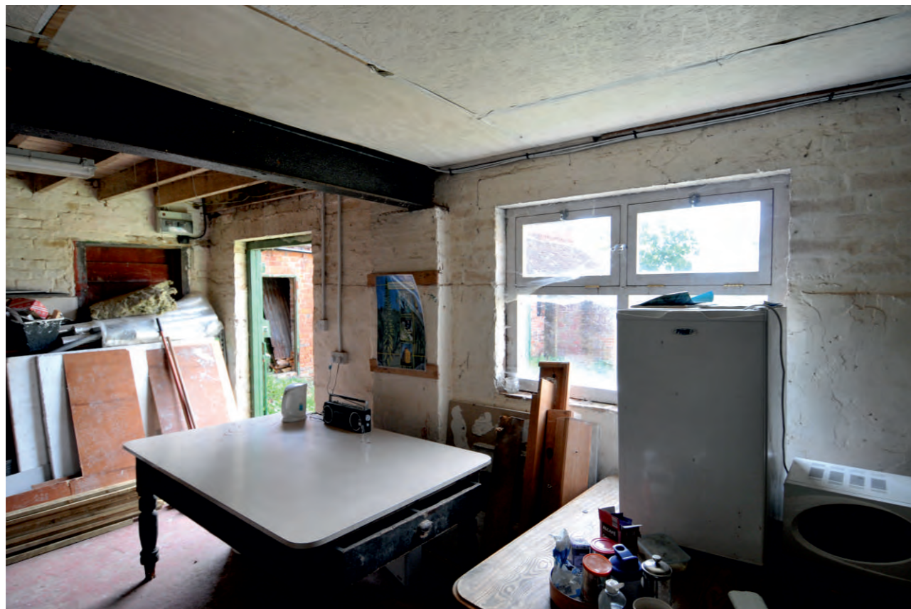
Middle ground floor room created by removal of stable partitions - note relatively recent RSJ on former wall line
