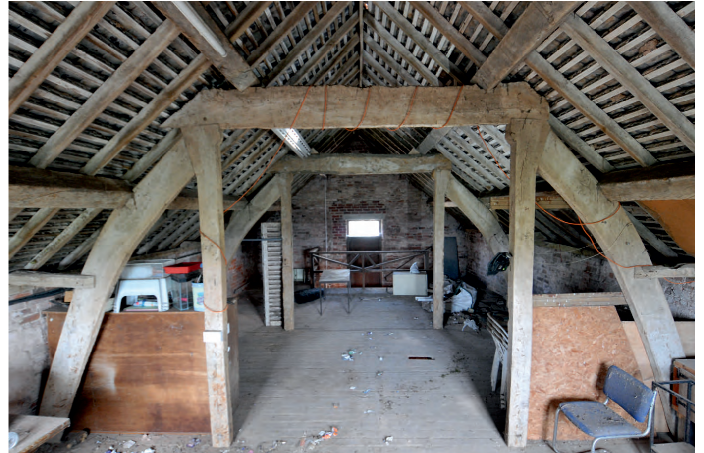
Former granary facing SW
