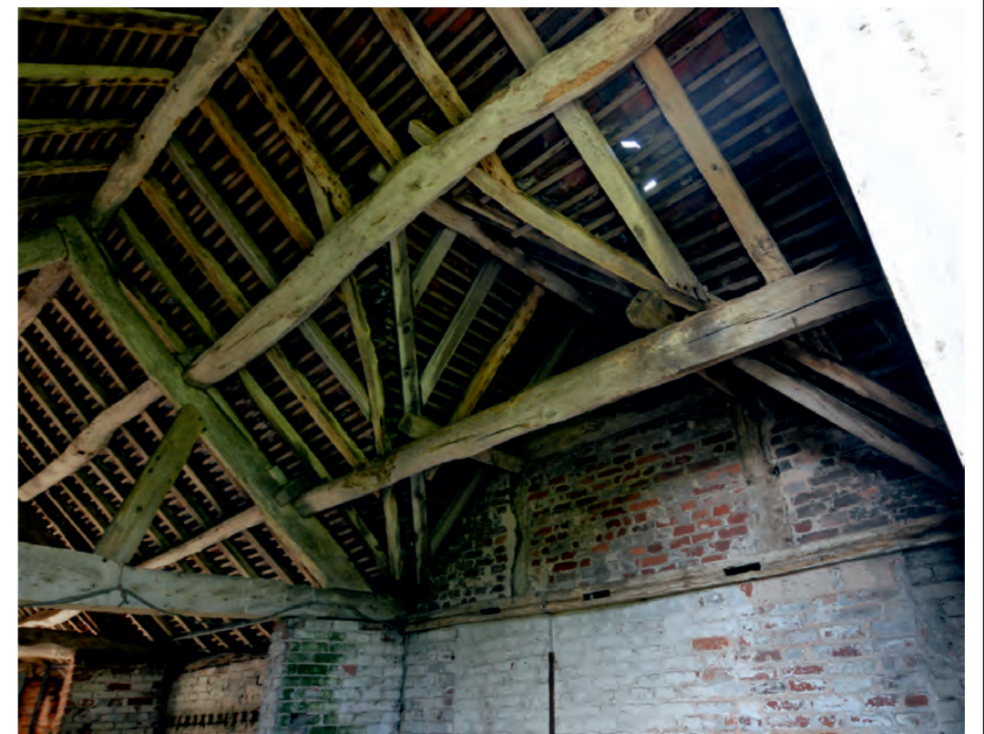
Link to stable block roof
