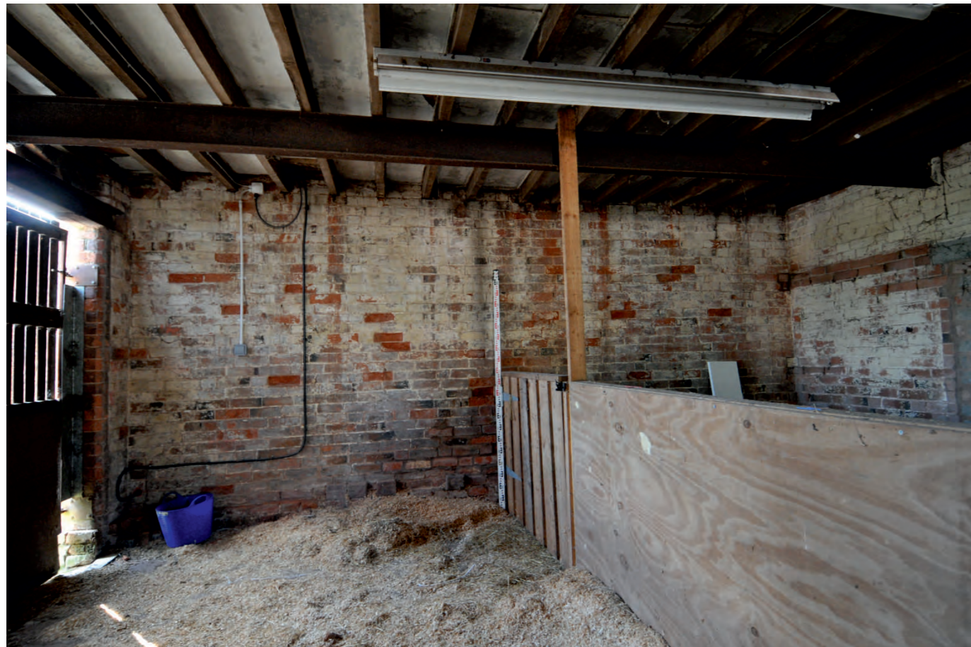
GF view facing SW
