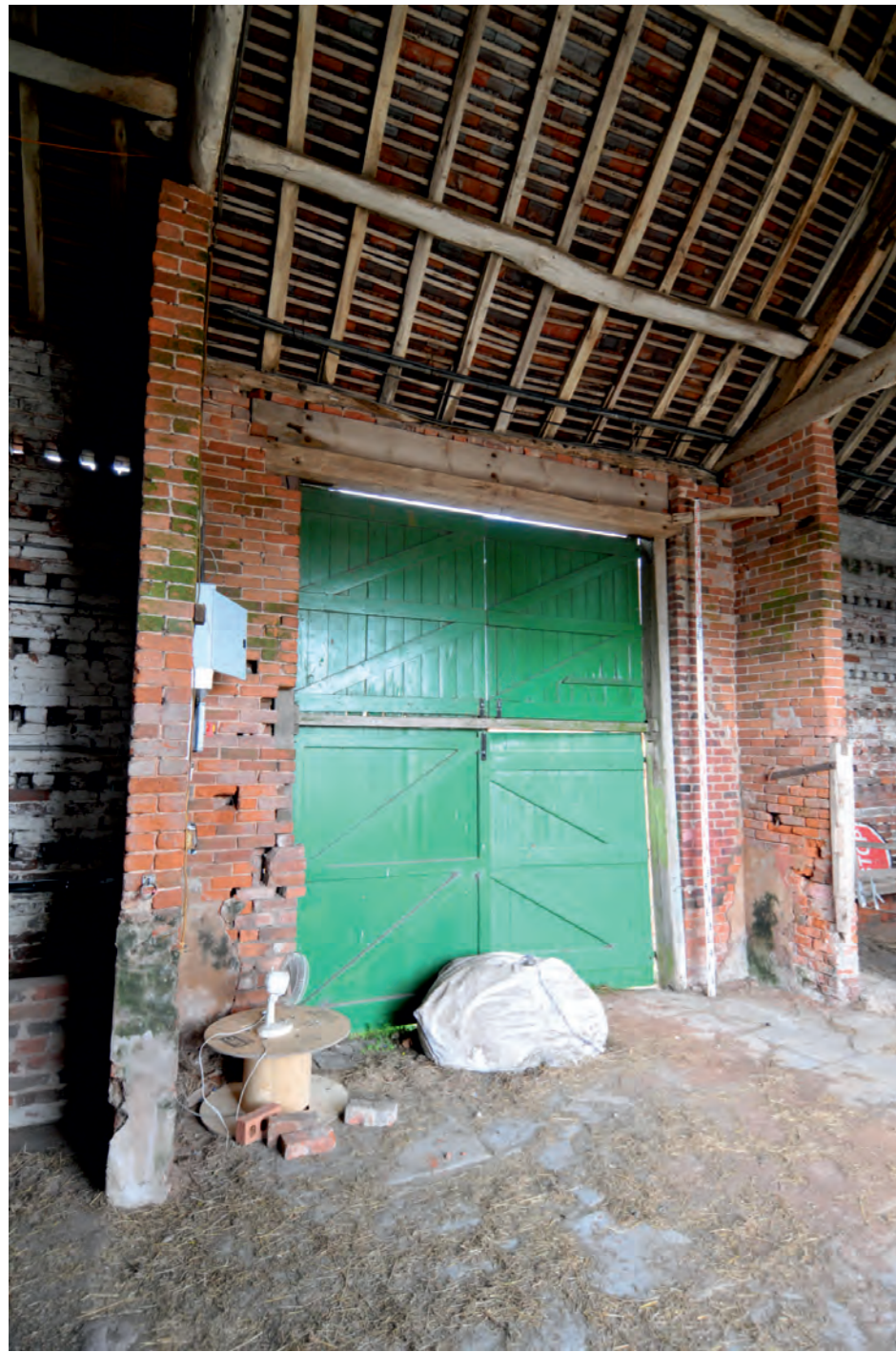
Threshing floor and (replacement) doors
