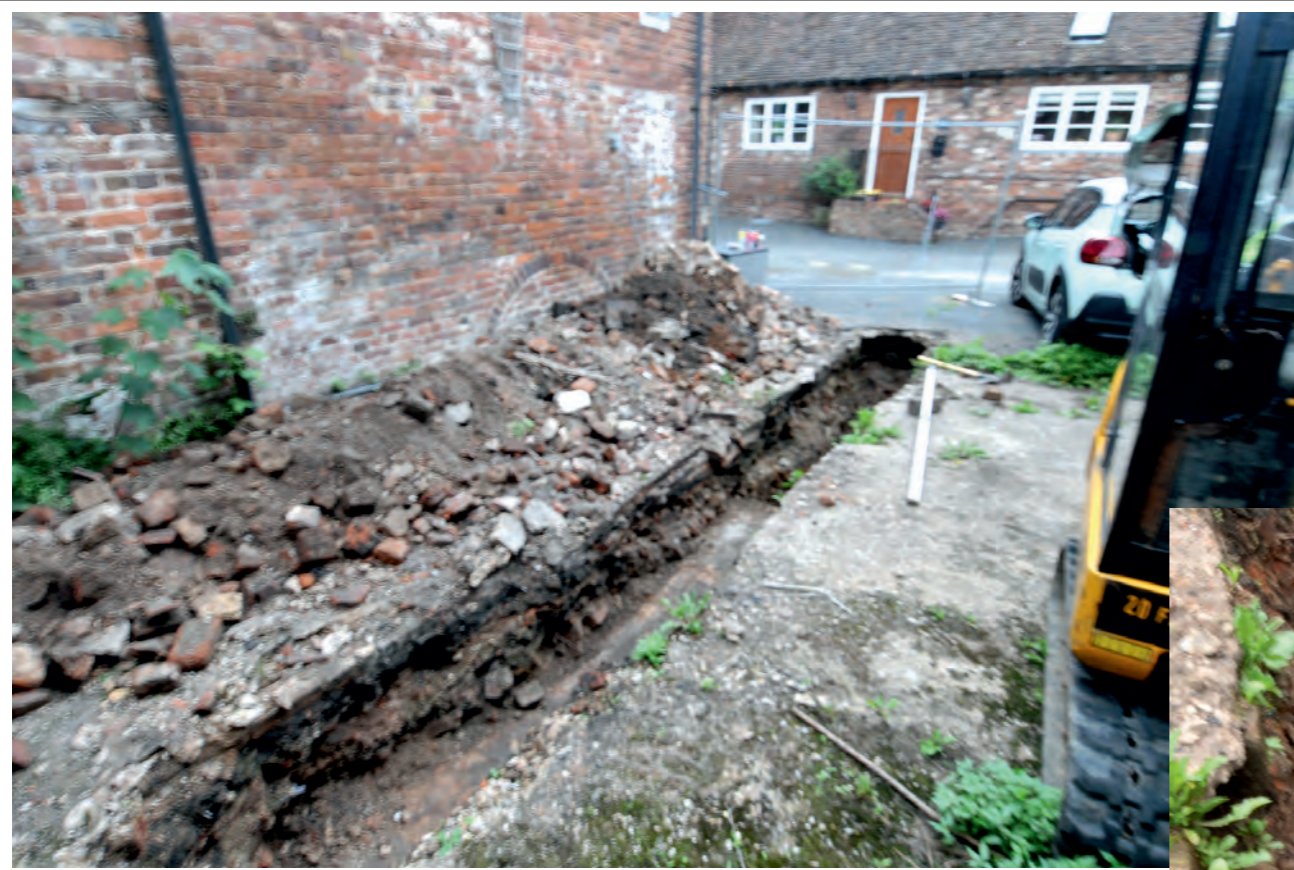
Trench location - facing south-east
