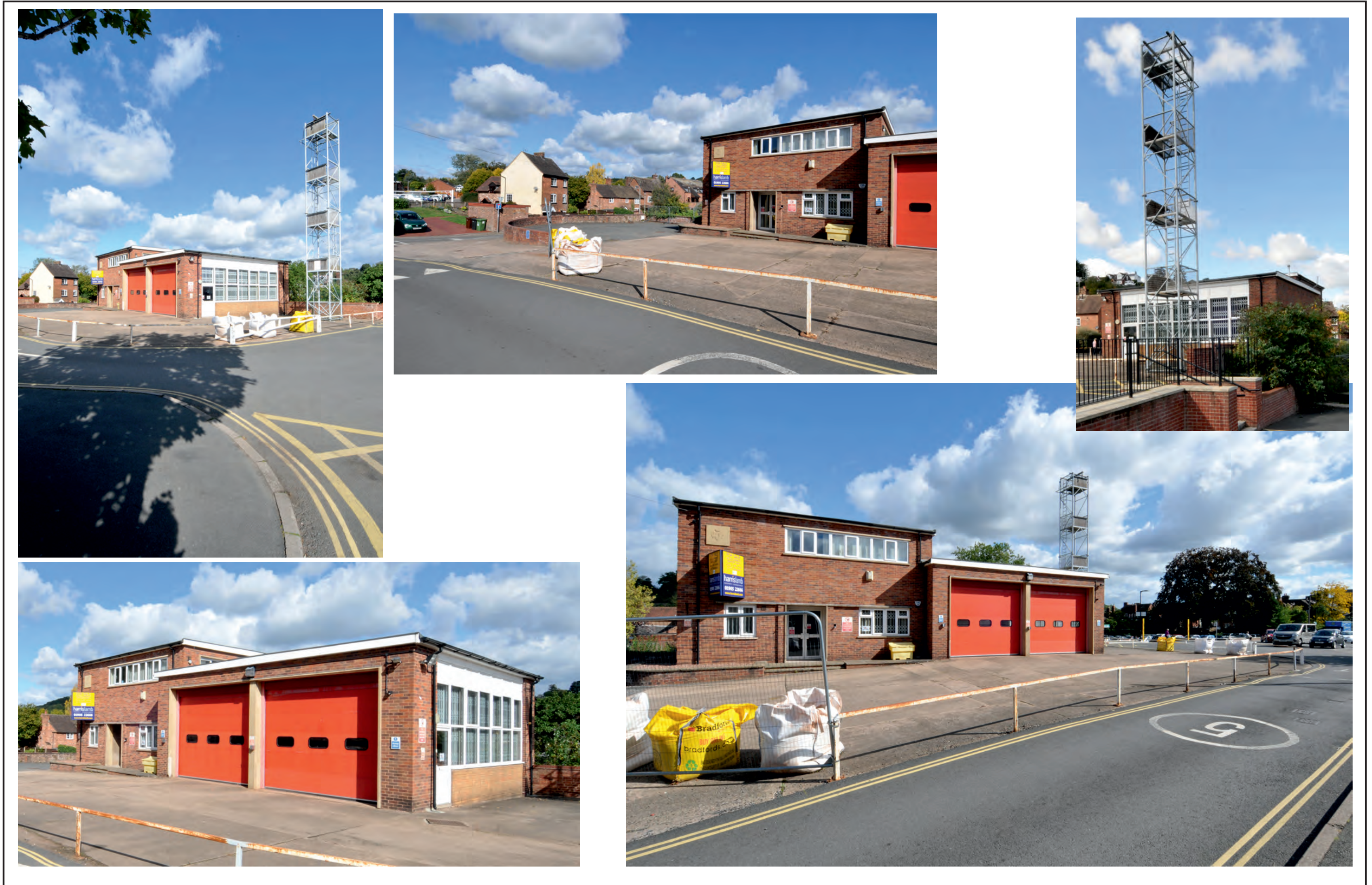
Figure 7: General views of firestation site
