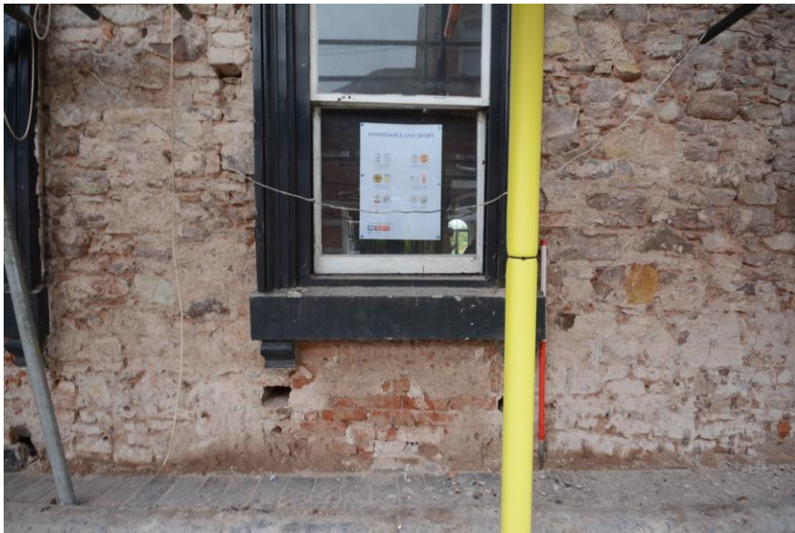
Fig. 28 Central ground-floor window, with blocking of earlier doorway beneath (photo ref: 7064).
