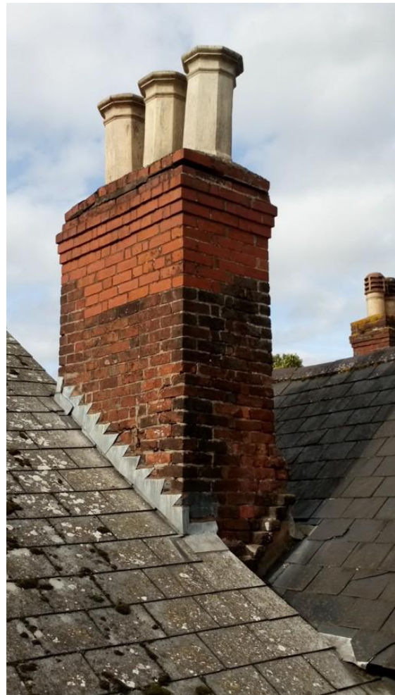
Fig. 49 Chimney of north gable, showing top eleven course rebuilt (photo ref: 0062).
