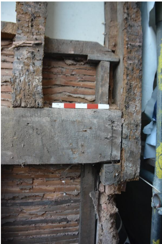
Fig. 40 Rear elevation, detail of timber framing, looking east (photo ref: 7489).
