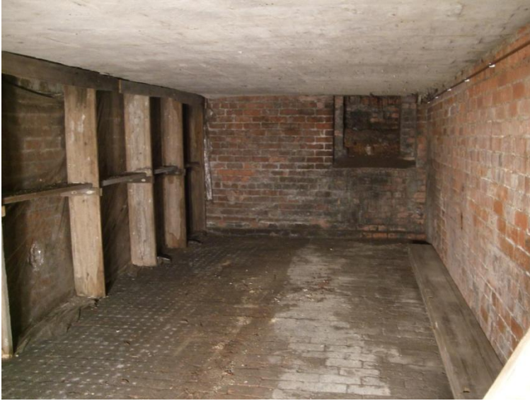
Plate 14 South extension: cellar viewed from the east.
