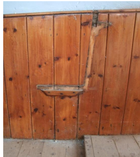
Plate 6 Wroot Wesleyan Chapel: pew fixings detail.
