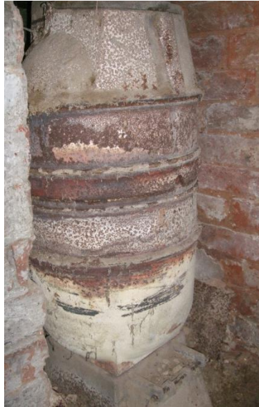
Plate 8 Wroot Wesleyan Chapel: the furnace in the subterranean chamber.
