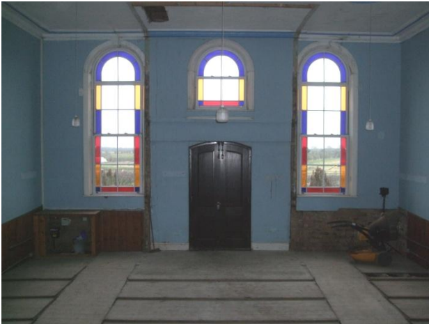
Plate 3 Wroot Wesleyan Chapel: interior, viewed from the south, showing stepped floor and the main entrance, minus lobby.
