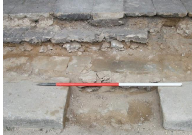
Plate 49 (Archive image PCGC 302) North Portico steps, north of centre: stone-capped duct beneath the middle step. Photograph: Caroline Atkins
