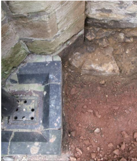
Plate 13 (Archive image PCGC 389) Eastern Gateway: west side, east elevation: blocking wall footing, south end. Photograph: Caroline Atkins
