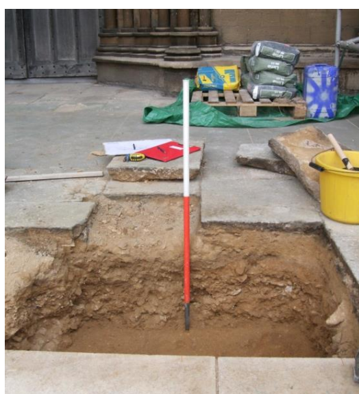
Plate 66 (PCGC 328) South Portico floodlight trench. Photograph: Caroline Atkins
