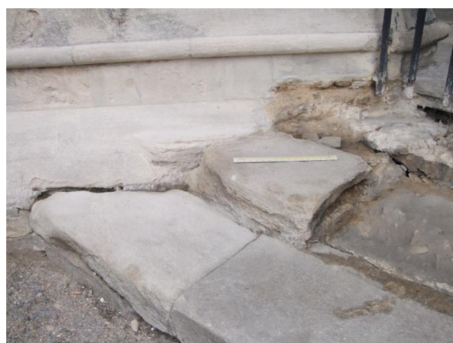
Plate 47 (Archive image PCGC 235) North Portico steps, north end: with evidence for the original Clipsham step profiles. Photograph: Caroline Atkins
