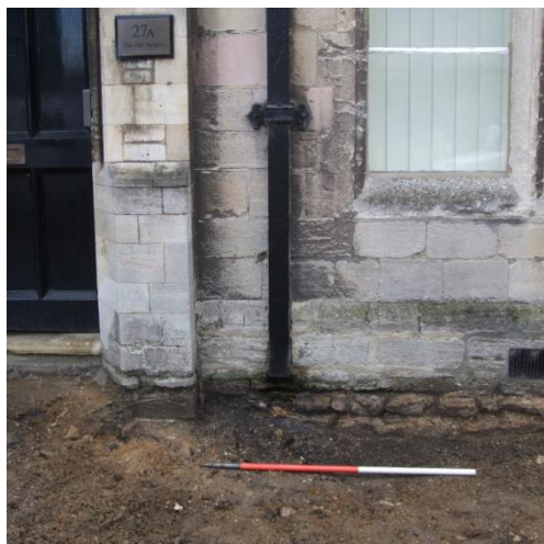
Plate 31 (Archive image PCGC 163) No. 28: potential medieval footings to the east of the buttress. Photograph: Caroline Atkins
