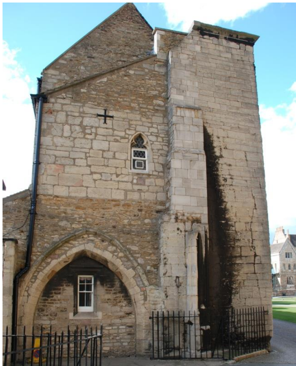
Plate 3 The Eastern Gateway. Note the wall rib of the vaulted gate passage above the main arch connecting the gateway with No. 24. No. 24's NE tower is right of frame). Photograph: Jackie Hall
