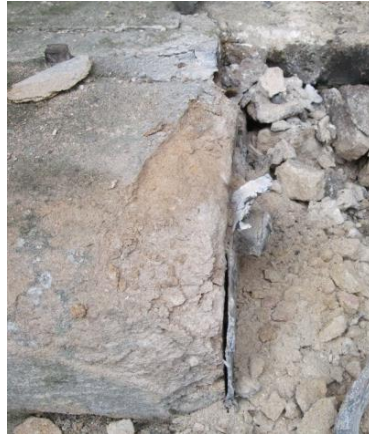
Plate 44 (Archive image PCGC 198) North Portico, top step: the lead cramp exposed. Photograph: Caroline Atkins
