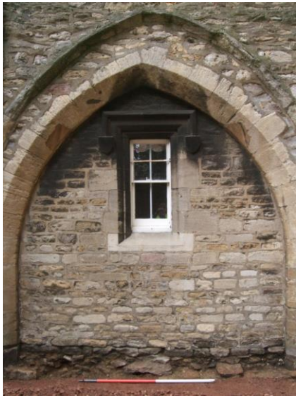
Plate 11 (Archive image PCGC 380) Eastern Gateway: west side, east elevation with exposed footing. Photograph: Caroline Atkins
