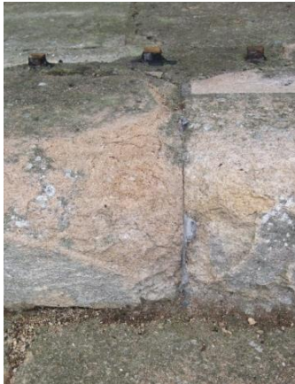
Plate 43 (Archive image PCGC 194) North Portico, top step: lead visible in the vertical joint between the 2 nd and 3 rd stones from the N end. Photograph: Caroline Atkins
