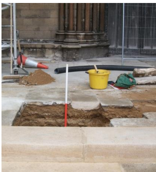
Plate 65 (PCGC 331) North Portico floodlight trench. Photograph: Caroline Atkins
