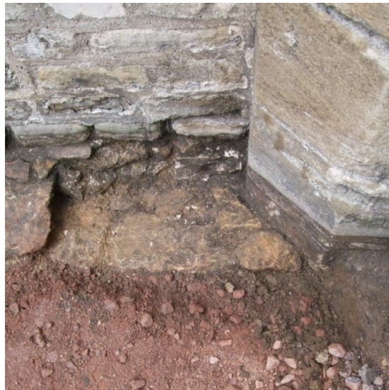
Plate 14 (Archive image PCGC 390) Eastern Gateway: west side, east elevation: blocking wall footing, north end. Photograph: Caroline Atkins
