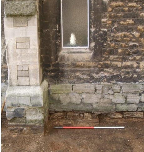
Plate 33 (Archive image PCGC 111) No. 28: potential medieval footings to the west of the buttress. Photograph: Caroline Atkins
