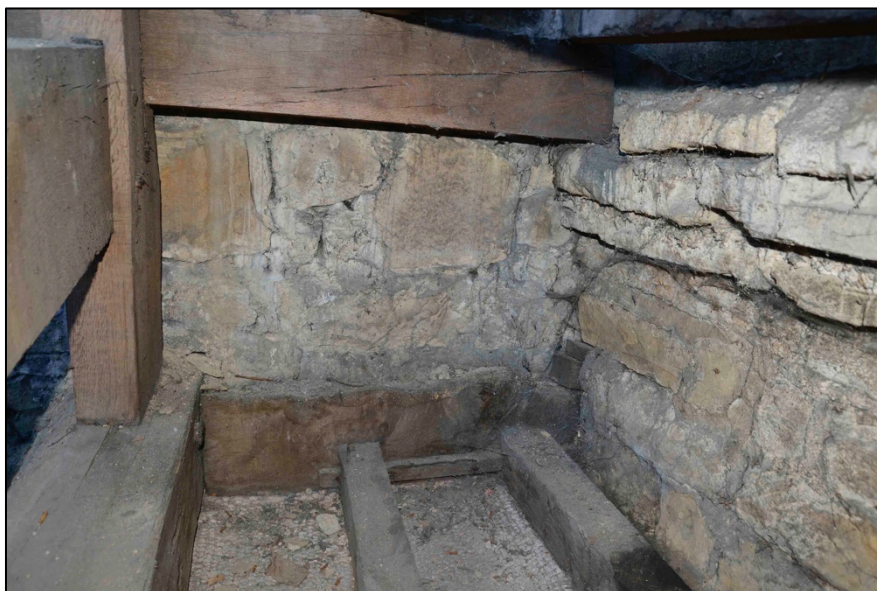
Appendix I.37: Detail of south-east corner of Area A within ceiling void; note stone offset.
