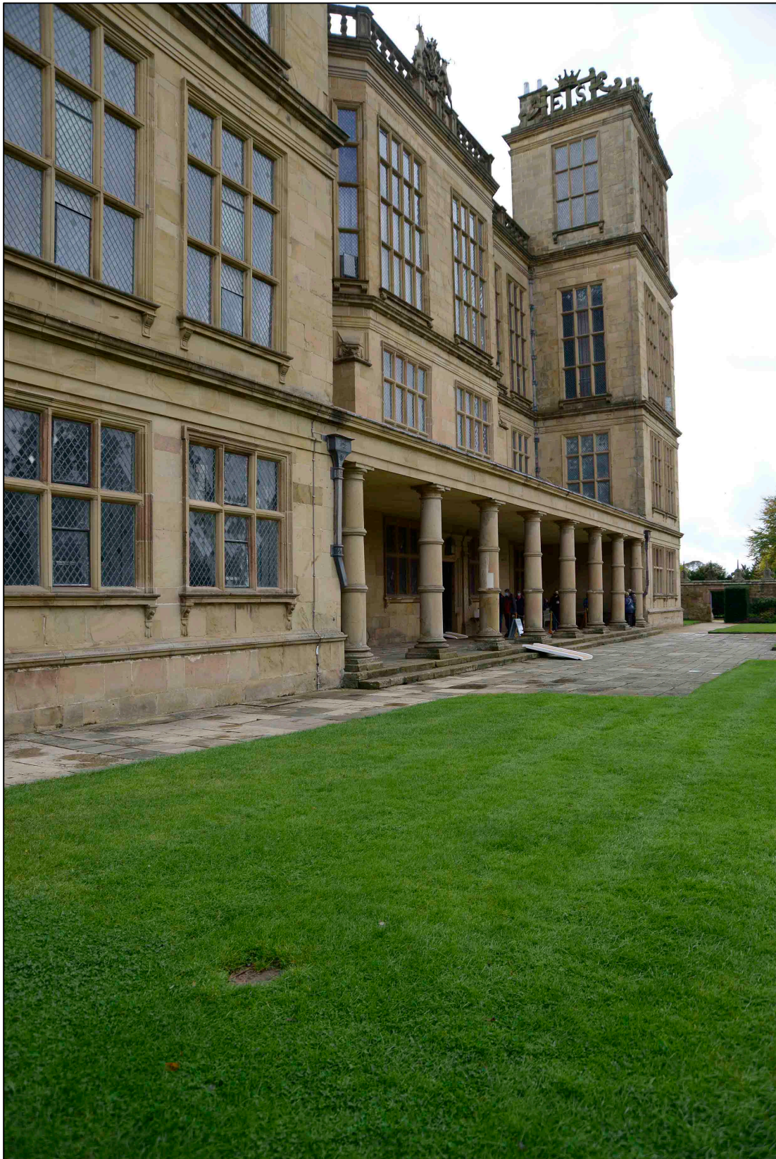
Appendix I.1: View of West Loggia prior to repairs in October 2020, looking south-east
