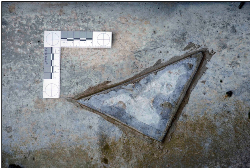
Appendix I.13: Detail of patch repair in lead.
