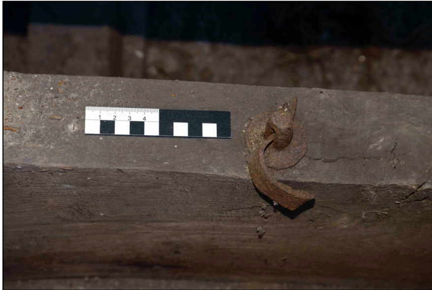
Appendix I.39: Detail of iron peg with cotter pin on T9.
