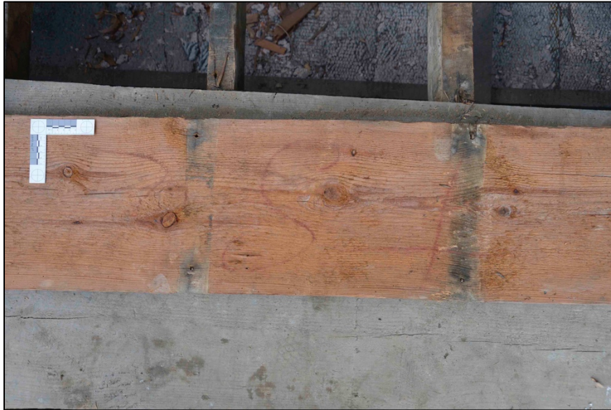
Appendix I.18: Detail of underside of 'original' pine board; note red letters T S 2.
