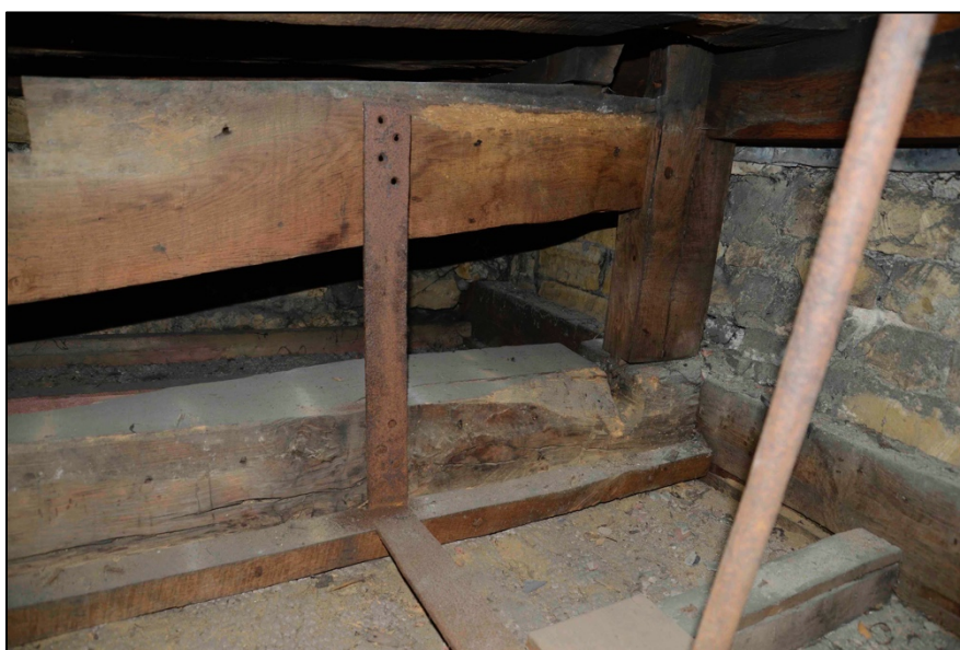
Appendix I.44: Detail of iron strap against T1 in Area C .
