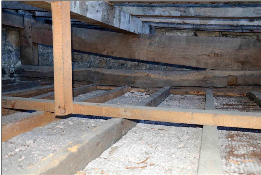
Appendix I.32: Detail of roof void in Area A , looking south.
