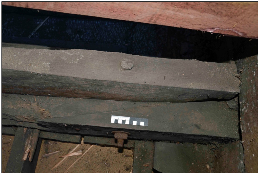
Appendix I.40: Detail of bolted repair on T10.
