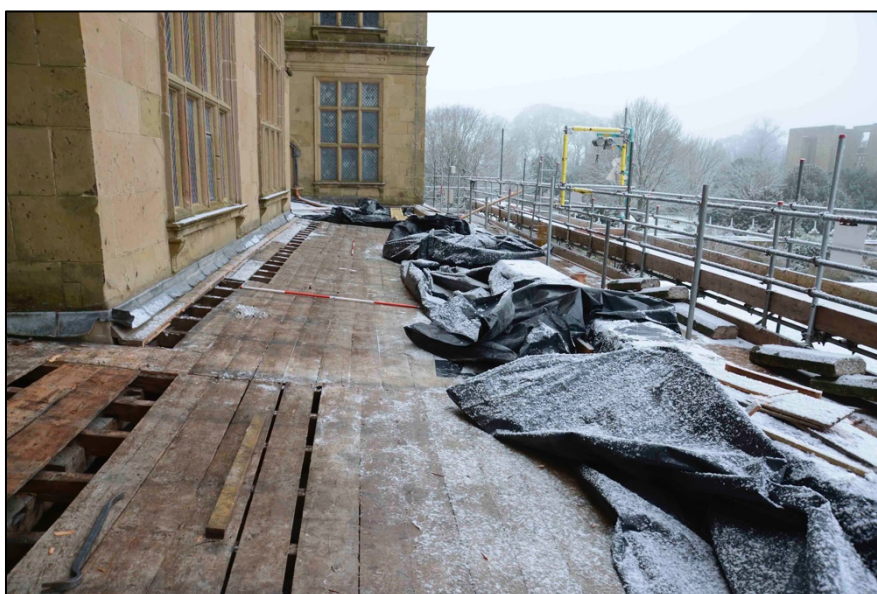
Appendix I.17: View looking south along exposed boards below leads.
