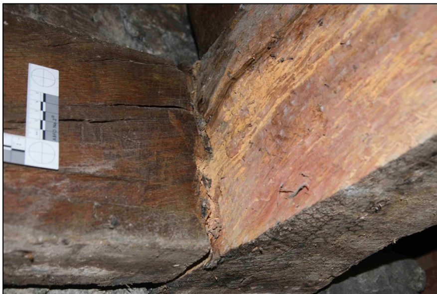
Appendix I.52: Detail of chisel cut assembly marks (IX) on lower timber bearer against west wall of Hall in Area C .
