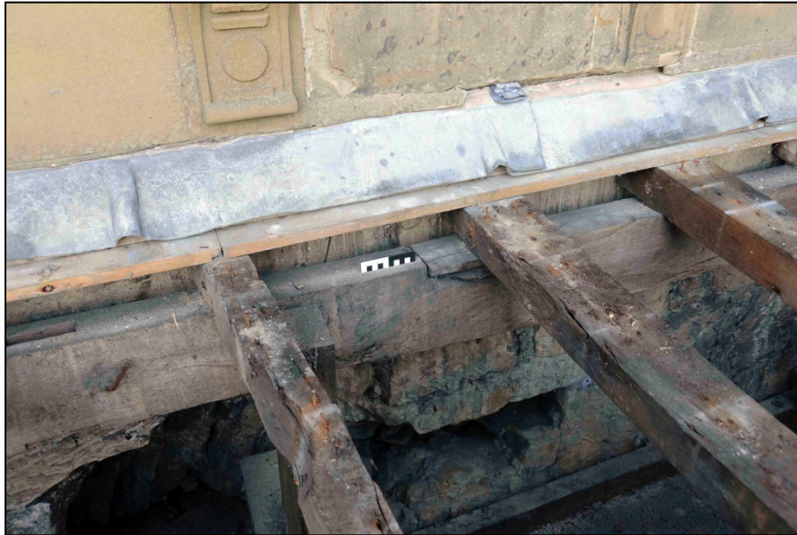
Appendix I.28: Detail of timber construction along the west wall of the Hall in Area A ; note inset hole in masonry within roof void.
