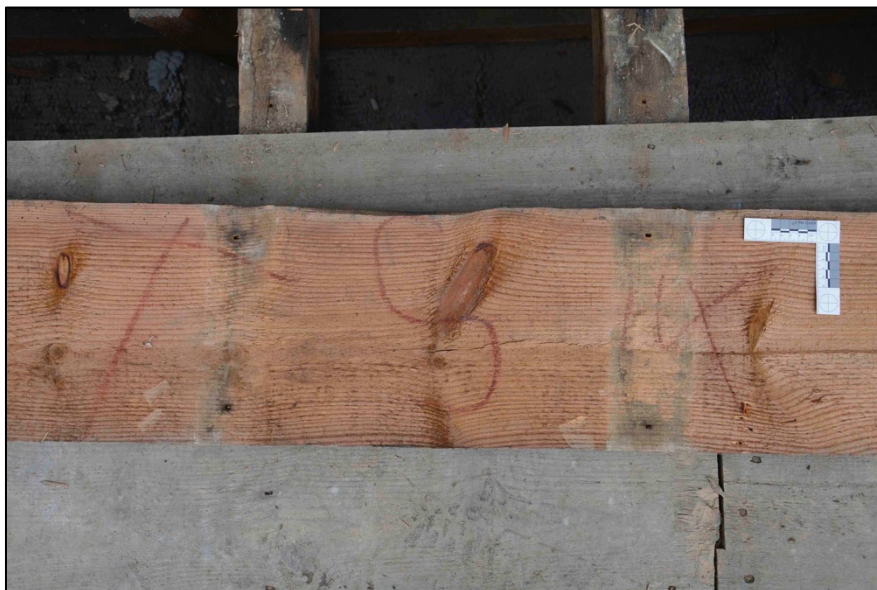
Appendix I.19: Detail of underside of 'original' pine board; note red letters T S 14.
