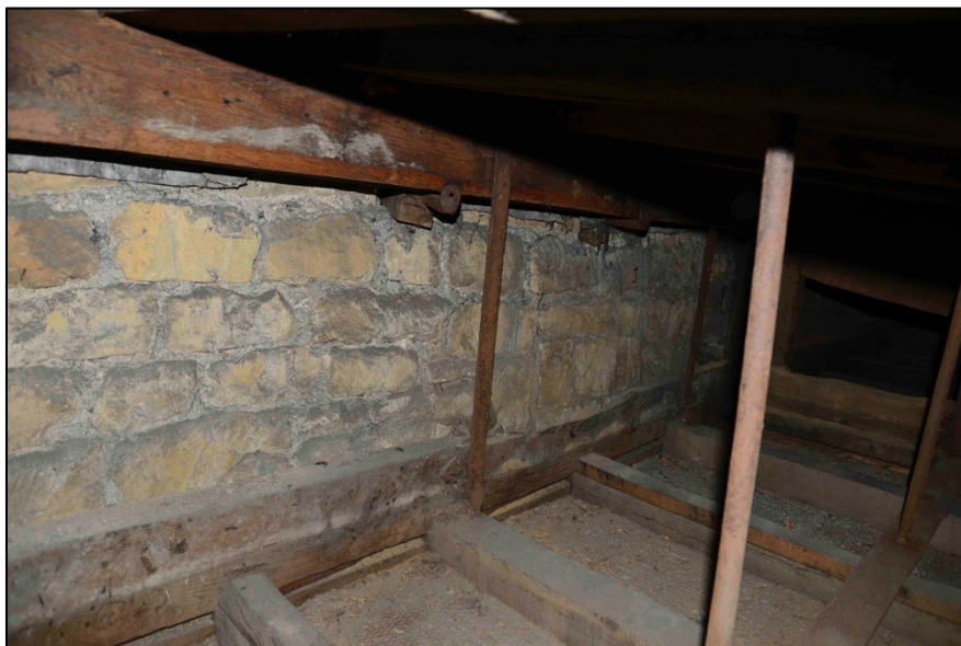
Appendix I.43: Detail of rough coursed walling (not ashlar) within ceiling void of Area C ; note inserted iron rods.
