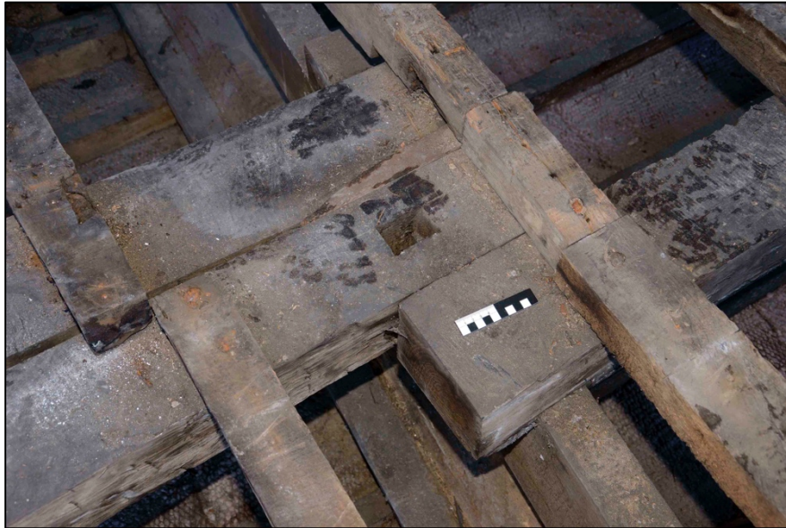
Appendix I.54: Detail of three parallel upper purlins in Area A ; note reused timbers.
