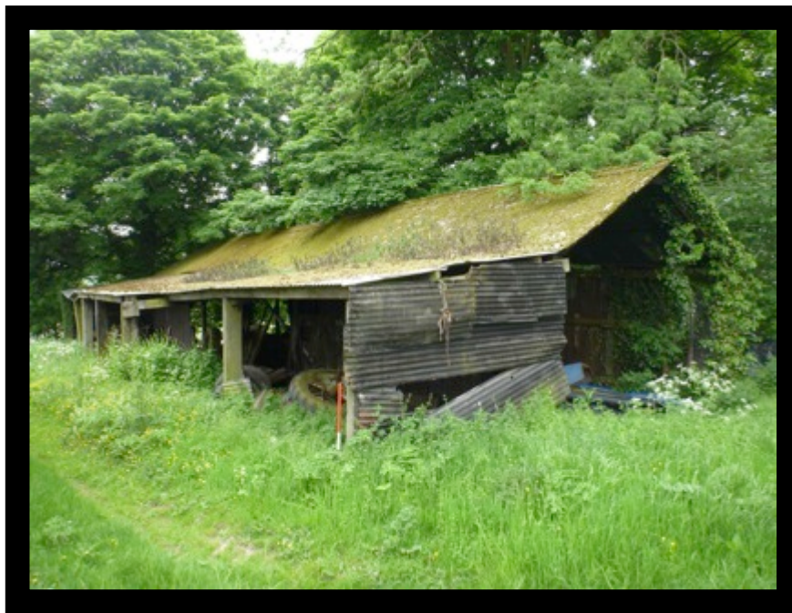
Photo: General view, looking southwest (1m scale)
