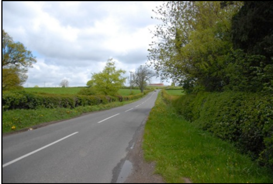
View along Brookhill Lane from Brookhill Farm, looking northeast
