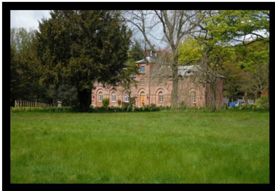
Photo: General view of Stableblock, looking north
