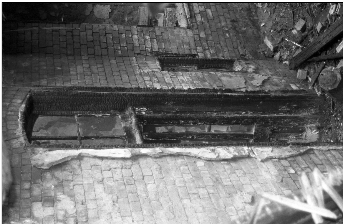
Appendix 5.22: Detail of north end of central north-south corridor; note glazed fanlight (Film 2.10).
