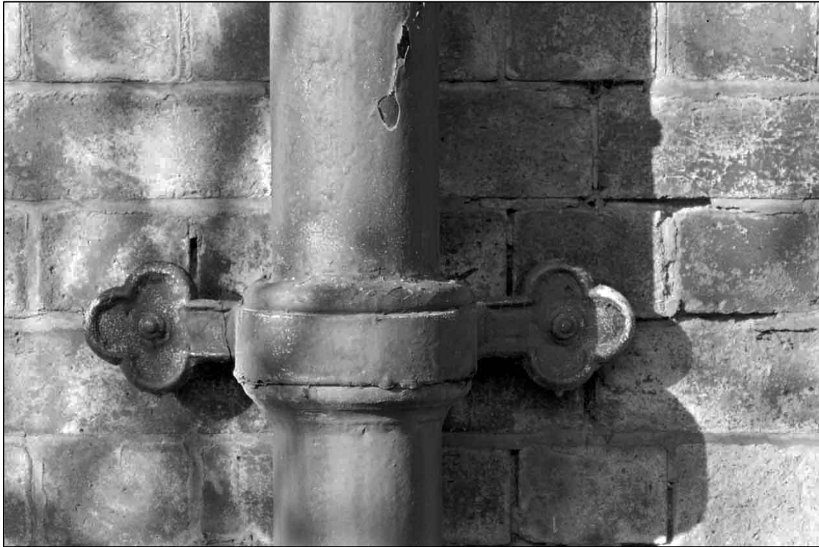
Appendix 5.13: Detail of cast-iron downpipe bracket with trefoil terminals (Film 1.7).
