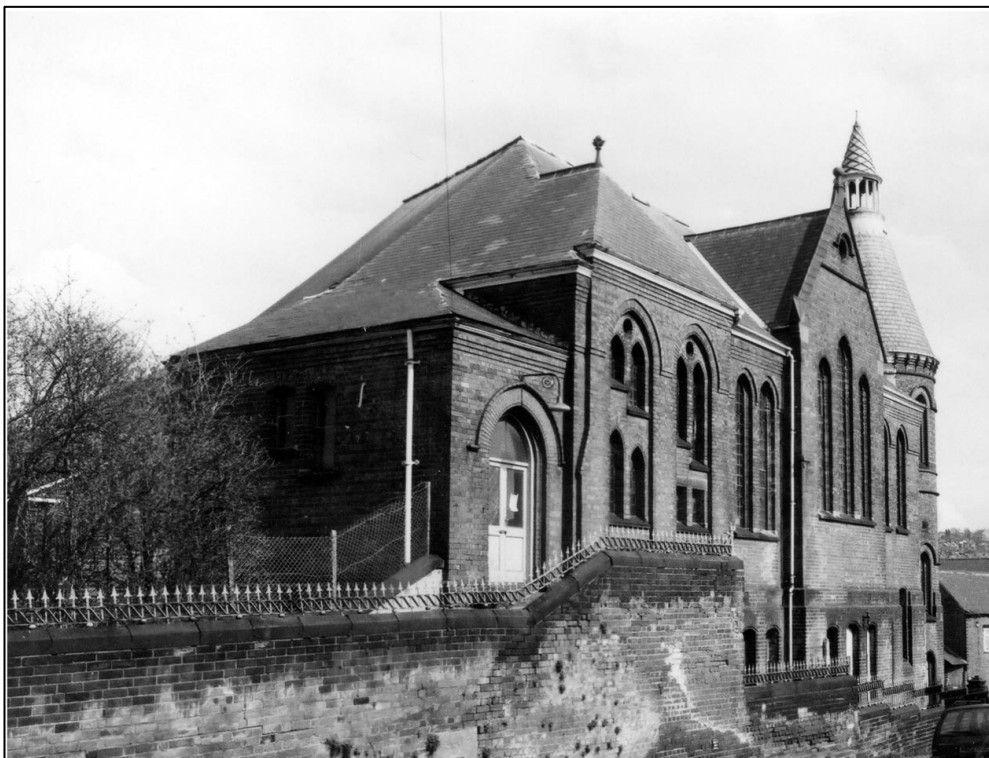
Appendix 5.2: General view of South View Road elevation, looking south-east c.2001, before being damaged by fire. Picture Sheffield ref: v02709. © Stanley Jones, reproduced with permission
