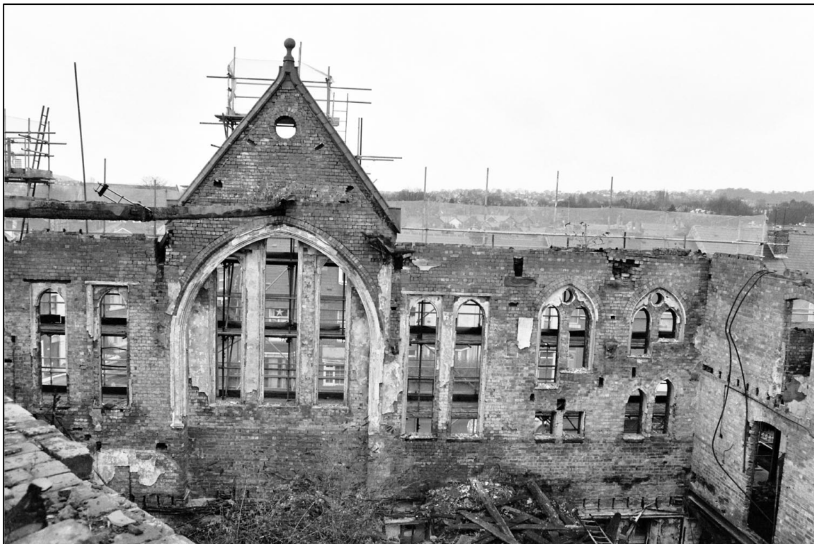
Appendix 5.32: Detail of internal South View Road elevation, looking west (Film 2.25).
