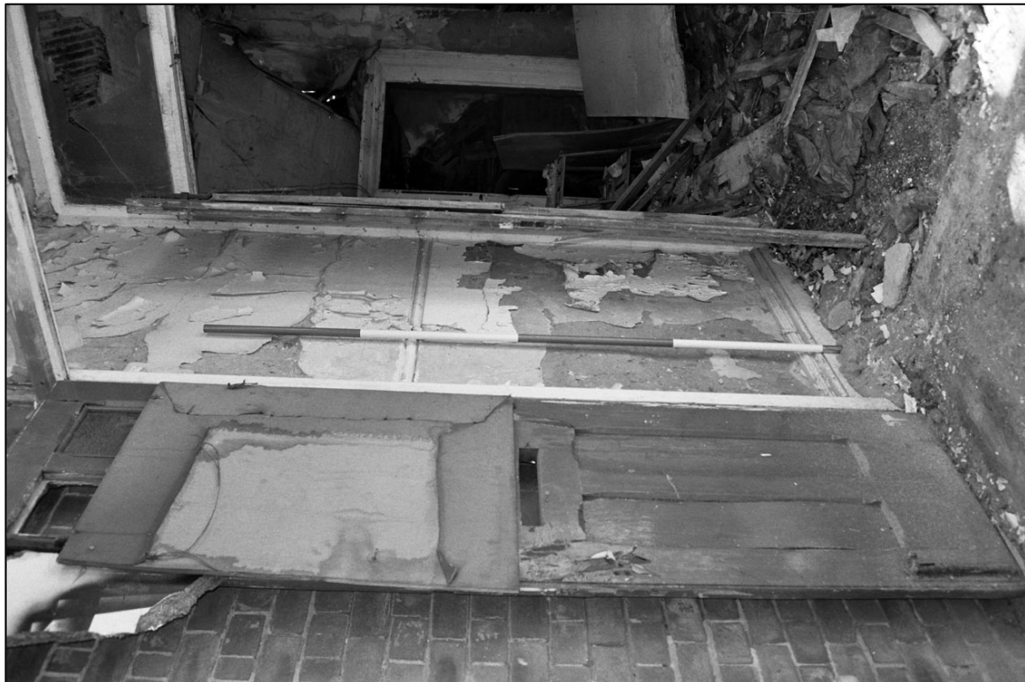
Appendix 5.12: Detail of ground floor doorway on Vincent Road, looking west; note plaster moulded dado (Scale 2m; Film 1.24).
