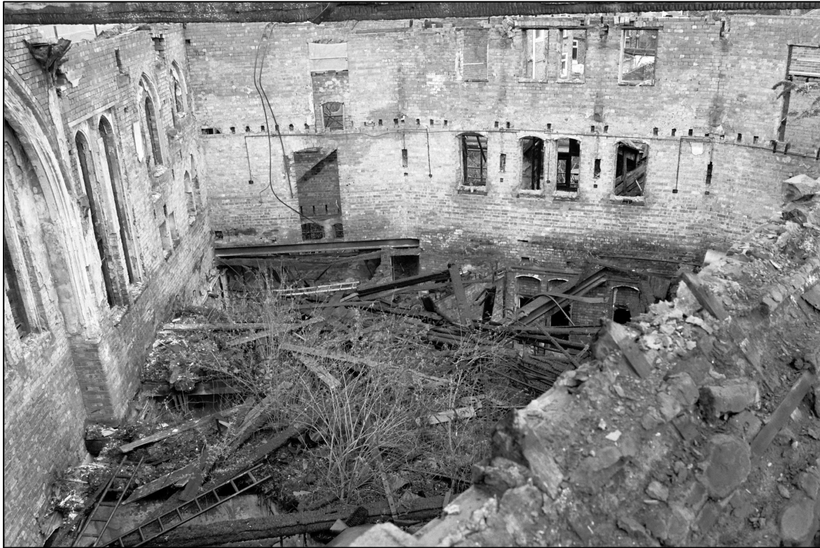
Appendix 5.31: General view of interior, looking north-west of north elevation (Film 2.26).
