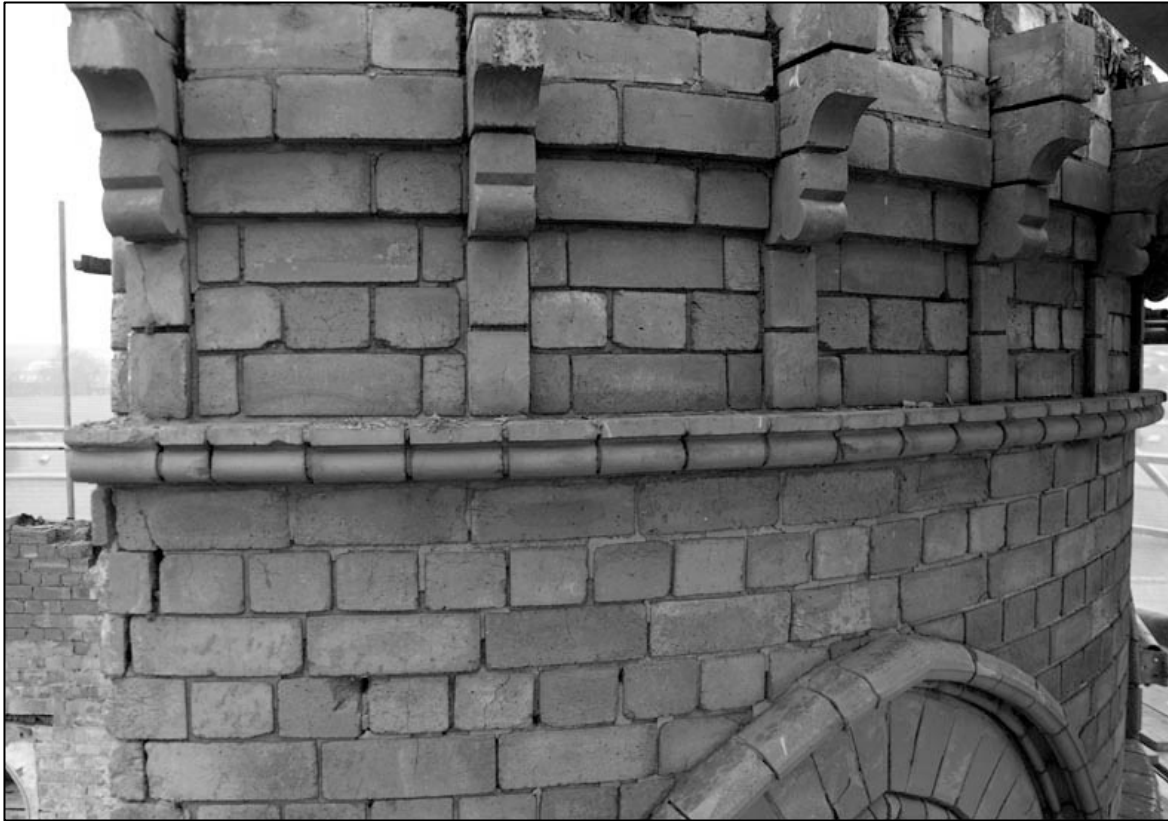
Appendix 5.17: Detail of decorative brickwork at eaves level of turret at south end of building (Digital photograph).
