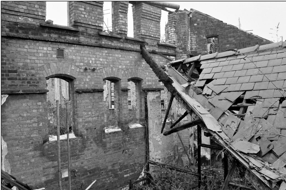
Appendix 5.18: Detail of north extension; note original elevation concealed by later roof pitch (Film 2.19).
