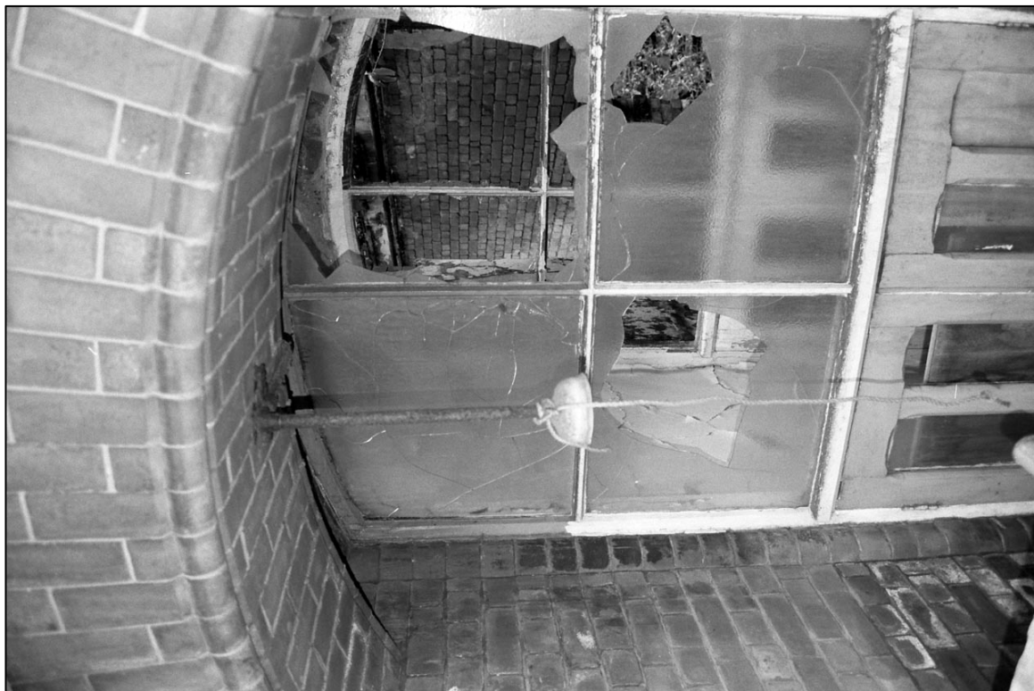
Appendix 5.16: Detail of glazed fanlight in doorway at ground floor level on South View Road (Film 2.4).
