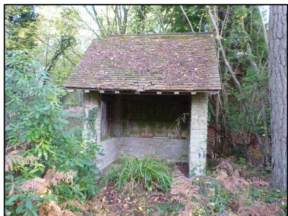
Appendix 3.12: Small summer house (dated 1929), on east bank of north pond.
