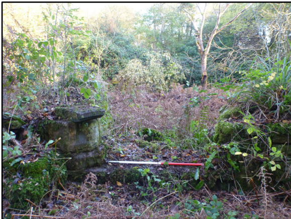
Appendix 3.9: Surviving stone doorway with carved jamb in east part of inner ward (1m scale).
