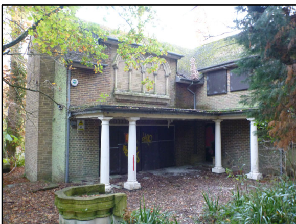
Appendix 3.11: Modern house (1980s) on west bank of north pond.
