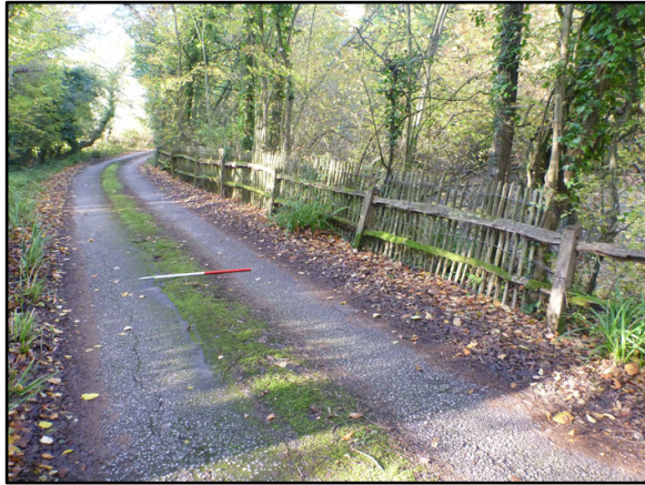
Appendix 3.1: Earth dam, looking northwest.
