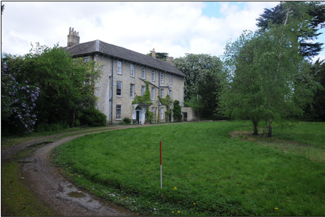
Appendix 3.47: View across the entrance forecourt HA17 towards Woodstock House HA1 (1m scale).
