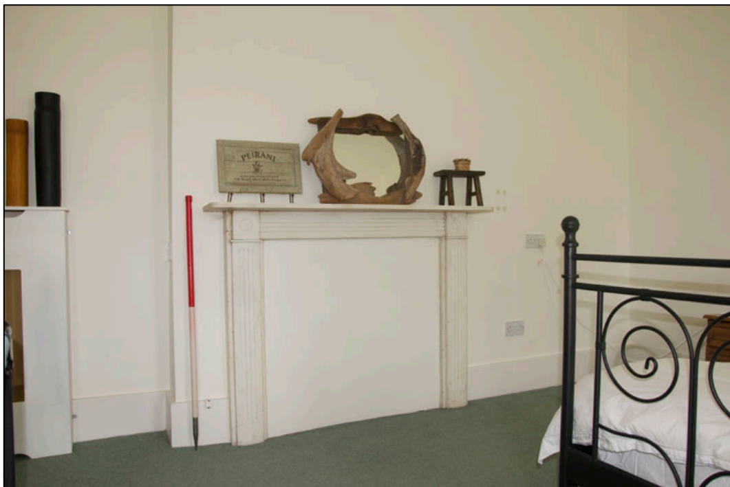
Appendix 3.16: Detail of blocked marble fireplace on first floor of Woodstock House HA1 (1m scale).
