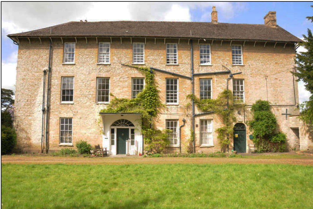
Appendix 3.2: General view of east elevation of Woodstock House HA1 from Entrance Forecourt HA17 (1m scale).
