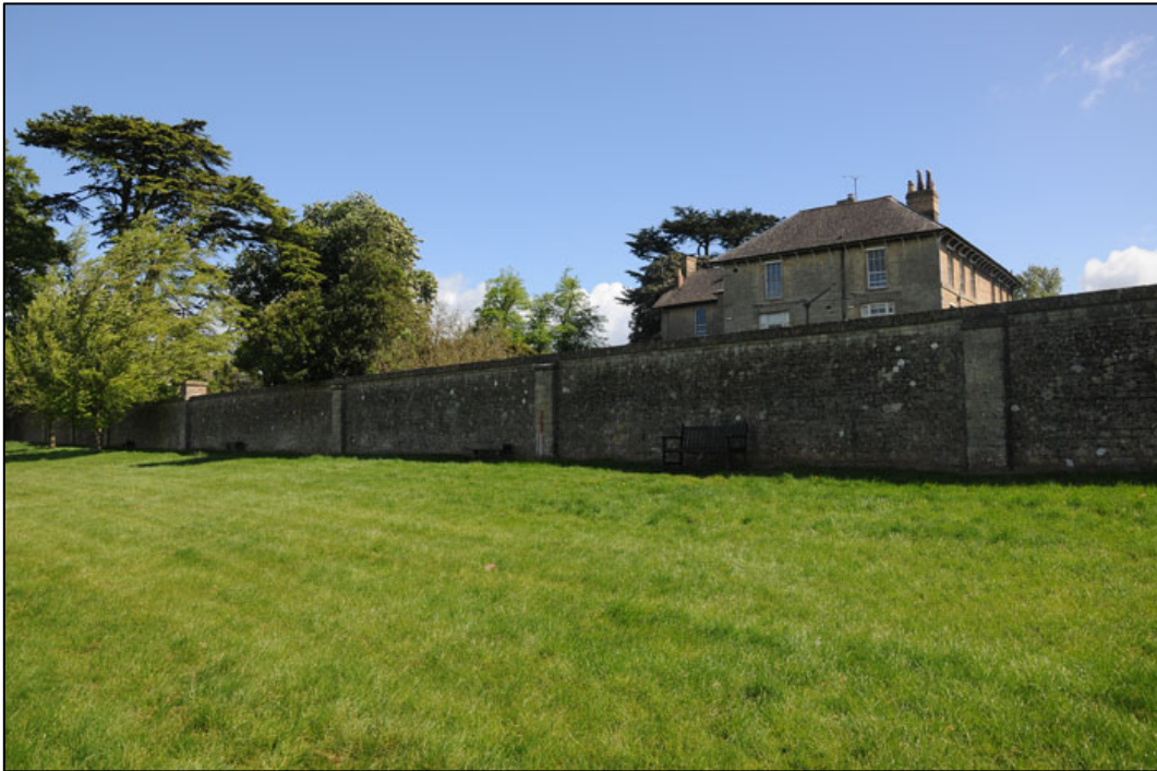
Appendix 3.37: General view of parkland boundary wall HA10 , looking northeast from parkland (1m scale).
