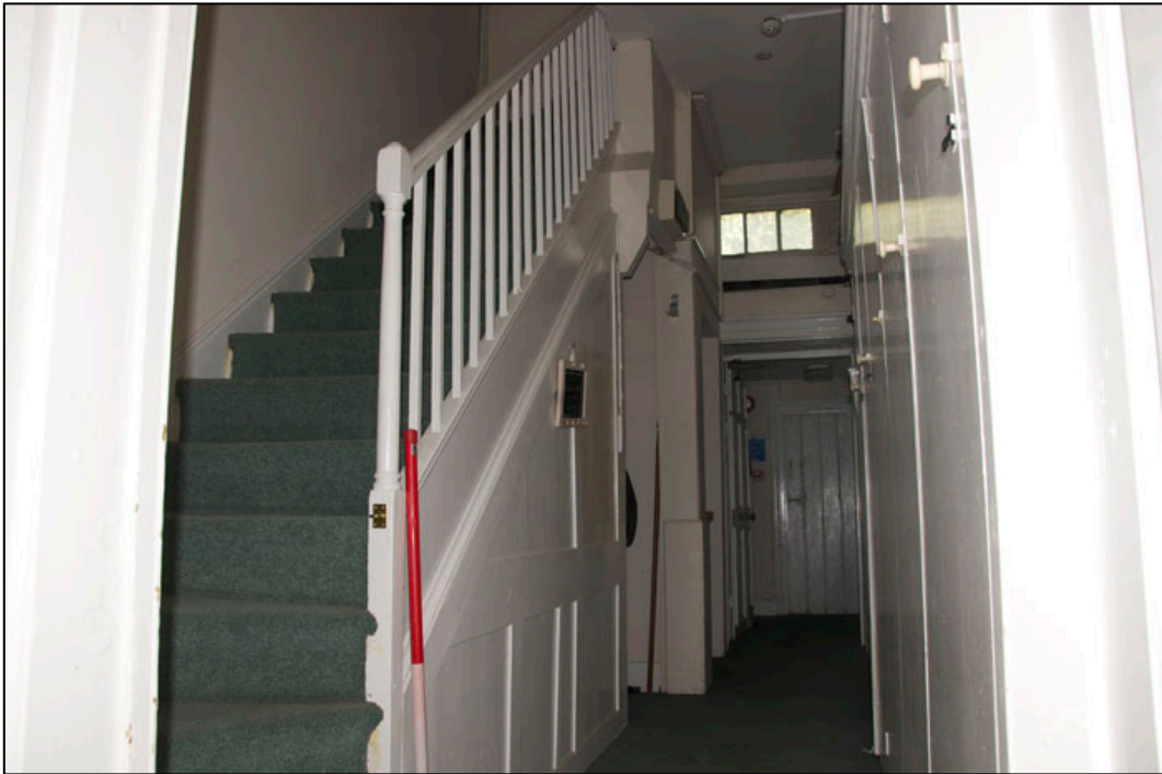
Appendix 3.11: General view of ground floor service staircase in Woodstock House HA1 (1m scale).
