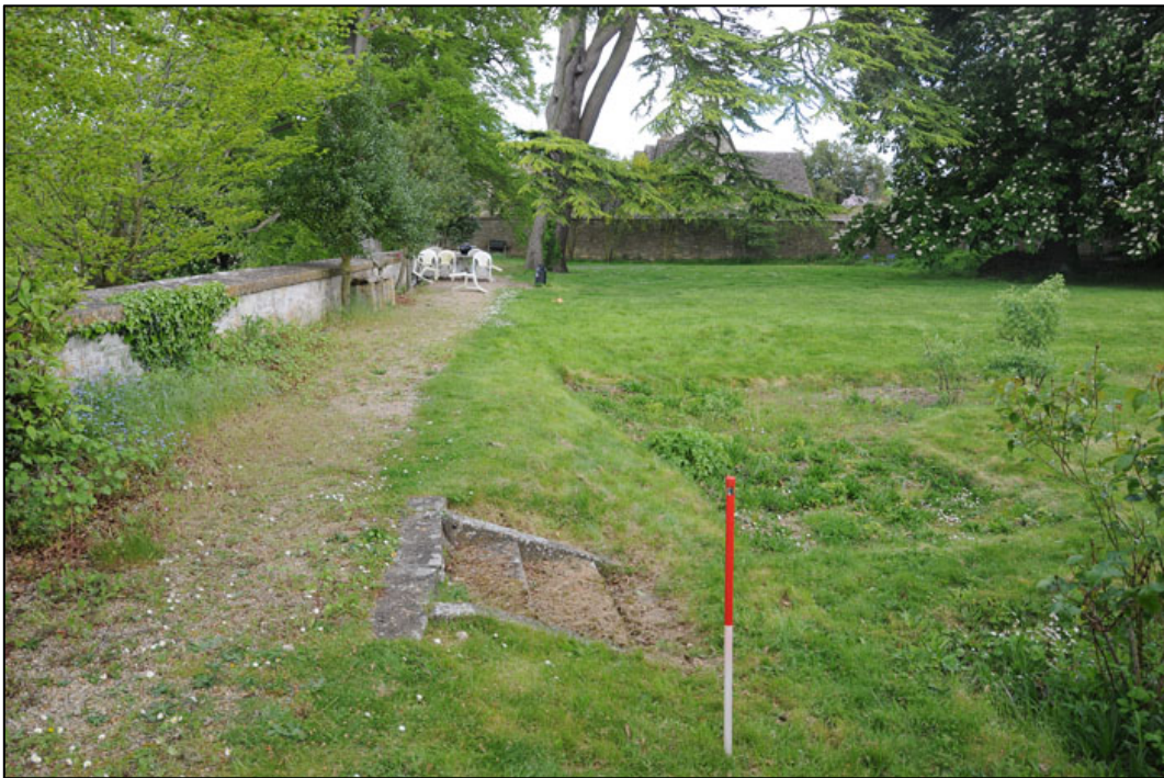
Appendix 3.52: General view of steps HA22 that provide access from the North Garden HA23 up to the terrace walk H20 , looking north (1m scale).
