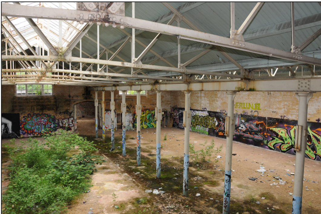
Appendix 2.31: General view of central columns in G6, looking northwest.
