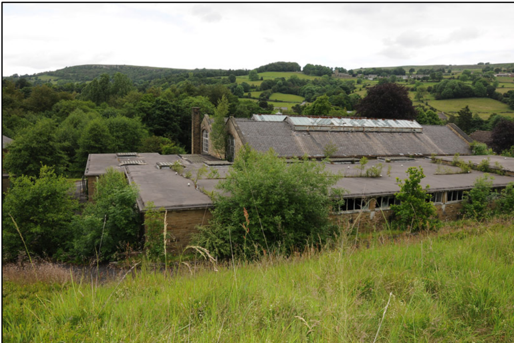
Appendix 2.2: General of roof scape of central section of Site, looking northeast.
