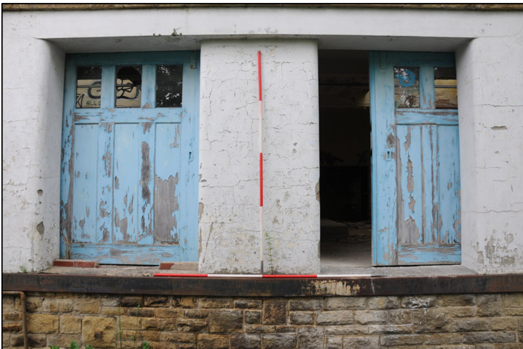
Appendix 2.10: Detail of sliding loading doors into rooms G11 and G12 (2m scale).
