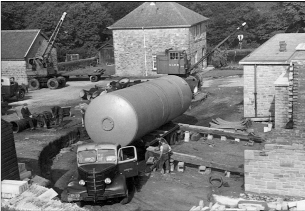
Figure 9: Photograph taken in 1954 during the installation of horizontal tanks in G13.
