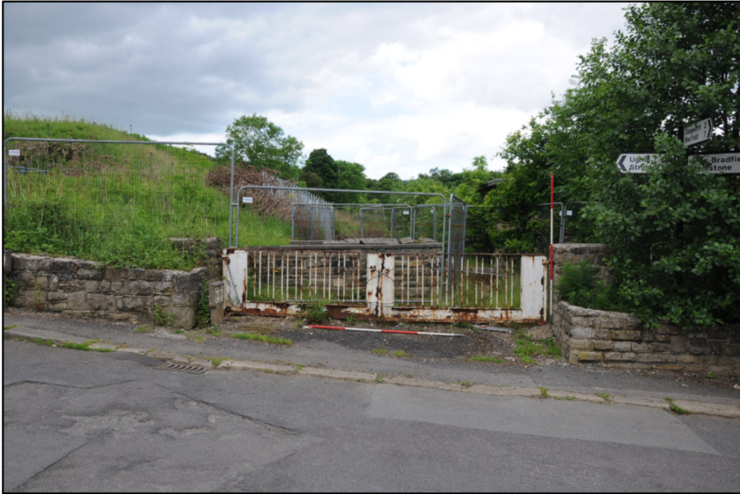
Appendix 2.5: Detail of south entrance that was blocked during decommissioning in 1994 (2m scale).
