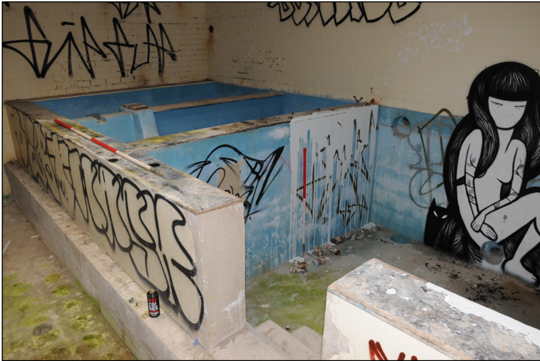
Appendix 2.27: General view of concrete tanks in G11 (1m/2m scale).
