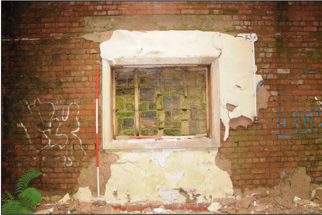
Appendix 2.19: General view of picture recess in north wall of G15 ; note earlier stonework (1m/2m scale).
