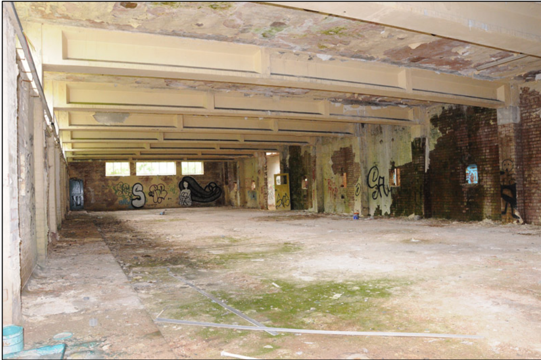
Appendix 2.23: General view of G13, looking west (2m scale).
