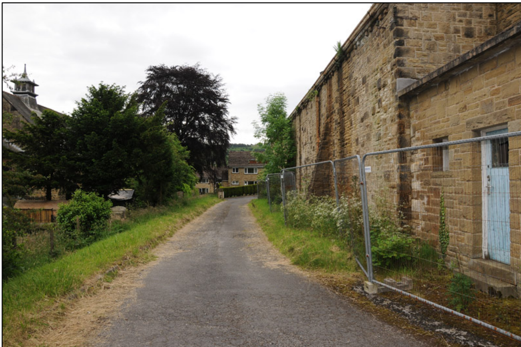
Appendix 2.8: General view along north elevation of Filtration Building, looking east.
