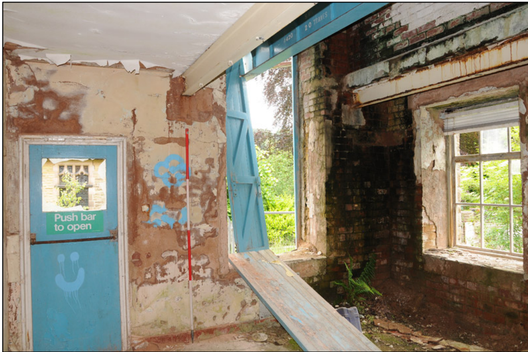
Appendix 2.38: General view of G1 , looking northeast; note inserted girder for hoist (2m scale).
