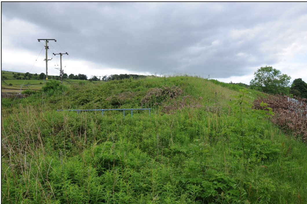
Appendix 2.16: General view of Covered Reservoir, looking west.
