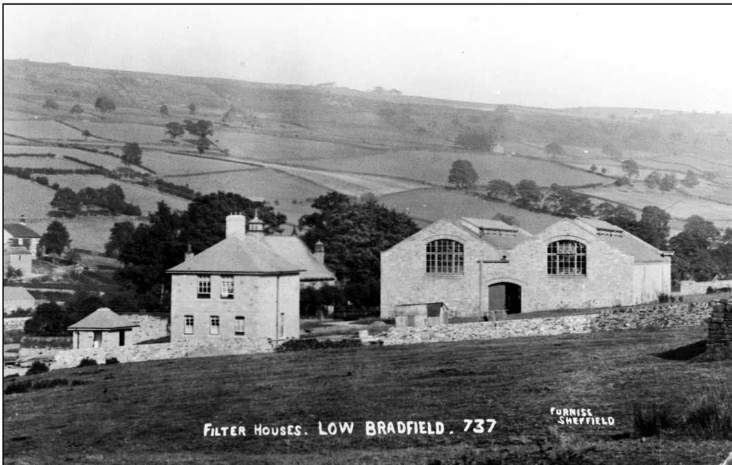
Figure 4: Photograph of filter houses at Low Bradfield following construction in 1913 © Picture Sheffield s11801 reproduced with permission.
