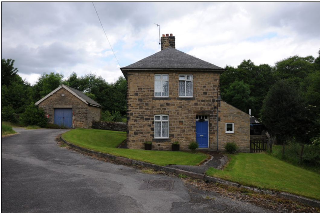
Appendix 2.14: General view of Garage and Caretakers House, looking west (2m scale).
