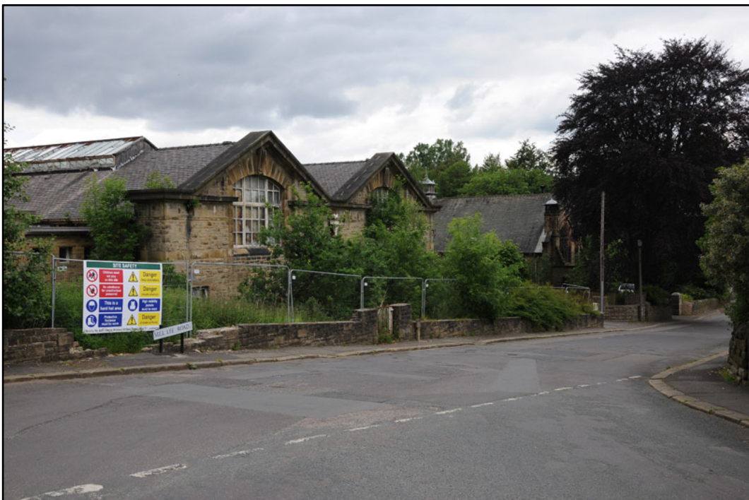
Appendix 2.4: General view of frontage, looking northwest along Mill Lee Road.
