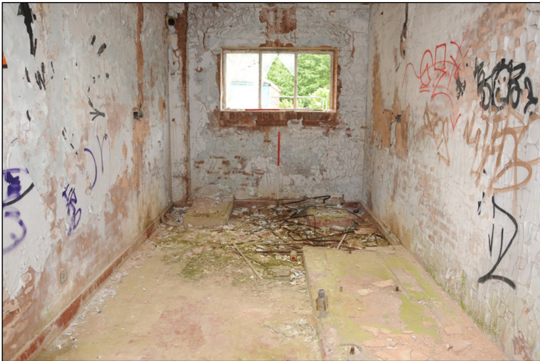
Appendix 2.28: General view of G9, looking west (1m scale).
