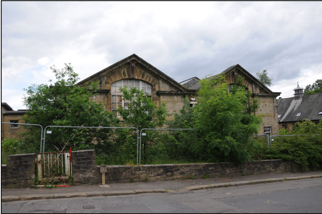
Appendix 2.3: General view of front elevation; note pedestrian gate (1m scale).
