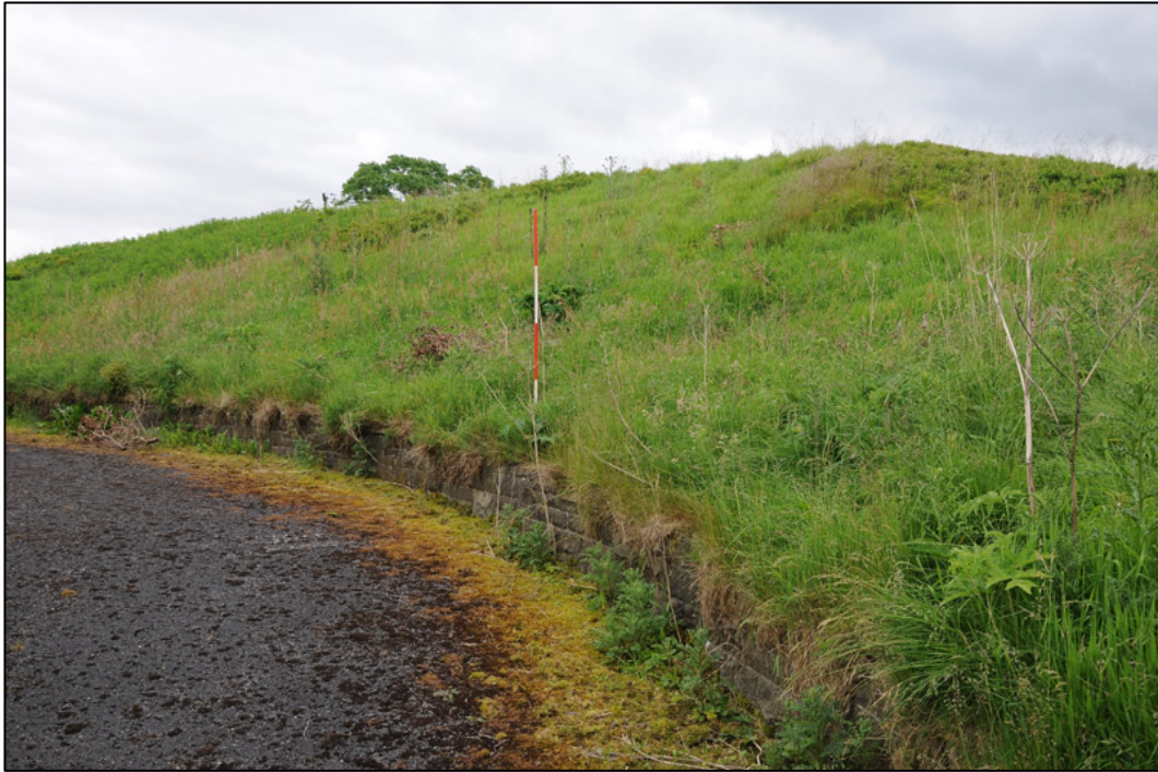
Appendix 2.15: General view of Covered Reservoir, looking southeast (2m scale).
