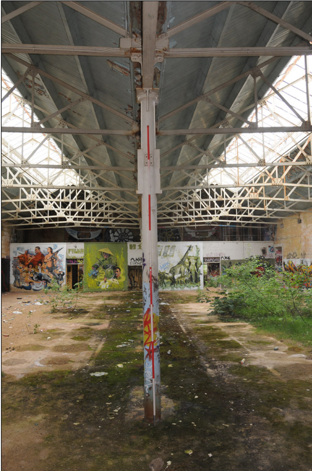
Appendix 2.29: General view of G6, looking east; note floor scars from removed filtration tanks (4m scale).
