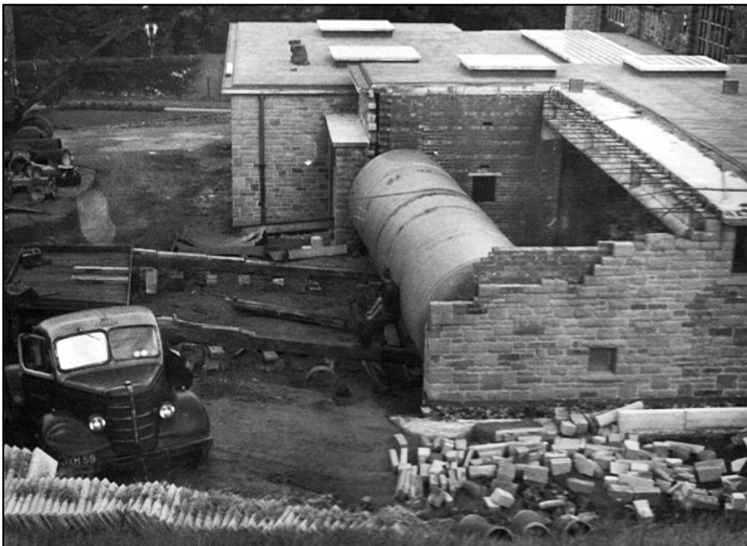
Figure 10: Photograph taken in 1954 during the installation of horizontal tanks in G13.
