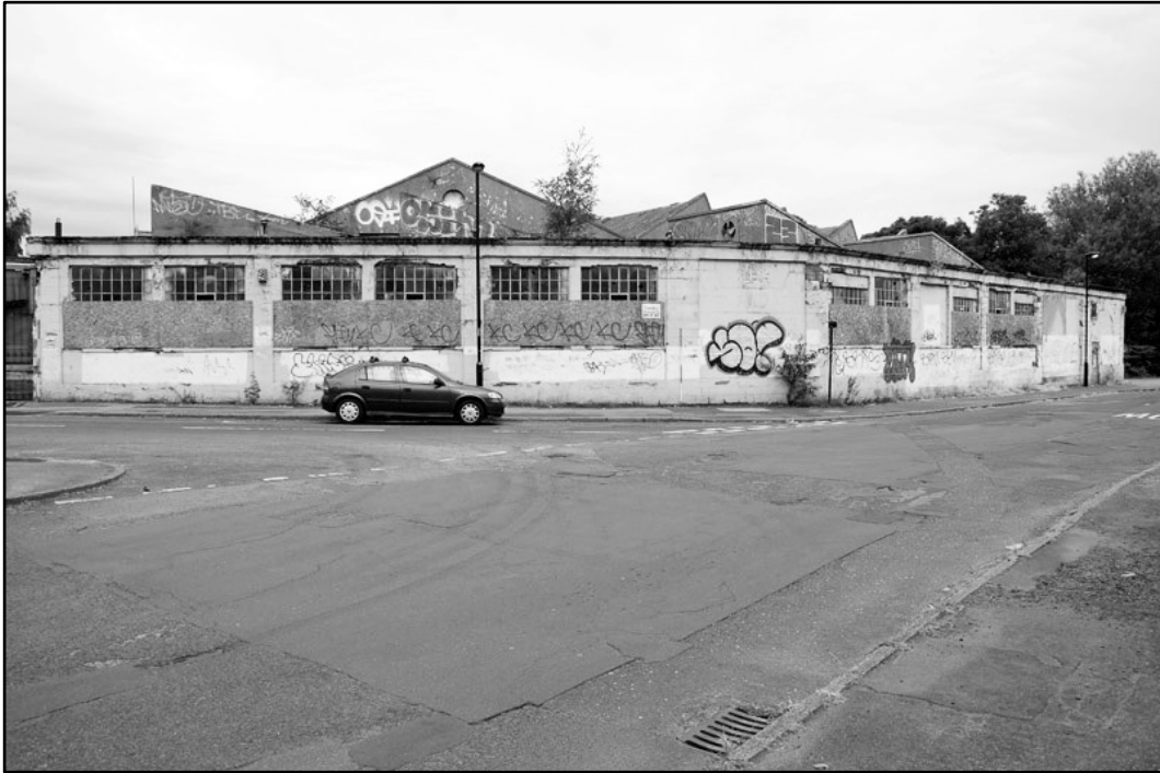
Appendix 4.5: General view of Little London Road Elevation, looking southwest; Film 1.6 (2m scale).
