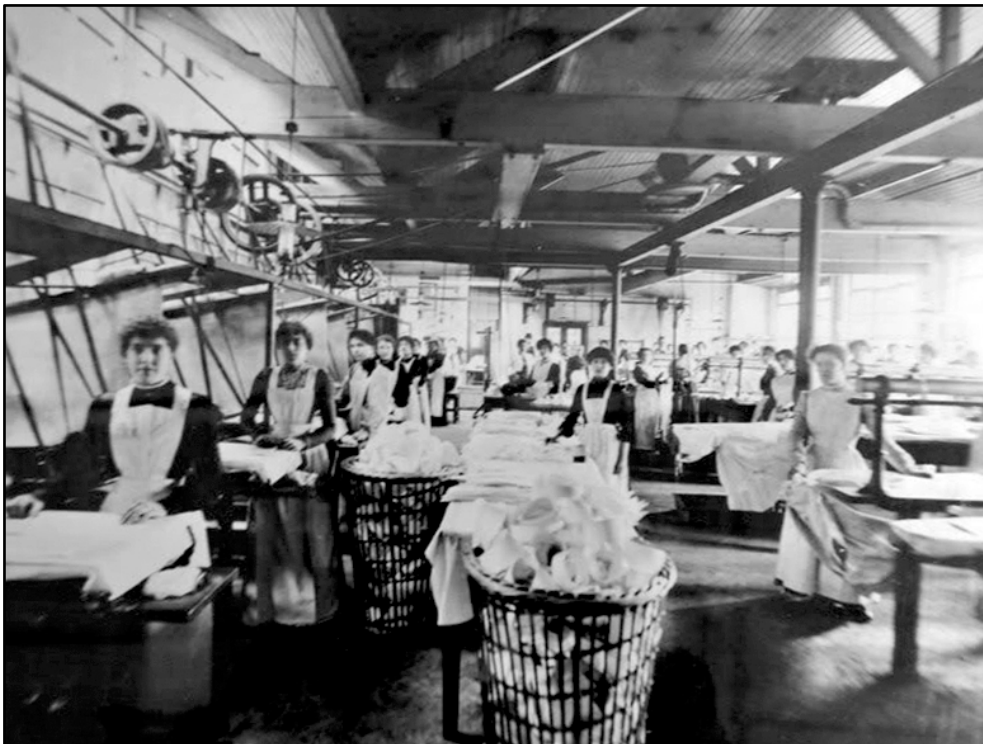
Figure 7: Early 20 th C photograph of the interior of the laundry; note line shafting and timber trusses.
