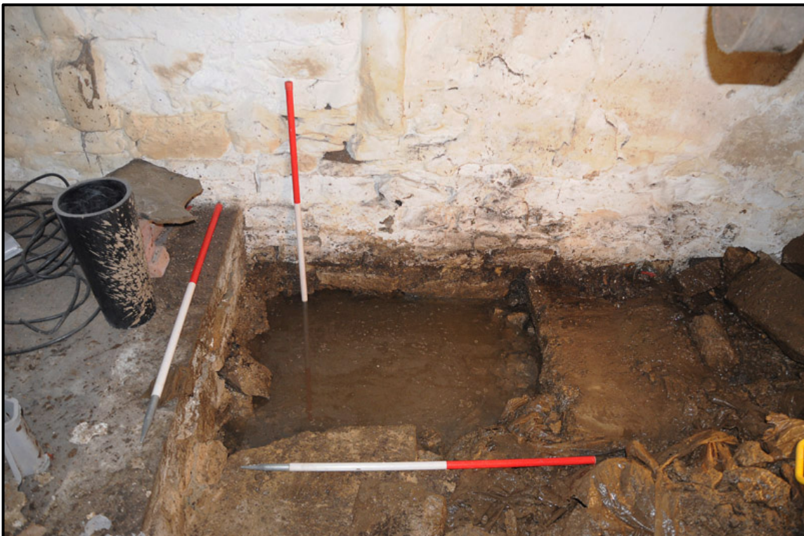
Appendix 3.2: General view of Trial Hole 1 after excavation, looking east (1m scale).
