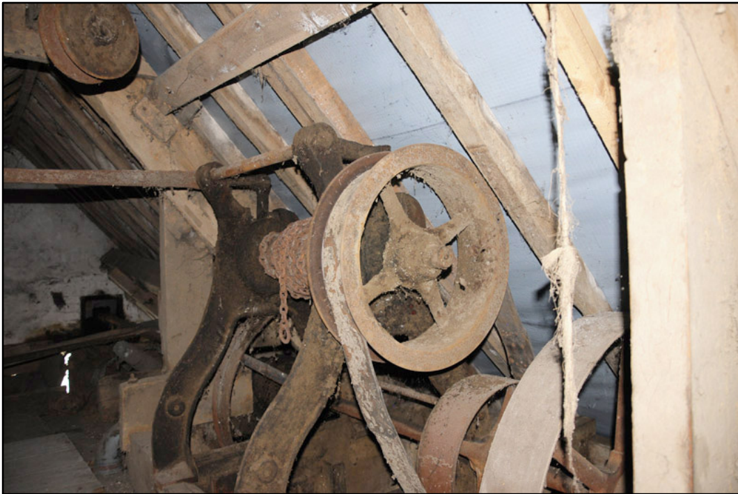
Appendix 5.36: Detail of hoist machinery on second floor walkway above the west range.
