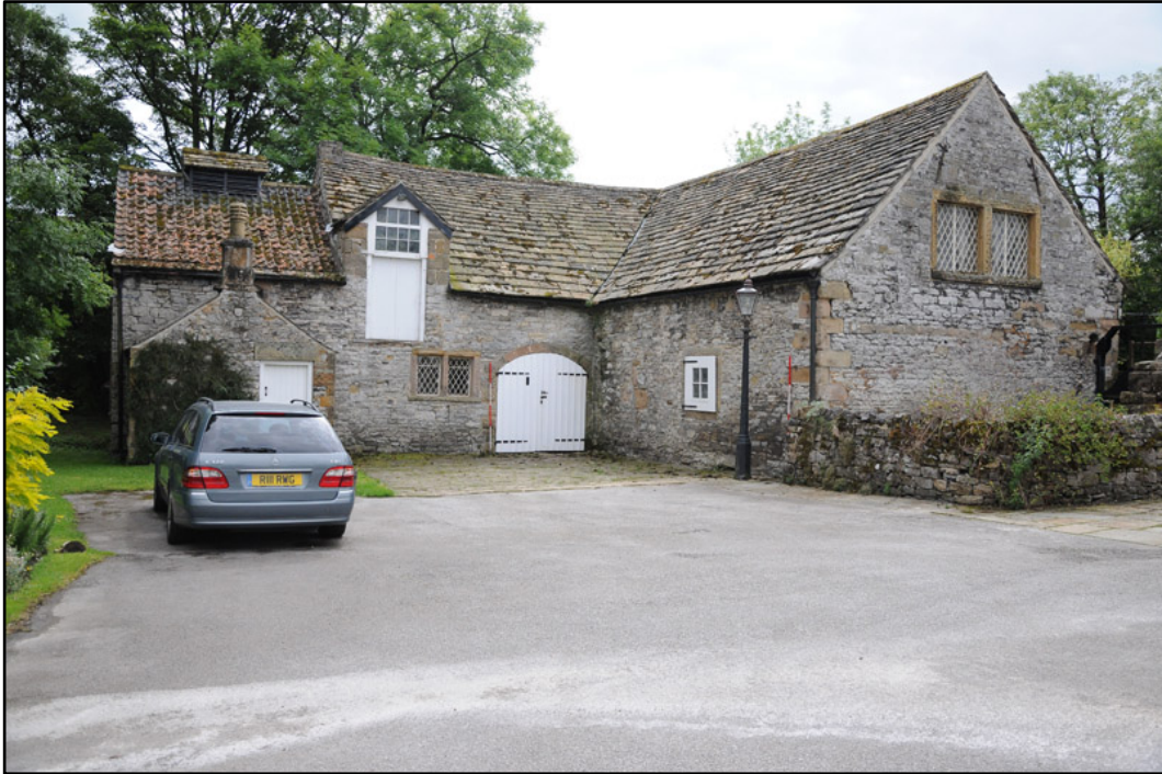
Appendix 5.1: General view of north elevation, looking southwest (2m scale).
