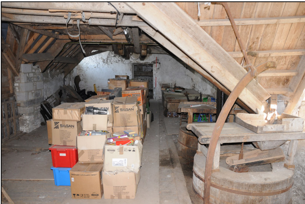
Appendix 5.27: General view of first floor of south range, looking west; note door to the kiln at the rear (2m scale).
