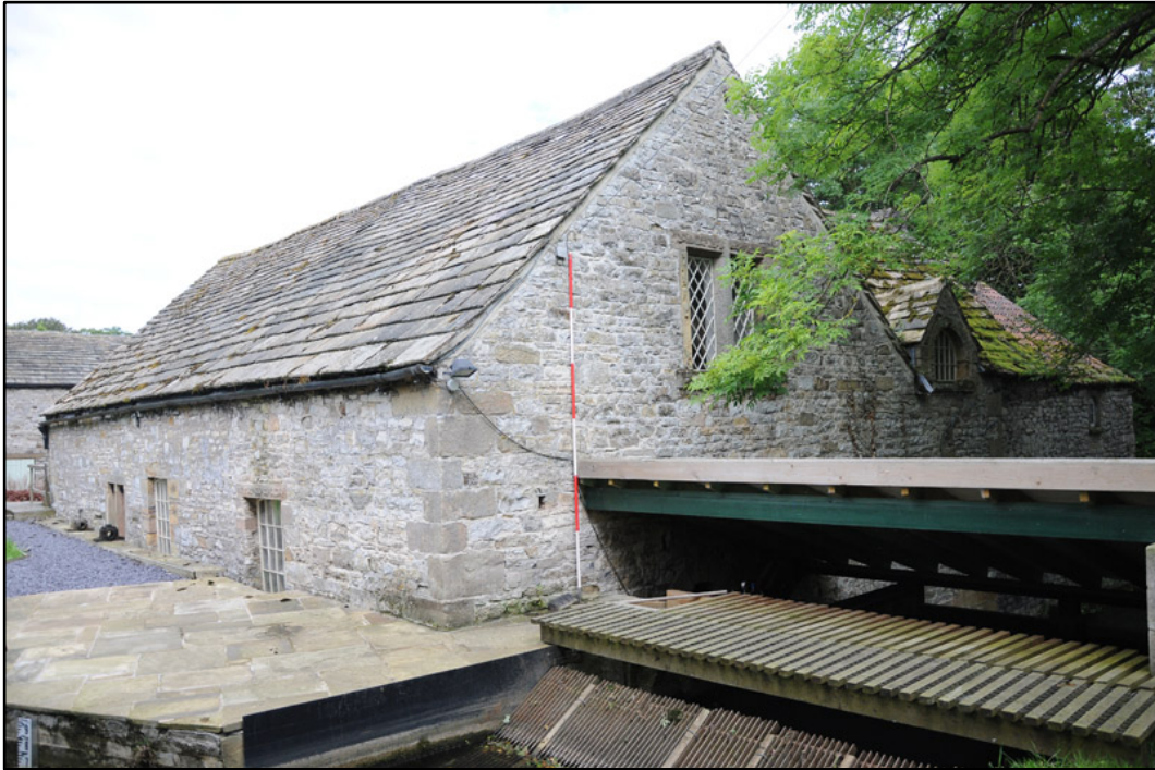
Appendix 5.7: General view of southwest corner of mill, looking northeast (3m scale).
