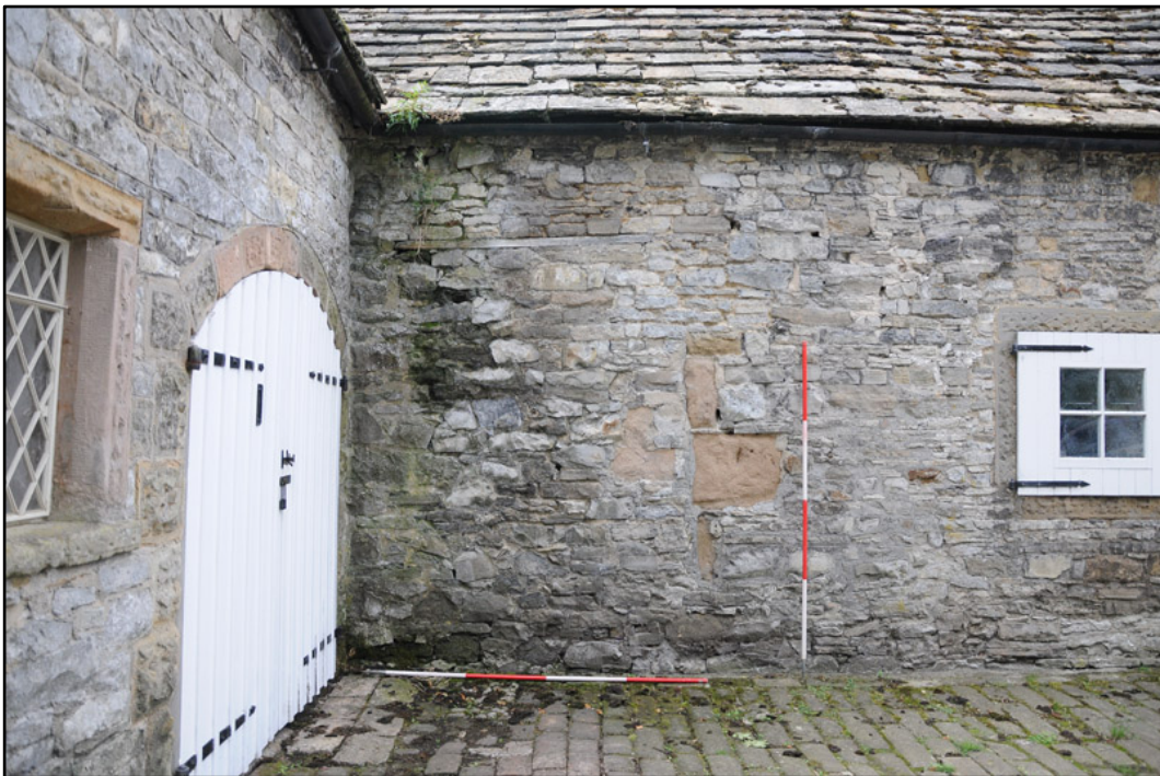
Appendix 5.4: Detail view of east elevation of courtyard, looking west; note quoins from earlier building (2m scale).
