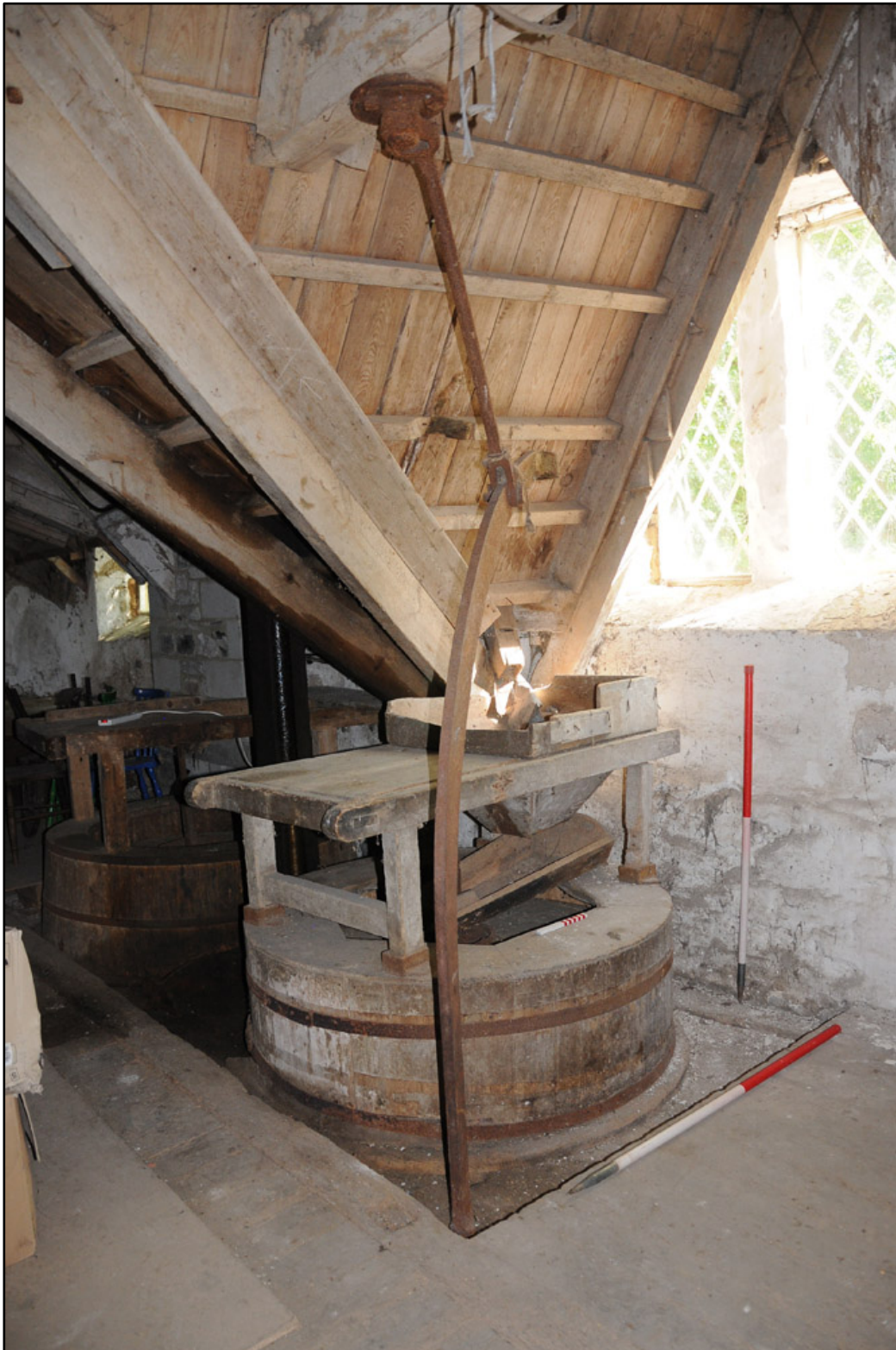
Appendix 5.30: Detail of in-situ mill wheel, hopper and crane on first floor, looking southeast (20cm/1m scale).
