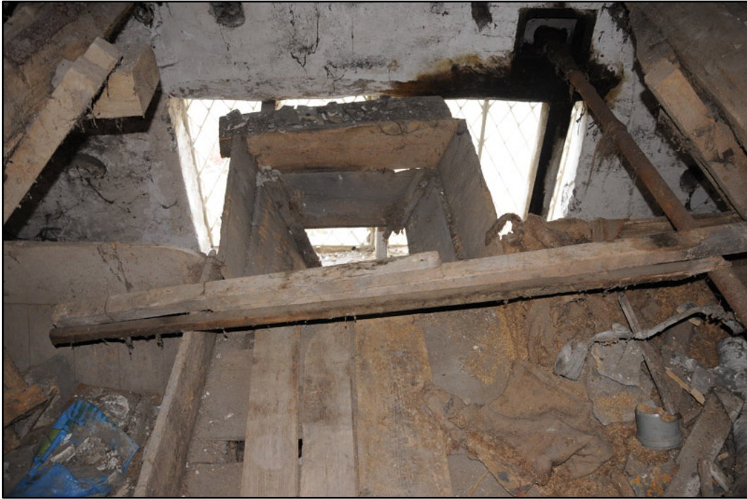
Appendix 5.35: General view of timber hopper on second floor walkway at north end of west range.
