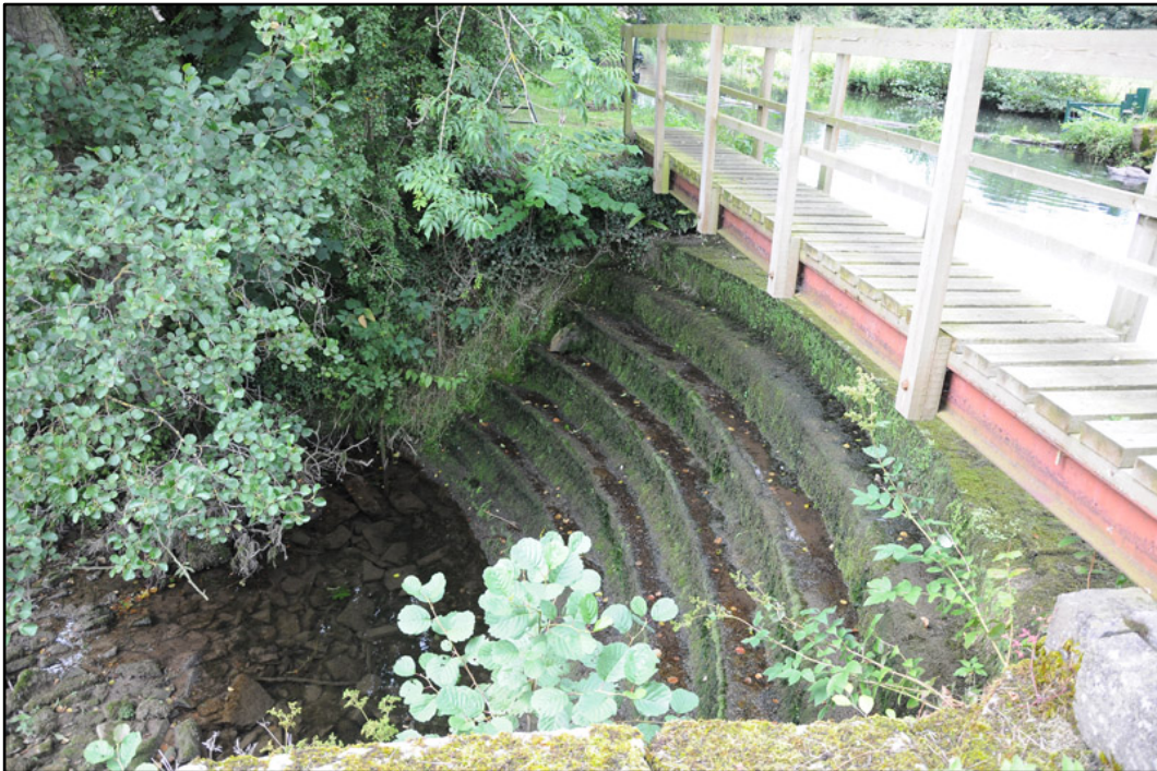
Appendix 5.14: Detail of stepped horseshoe weir between the south head race and the River Wye.
