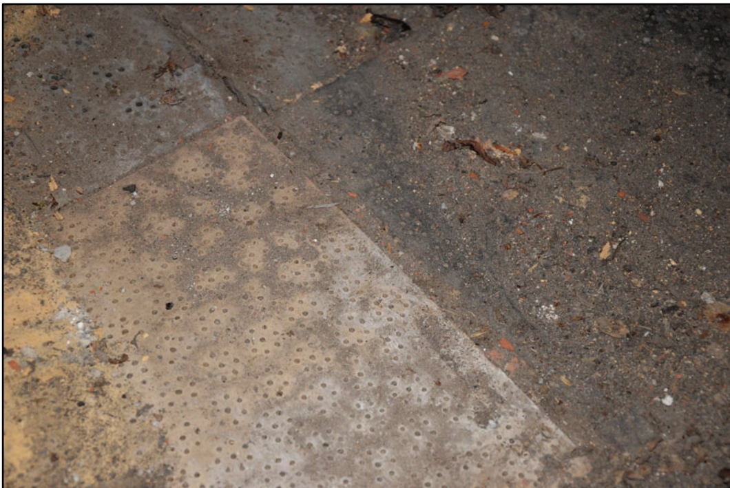
Appendix 5.29: Detail of perforated floor tiles from corn drying kiln on first floor.
