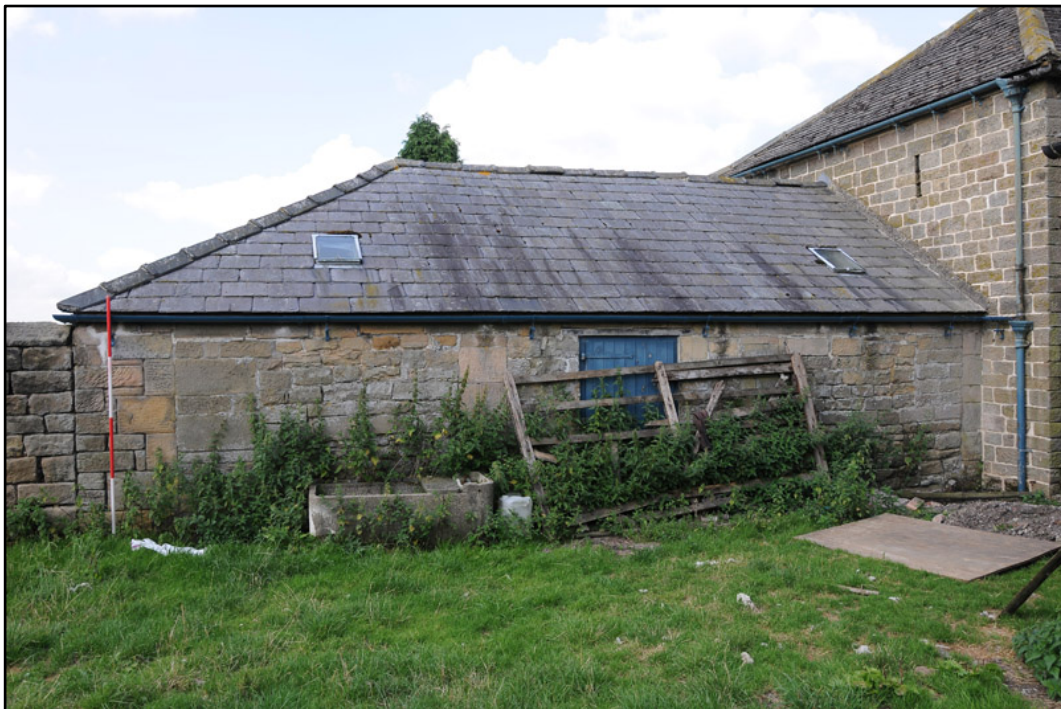
Appendix 5.31 General view of east elevation of G12 , looking west; note blocked openings (2m scale).
