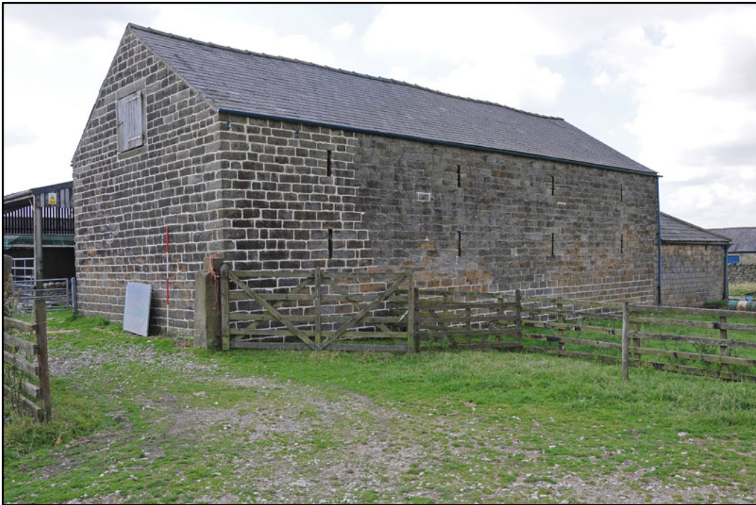
Appendix 5.36: General view of hay barn G16 , looking southwest; note first floor pitching door (2m scale).
