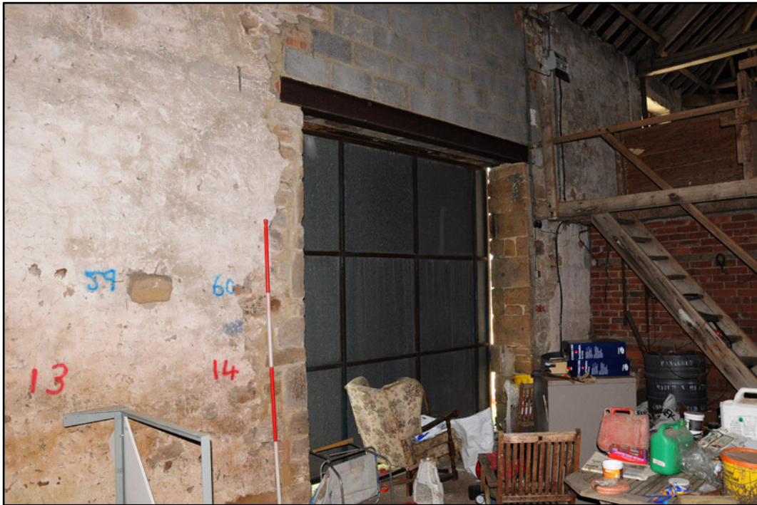
Appendix 5.26: Detail of altered doorway in west wall of barn G13 (2m scale).
