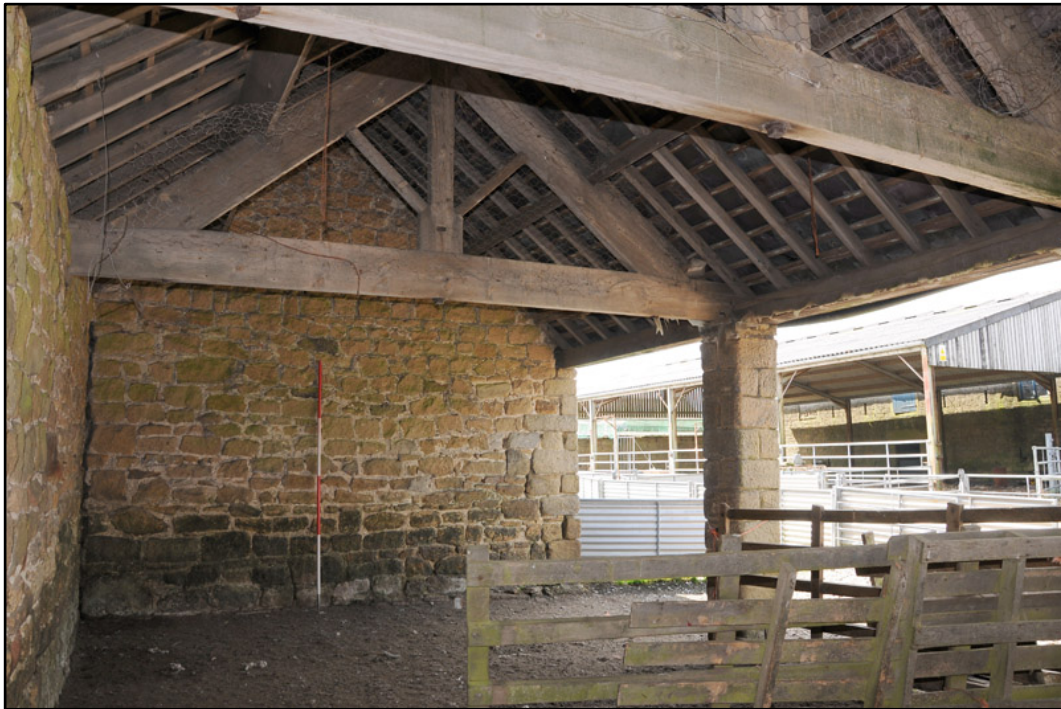
Appendix 5.40: General view of interior of G17 looking southwest; note kingpost roof (2m scale).
