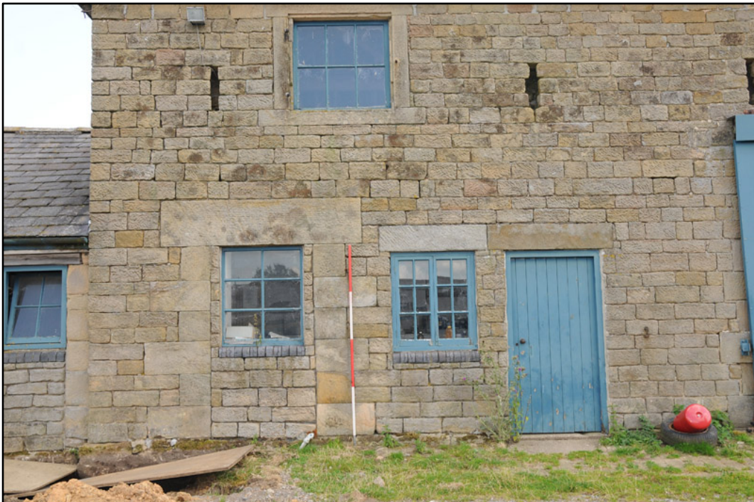
Appendix 5.22: Detail of northwest corner of G13/14 ; note alterations to doorway and windows (2m scale).
