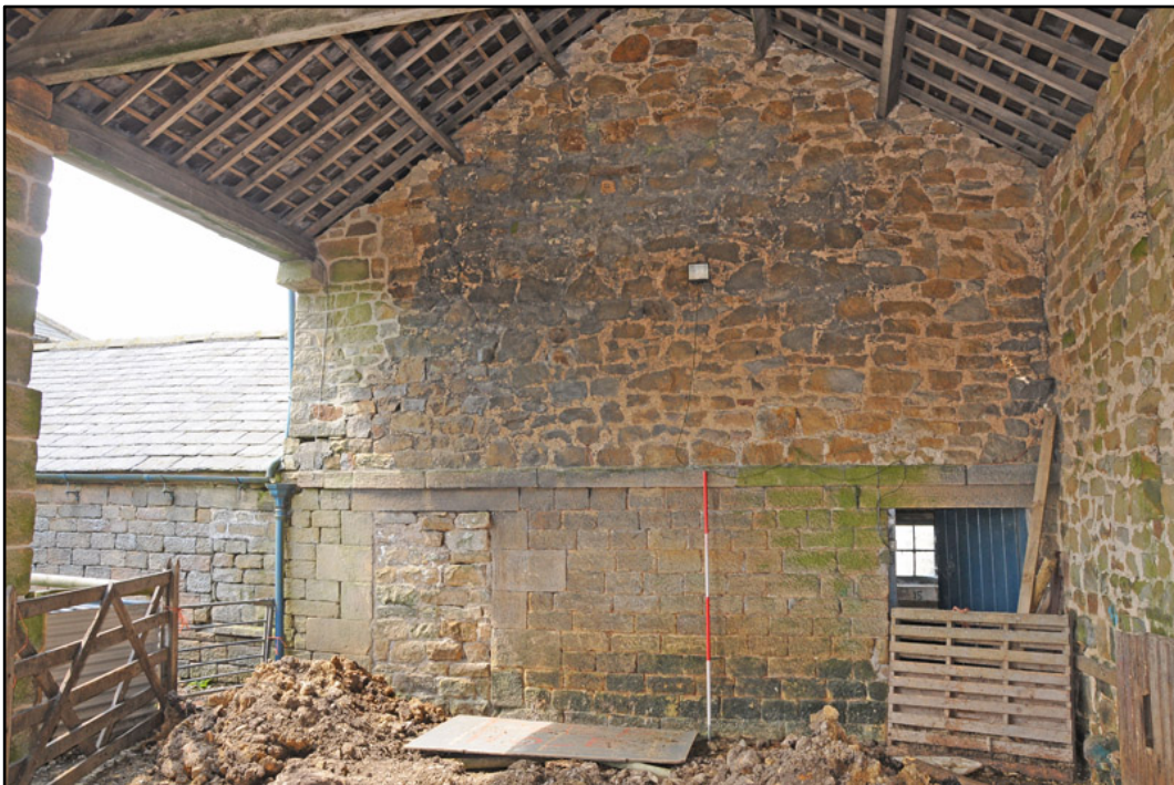
Appendix 5.20: Detail of internal west gable of G16 , built over G15 ; note blocked doorway (2m scale).
