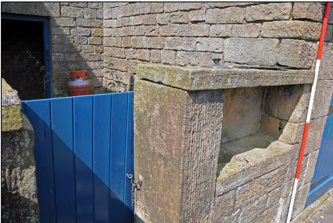
Appendix 5.14: Detail of pigsty G2 at south end of West Range; note feeding holes (2m scale).
