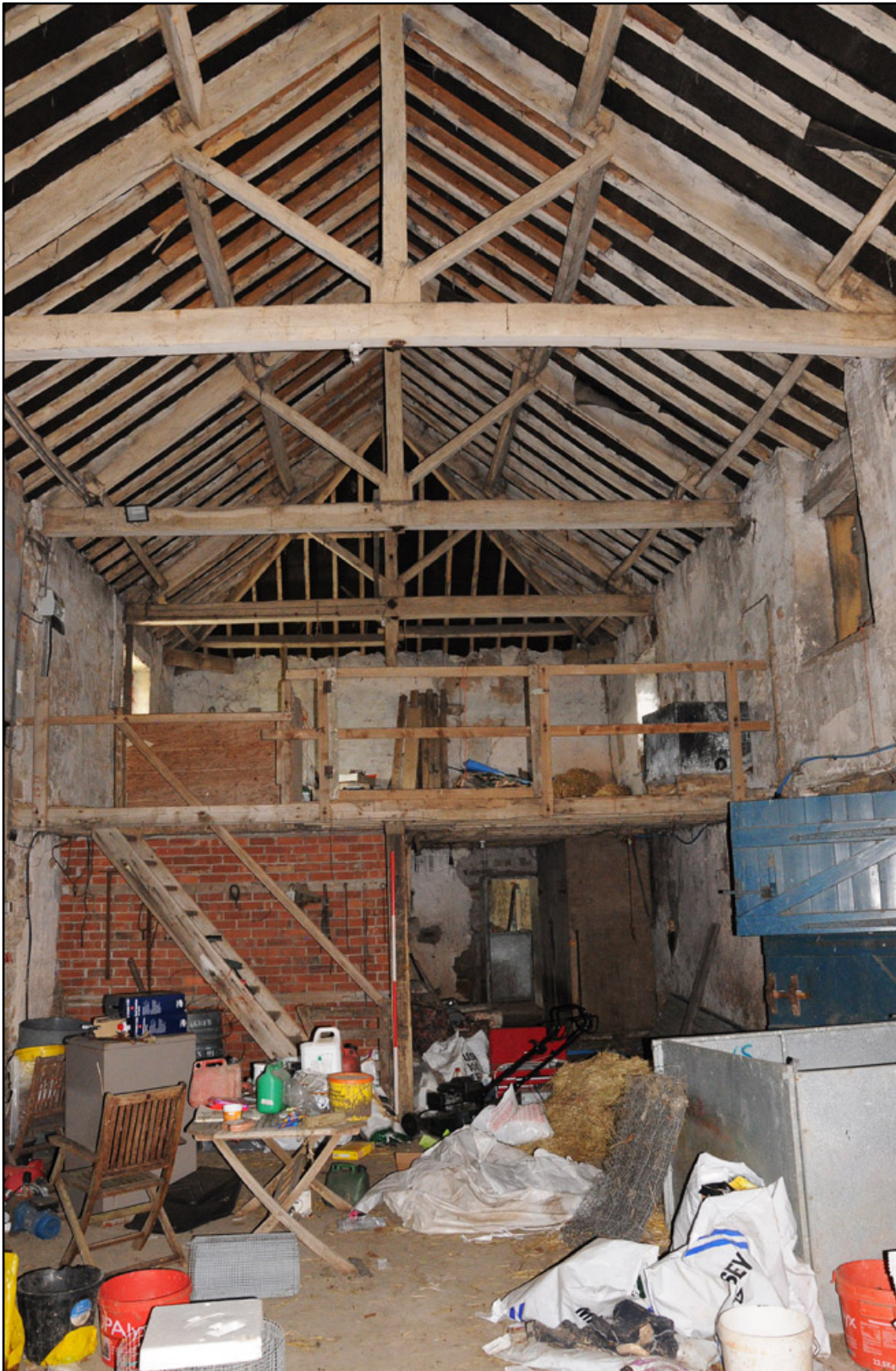
Appendix 5.25: Interior view of barn G13 , looking north; note secondary brick addition G14 (2m scale).
