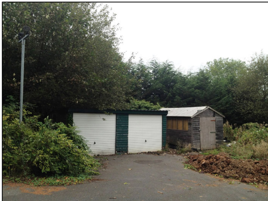
Modern timber garages and shed in southern section of Site, looking north.
