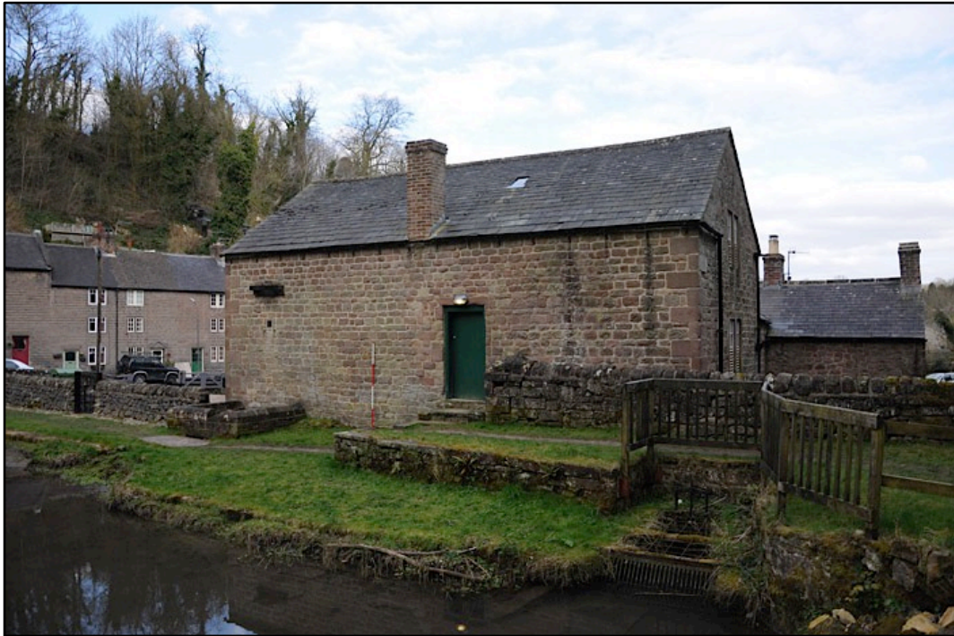
Appendix 3.3: West elevation of mill, looking southeast; note intake sluice to former water wheel (2m scale).
