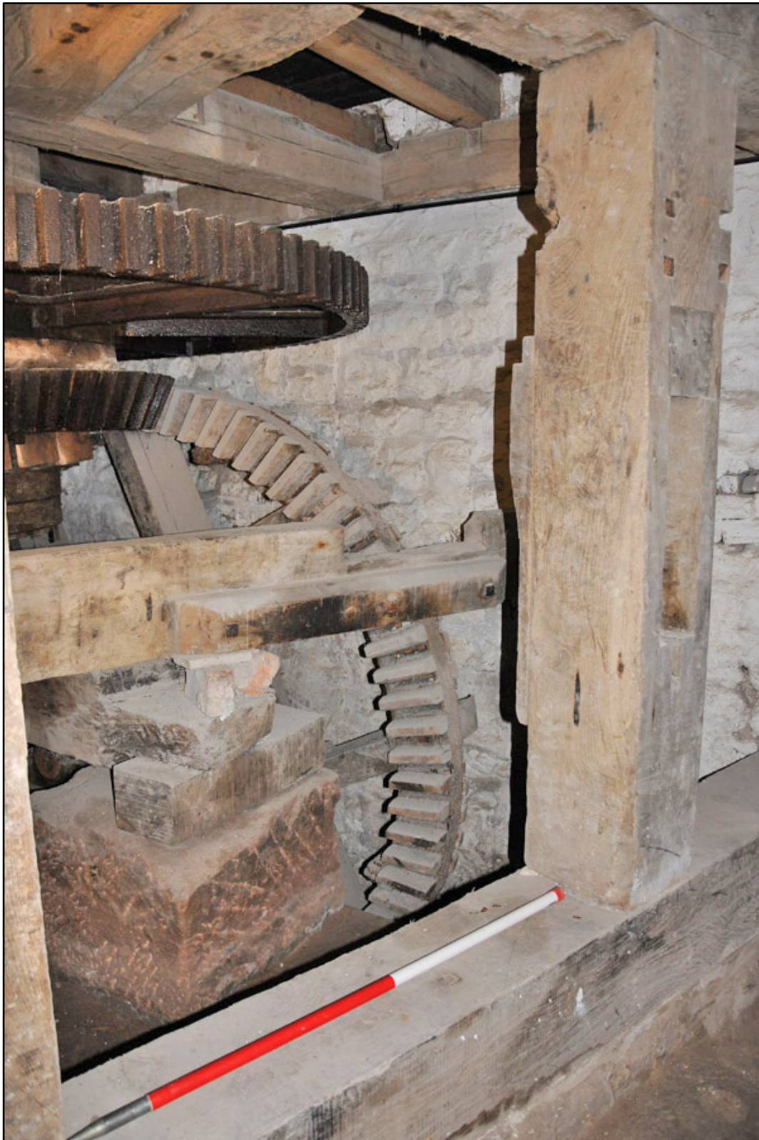
Appendix 3.9: Detail of modern insertion of mill machinery in G1, looking northwest (1m scale).
