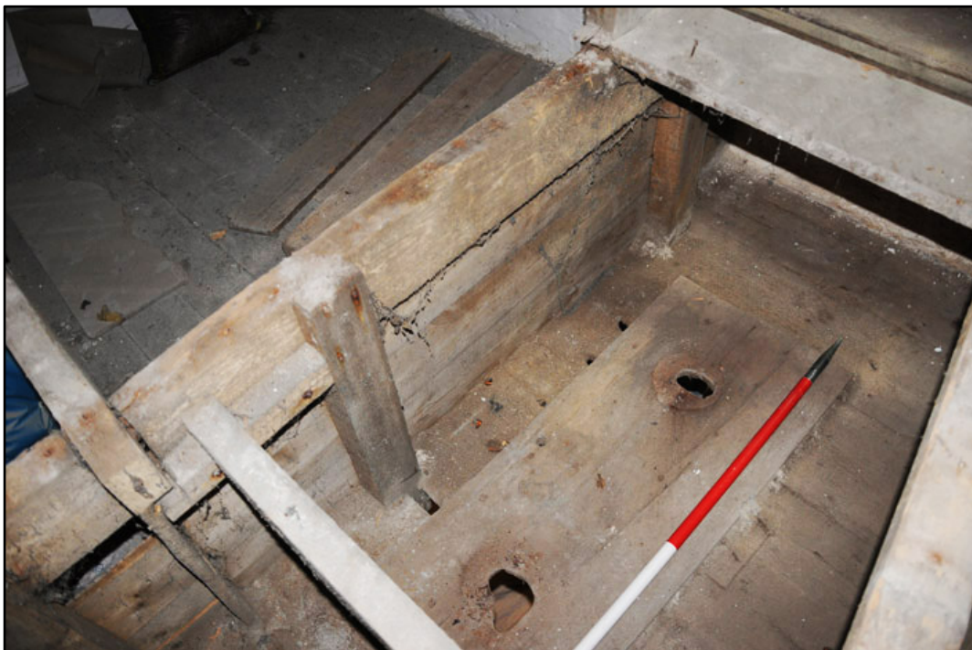
Appendix 3.32: Detail of holes in floor of T1 for the control ropes to operate the winch for the sack hoist (1m scale).
