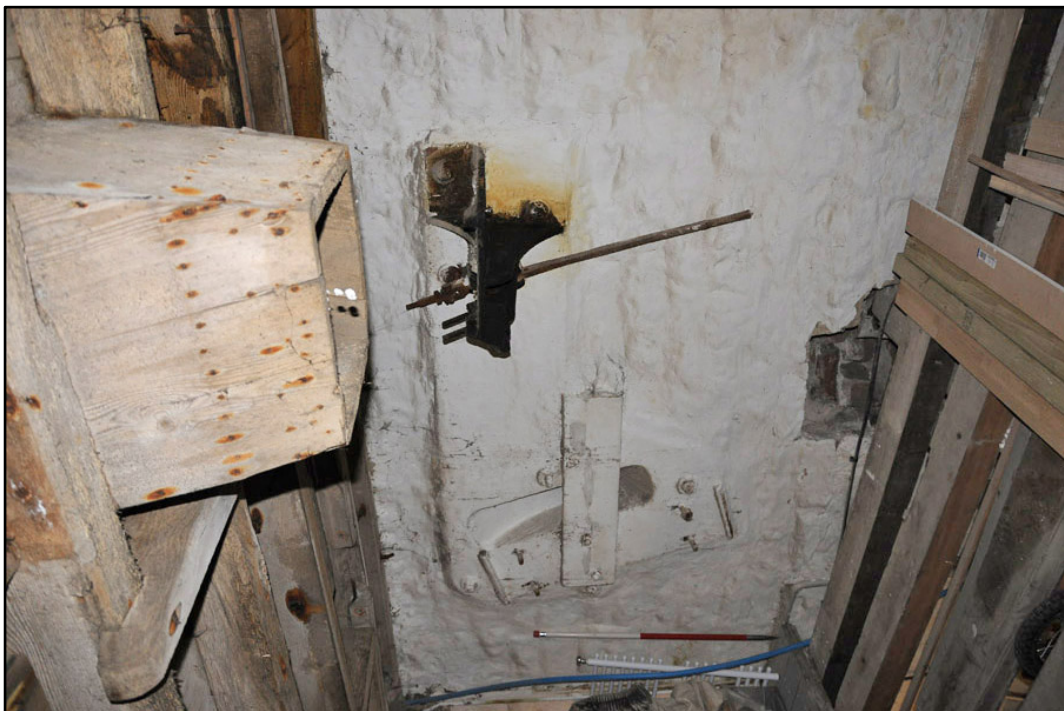
Appendix 3.19 Detail of hopper chute in ceiling and bevel gear mounting brackets in southeast wall of FI (1m scale).
