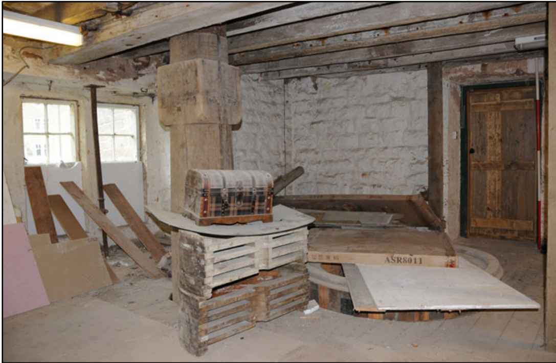
Appendix 3.14: General view of north end of FI; note modern floor and raised timber up-stand (2m scale).
