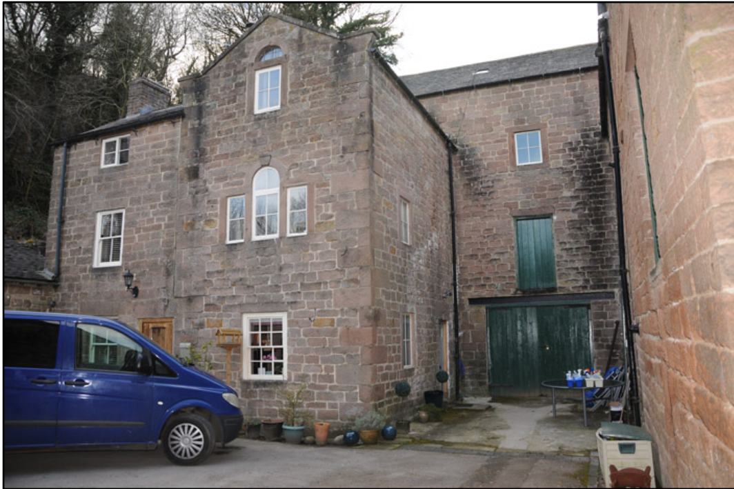
Appendix 3.7: General view of east yard and adjacent cottages to the left; note inserted double doors at ground level.
