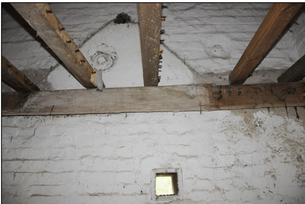
Appendix 3.29: Detail of timber lined slot in northwest wall of SI for former horizontal drive shaft (10cm scale).
