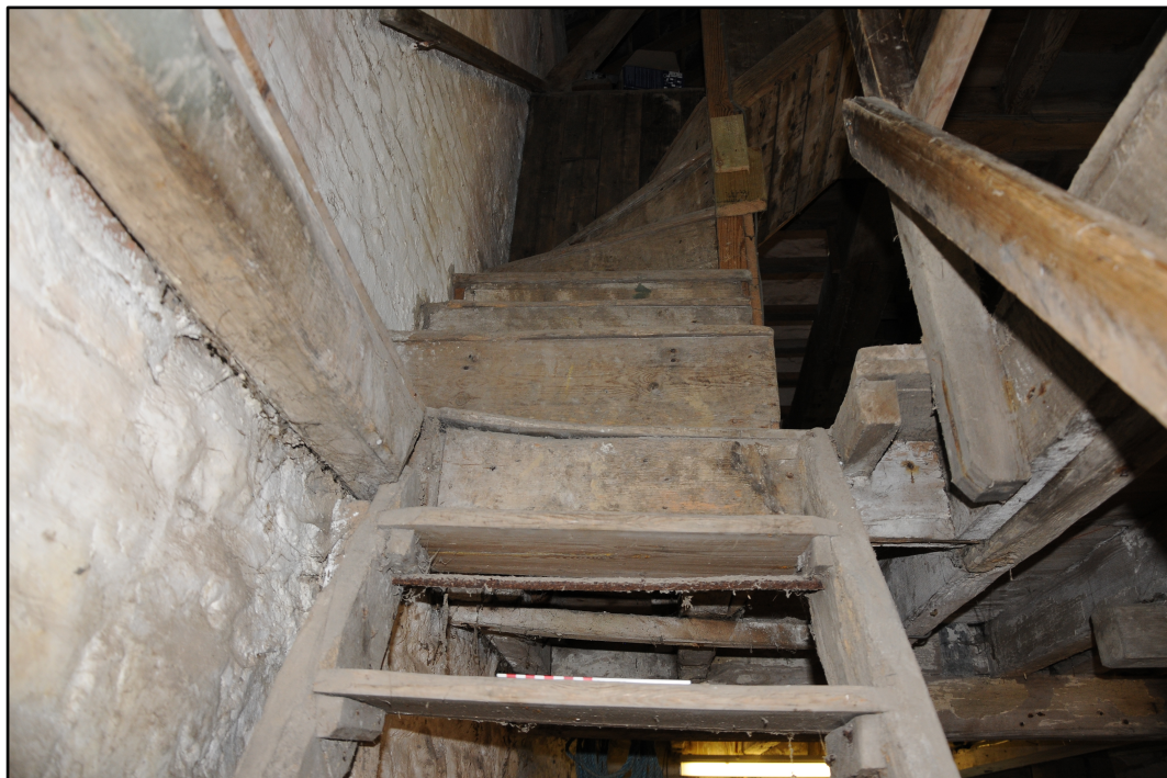
Appendix 3.15: Detail looking up winder stair against west wall of building between FI and SI (20cm scale).
