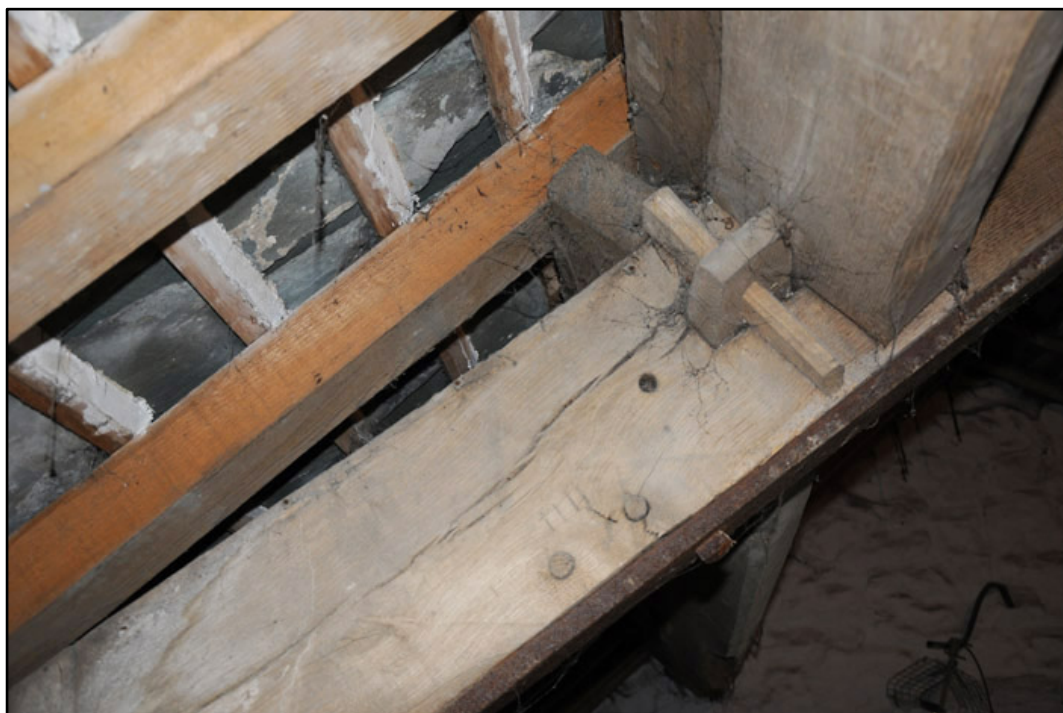
Appendix 3.34: Detail of assembly marks and fixing pegs on roof truss in T1; note through purlins.
