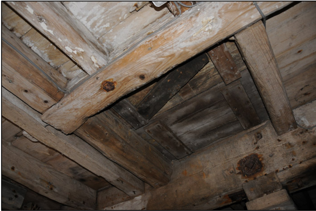
Appendix 3.20: Detail of underside of trapdoor in ceiling of F1.
