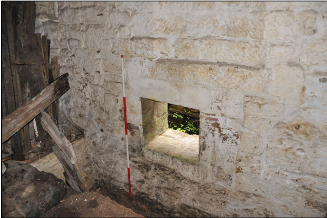
Appendix 3.12: Detail of recessed slot in floor for the pit wheel (removed) against south wall of G1 (2m scale).
