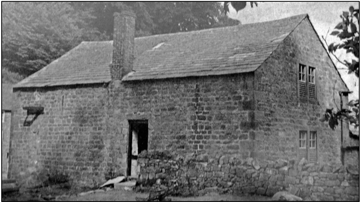
Appendix 2.3: External picture of the west elevation of the mill in 1971, after Derbyshire Life
