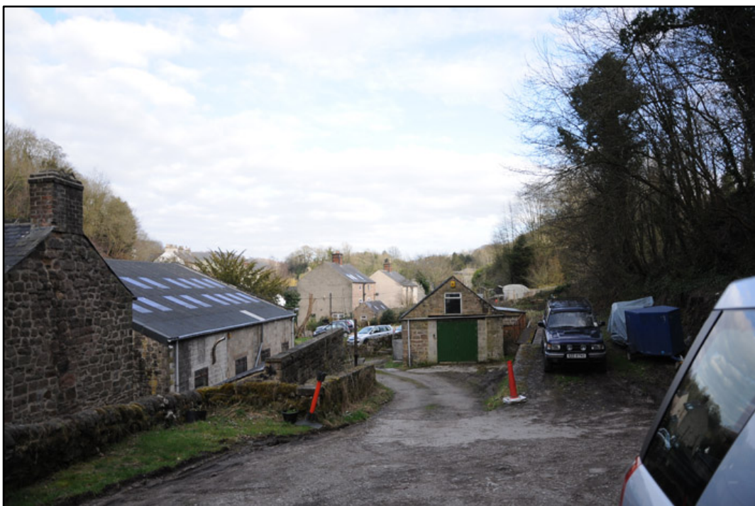
Appendix 3.2: General view of south access yard and outbuildings, looking east.
