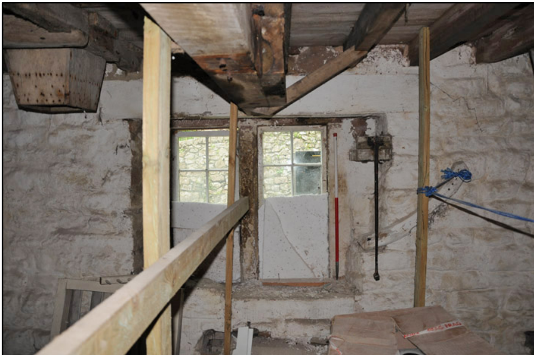
Appendix 3.21: Detail of south wall of F1; note lever for external pentrough and ceiling mounted grain chute (1m scale).
