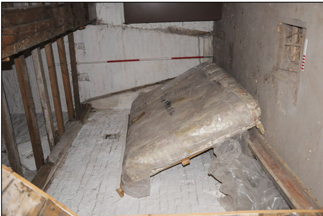
Appendix 3.27: Detail of scar of former grain chute in northwest corner of S1, and floor opening (20cm/1m scale).
