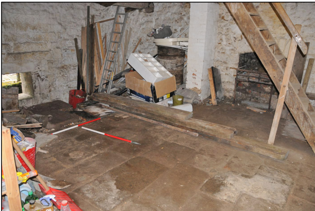
Appendix 3.11: General view looking west of flagstone floor in GI; note opening for water wheel axel in rear wall (1m scale).
