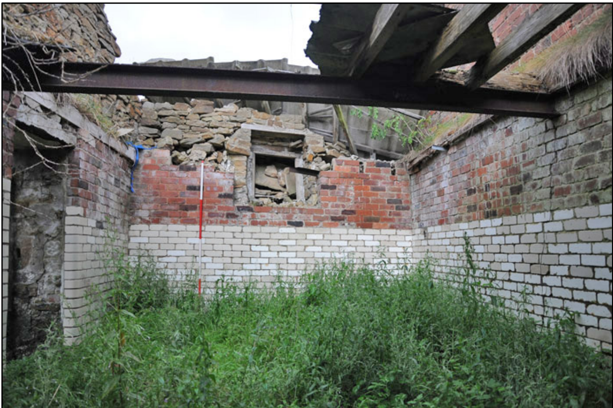
Appendix 3.18 General view looking north of room G5 ; note glazed tiles and high level window (2m scale).
