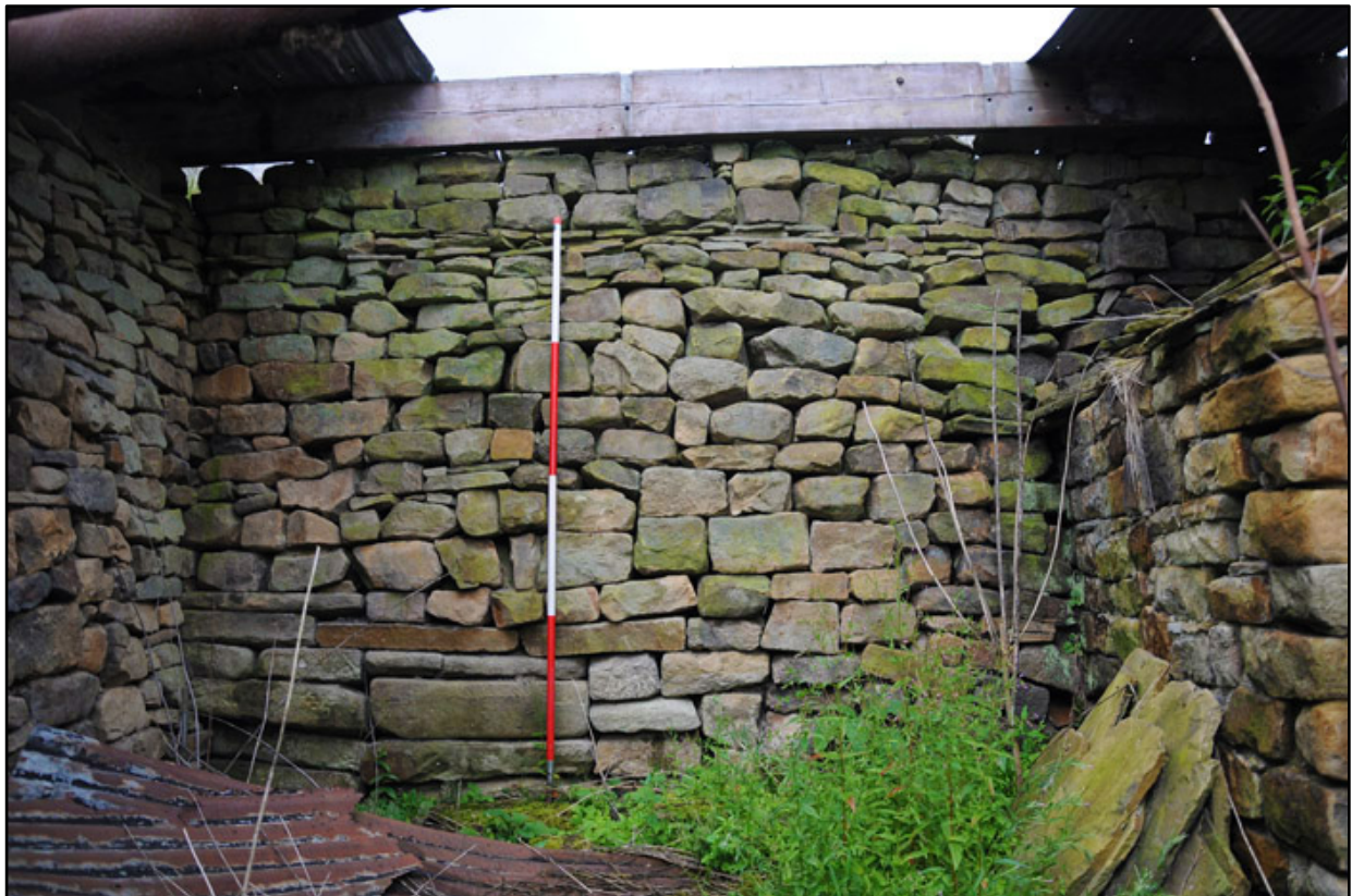
Appendix 3.22: General view of covered yard G8, looking north (2m scale).
