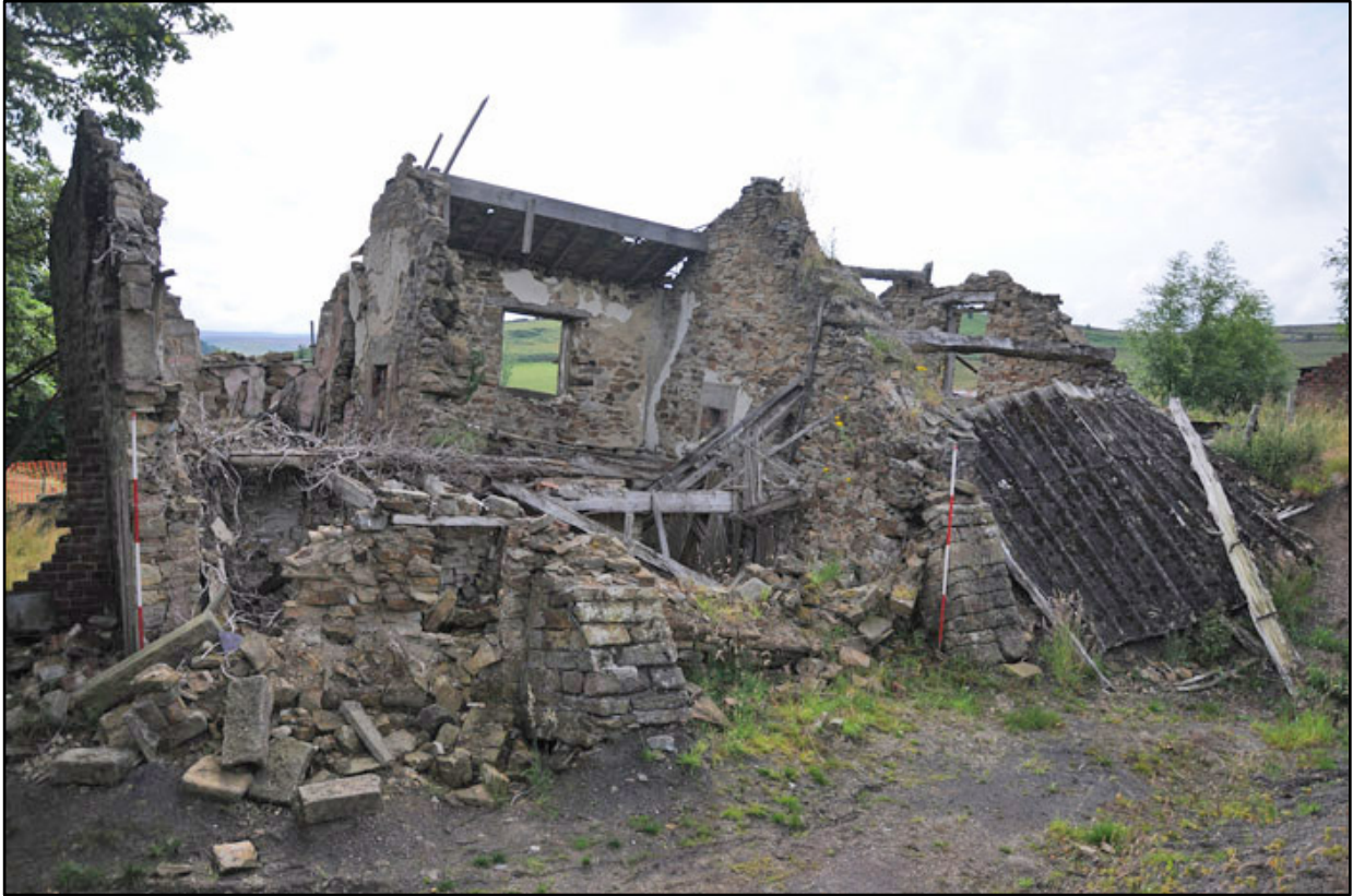
Appendix 3.11: General view of former north elevation of Smelters Cottage, looking south; note added buttresses (2m scale).
