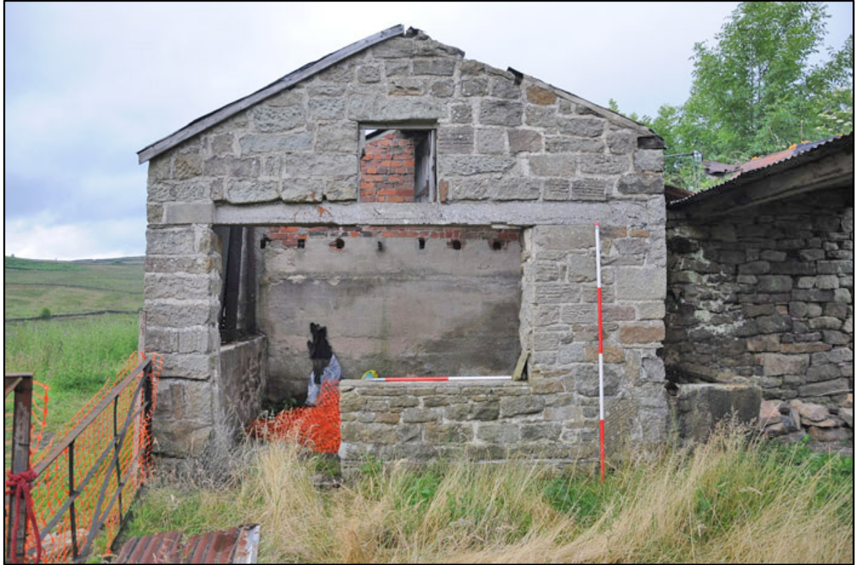
Appendix 3.19: General view of extended out-building G9 , looking west (2m scale).
