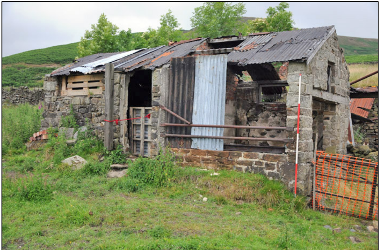
Appendix 3.20: General view of out-building G10 , with extension G9 (2m scale).
