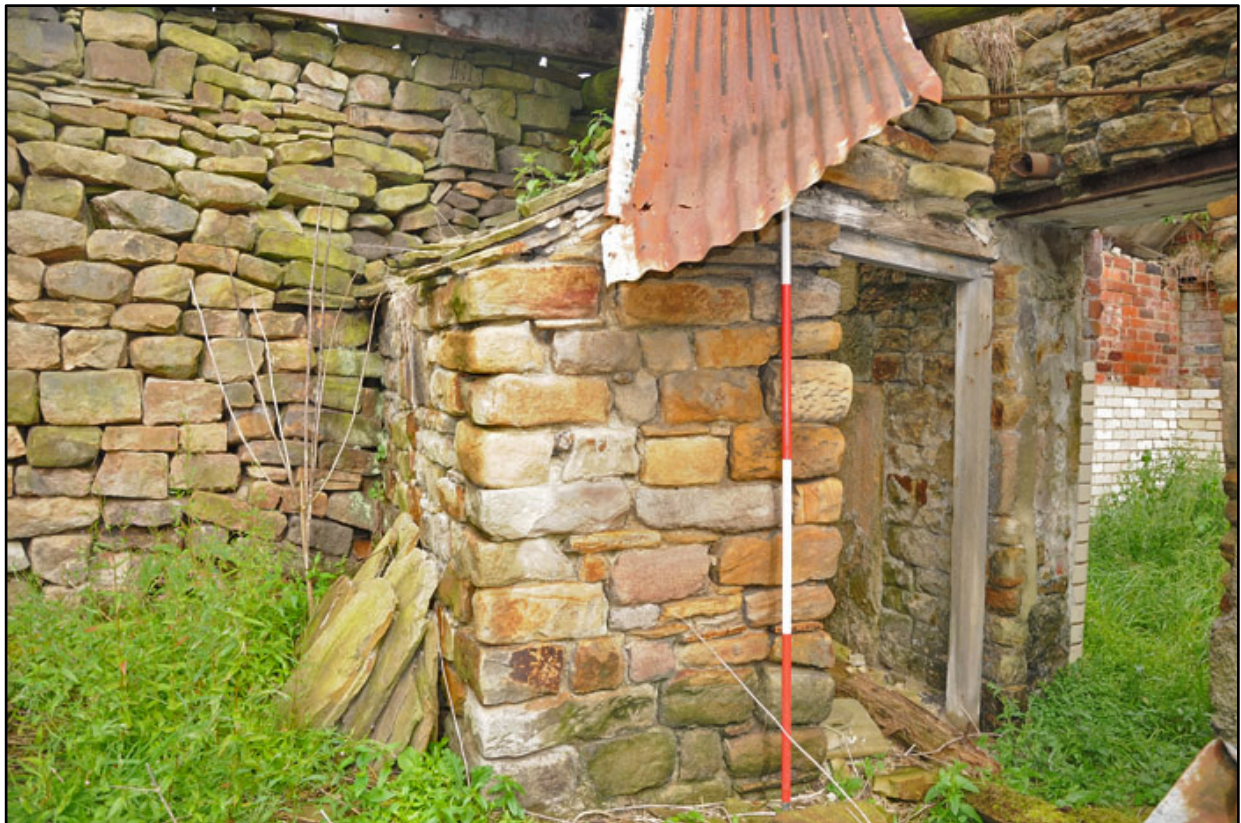
Appendix 3.16: Detail of toilet (privy) G7 (2m scale).
