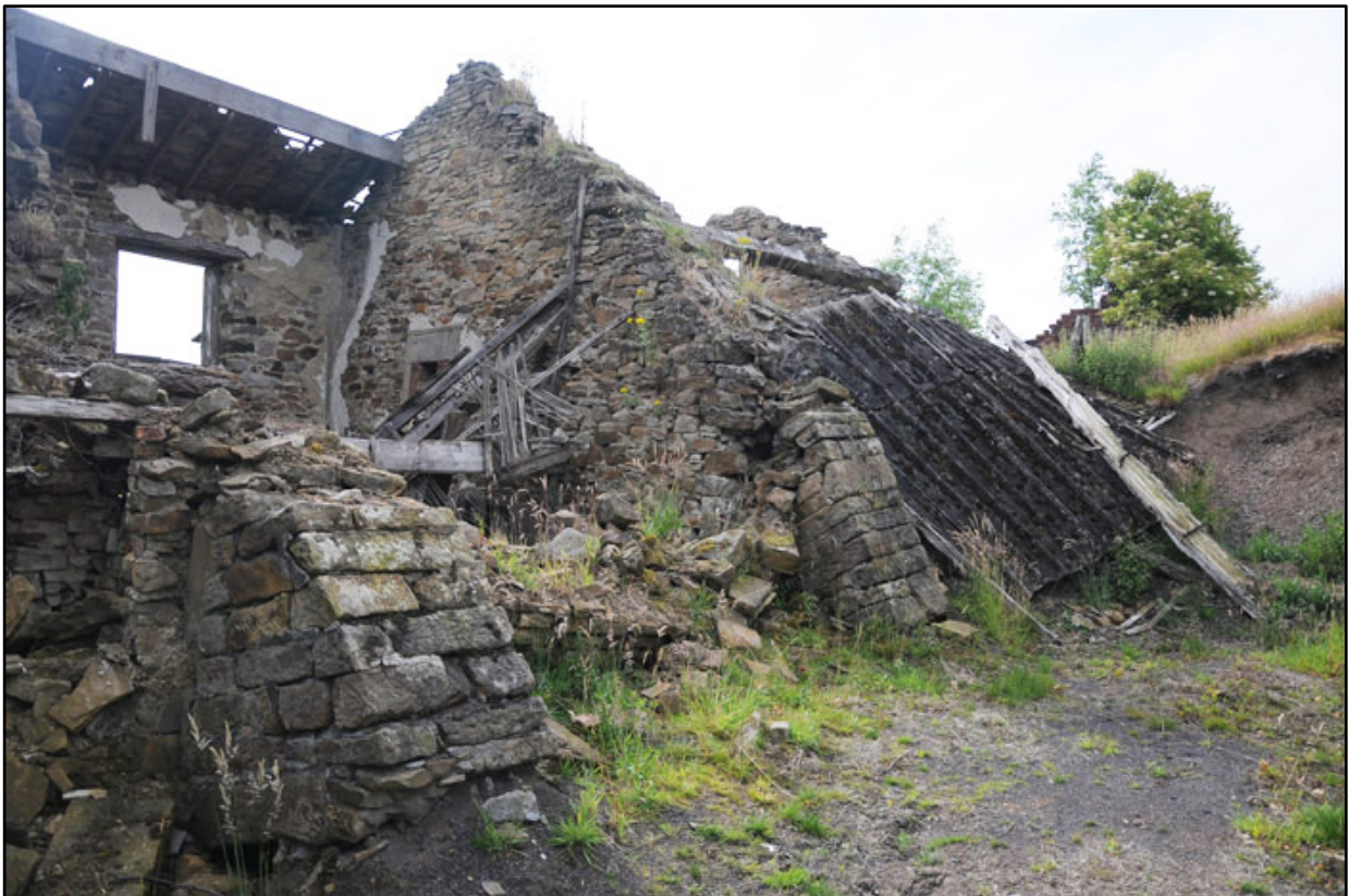
Appendix 3.12: Detail of upper floor room F2, looking southwest.
