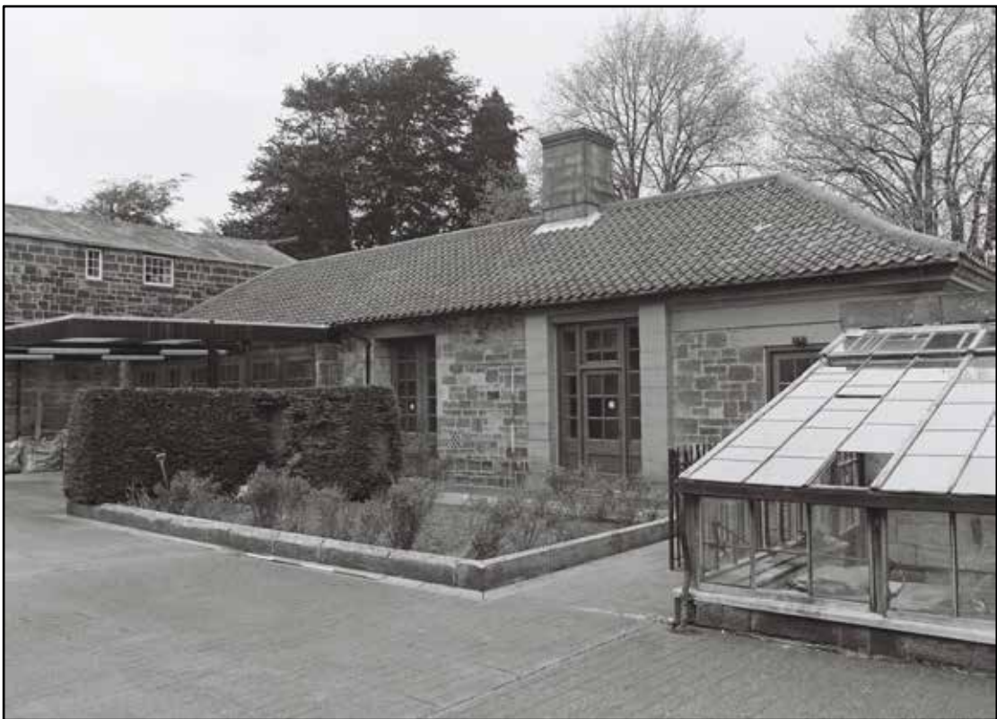
Appendix 5.237: Detail of south elevation of motor house (2m scale) (Film 10.09)
