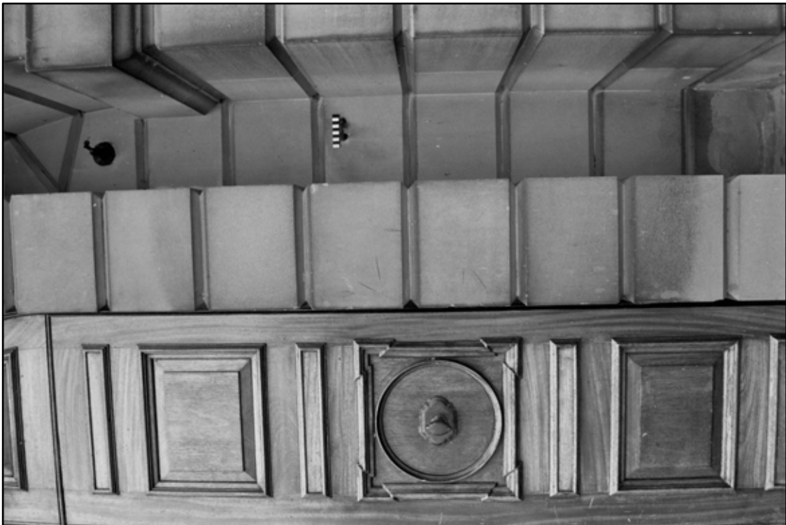
Appendix 5.50: Detail of remains of external bell pull adjacent to north entrance doors (10cm scale) (Film 32.36)
