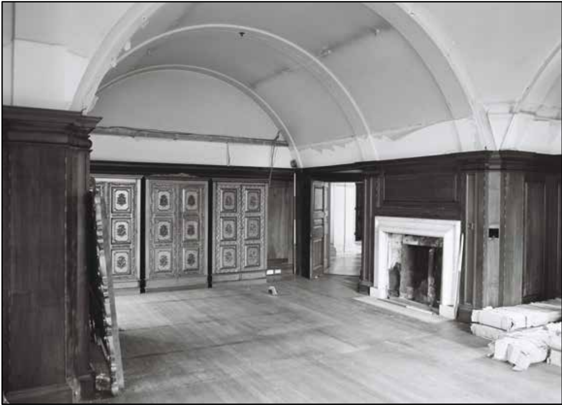
Appendix 5.143: General view across vaulted billiard room G1, looking southeast (1m/2m scale) (Film 25.04)
