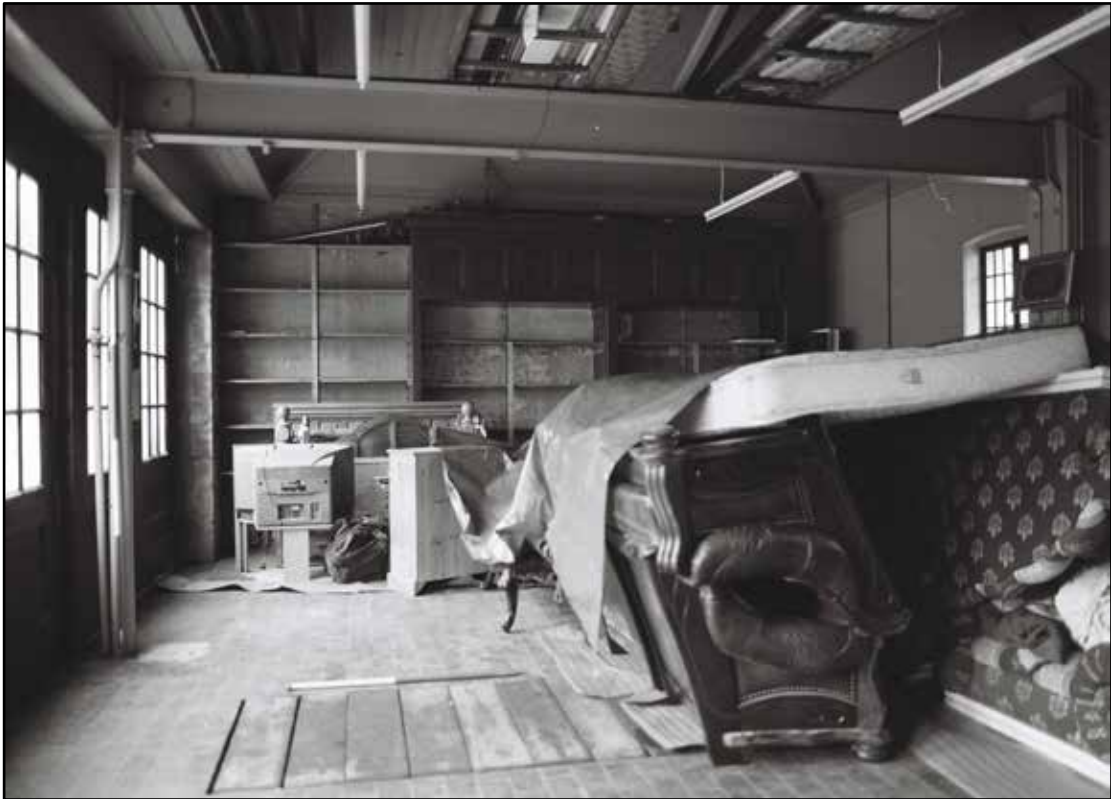
Appendix 5.245: General view of the vehicle garage GA4 in motor house, looking west (1m/2m scale) (Film 19.15)
