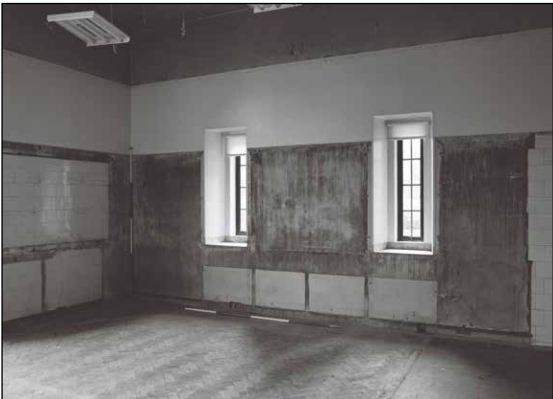
Appendix 5.159: General view of kitchen G1 I, looking south; note scars of former cupboards (2m scale) (Film 31.08)
