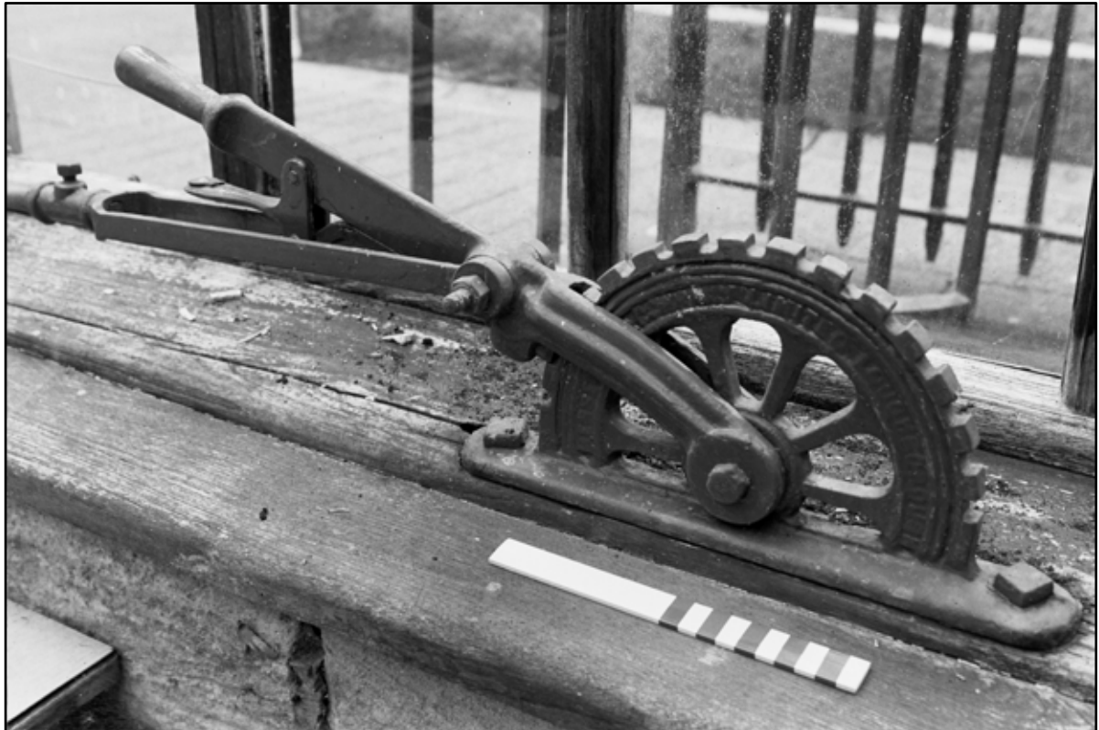
Appendix 5.41: Detail of winding handle for greenhouse windows (20cm scale) (Film 32.31)
