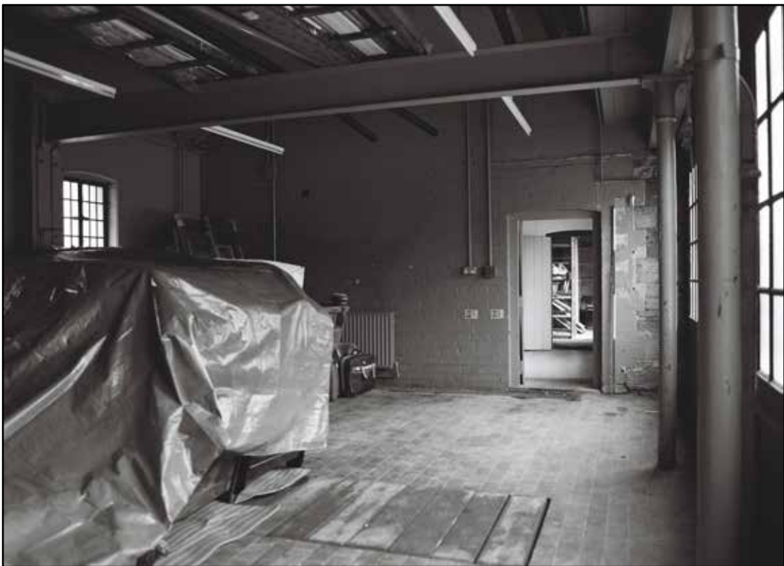
Appendix 5.246: General view of the vehicle garage GA4 in motor house, looking east (2m scale) (Film 20.02)
