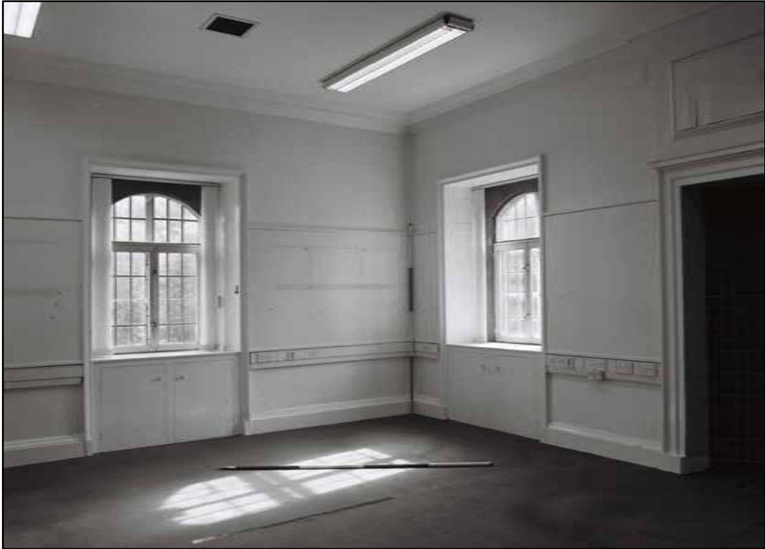
Appendix 5.175: General view of F1, looking southwest (2m scale) (Film 17.08)
