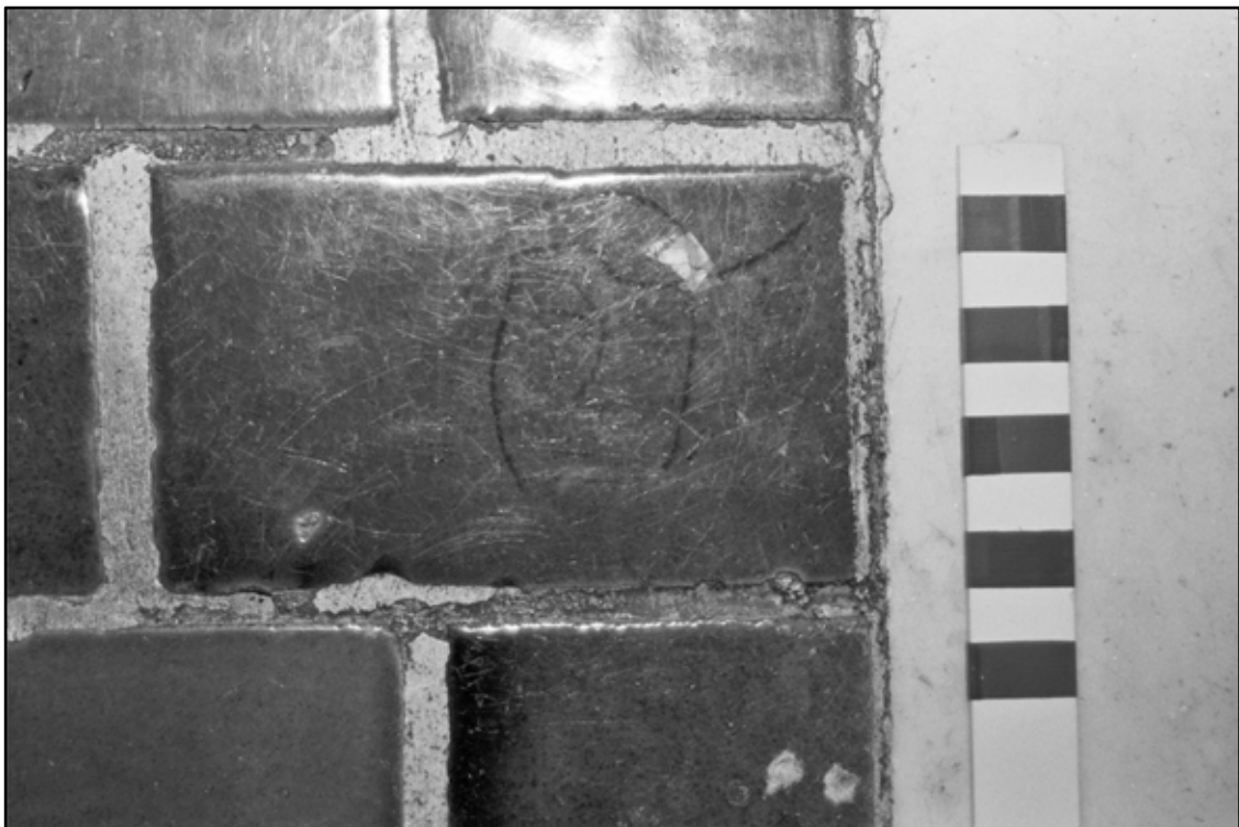
Appendix 5.200: Detail of face beneath glazing of fireplace tile in F10 (1 cm scale divisions) (Film 33.12)
