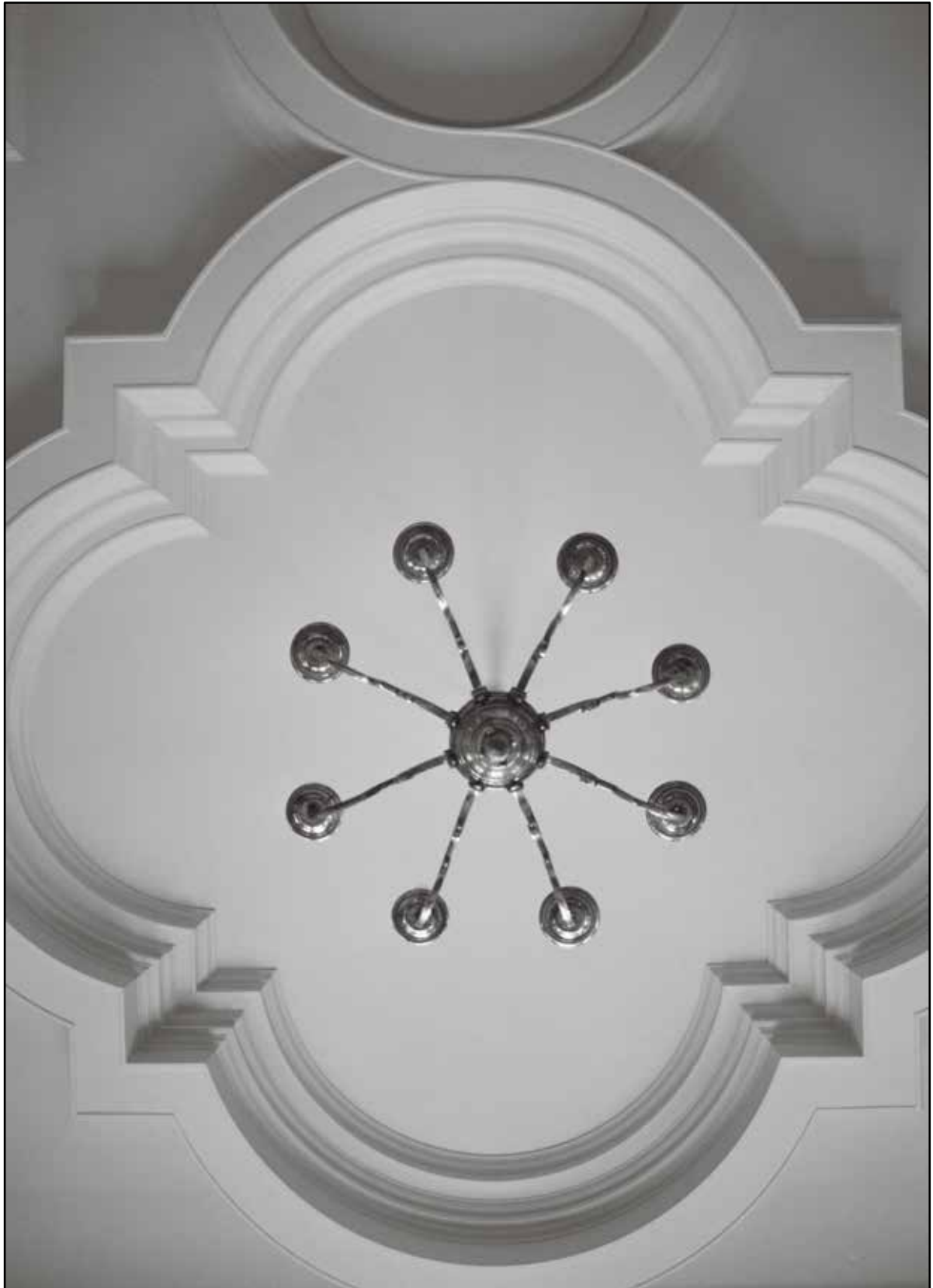
Appendix 5.129: Detail of ceiling in G7 (Film 27.09)
