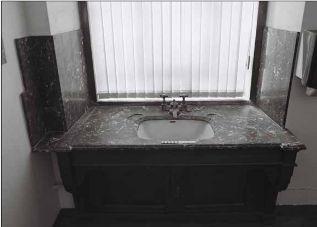
Appendix 5.141: Detail of sink with marble surround in G3, looking east (20cm scale) (Film 25.12)
