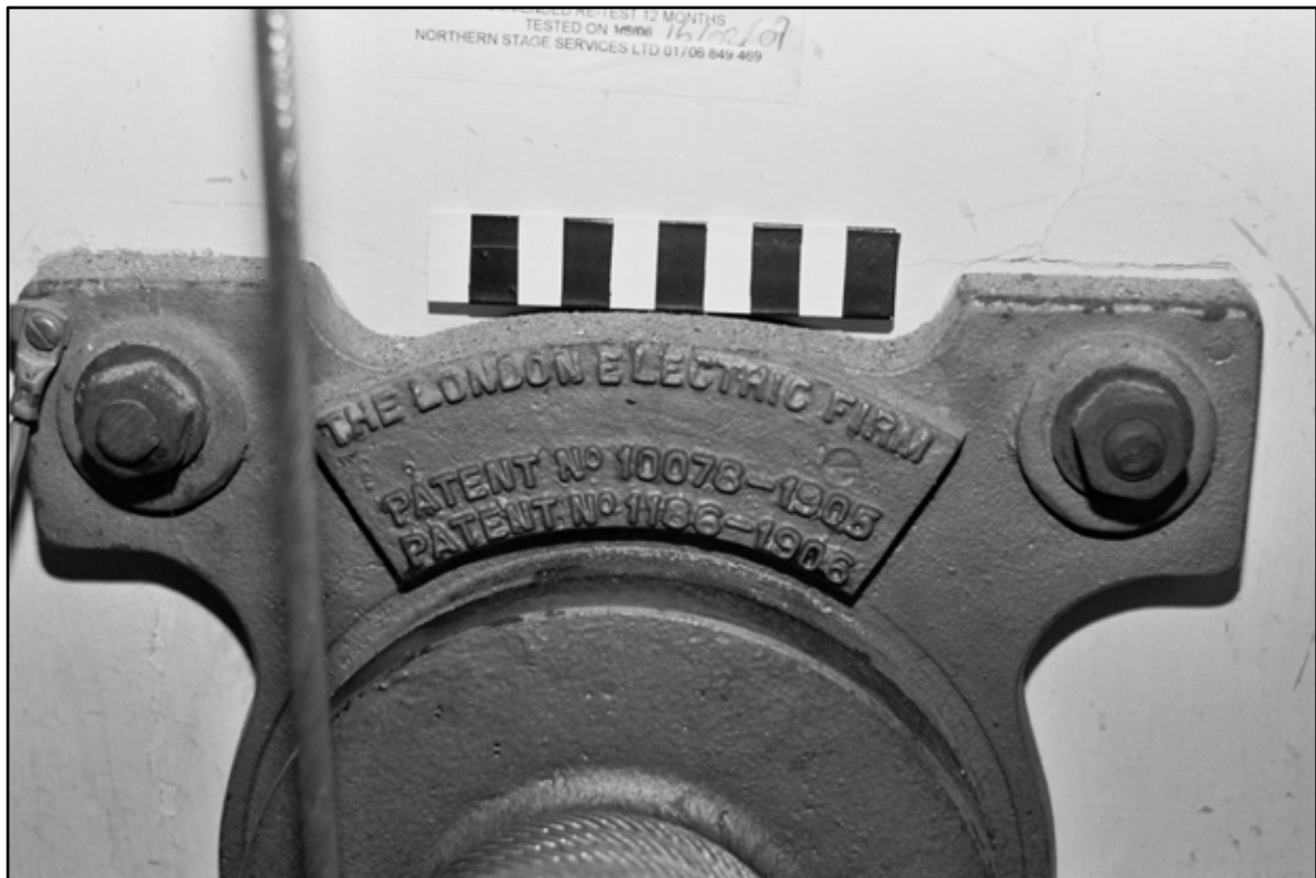
Appendix 5.170: Detail of winding mechanism for chandelier in F5 (10cm scale) (Film 33.15)
