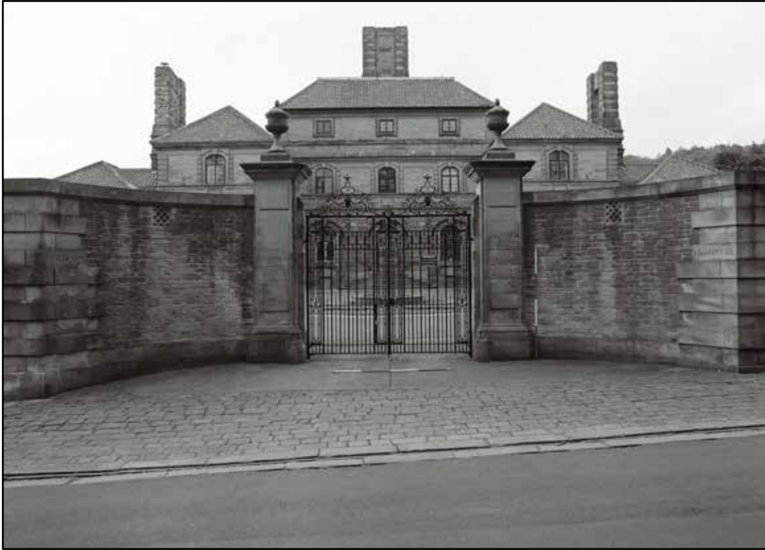
Appendix 5.3: Detail of entrance on Kings Road (gates closed), looking south (2m scale) (Film 4.07)
