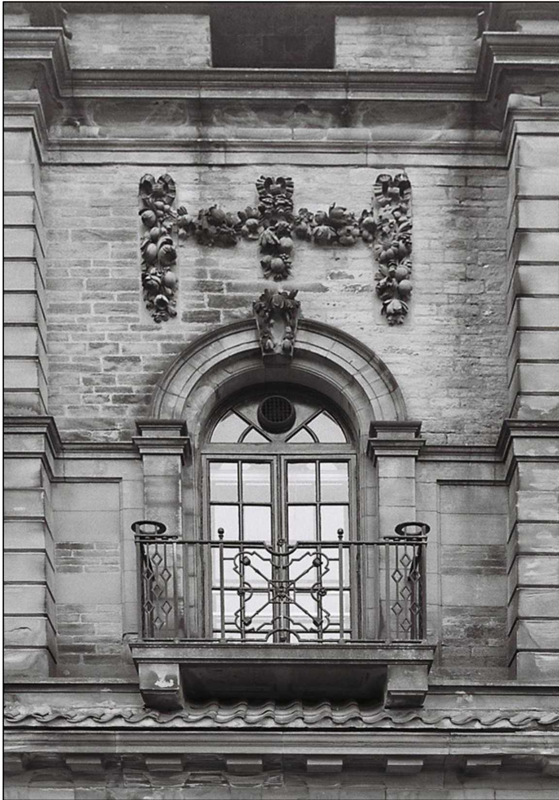
Appendix 5.78: Detail of first floor balcony on south elevation (Film 7.11)
