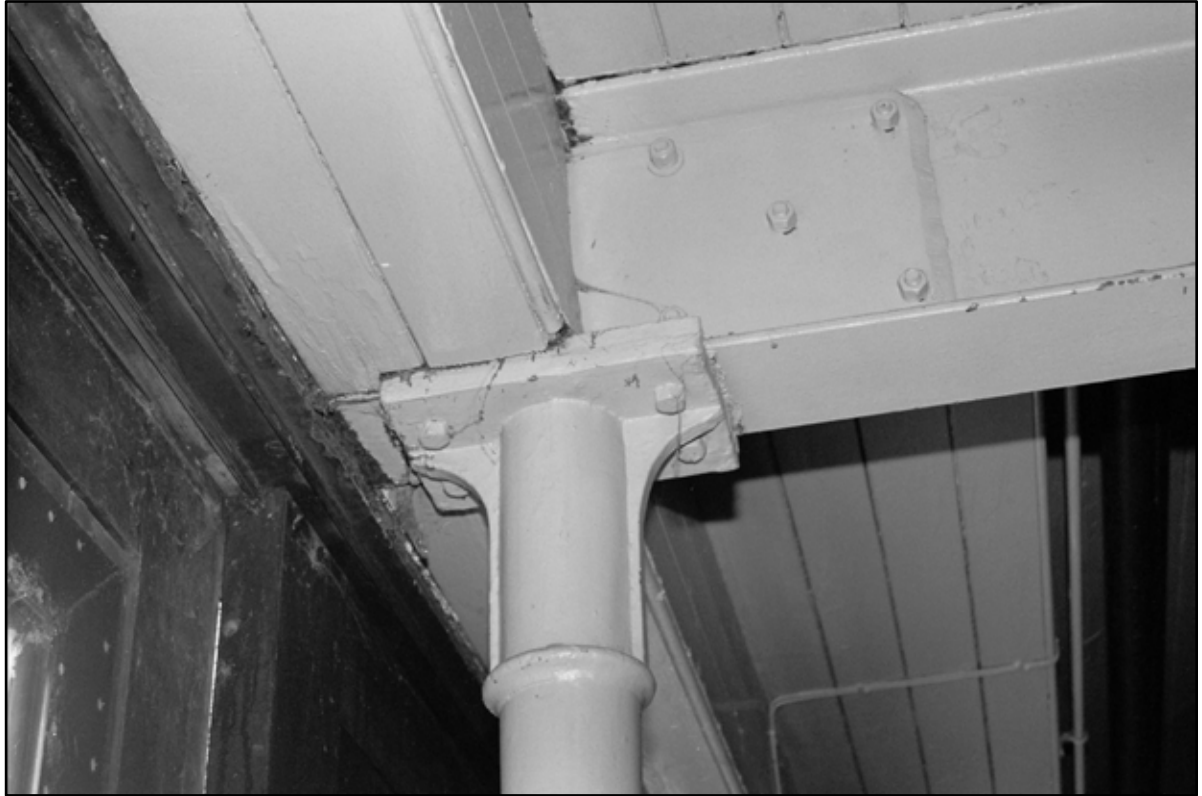
Appendix 5.260: Detail of cast iron column in GA4 of motor house (Film 21.14)
