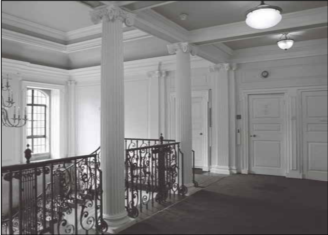
Appendix 5.167: General view across landing F9, looking north (2m scale) (Film 17.14)
