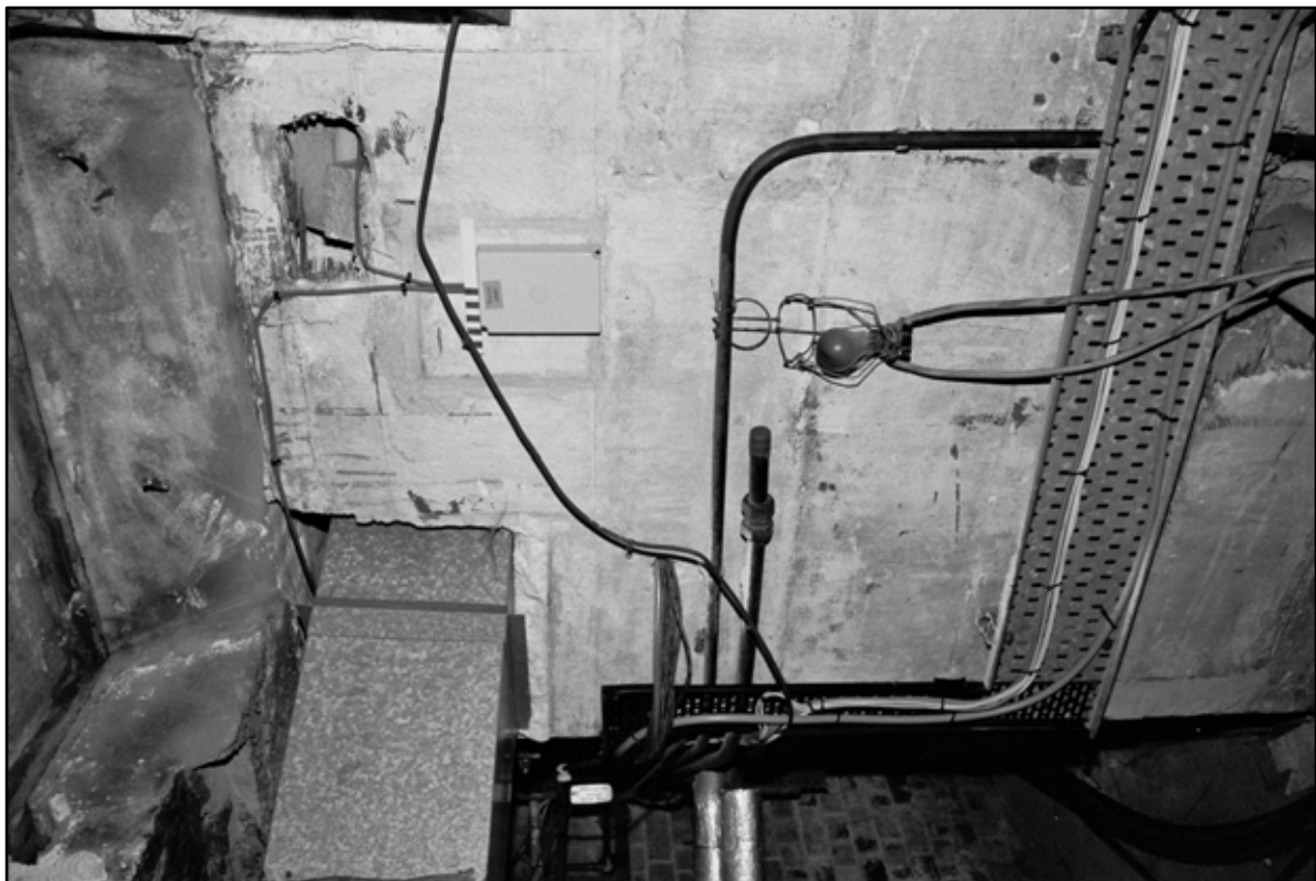
Appendix 5.93: Detail of walling forming plenum chamber; note rush and cement blockwork (20cm) (Film 22.35)
