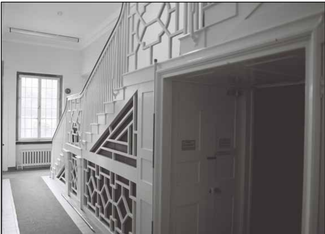
Appendix 5.152: General view along G10 looking east of ancillary staircase to upper floors (2m scale) (Film 29.06)
