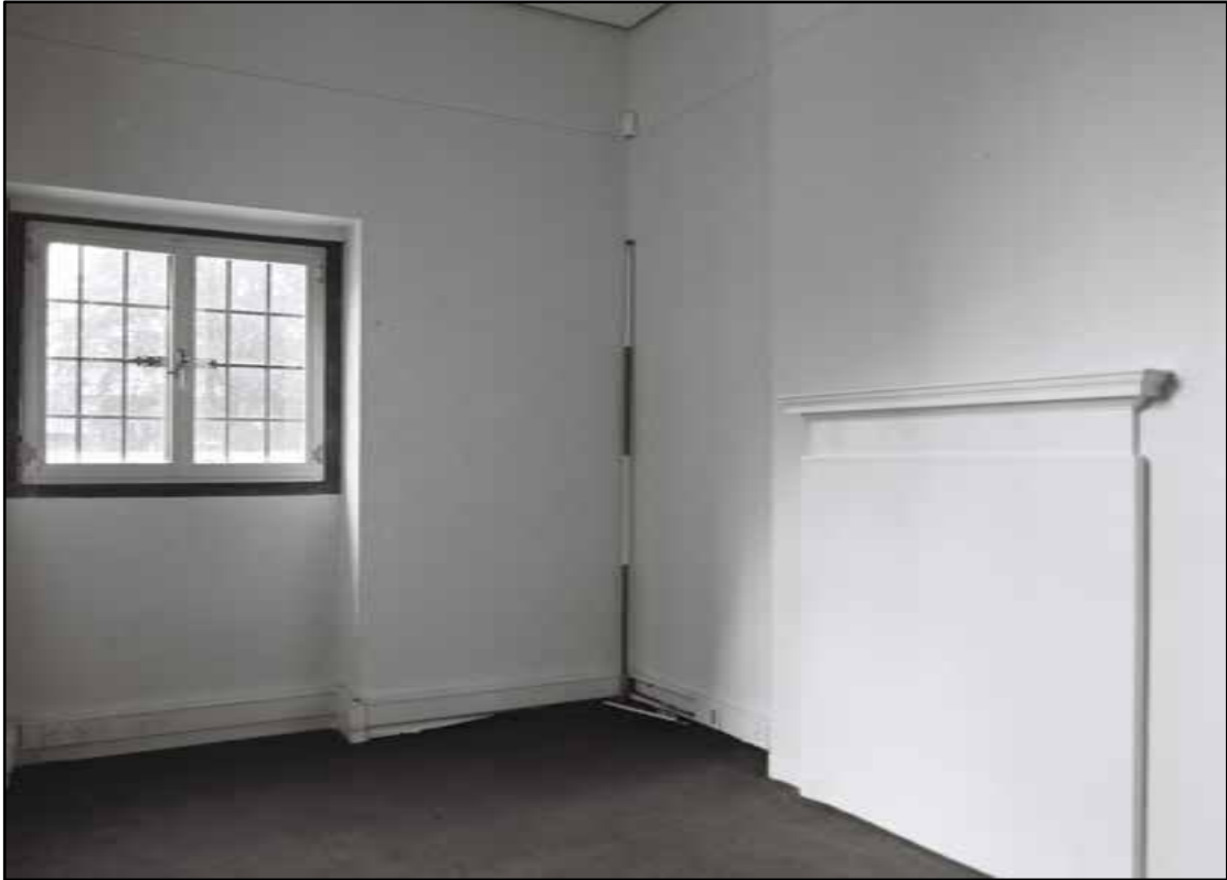
Appendix 5.153: General view of G13 (2m scale) (Film 30.10)
