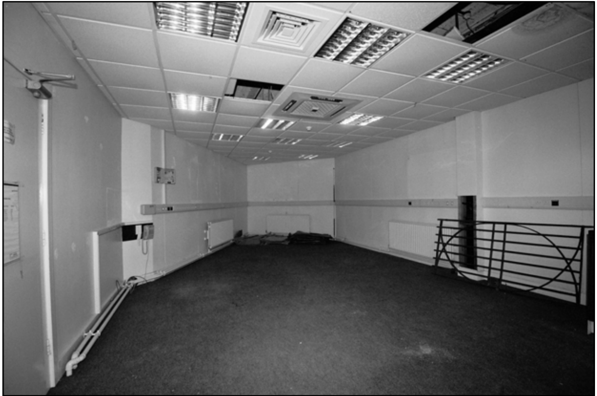
Appendix 5.226: General view of A4, looking west (2m scale) (Film 22.11)
