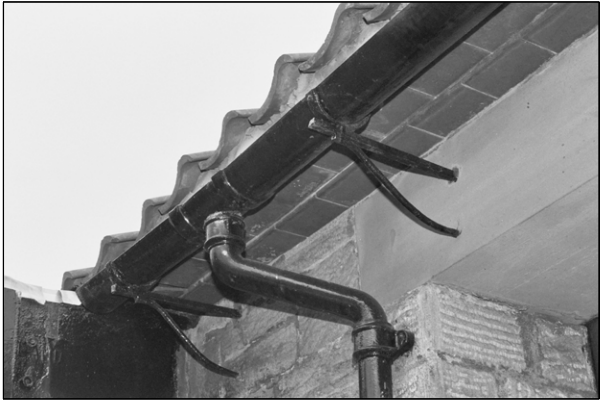
Appendix 5.243: Detail of external gutter brackets on motor house (Film 21.36)
