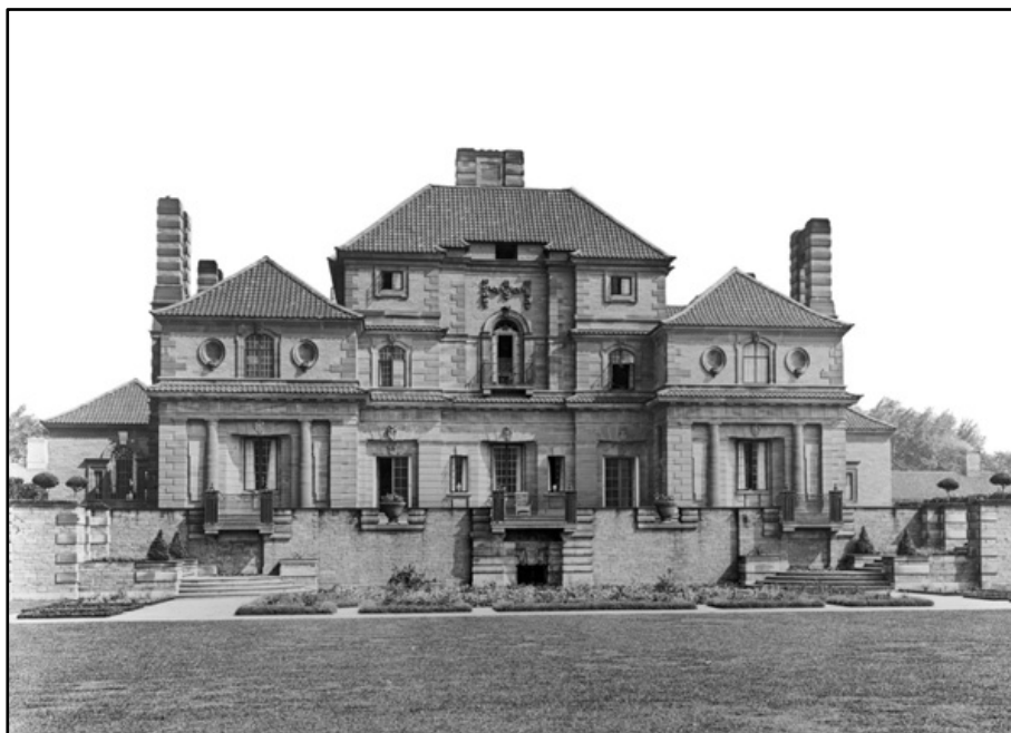
Appendix 6.1: South elevation of House. Country Life © photograph No. 715811. Date 9th July 1910
