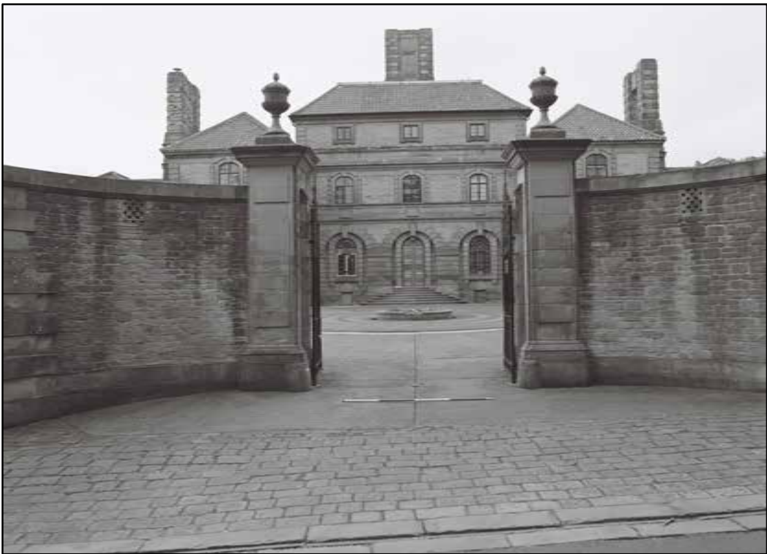
Appendix 5.4: Detail of entrance on Kings Road (gates open), looking south (2m scale) (Film 4.09)
