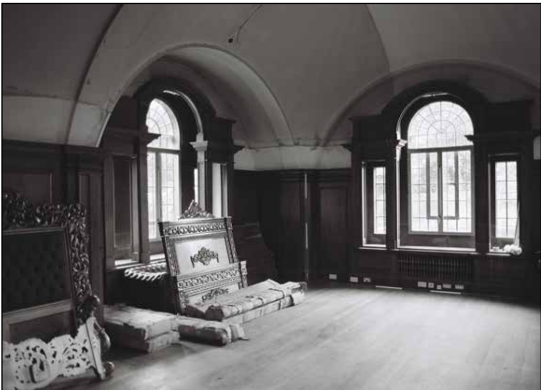
Appendix 5.144: General view across vaulted billiard room G1, looking west (2m scale) (Film 25.03)
