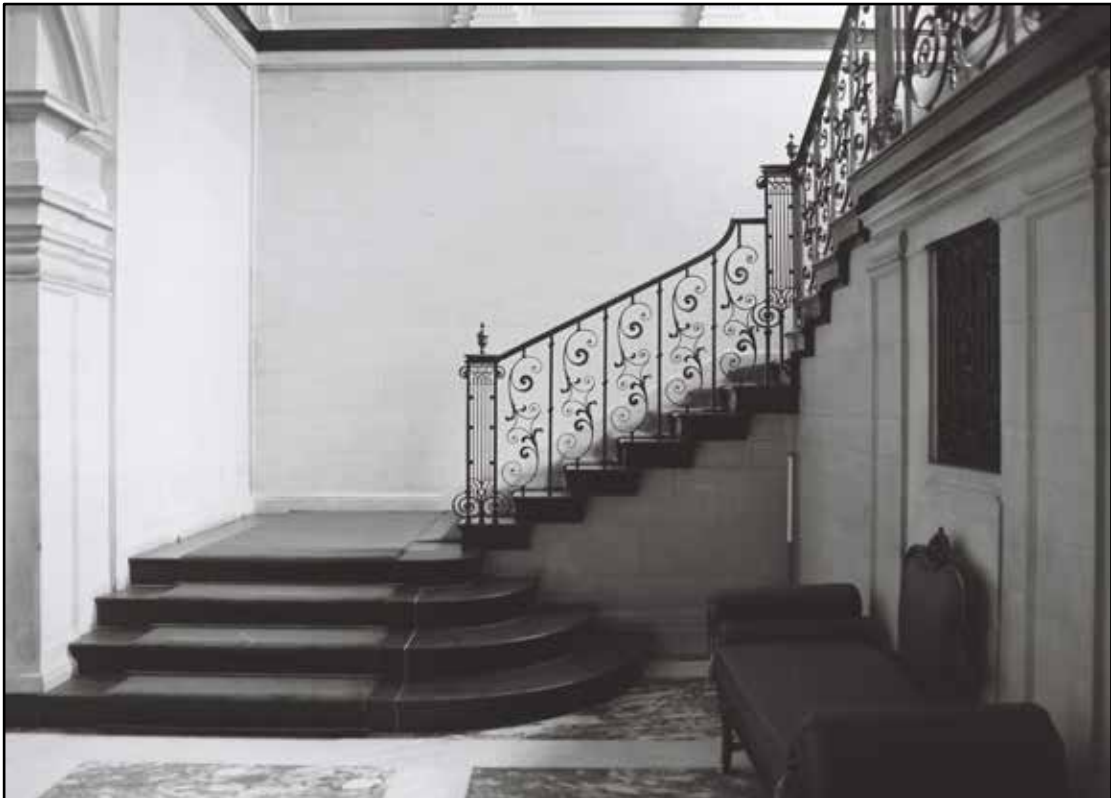
Appendix 5.131: General view of staircase leading to first floor in G5 (1m scale) (Film 26.03)
