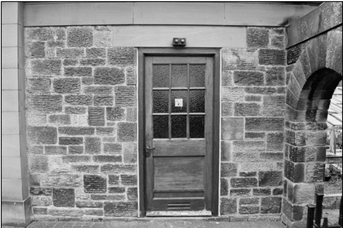
Appendix 5.239: Detail of doorway into room GA1 of motor house (Film 21.29)
