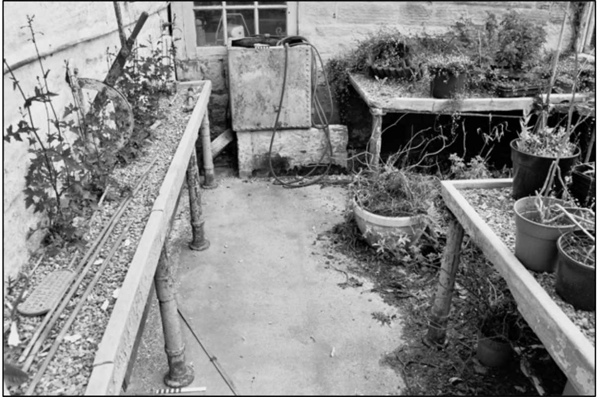
Appendix 5.45: Detail of greenhouse and original staging with cast iron columns (20cm scale) (Film 32.03)
