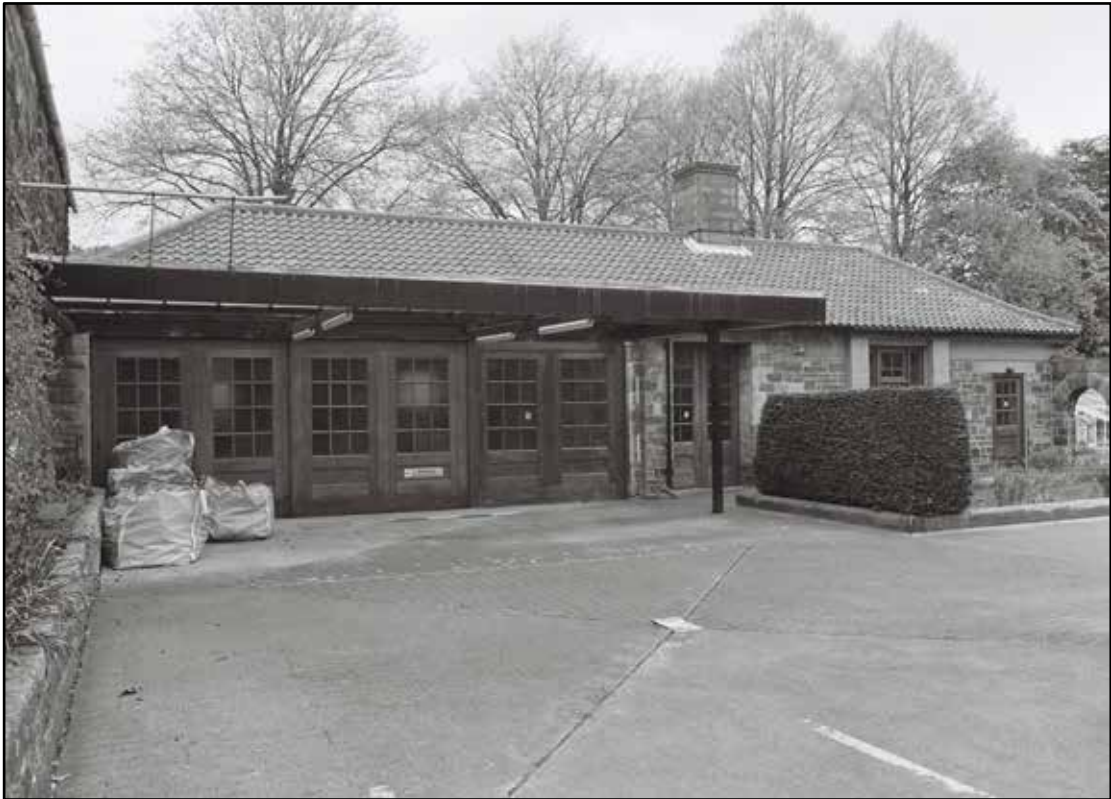
Appendix 5.236: Detail of south elevation of motor house (2m scale) (Film 10.07)
