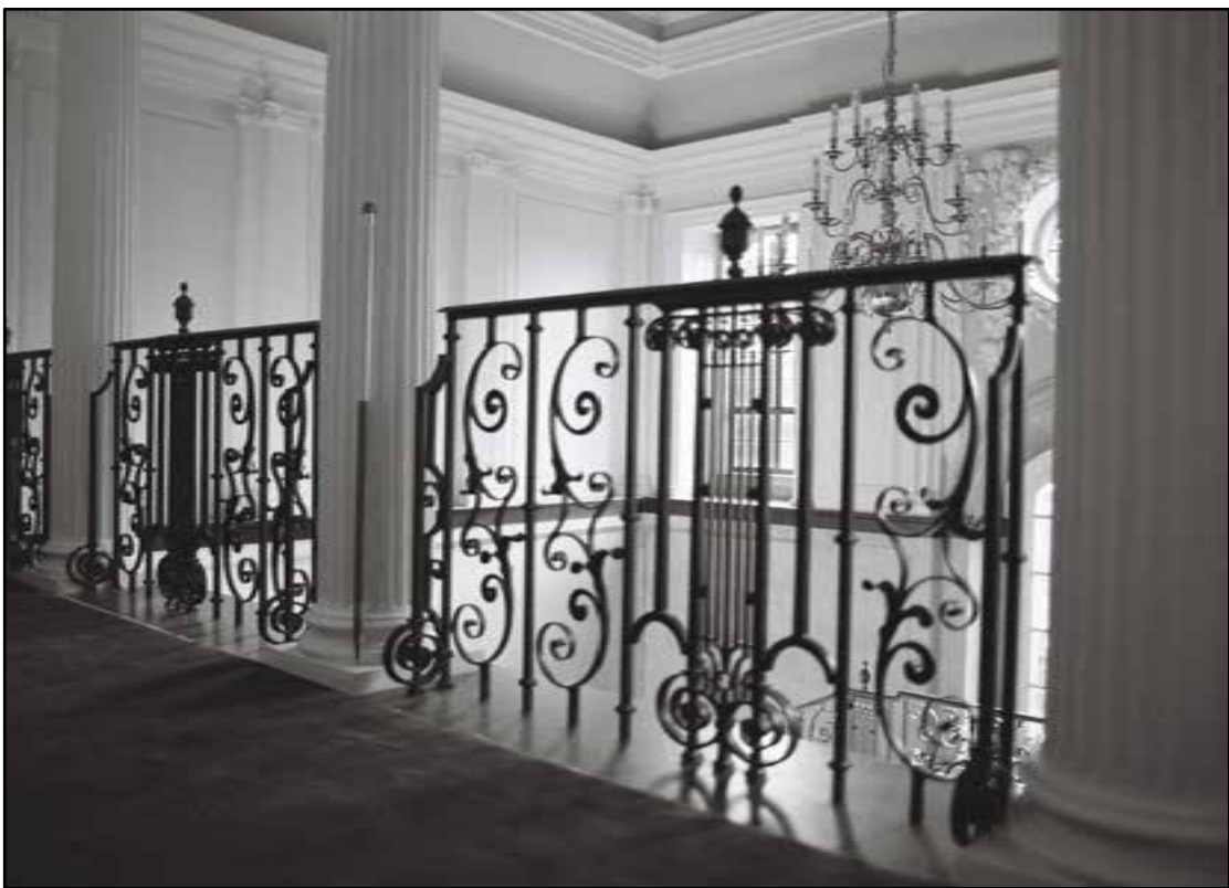
Appendix 5.168: Detail of metal balustrade in F9, looking southwest (2m scale) (Film 18.03)
