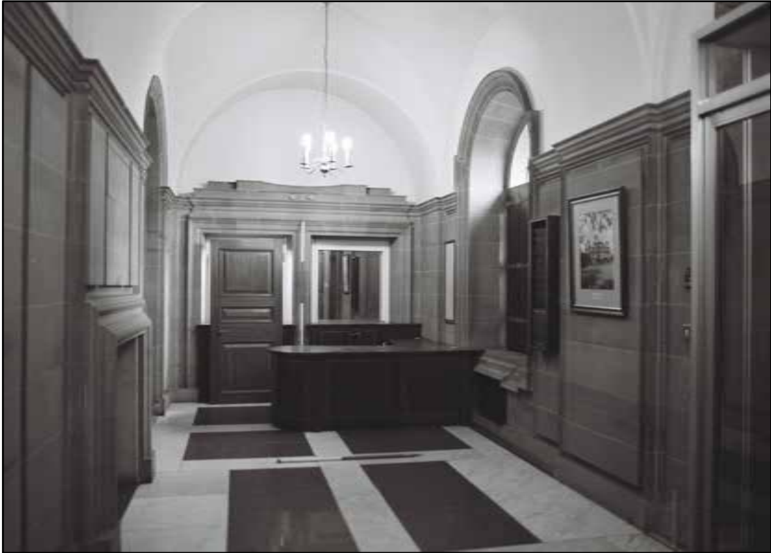
Appendix 5.II10: General view of entrance hall G4 looking west (1m/2m scale) (Film 28.10)
