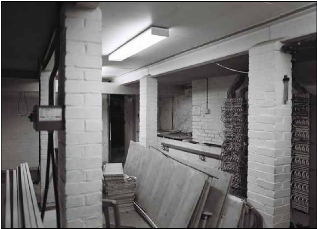
Appendix 5.101: General view of basement room B3 converted to an air-raid shelter (2m scale) (Film 23.03)
