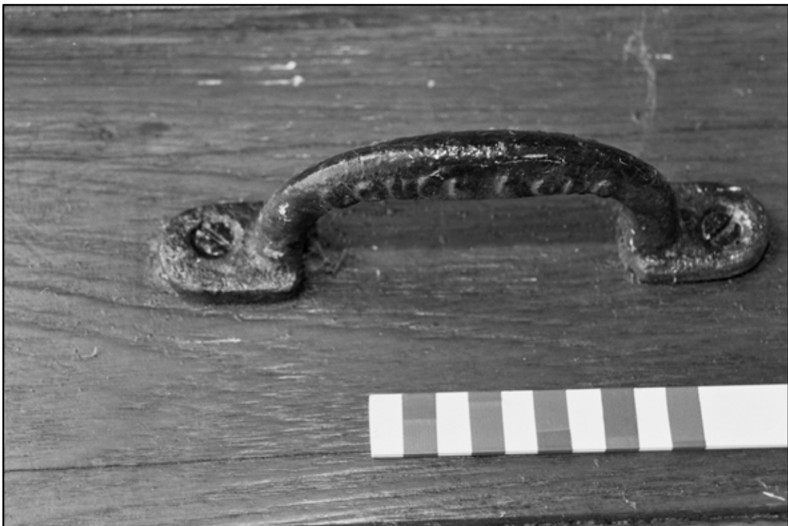
Appendix 5.259: Detail of exterior handle to sliding doors of motor house (1cm scale divisions) (Film 21.35)
