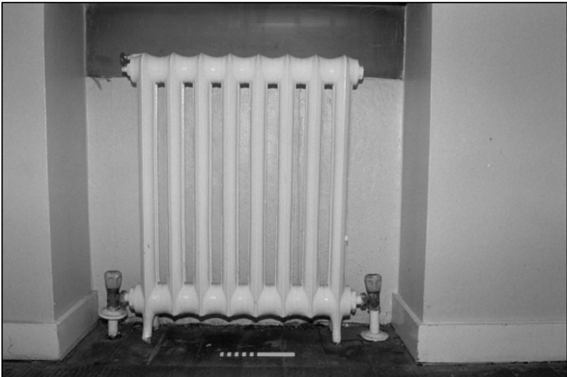
Appendix 5.209: Detail of cast-iron radiator in S4 (20cm scale) (Film 33.03)
