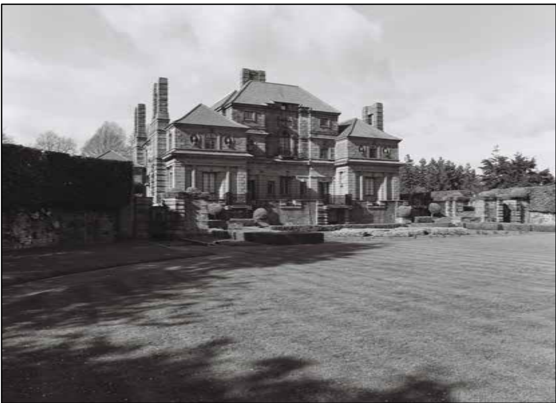
Appendix 5.13: General view of south façade of the house (2m scale) (Film 1.09)
