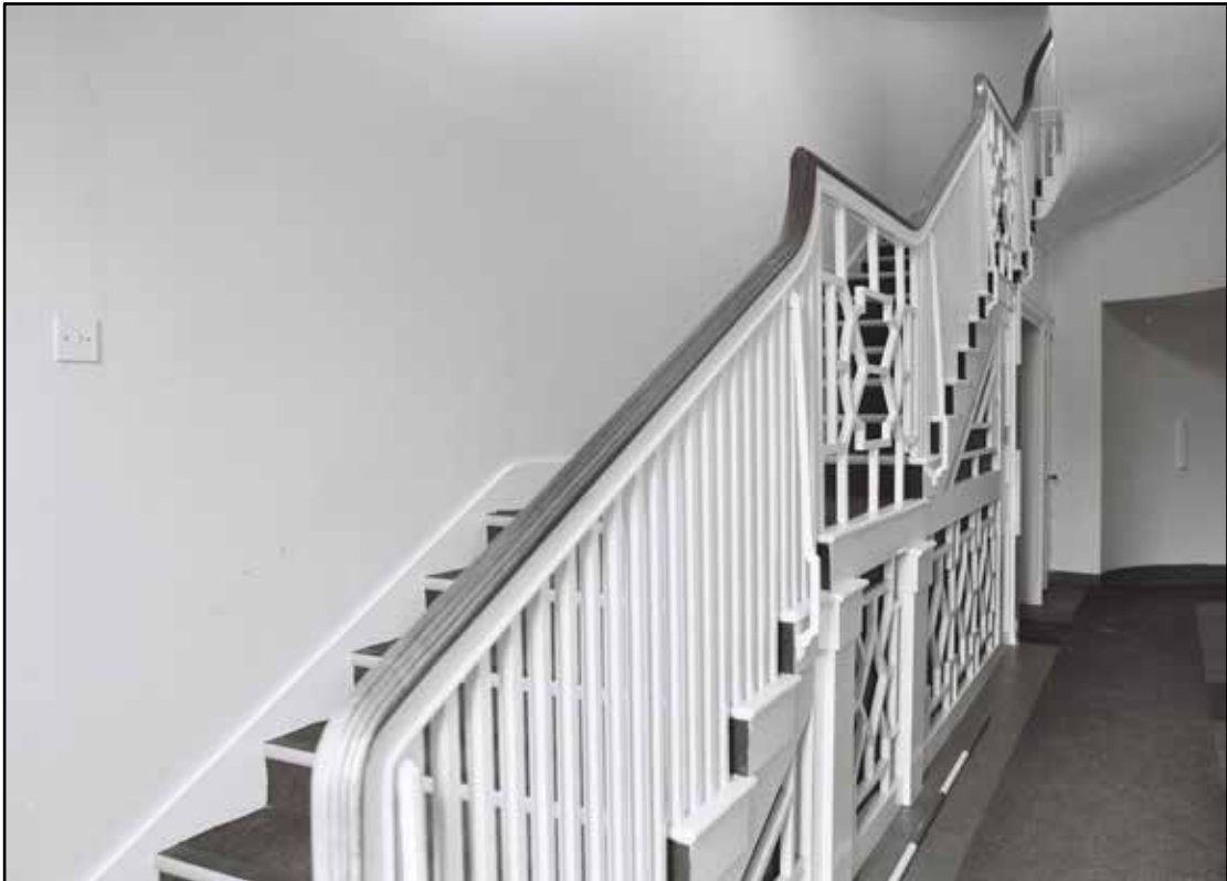
Appendix 5.151: General view along G10 looking west of ancillary staircase to upper floors (2m scale) (Film 29.09)
