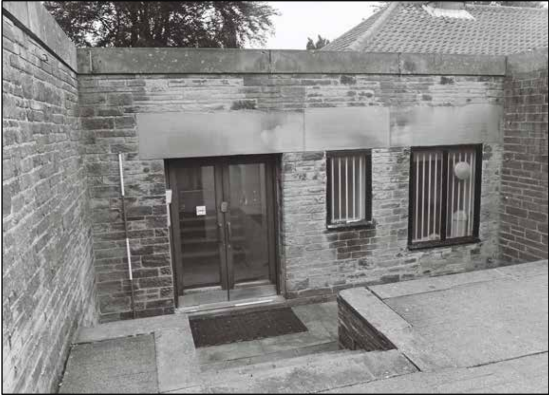
Appendix 5.222: General view of entrance to Annex, looking north (1m/2m scale) (Film 6.02)
