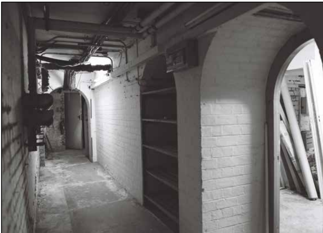
Appendix 5.95: General view of corridor B5, looking south (2m scale) (Film 24.07)
