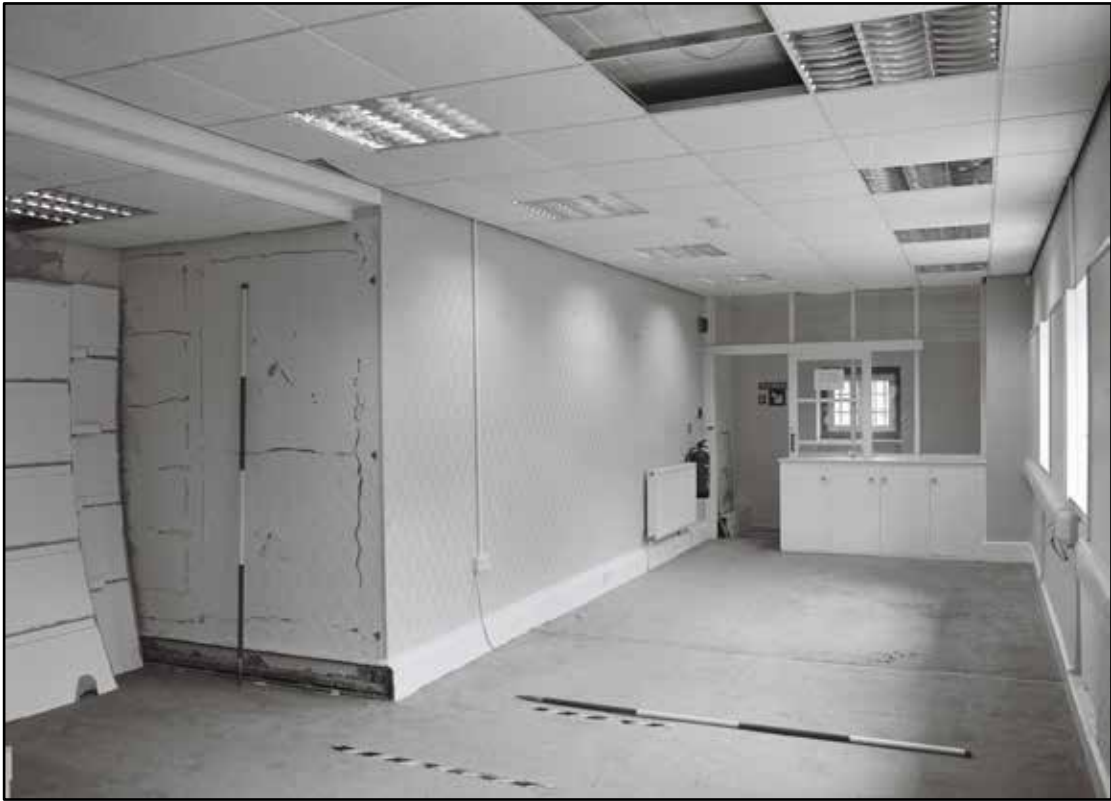
Appendix 5.211: General view of S7, looking south (2m scale) (Film 12.14)
