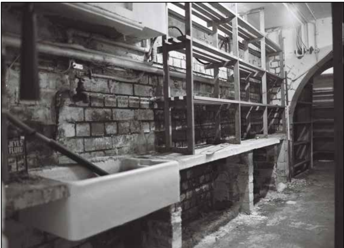
Appendix 5.103: General view of north wall of B8; note Belfast sink and stone tables (2m scale) (Film 24.02)
