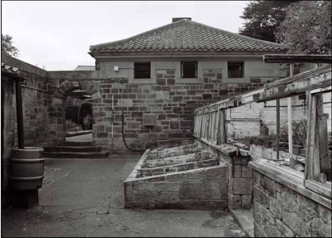
Appendix 5.238: Detail of east elevation of motor house; note high level vents (2m scale) (Film 10.12)
