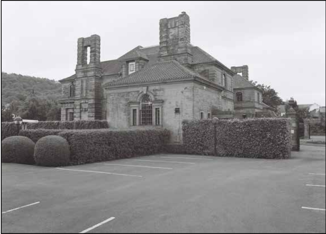
Appendix 5.59: General view looking southwest across kitchen block (2m scale) (Film 6.04)
