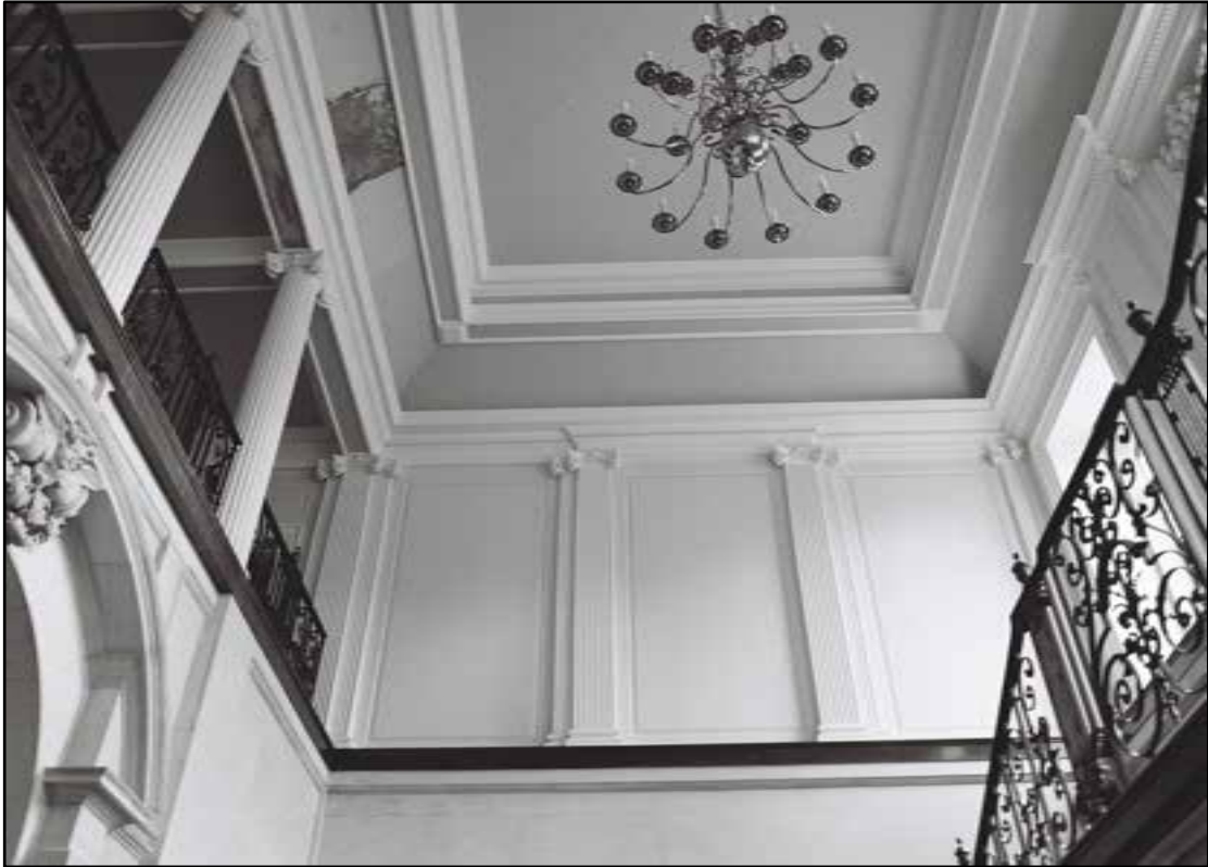
Appendix 5.169: General view of ceiling above stairwell F2 (Film 26.05)
