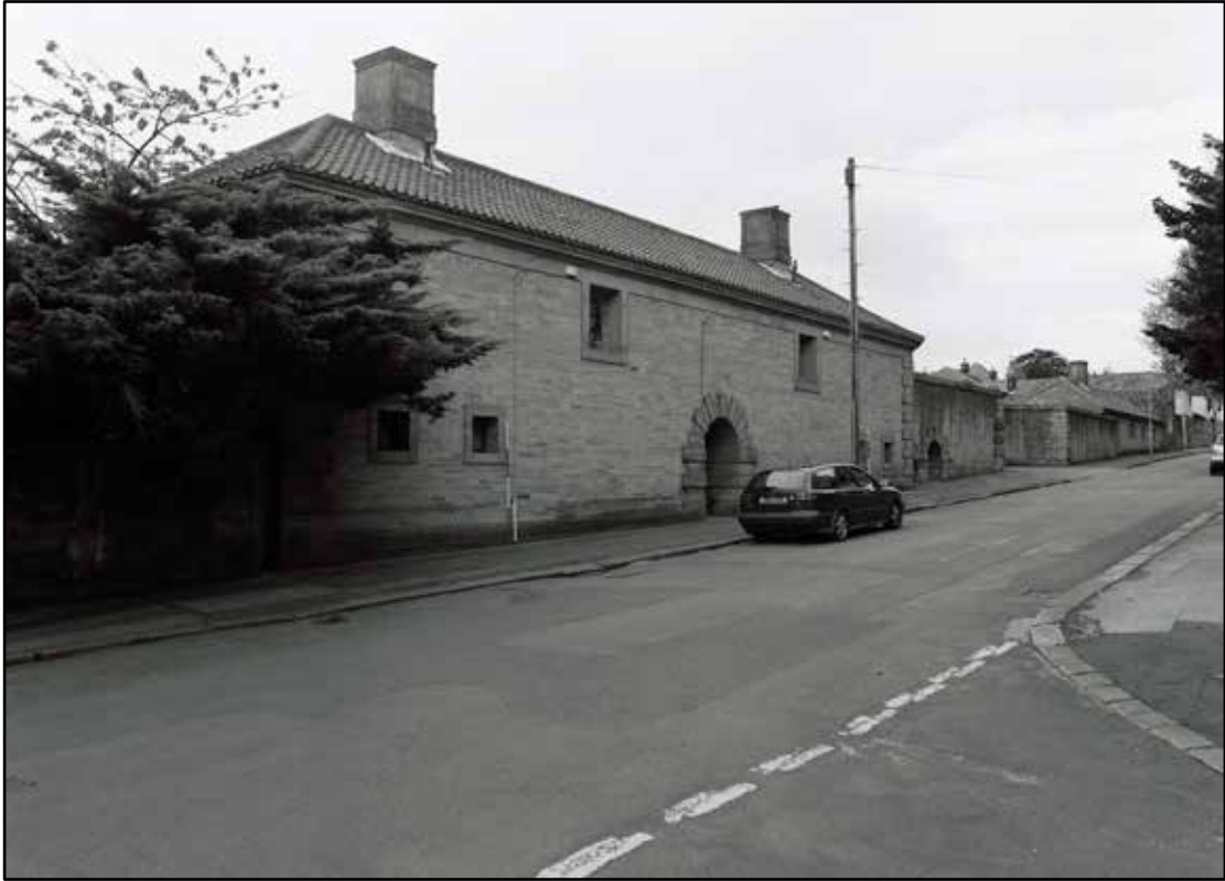
Appendix 5.5: General view looking southeast along Kings Road (2m scale) (Film 4.10)
