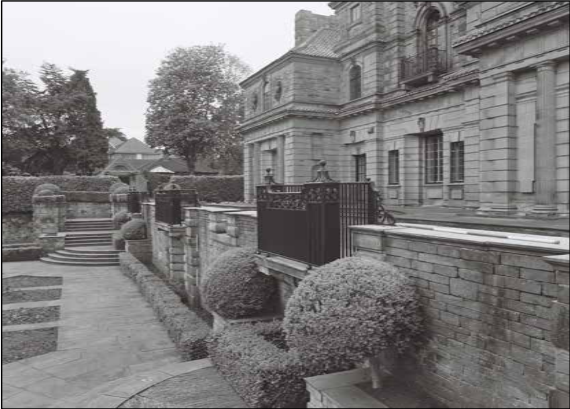
Appendix 5.24: General view along lower terrace retaining wall, looking west (2m scale) (Film 7.05)
