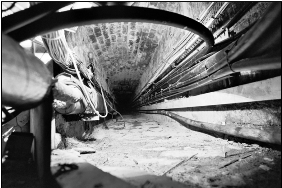
Appendix 5.235: General view along vaulted tunnel in A10, looking northeast (Film 22.25)
