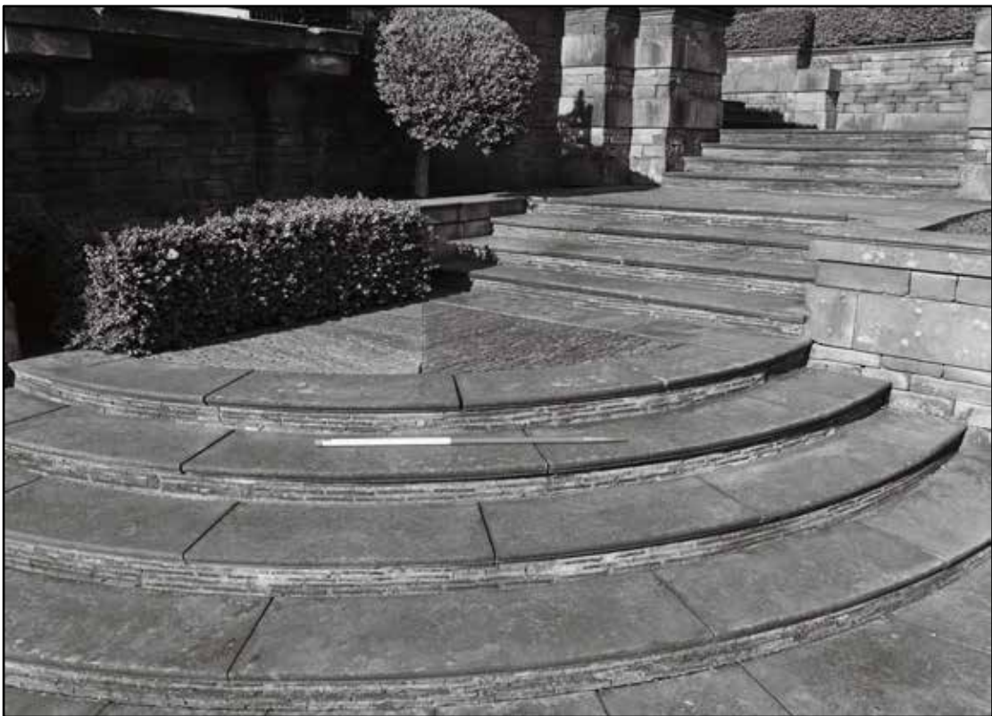
Appendix 5.21: General view of lower parterre steps (1m scale) (Film 2.15)
