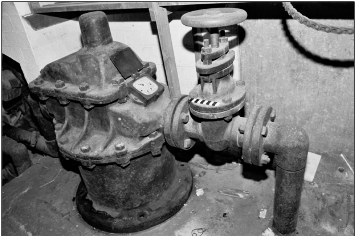
Appendix 5.106: Detail of water meter in B8 (10cm scale) (Film 33.36)
