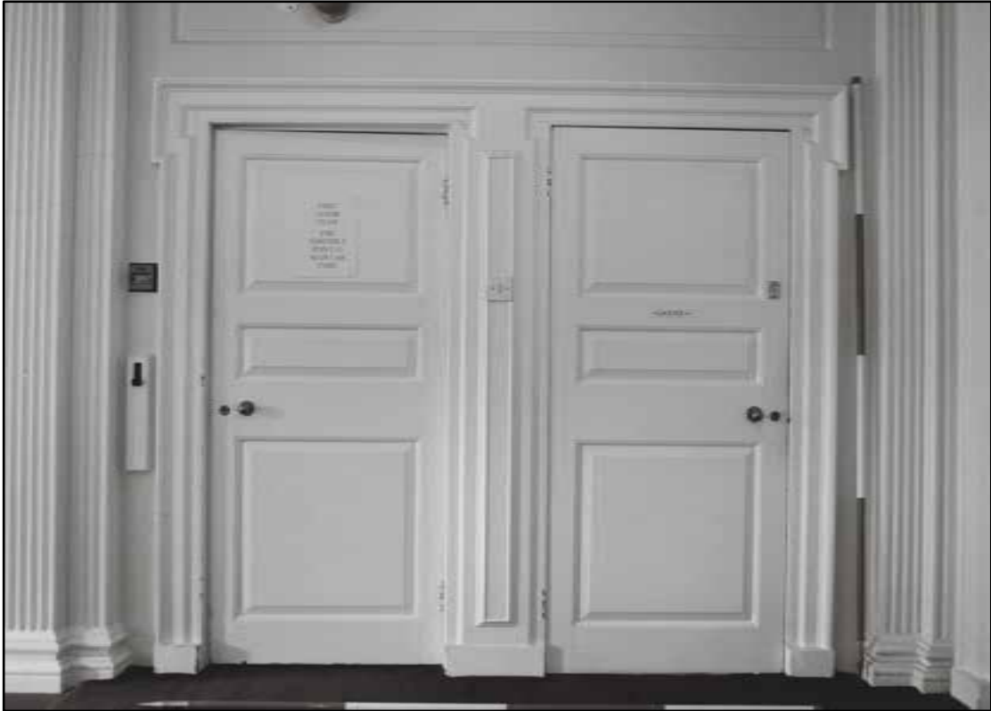
Appendix 5.171: Detail of double doorway in F9, looking north (2m scale) (Film 17.02)
