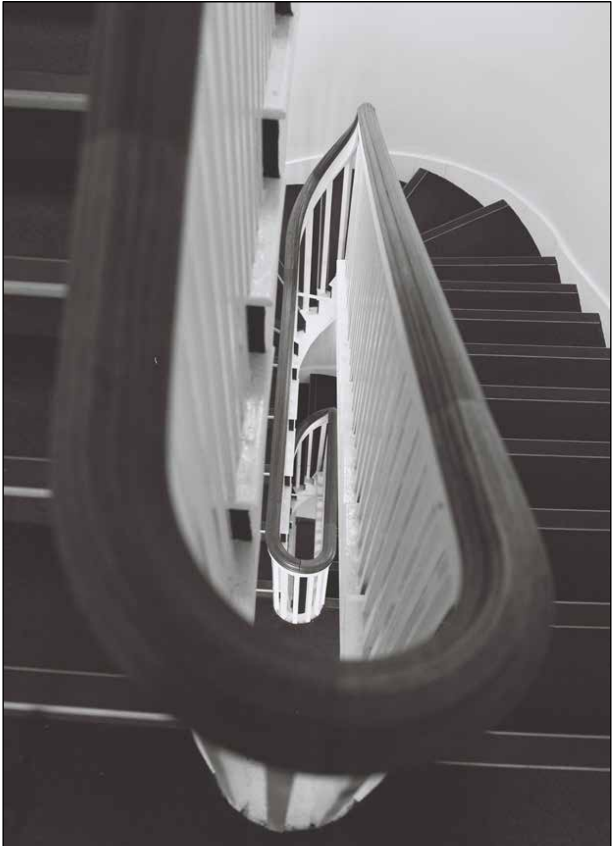
Appendix 5.182: Detail looking down stairwell in F15 (Film 16.02)
