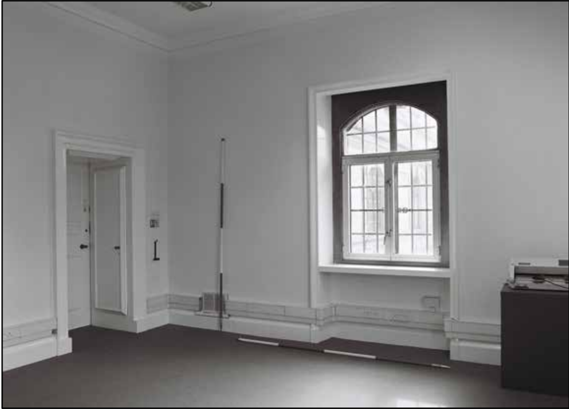
Appendix 5.190: General view of F18, looking southwest (2m scale) (Film 16.09)
