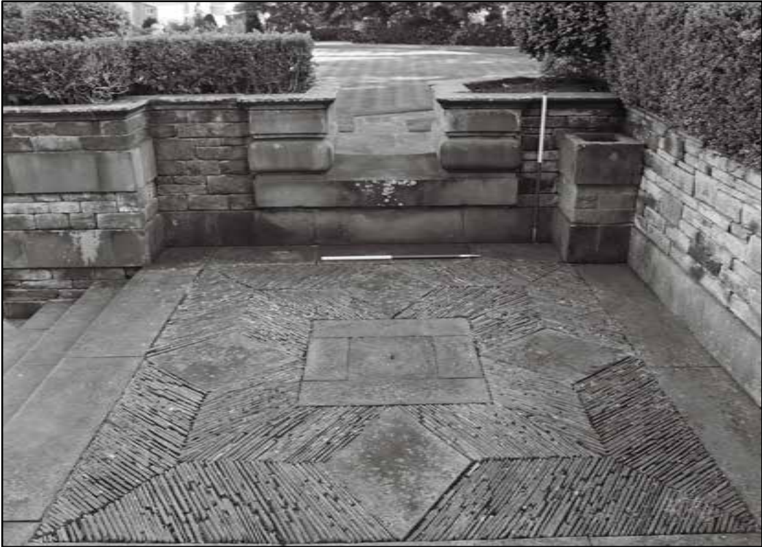
Appendix 5.20: General view of lower parterre steps (1m scale) (Film 3.15)
