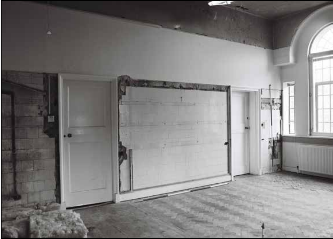
Appendix 5.160: General view of kitchen G11, looking northeast (2m scale) (Film 31.05)
