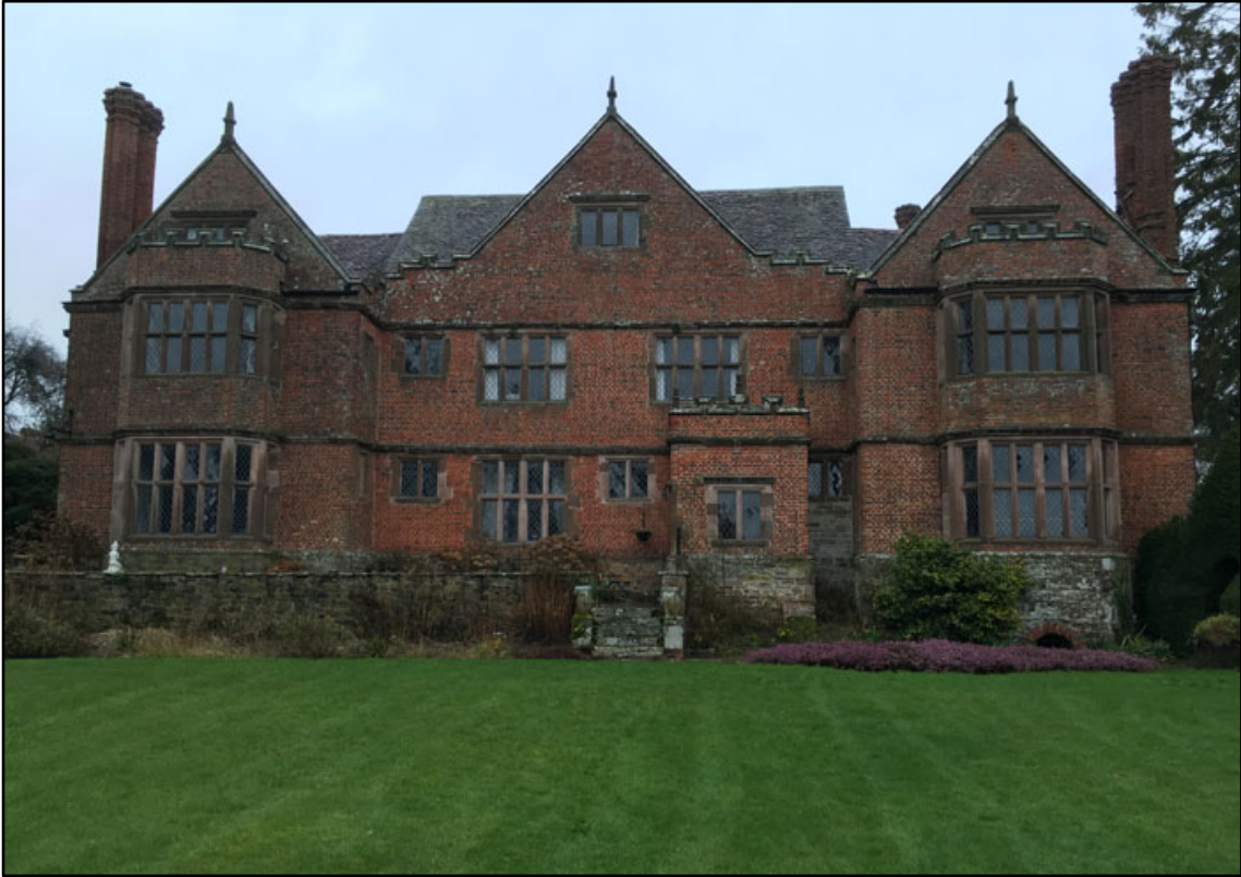
Appendix 3.1: View of south elevation of Whitton Court.
