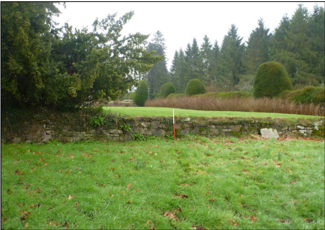
Appendix 3.8: General view of terrace wall F23 , looking north (1m scale).
