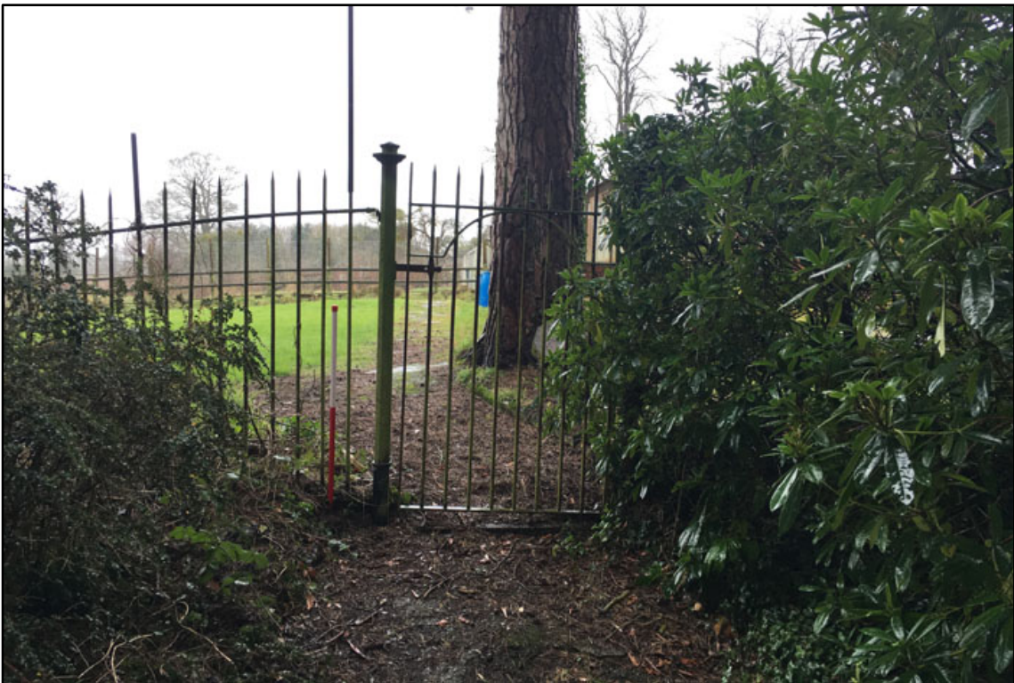
Appendix 3.16: Detail of gateway into walled garden, view west F18 (1m scale).
