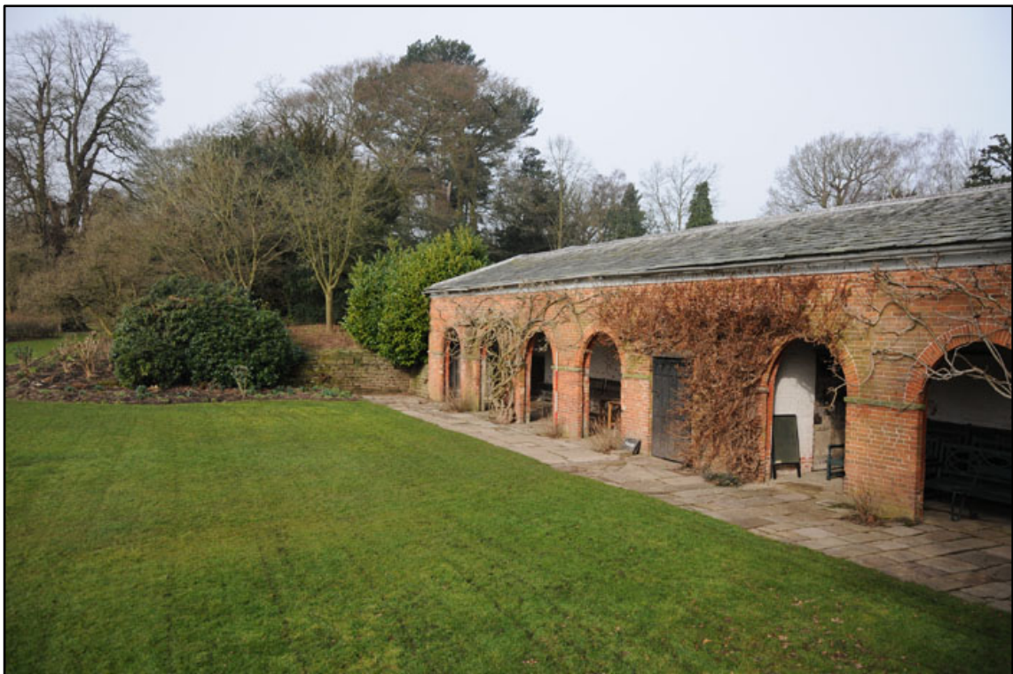
Appendix 2.4: General view of south façade of South Range, looking northwest (2m scale).
