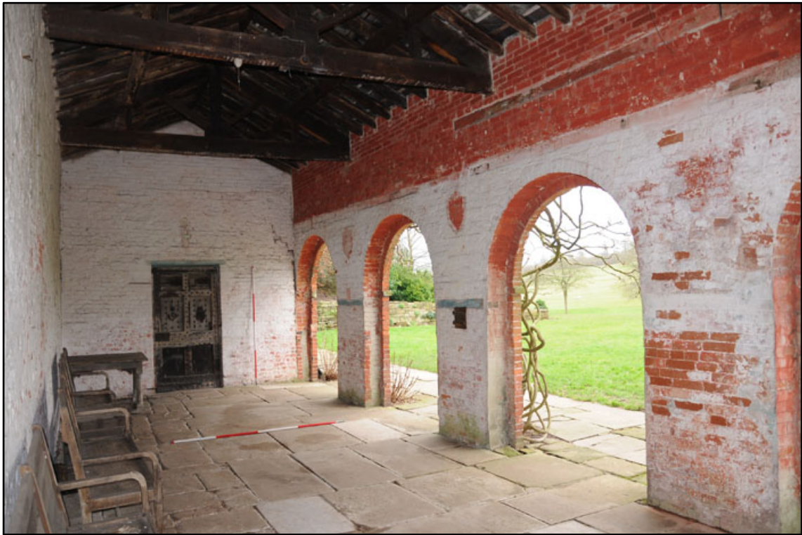
Appendix 2.21: General looking east of G1 (2m scale).
