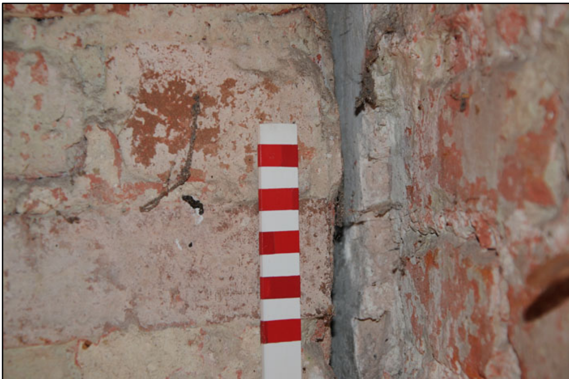
Appendix 2.44: Detail of plaster continuing behind inserted east wall of G2 (10cm scale).
