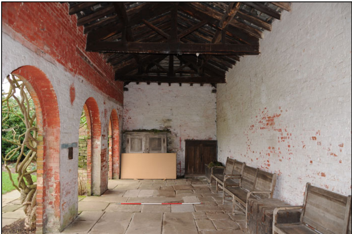
Appendix 2.22: General looking west of G1 (2m scale).
