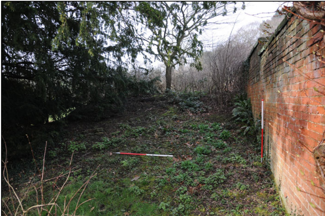
Appendix 2.6: General view of earth mound covering Ice House, looking west (1m scale).
