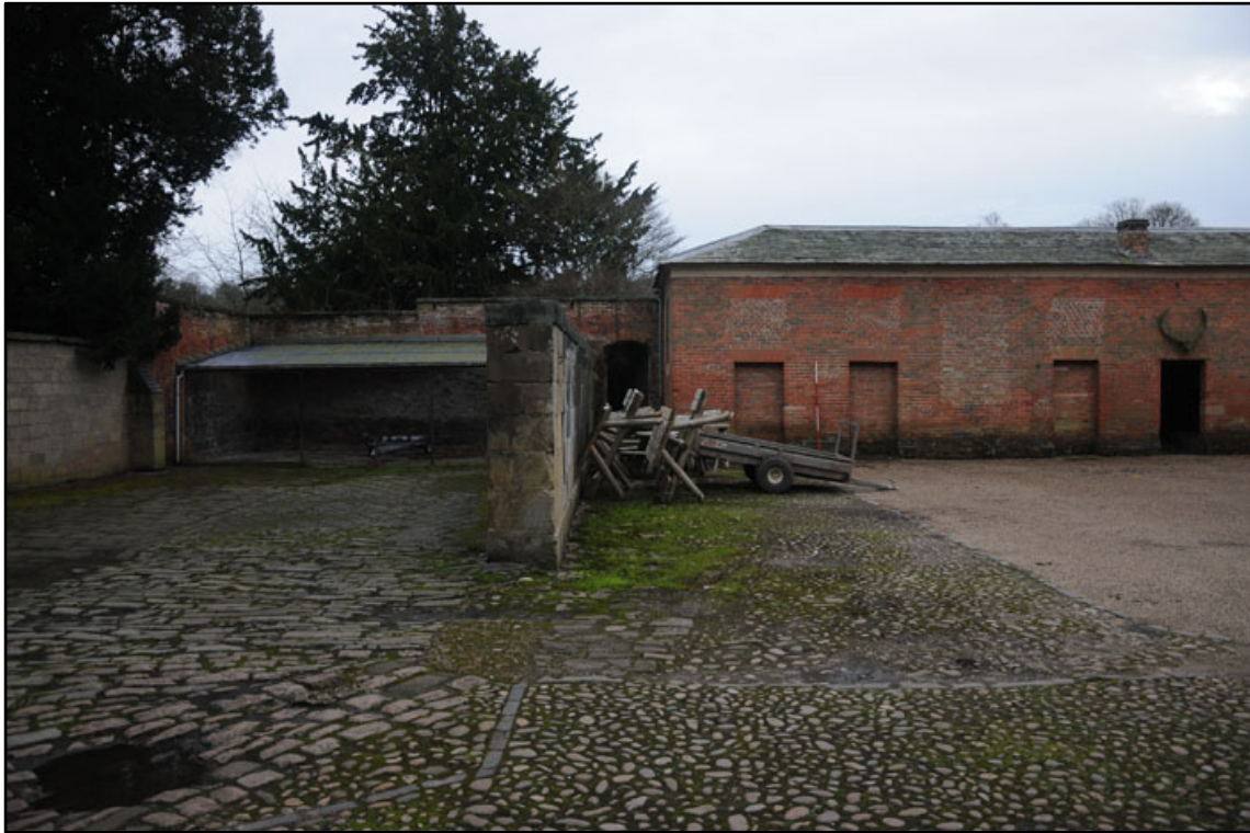
Appendix 2.9: General view of north elevation and stone boundary wall, looking south across Brewhouse Yard (2m scale).
