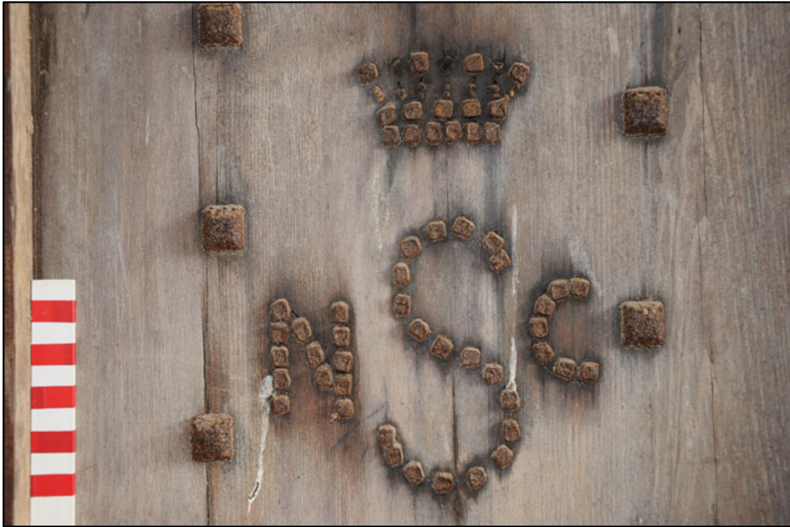
Appendix 2.68: Detail of stud decoration on door D4 in G3 (10cm scale).
