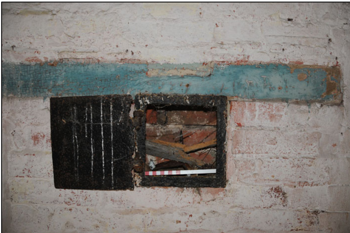
Appendix 2.30: Detail of cupboard interior with metal door between A2 and A3 in G1 (20cm scale).
