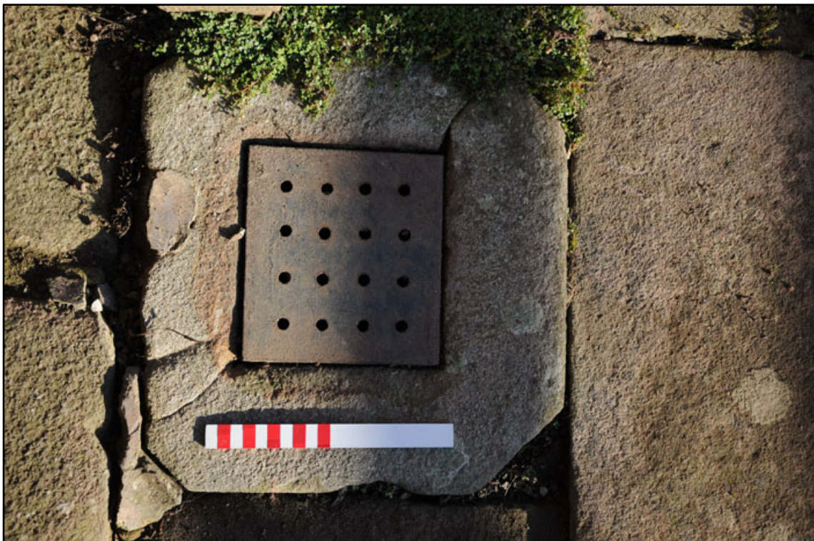
Appendix 2.50: Detail of external drain adjacent to A6 (20cm scale).
