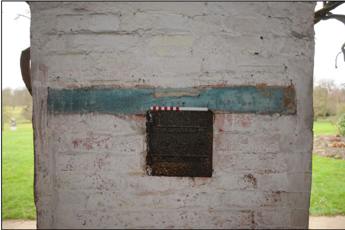
Appendix 2.29: Detail of cupboard with metal door between A2 and A3 in G1 (20cm scale).
