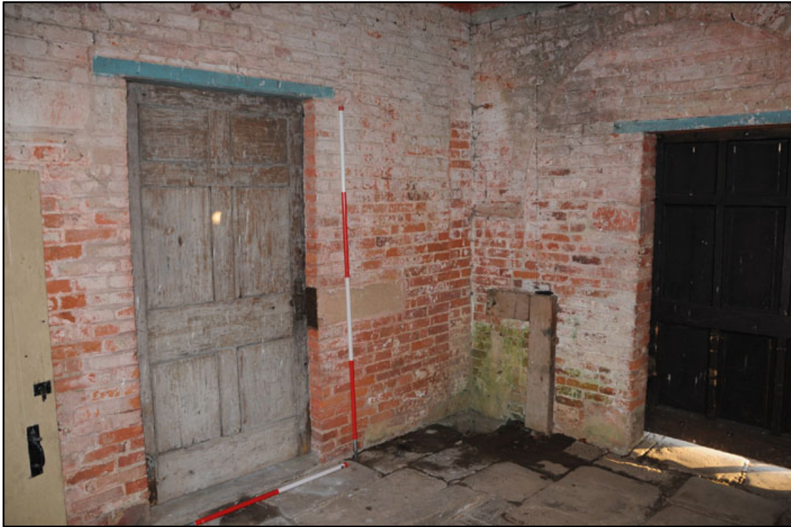
Appendix 2.39: General view of southeast corner of G2; note blocked arch and vertical joint in brickwork (1 m/2m scale).
