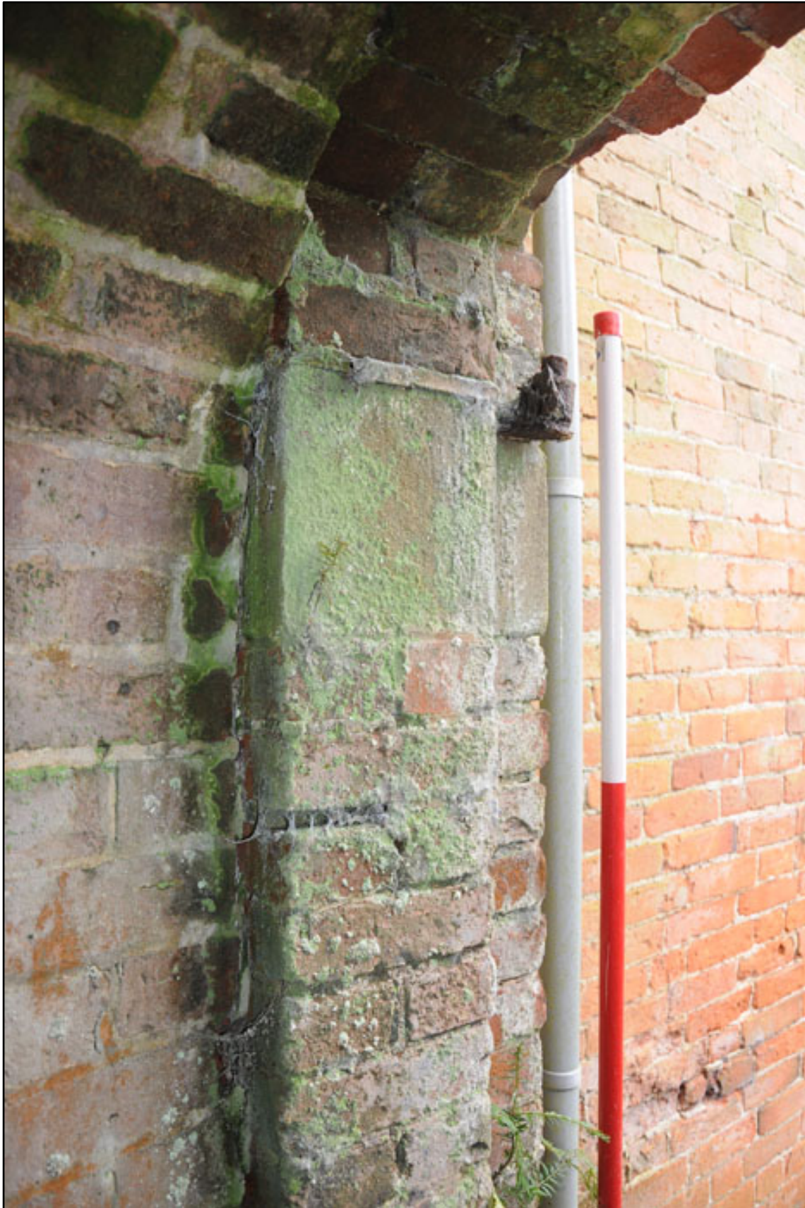
Appendix 2.72: Detail of entrance into Ice House; note that the ceiling arch is below that of the exterior doorway (2m scale).
