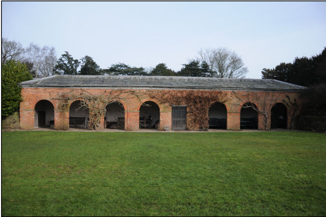
Appendix 2.1: General view of south façade of South Range, looking north (2m scale).
