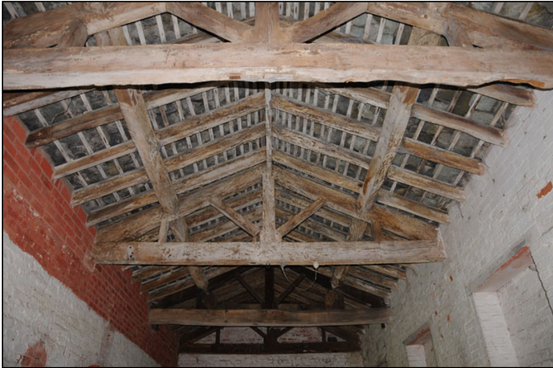
Appendix 2.56: General view of roof construction in G3, looking west.
