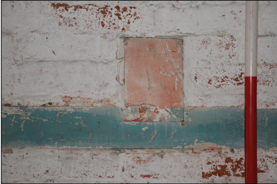
Appendix 2.31: Detail of sawn off timber in walling between A3 and A4 in G1; note how timber is integral to wall beam.
