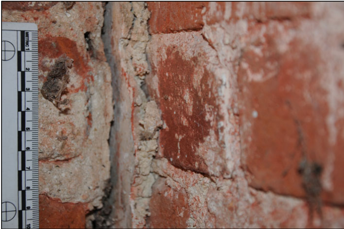
Appendix 2.43: Detail of plaster continuing behind inserted west wall of G2 (10cm scale).
