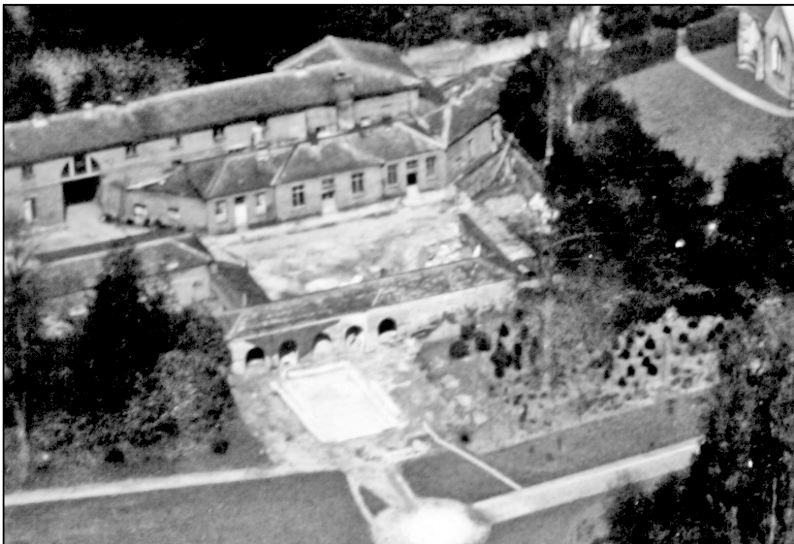
Appendix 1.14: Enlargement of aerial photograph from the southwest of Kedleston Hall, c.1930
