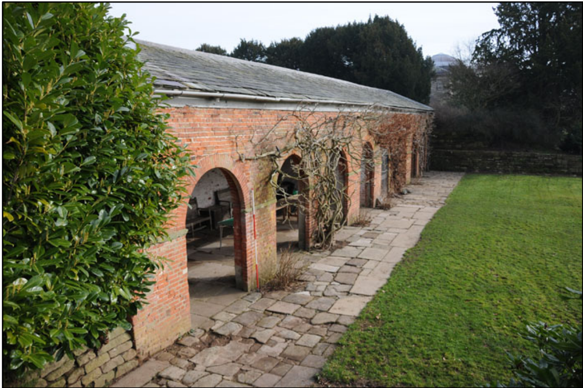
Appendix 2.3: General view of south façade of South Range, looking northeast (2m scale).
