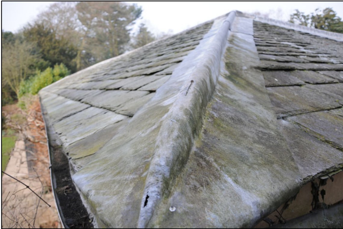
Appendix 2.17: Detail of ridge on hip of southeast corner of roof.
