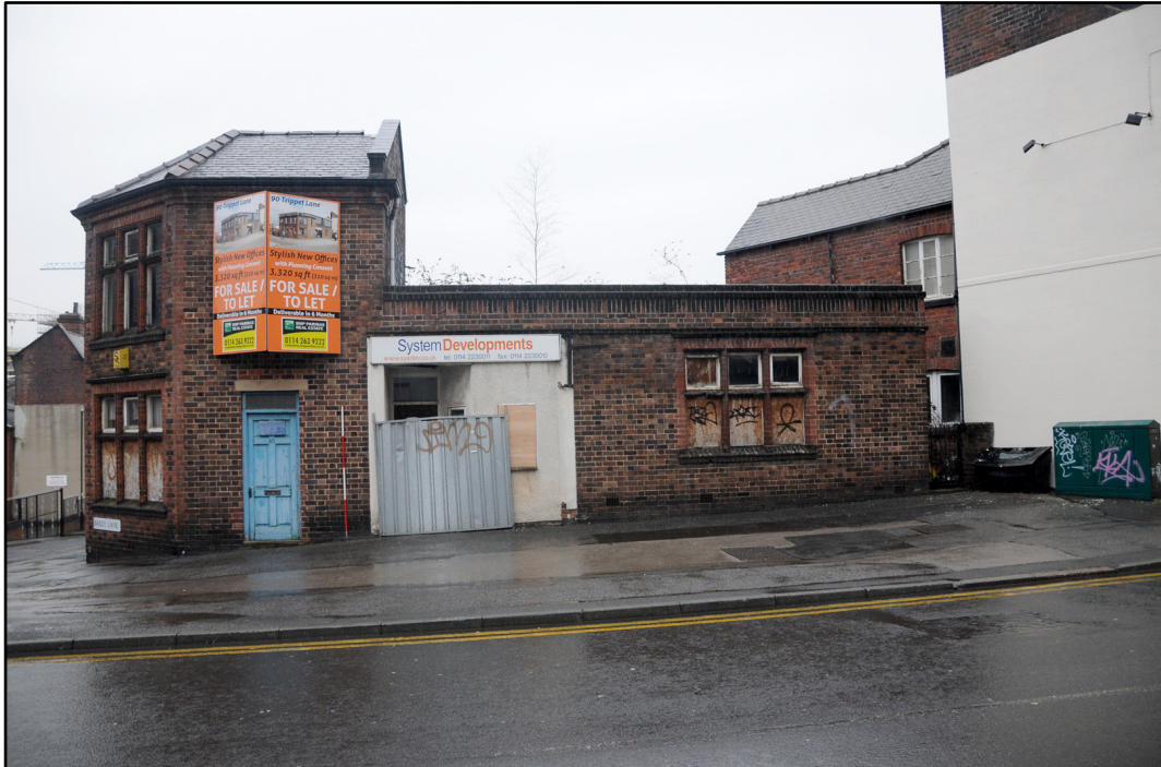
Appendix 3.2: General view of Trippet Lane façade (2m scale).
