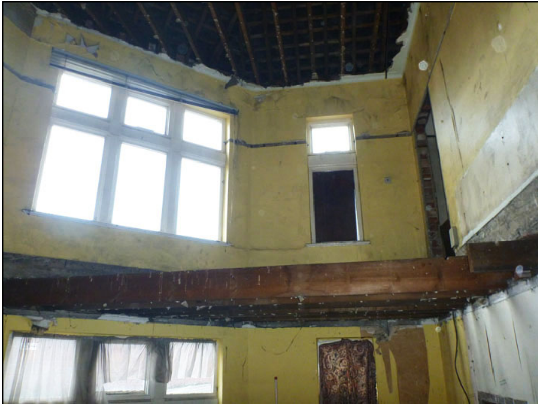
Appendix 3.9: General view of interior of building, note removed flooring.
