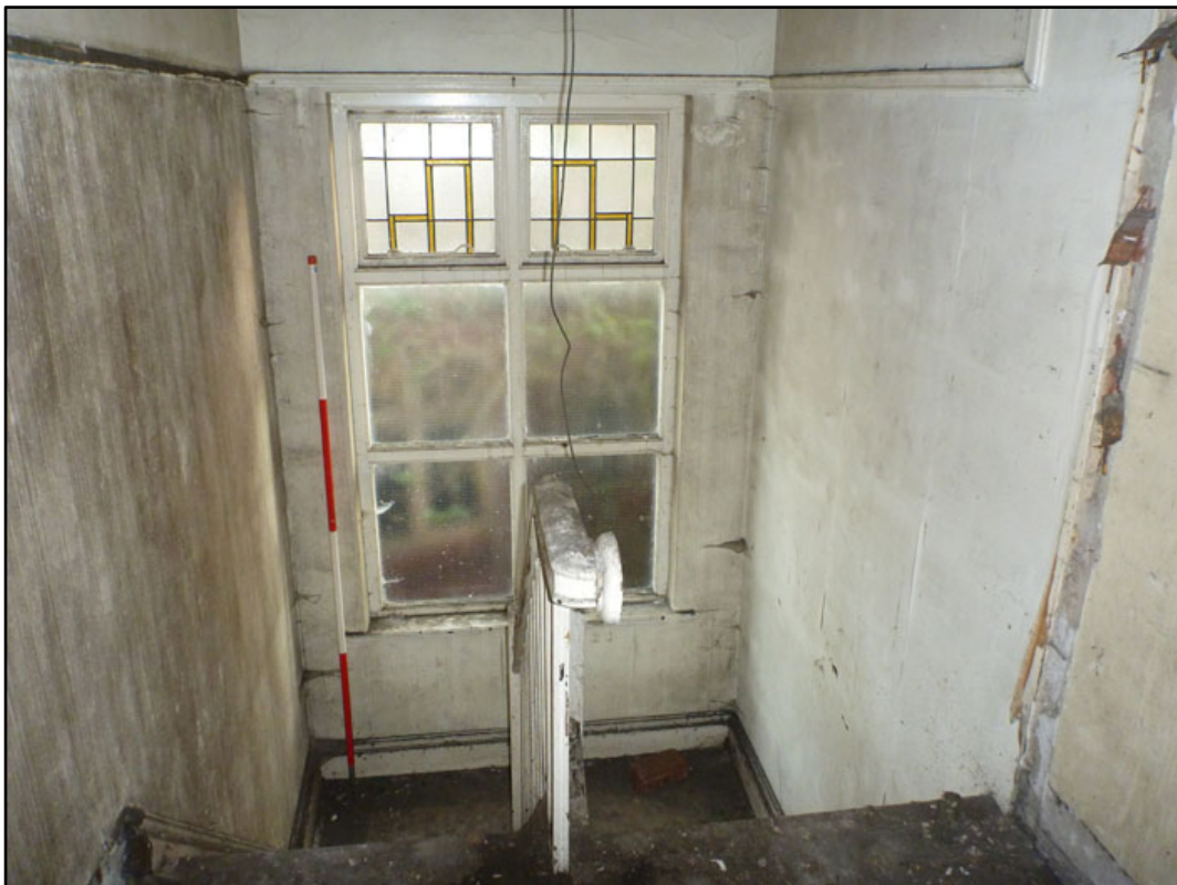
Appendix 3.12: General view of stairwell, looking east (2m scale).
