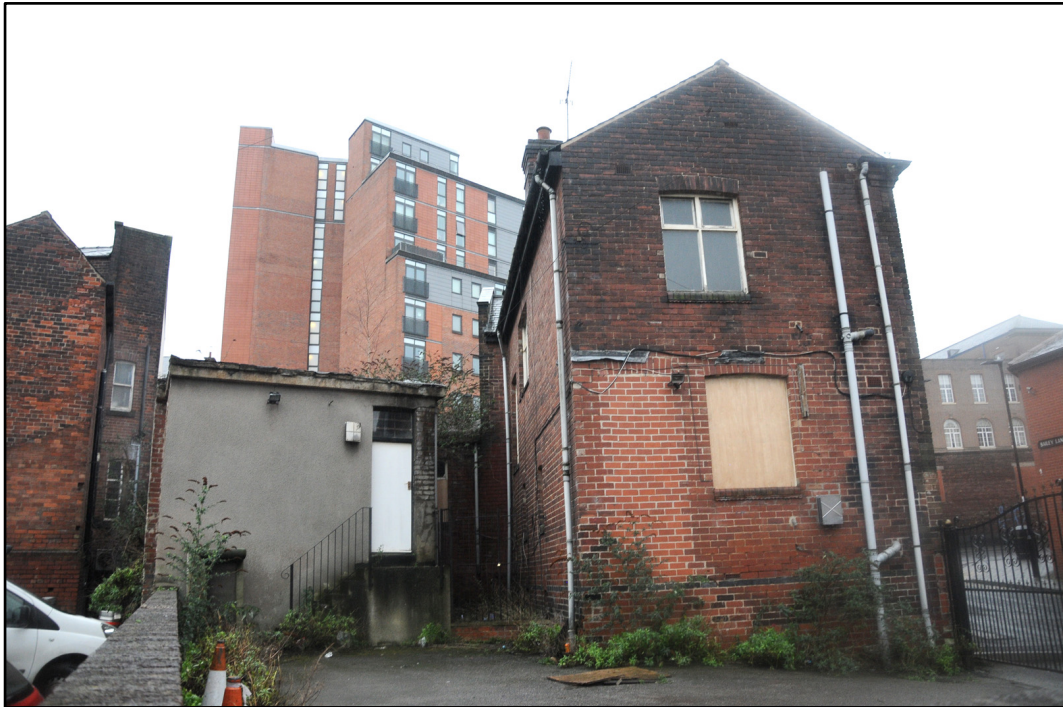
Appendix 3.5: General view of rear of the building, looking south.
