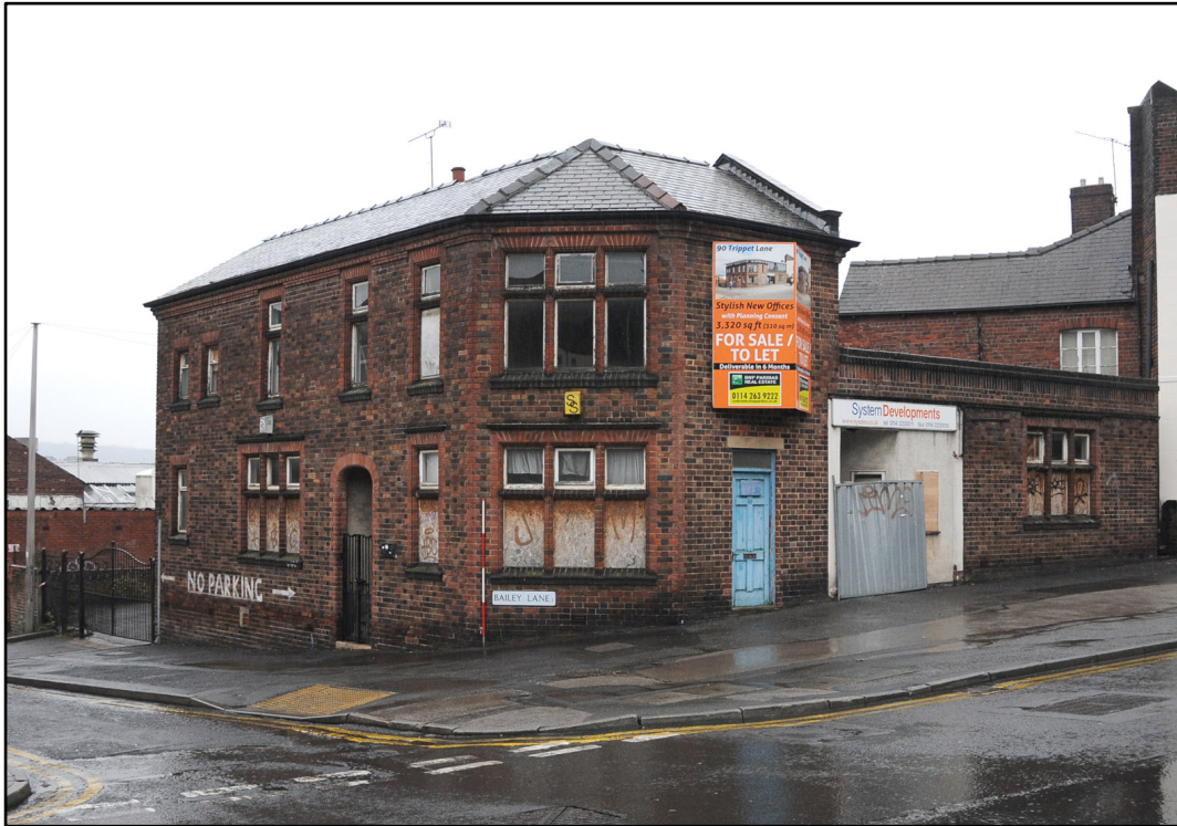
Appendix 3.1: General view of the corner of the building, looking northeast (2m scale).
