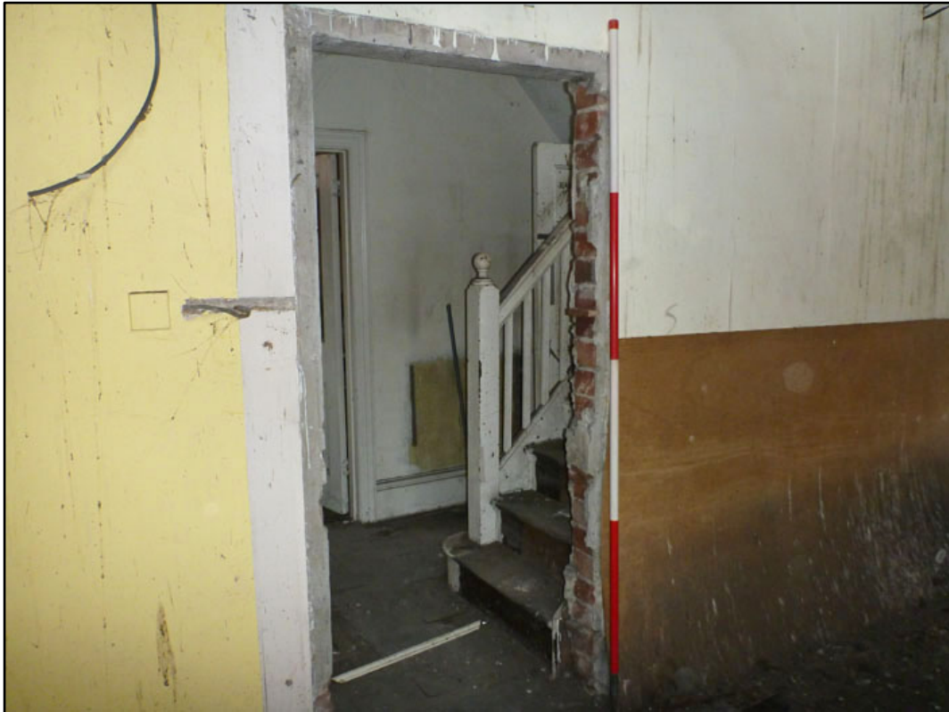
Appendix 3.7: View of ground floor stairwell (2m scale).
