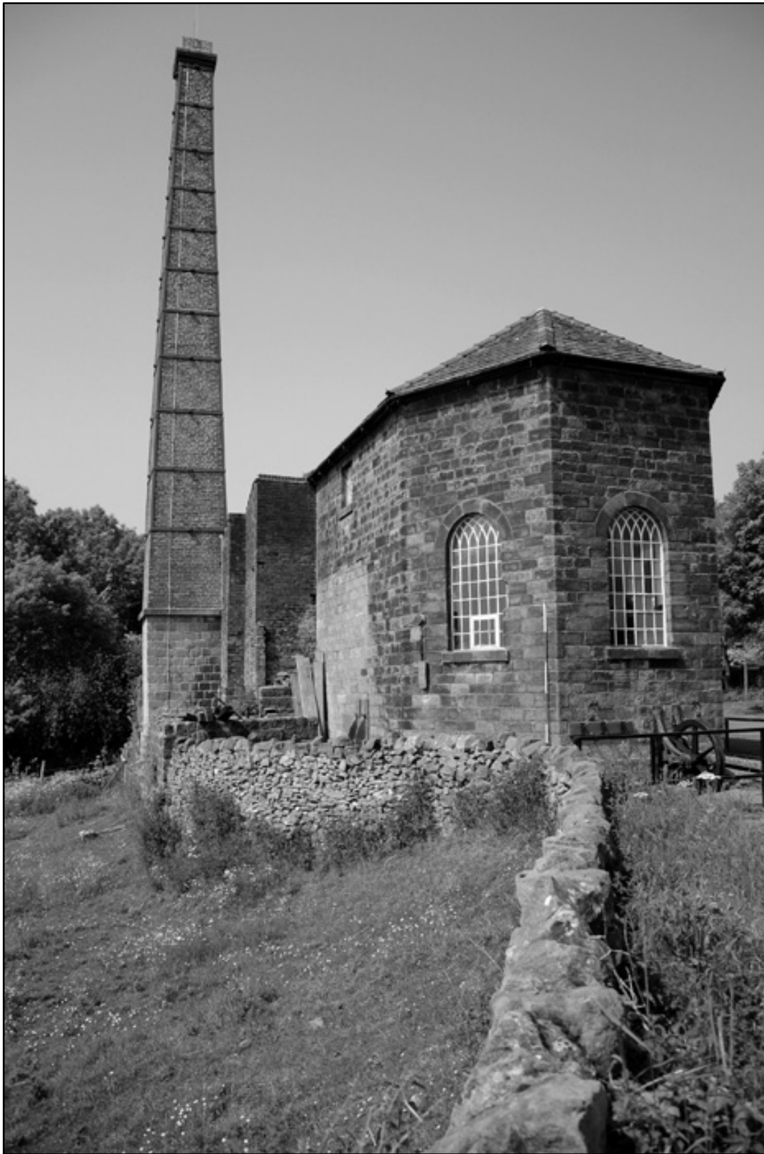
Appendix 2.3: Detail of south side of Winding House and Chimney, looking southwest (3m scale). Film 1.3.
