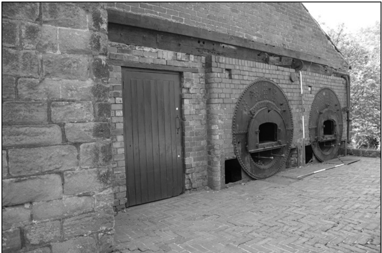
Appendix 2.9: General view of north elevation, looking southwest (2m scale). Film 1.24.
