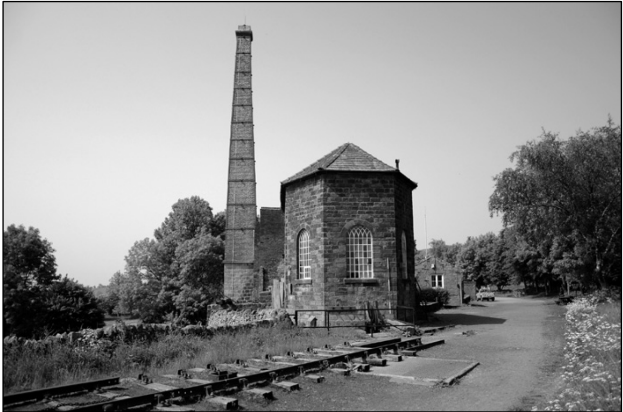
Appendix 2.1: General view of external elevation from top of incline, looking southwest (3m scale). Film 1.2.
