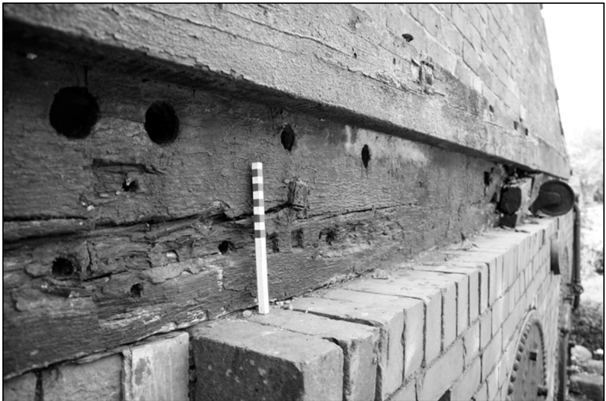
Appendix 2.12: Detail of timber beam along north elevation; note compression scars and bolt holes (20cm scale). Film 1.30.
