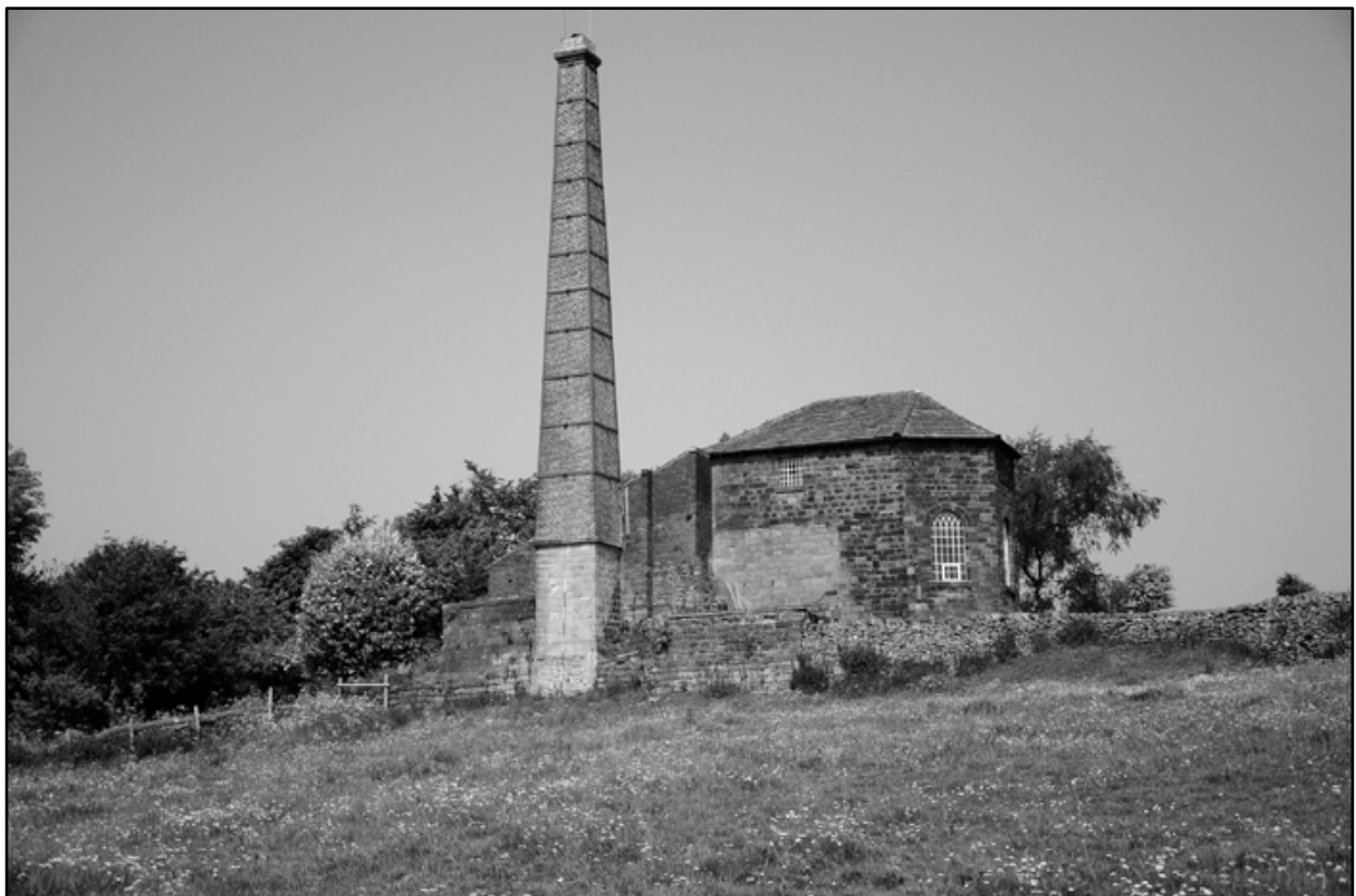
Appendix 2.2: General view of south elevation, looking northwest (3m scale). Film 1.6.
