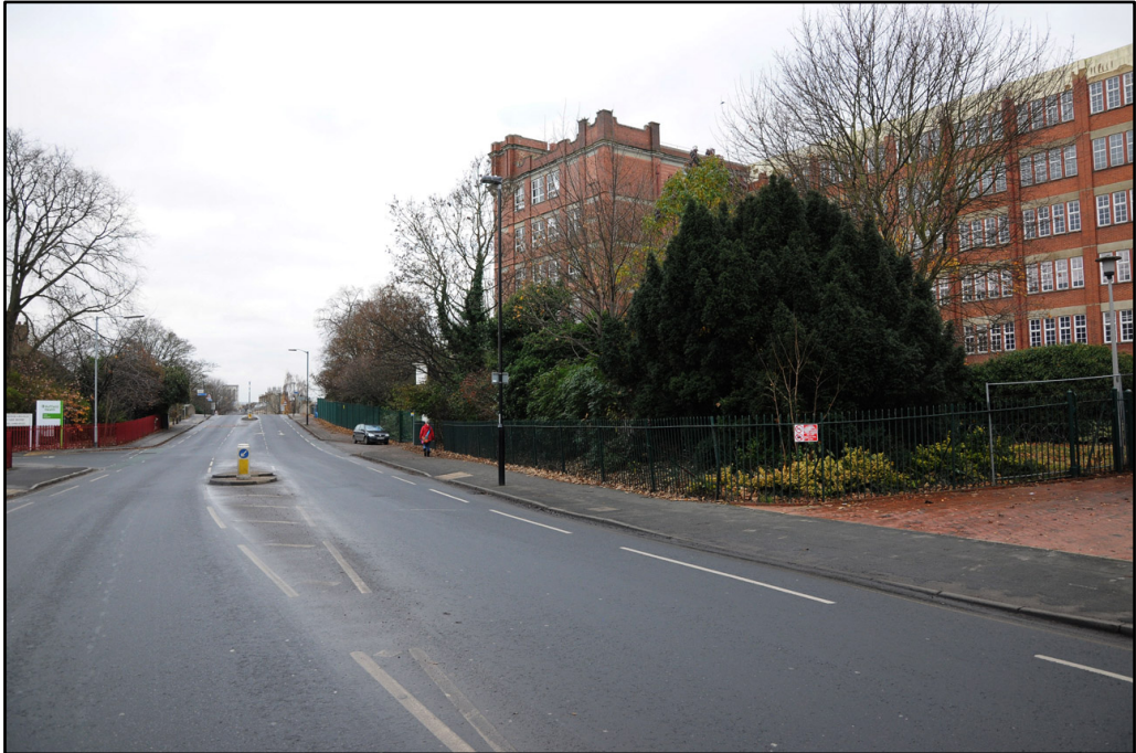
General view looking south along Haxby Road, note extent of railings and overgrown shrubbery
