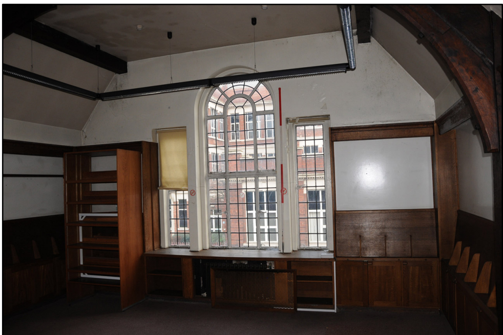
General view of upper floor of Joseph Rowntree Library, looking east (2m scale)
