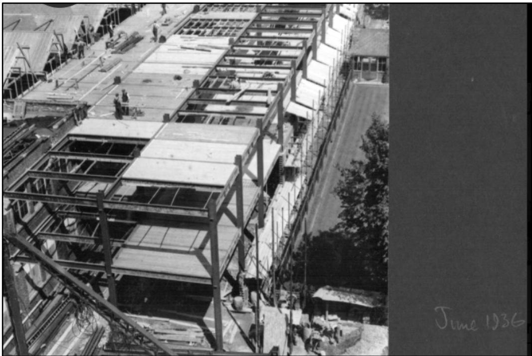
Construction of the Cream Block, June 1936 © Nestle S.A.
