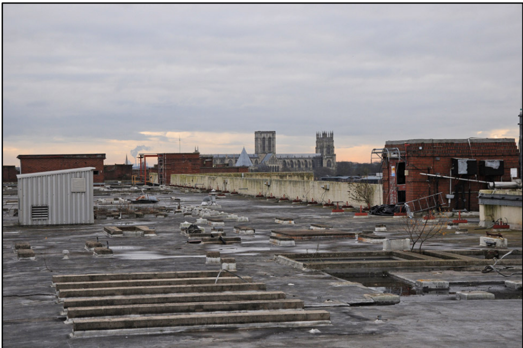
View looking south across flat roof of Cream Block towards York Minster
