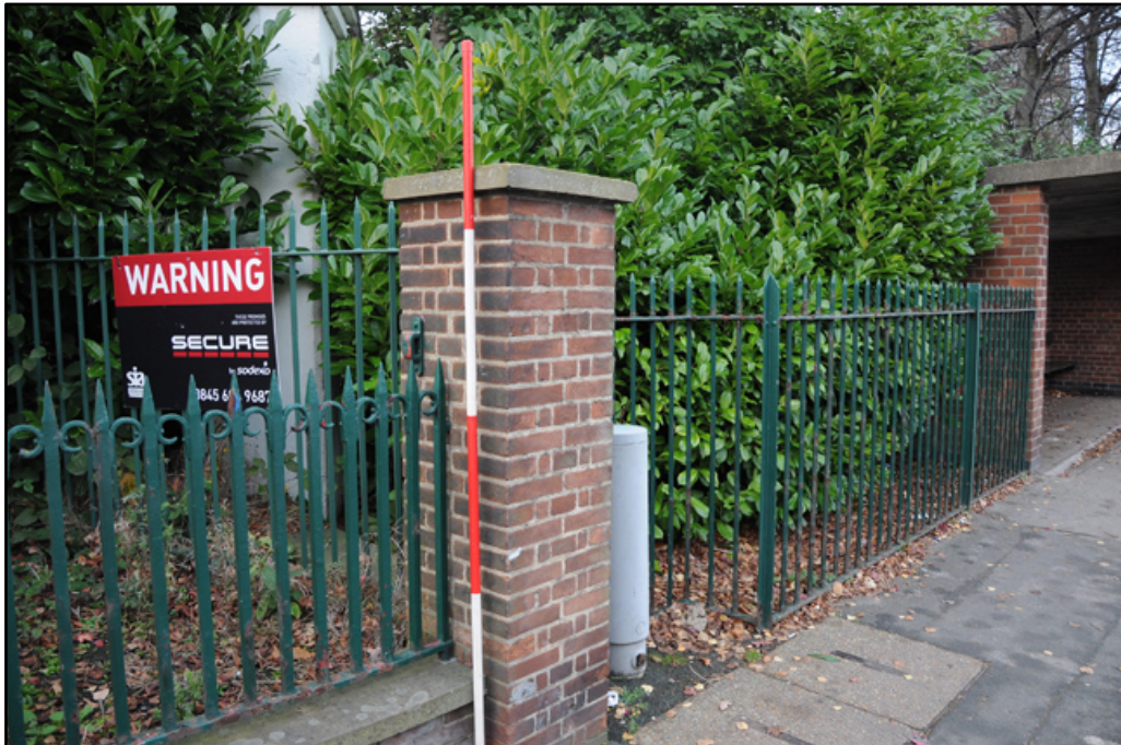
Detail of two styles of iron railing on Haxby Road frontage (2m scale)
