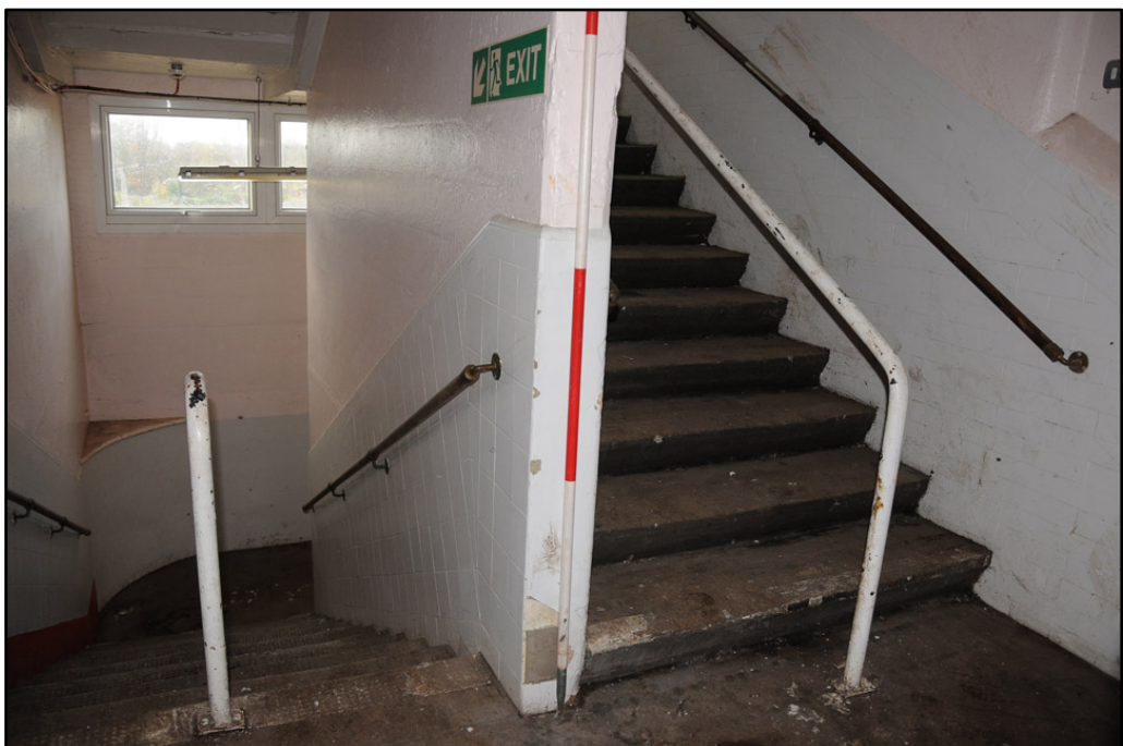
General view of stairwell in north end of Almond Block (scale 2m)
