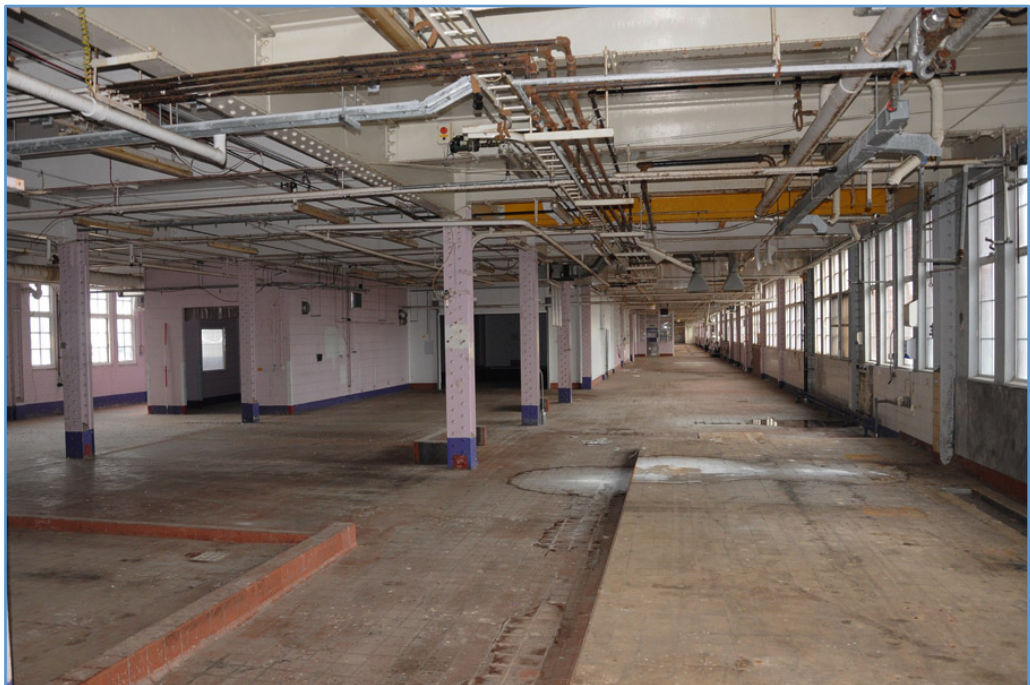
General view of fifth floor of Cream Block, looking north (2m scale)
