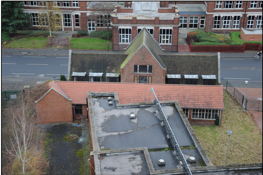
General view from above of subway corridor and Joseph Rowntree Library, looking east
