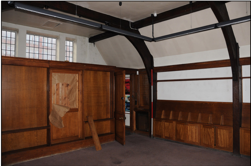
General view of upper floor of Joseph Rowntree Library, looking northwest (2m scale)
