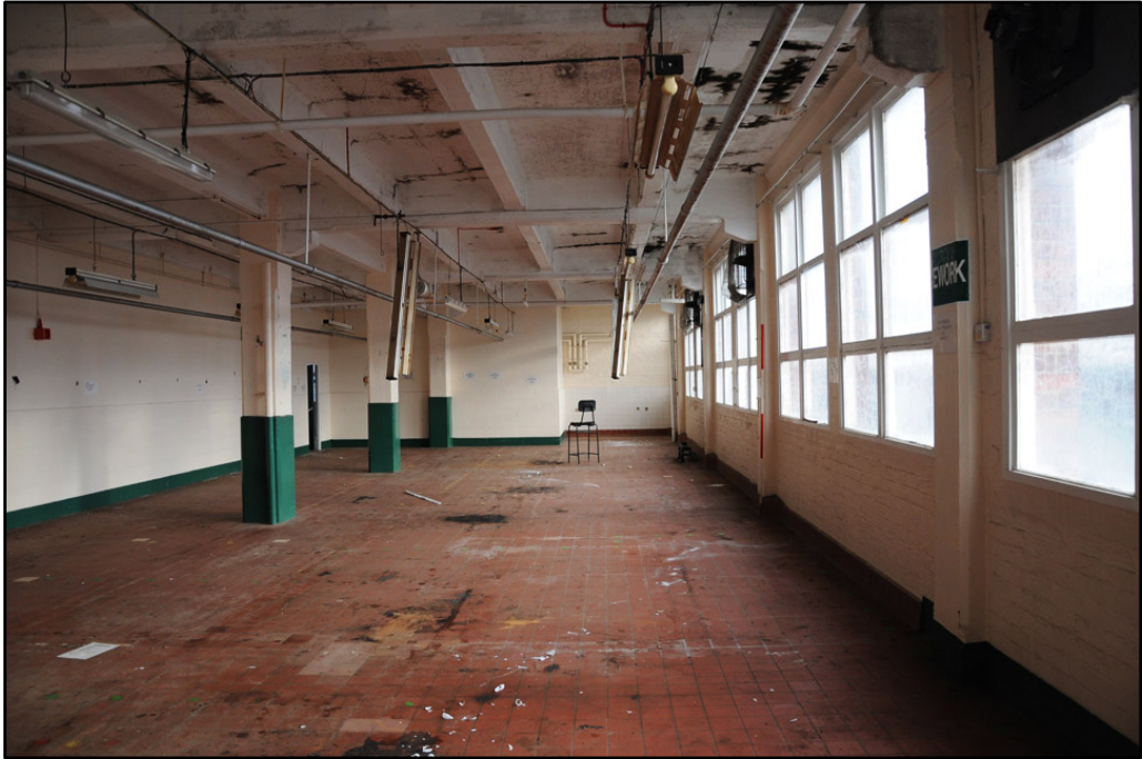
General view of fifth floor of Almond Block; looking east (2m scale)
