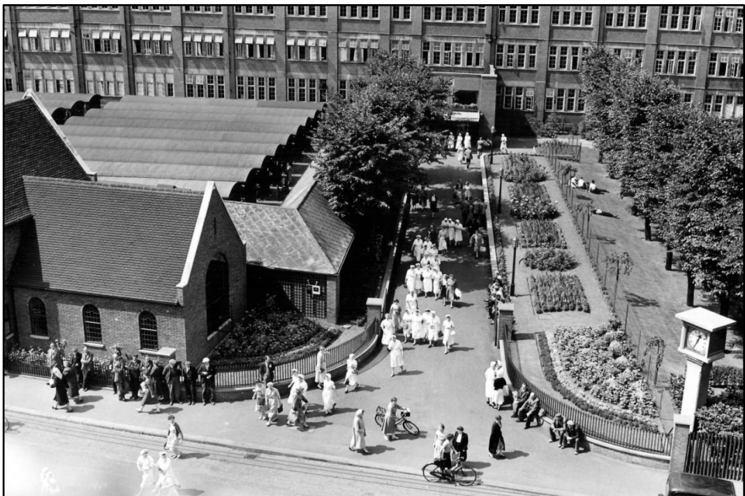
Entrance to Cream Block with gardens © Nestle S.A.
