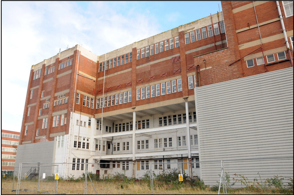
Northwest section of 1938 extension of Almond Block; note recessed 1936 building below
