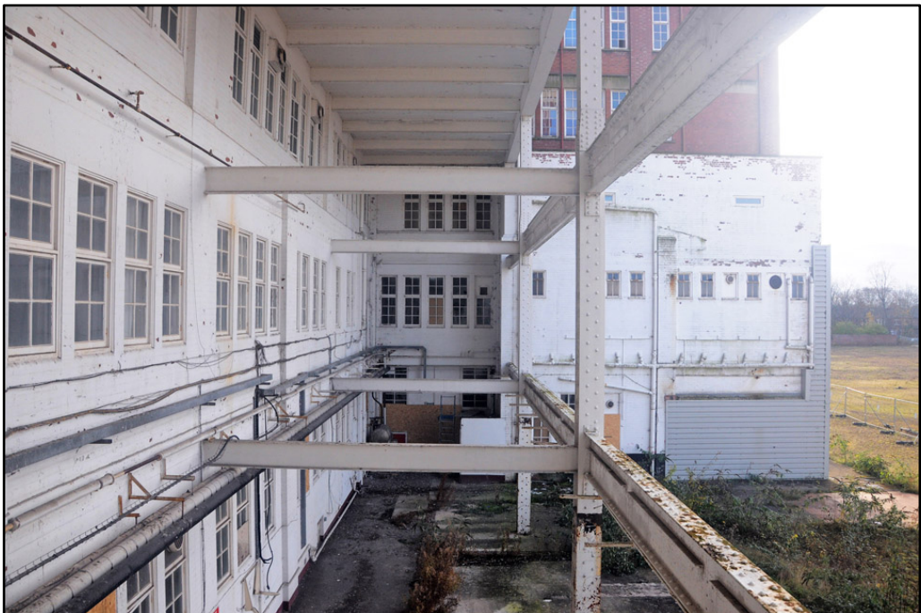
Detail of original window frames in 1936 block with 1938 steelwork above
