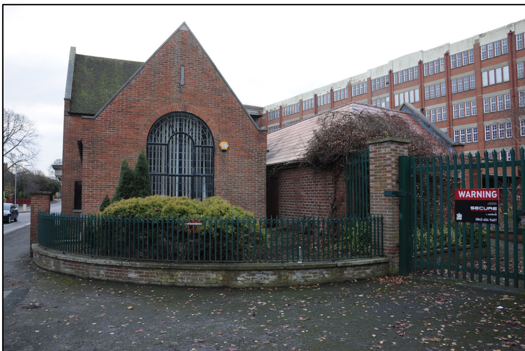
General view of north gable of Joseph Rowntree library looking south; note modern security gates
