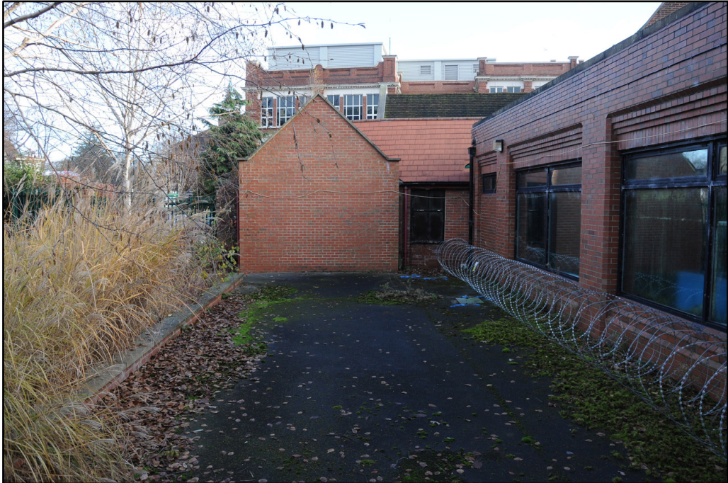
View of brick gable built following demolition of north wing of the connecting corridor
