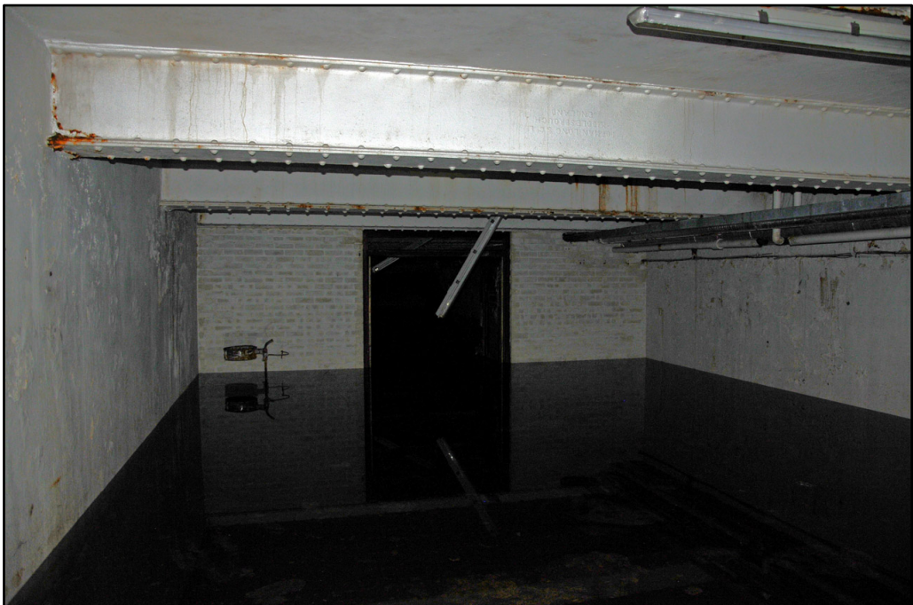
General view of flooded subway passage beneath Joseph Rowntree Library; note riveted box girders
