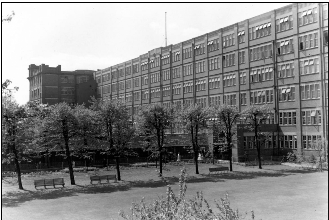
Completed (north section) of the Cream Block; note gardens in foreground © Nestle S.A.
