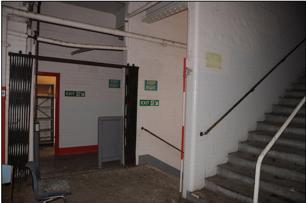
Detail of south stairwell on fifth floor of Cream Block; note sliding door gate (2m scale)
