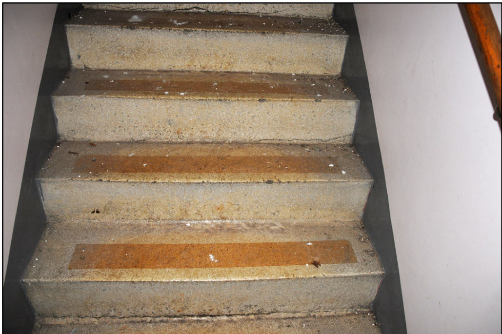
Detail of terrazzo treads on 1936 staircase in Cream Block
