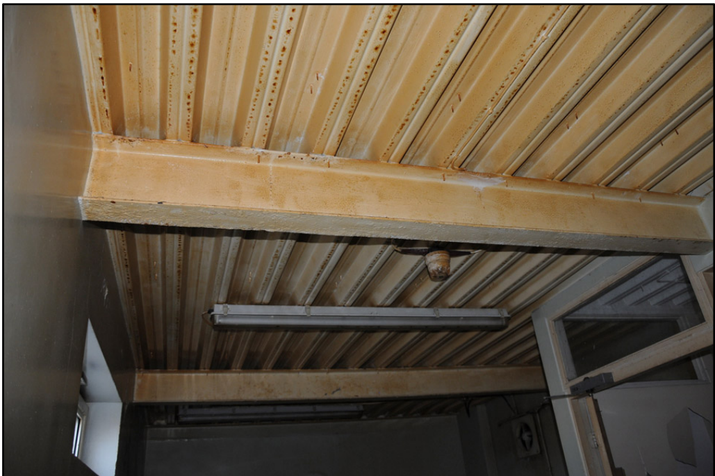
Detail of secondary sheet metal ceiling in rear extension of Cream Block; possible air-raid protection
