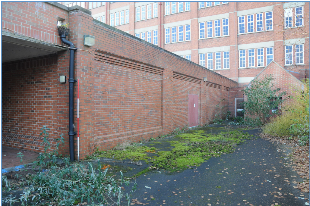
General view of north wall of amenity block; note bricked up gable of former access corridor (2m scale)
