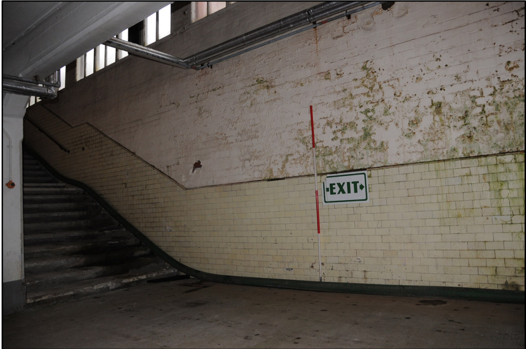
View looking up subway steps beneath Joseph Rowntree Library (2m scale)
