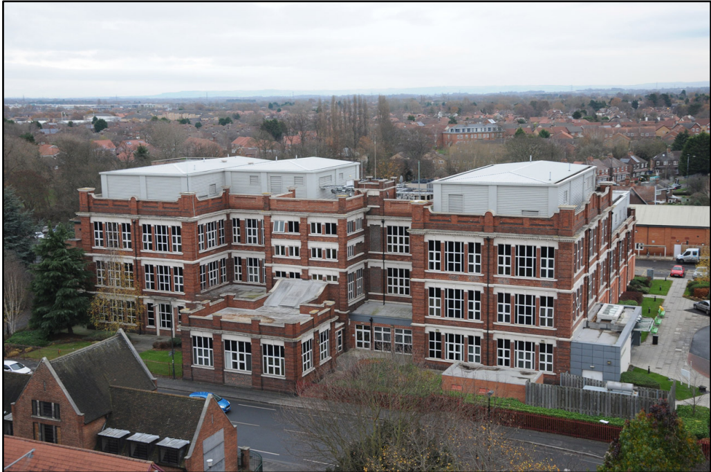
View of Nuffield Hospital on east side of Haxby Road, (former dining rooms and class rooms)
