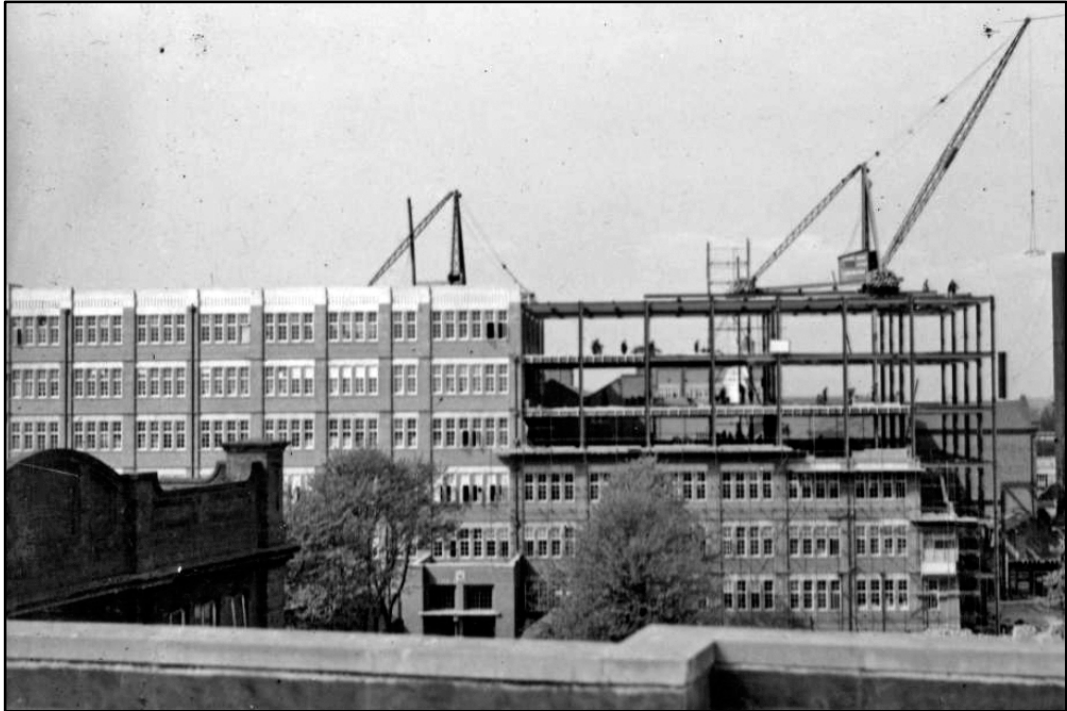
Construction of the Cream Block (south section), c.1938 © Nestle S.A.
