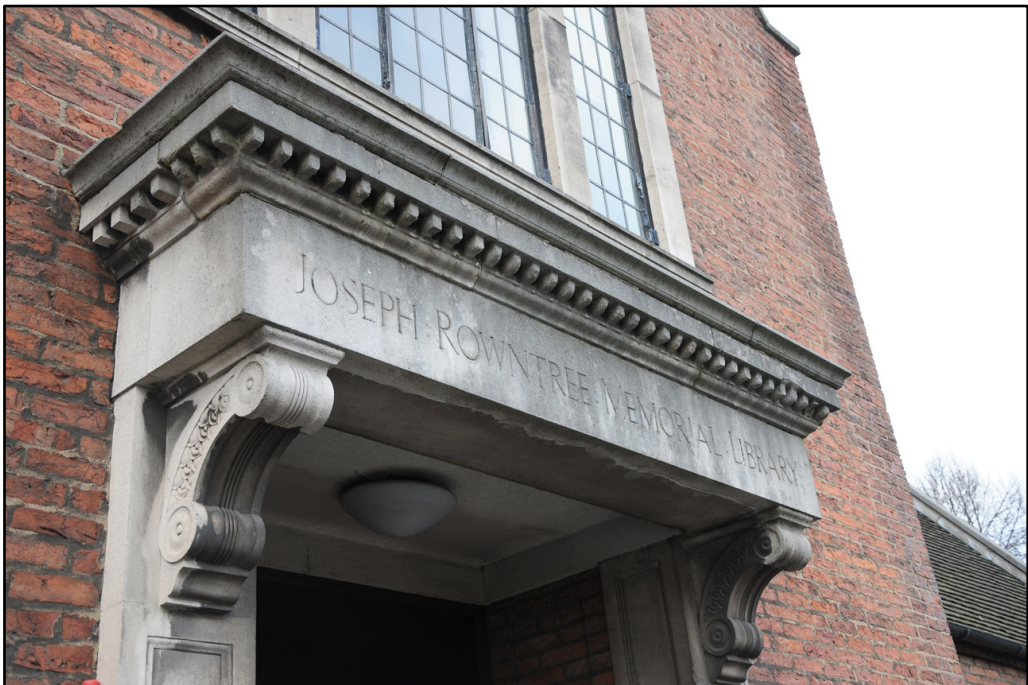
Detail of entrance porch to Joseph Rowntree Library
