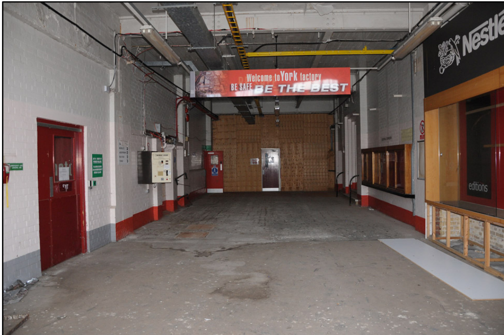
General view of main entrance corridor at north end of 1936 Cream Block
