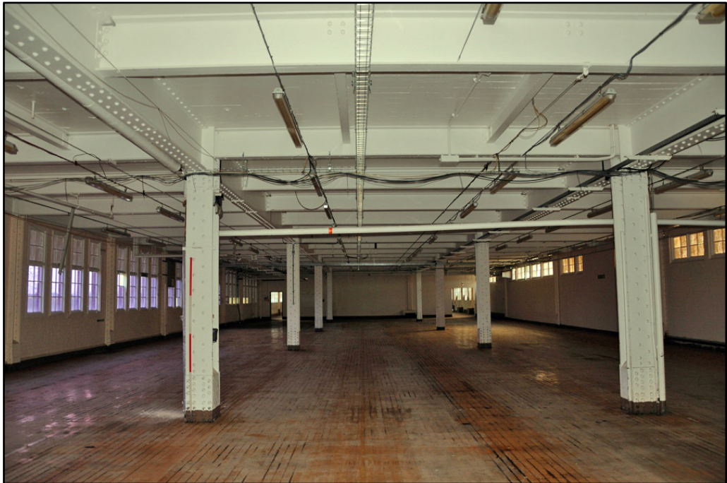
General view of north end of third floor of Cream Block, looking south (2m scale)
