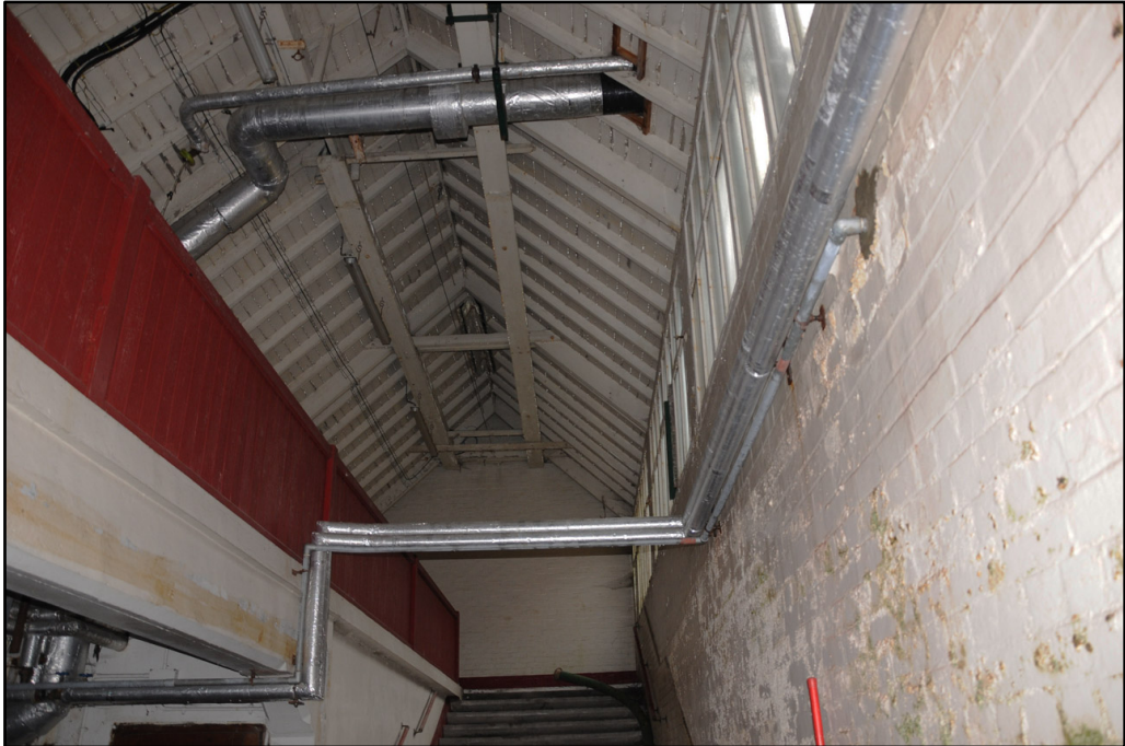
Detail of exposed timberwork roof above subway corridor
