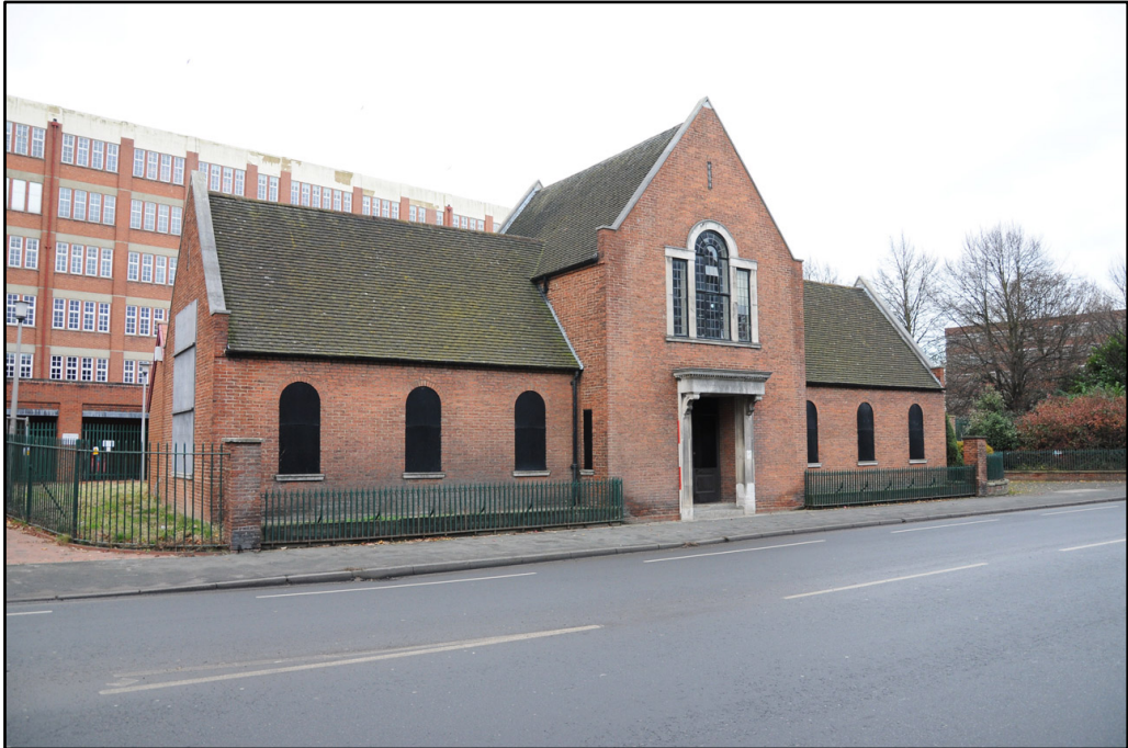
General view of Joseph Rowntree Library looking northwest (2m scale)
