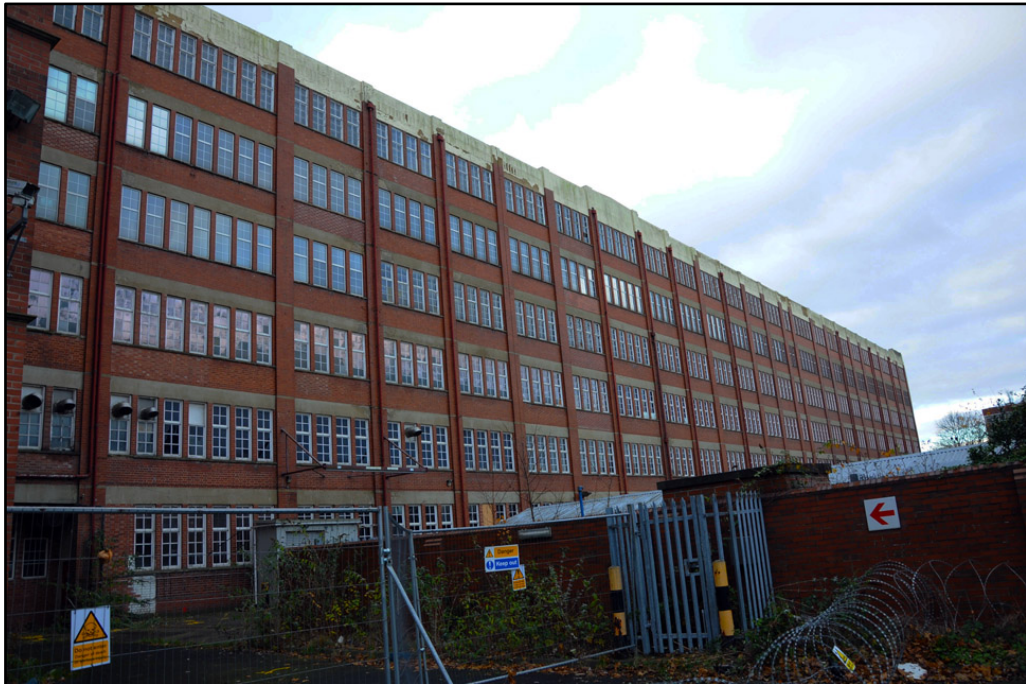
General view of east elevation of Cream Block, looking northwest
