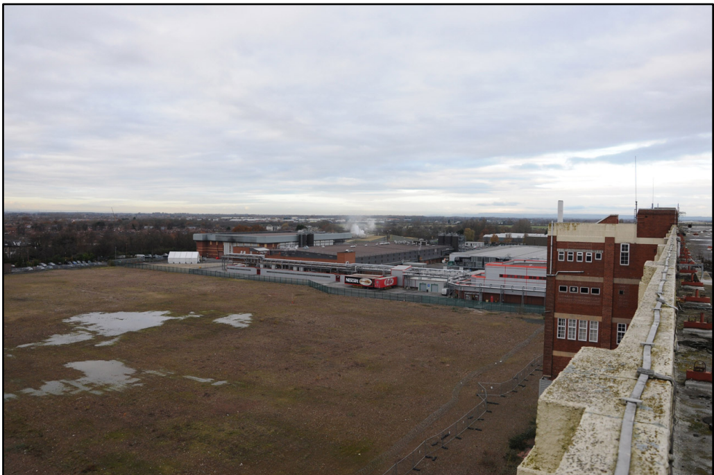
View of land to the west of the Cream Block following clearance of the associated factory buildings
