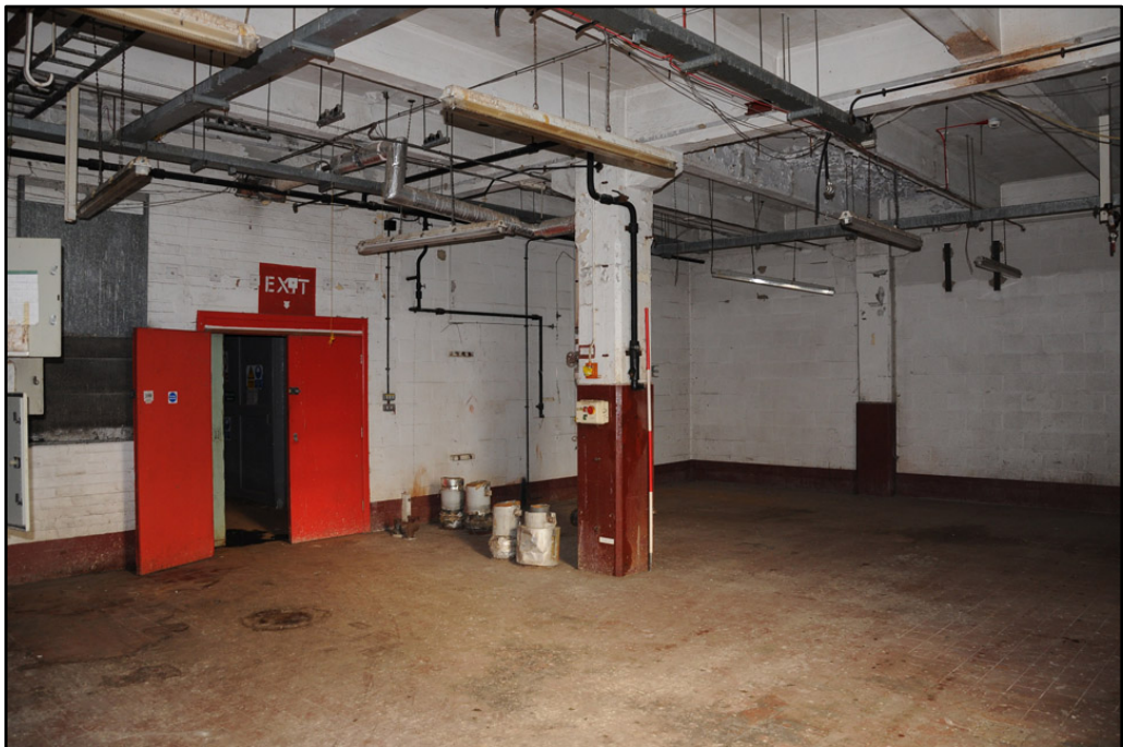
General view of west end of forth floor of Almond Block, looking northeast (2m scale)
