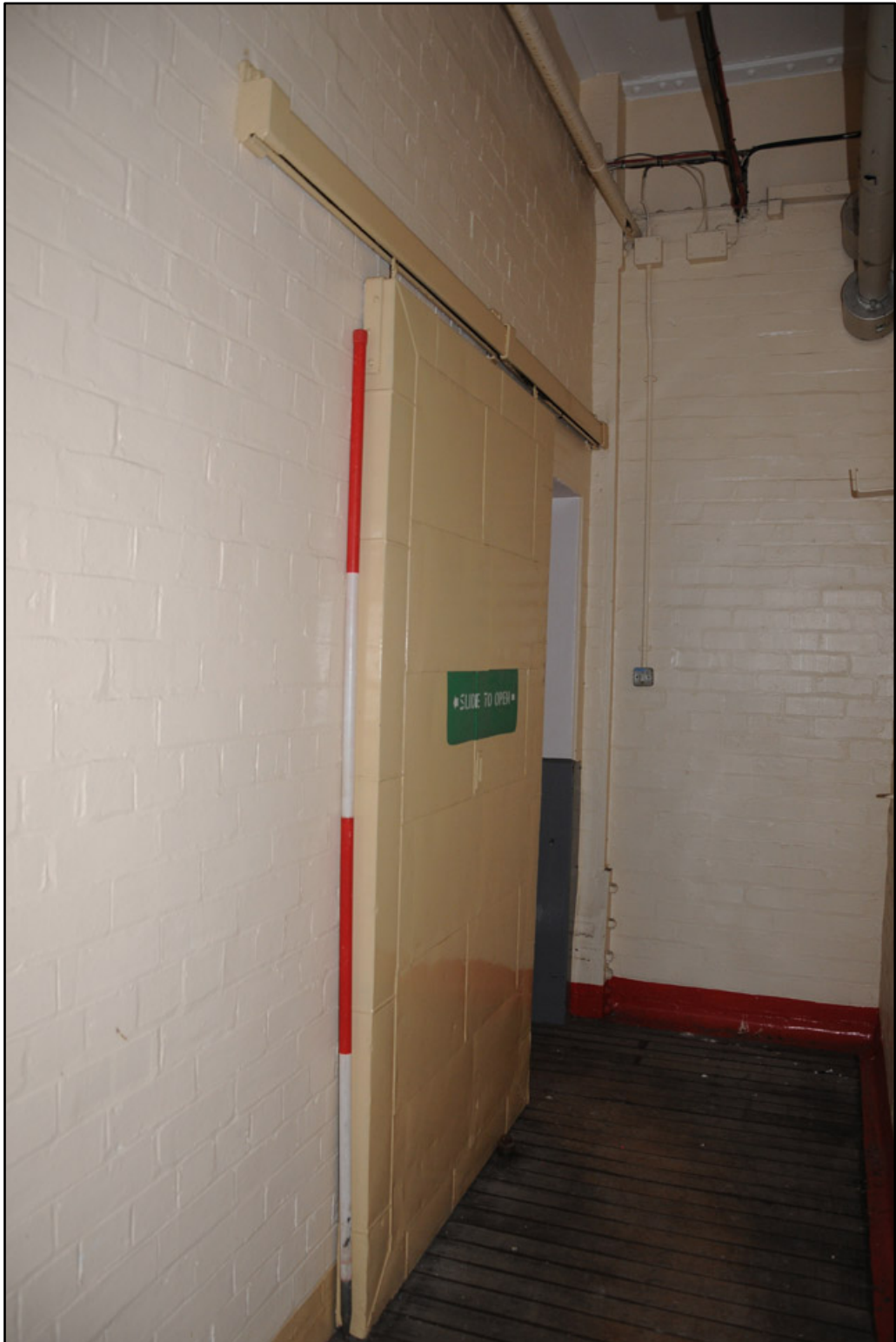
Detail of sliding metal door on fourth floor of Cream Block (2m scale)
