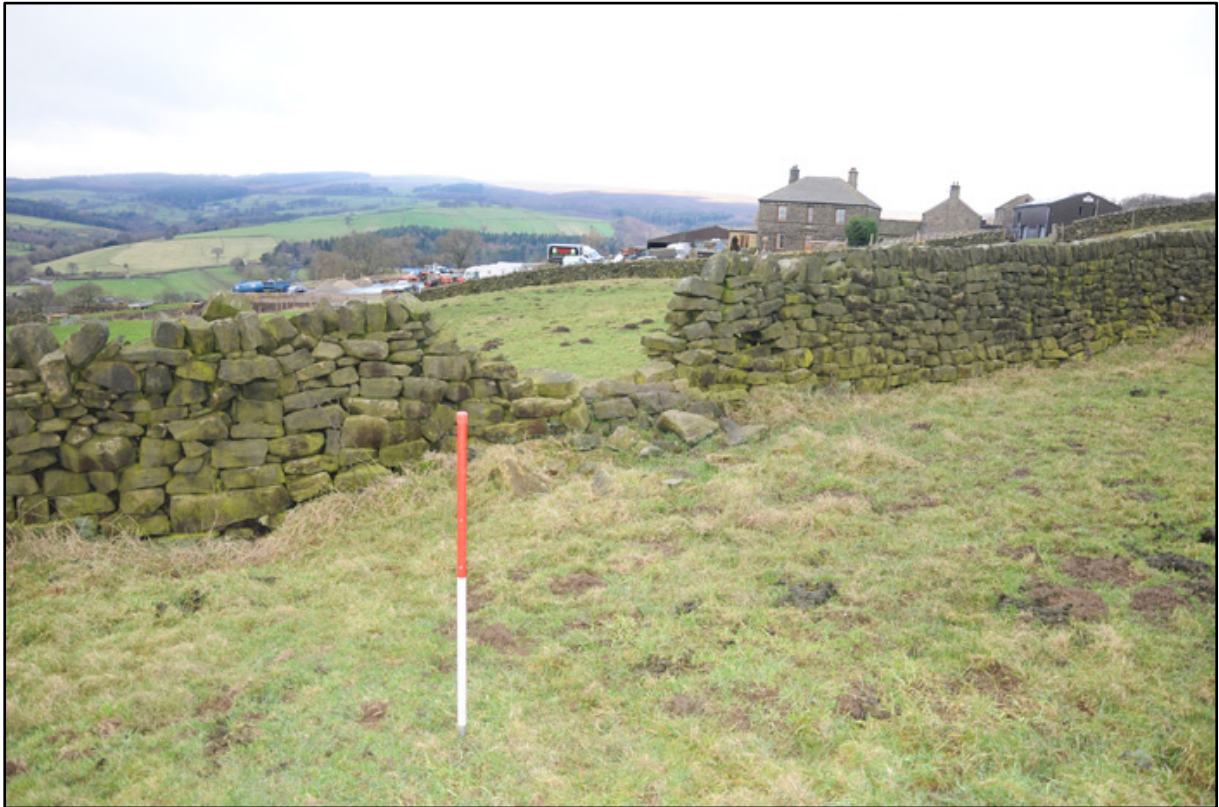
Appendix 3.11: Detail of raised causeway truncated by diagonal wall between fields F2, F3, looking west (1m scale).
