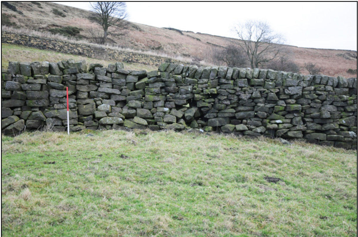
Appendix 3.12: Detail of straight joint and blocking in central section of diagonal wall between fields F2, F3 (1m scale).
