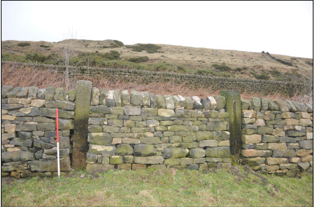
Appendix 3.5: Detail of blocked gateway in boundary wall along Loxley Road at north edge of field F2 (1m scale).
