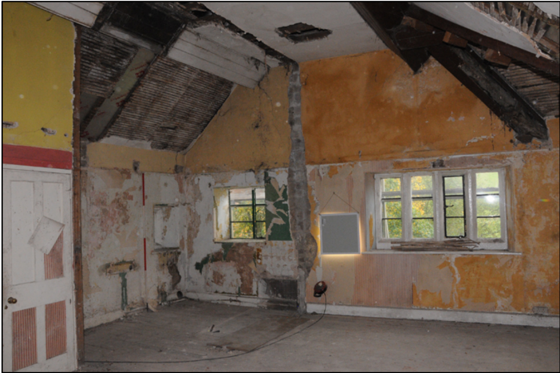
Appendix 5.46: General view of room F2, looking northeast (2m scale)
