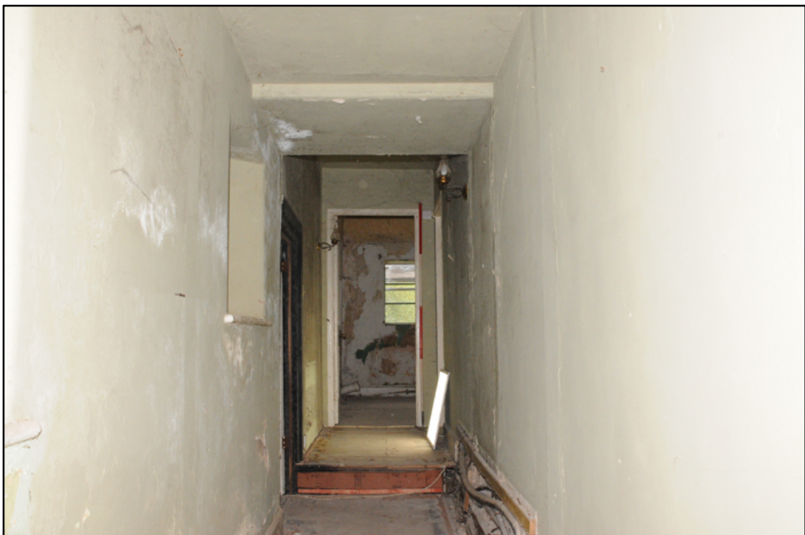
Appendix 5.41: General view looking east along corridor F4 (phase 7) (2m scale)
