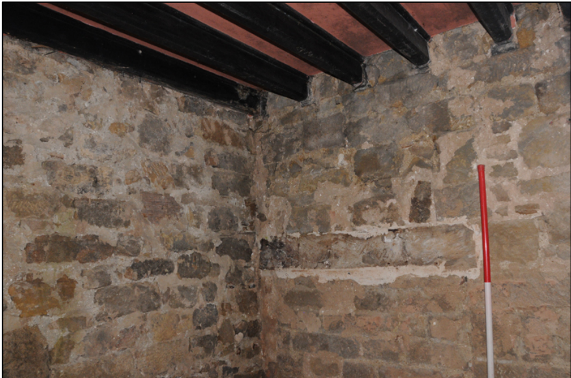
Appendix 5.35: General view of southeast corner of G5; note blocked opening into G2 (2m scale)
