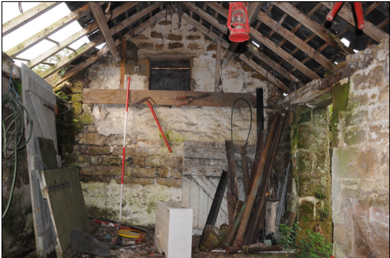
Appendix 5.57: General view of interior of piggyery, looking west (2m scale)
