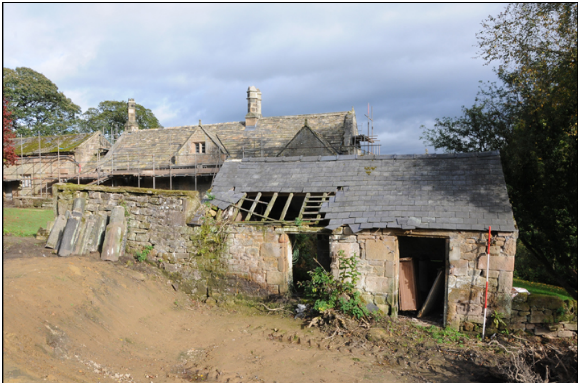
Appendix 5.55: Detail of south elevation of piggyery, looking north (2m scale)
