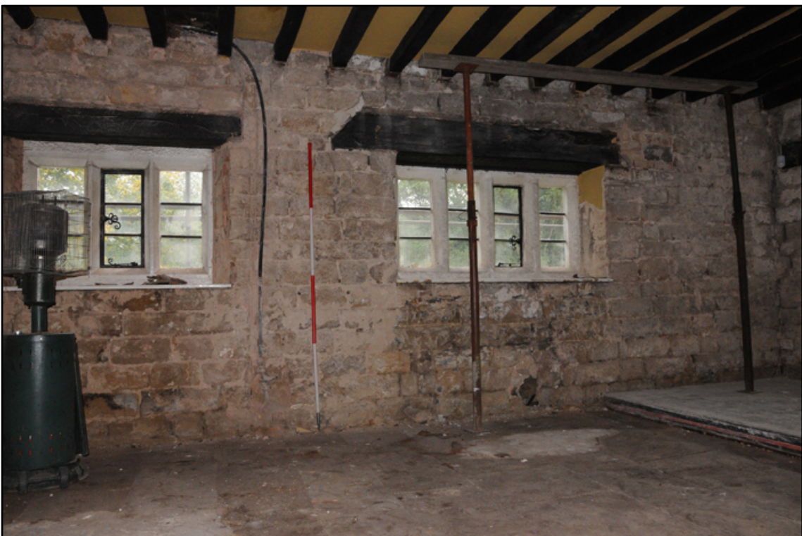
Appendix 5.23: General view of east wall of G2; note inserted (phase 8) left hand window (2m scale)
