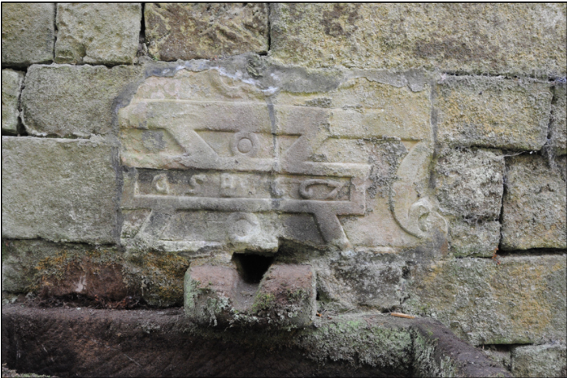
Appendix 5.8: Detail of re-used datestone '1667' above water trough opposite the doorway into G2.
