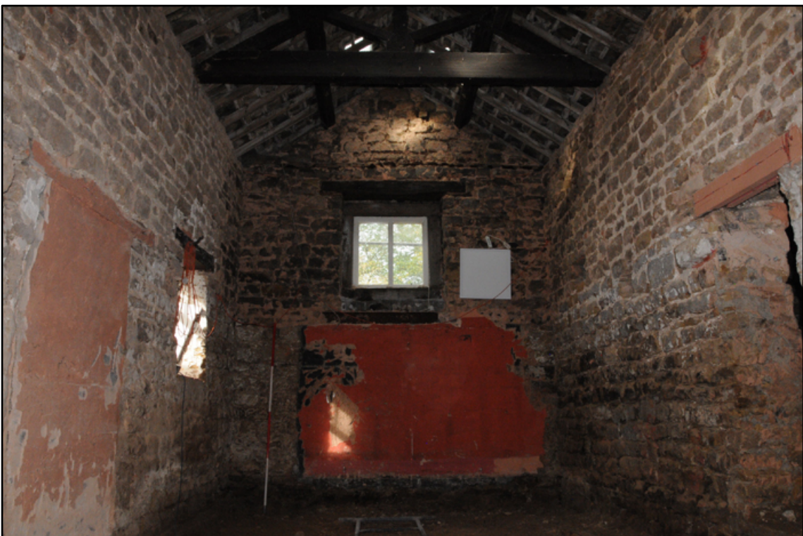
Appendix 5.63: General view of west end of G4; note inserted first floor window (2m scale)
