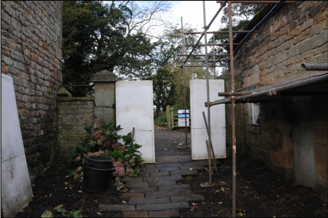
Appendix 5.52: General view of main entrance to yard, looking west; note blocked pedestrian doorway
