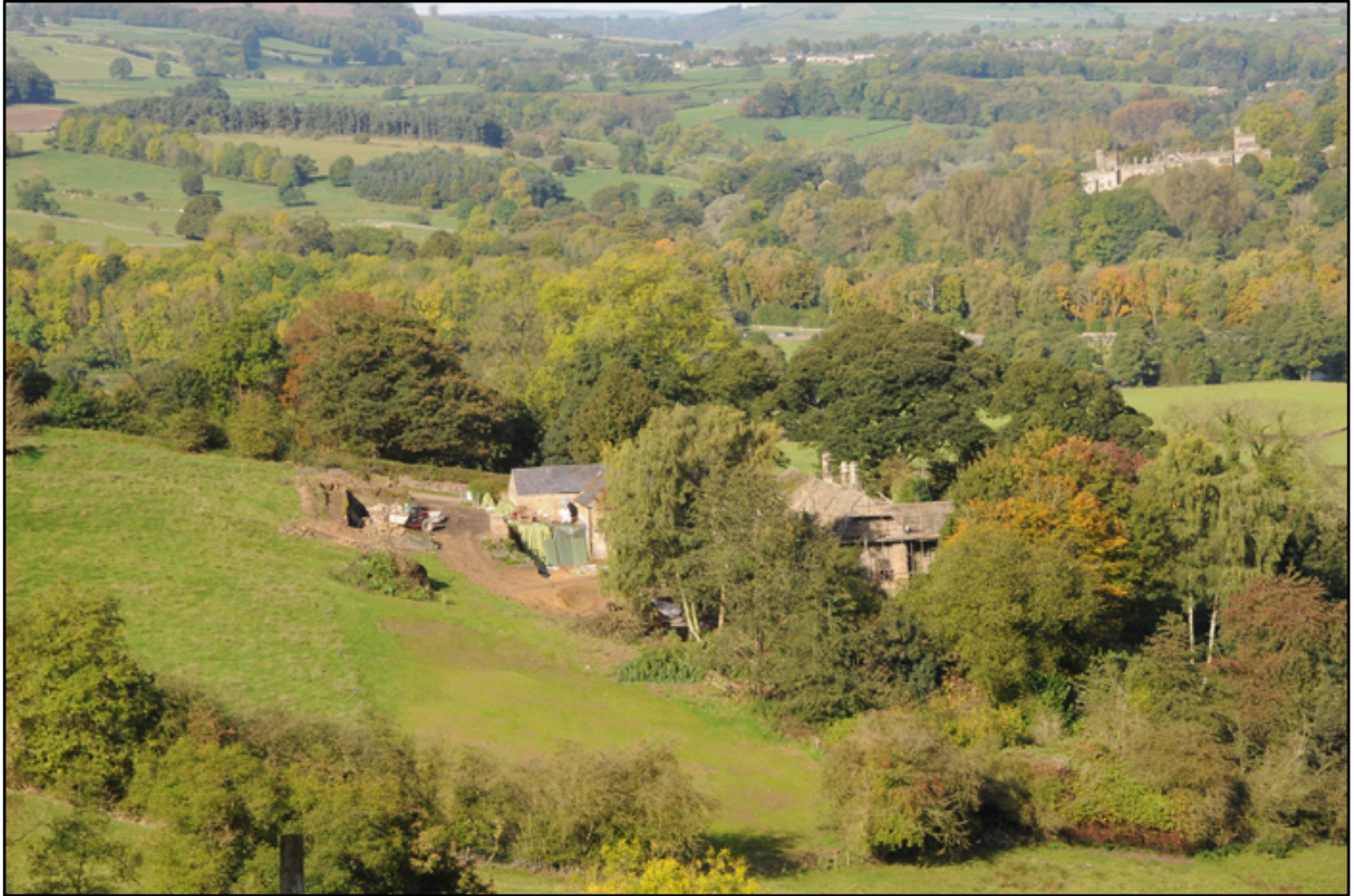
Appendix 5.1: General view of Stanton Old Hall, looking north (Note Haddon Hall in background)
