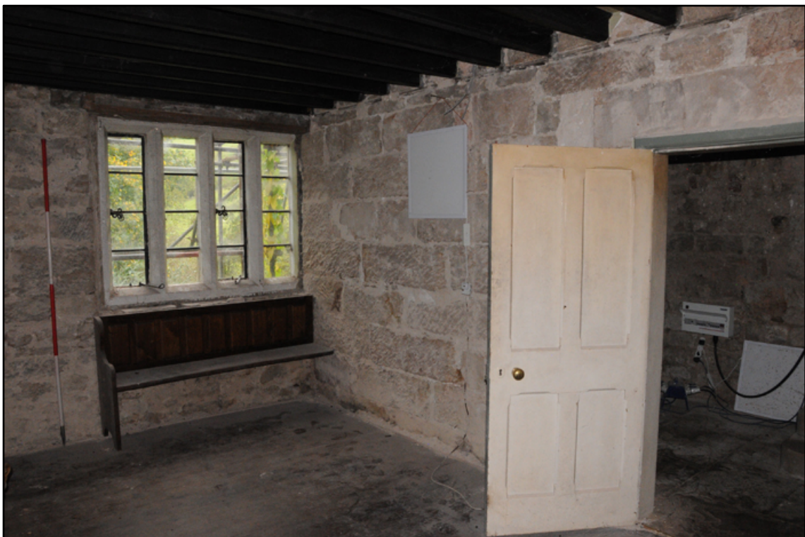
Appendix 5.33: General view of east wall of G7 (2m scale)
