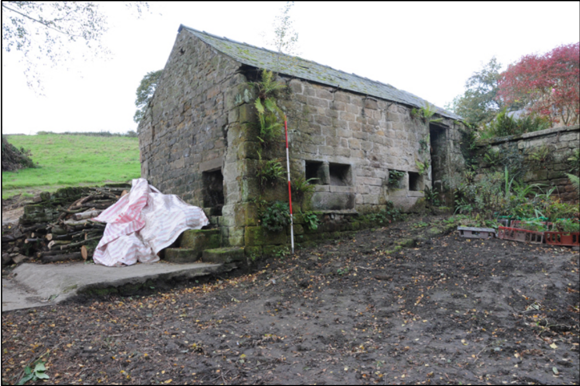
Appendix 5.56: General view of northeast corner of piggyery, looking southwest; note feeding chutes (2m scale)
