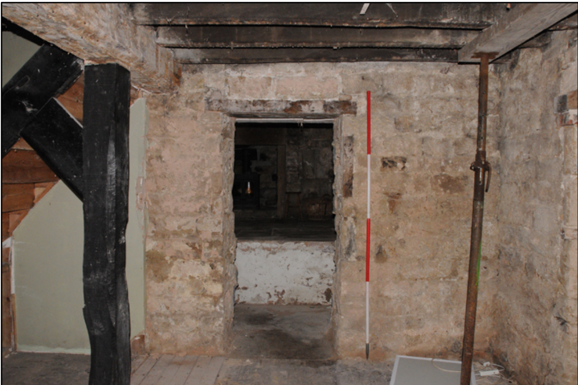
Appendix 5.17: Detail of inserted doorway (phase 7) in west wall of GI, looking west (2m scale)
