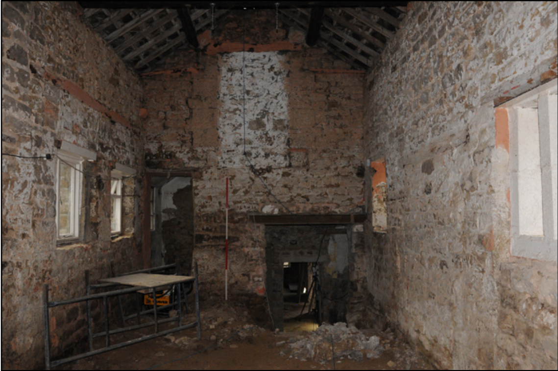
Appendix 5.64: General view of east end of G4 ; note blocked first floor doorway (2m scale)
