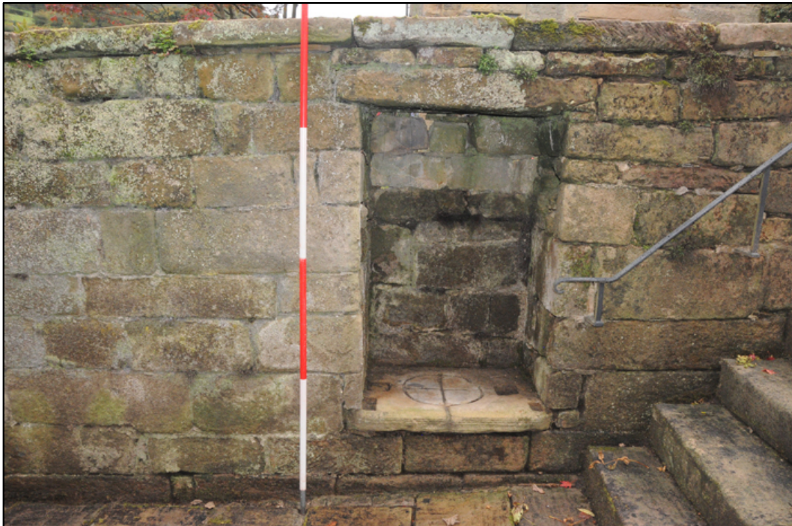
Appendix 5.6: Detail of recess for cheese press in retaining wall along south side of hall (2m scale)
