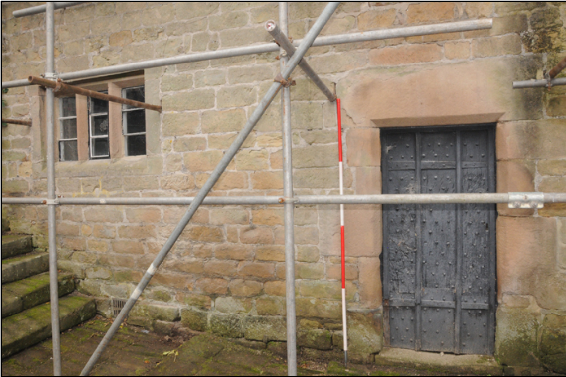
Appendix 5.9: Detail of doorway (phase 1) into room G1 (2m scale)
