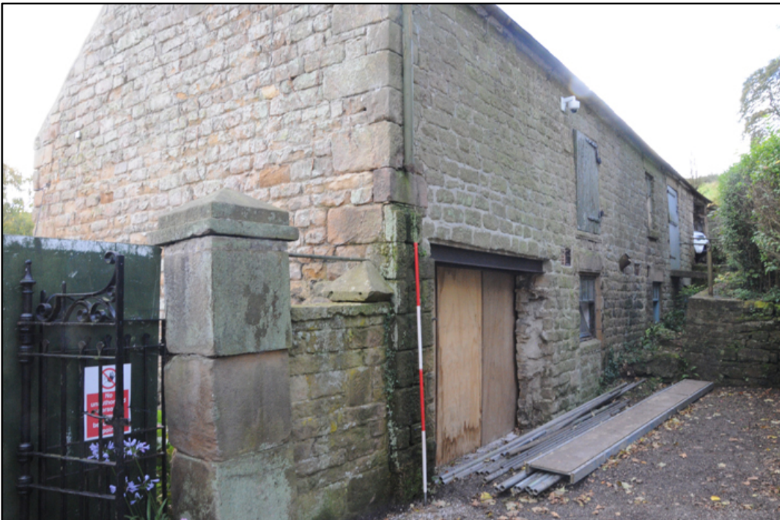
Appendix 5.69: Detail of northwest corner of T-shaped barn, looking south; note inserted door (phase 9) (2m scale)
