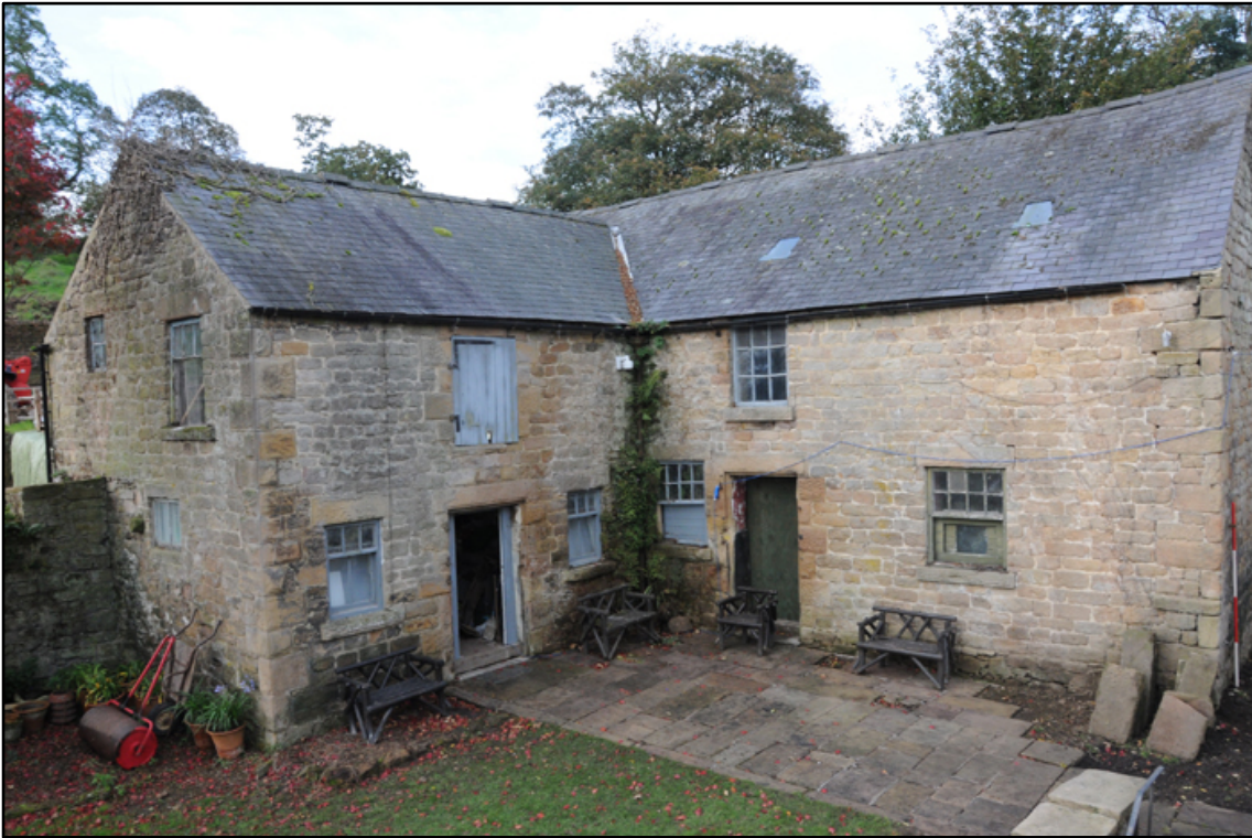
Appendix 5.68: General view of northeast elevations of T-Shaped barn (2m scale)
