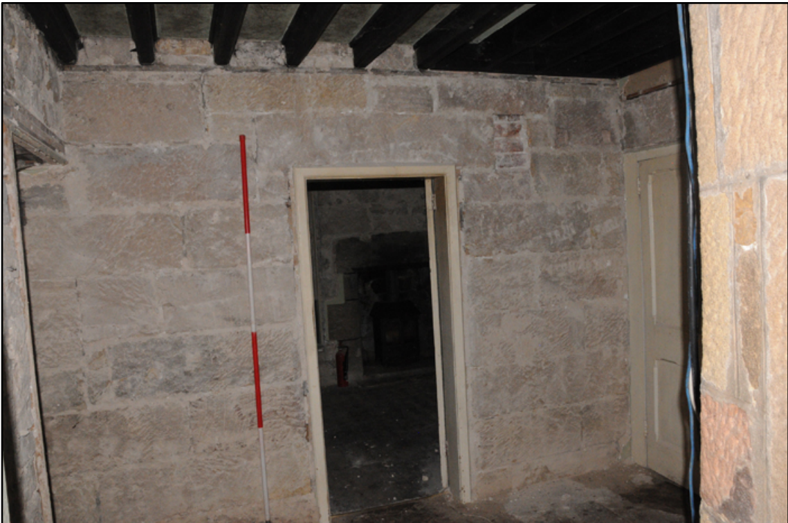
Appendix 5.37: General view of doorway into G7 from G6; note ceiling beam from former open-well staircase (2m scale)
