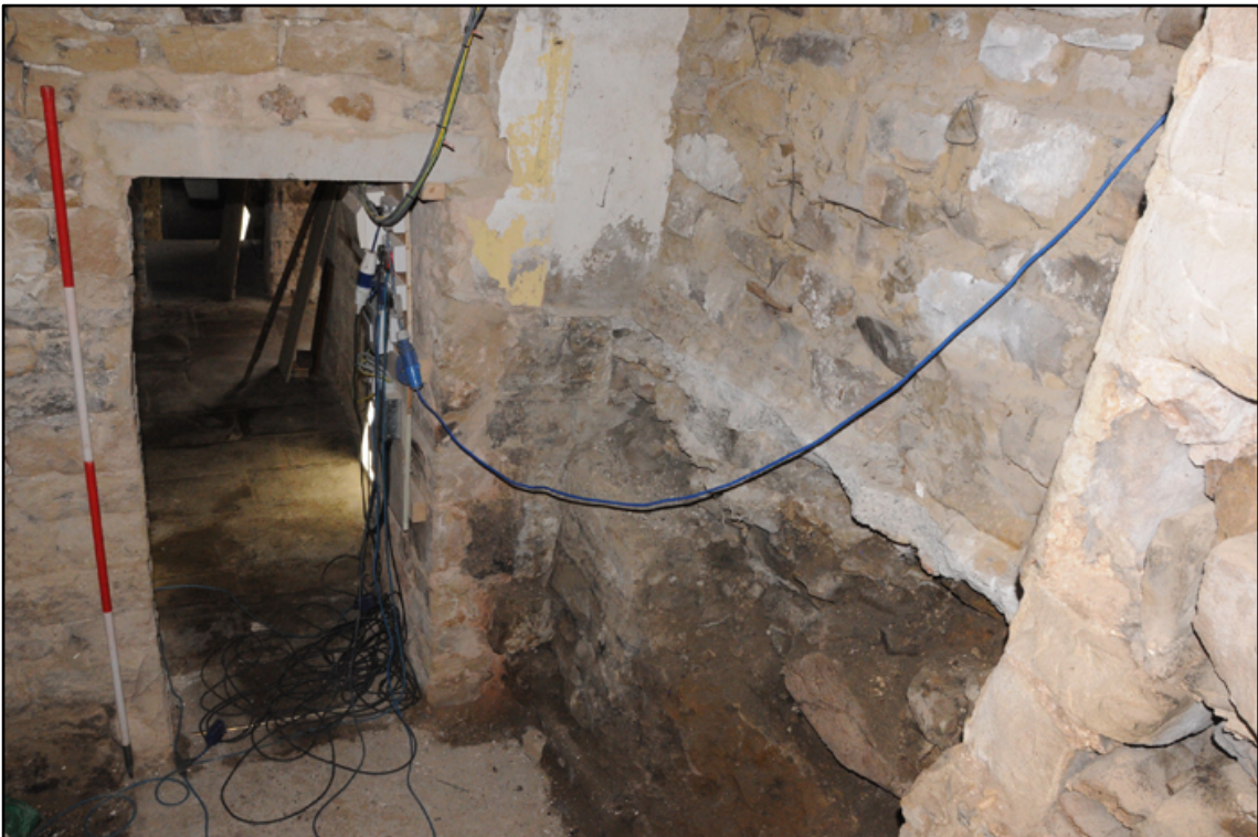
Appendix 5.39: General view of doorway into G3 from G9, looking east; note lowered floor level (2m scale)
