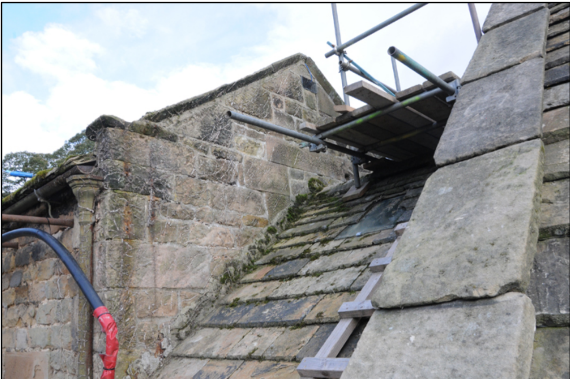
Appendix 5.61: Detail of blocked pitching door in east gable of F5, looking northwest
