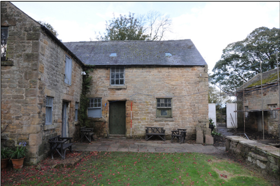
Appendix 5.71: General view east elevation of T-shaped barn; note alterations to windows (2m scale)
