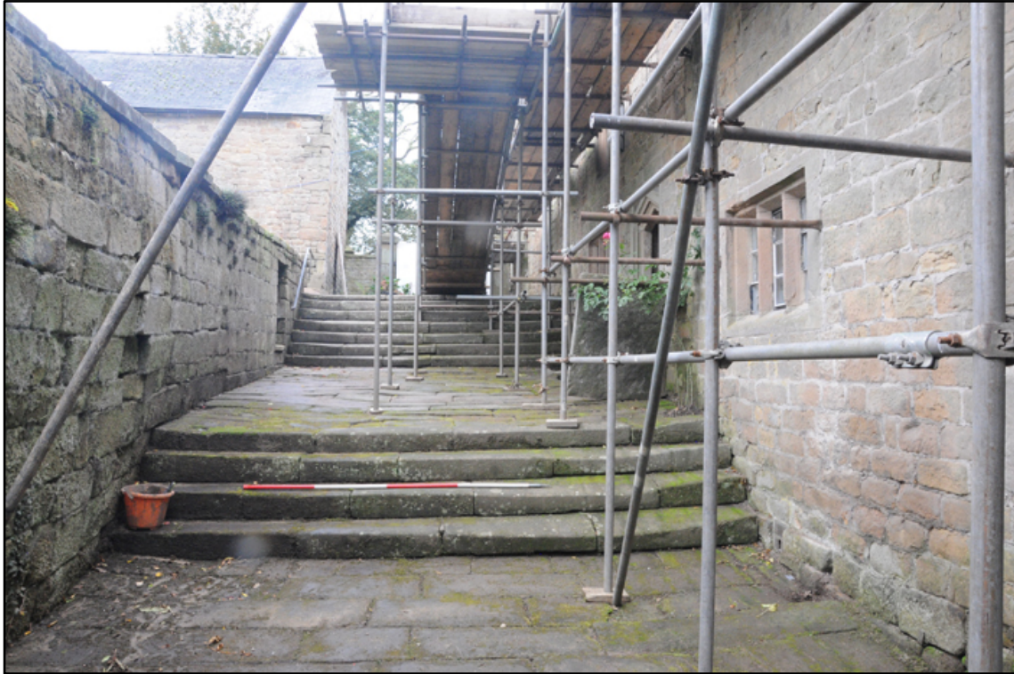
Appendix 5.5: General view looking up entrance walkway along south side of hall (2m scale)
