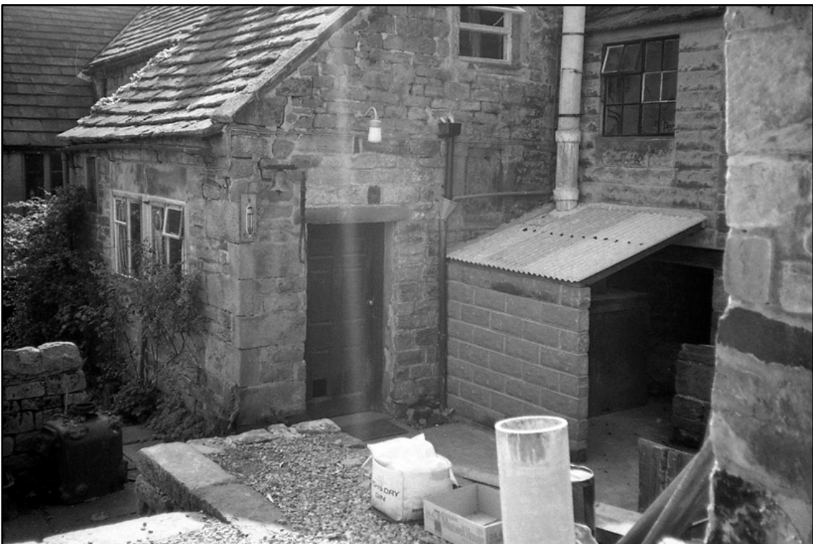
Appendix 3.2: View of rear of building, c.1980s (archive photo from PDNPA)
