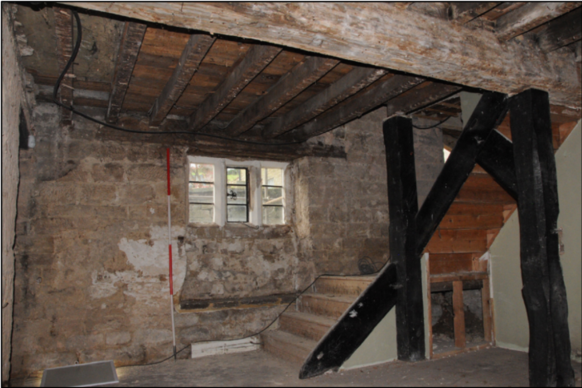
Appendix 5.16: General view of interior of GI, looking southwest; note inserted staircase (phase 9) (2m scale)
