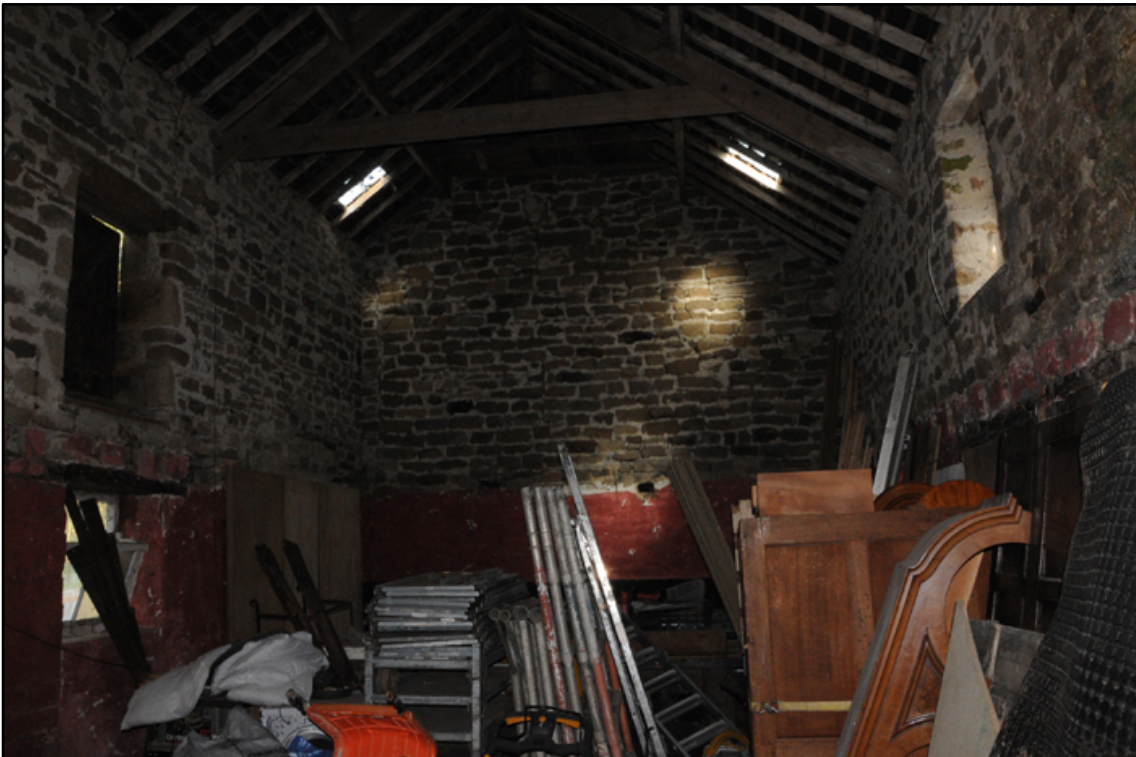
Appendix 5.73: General view of interior of T-shaped barn looking north
