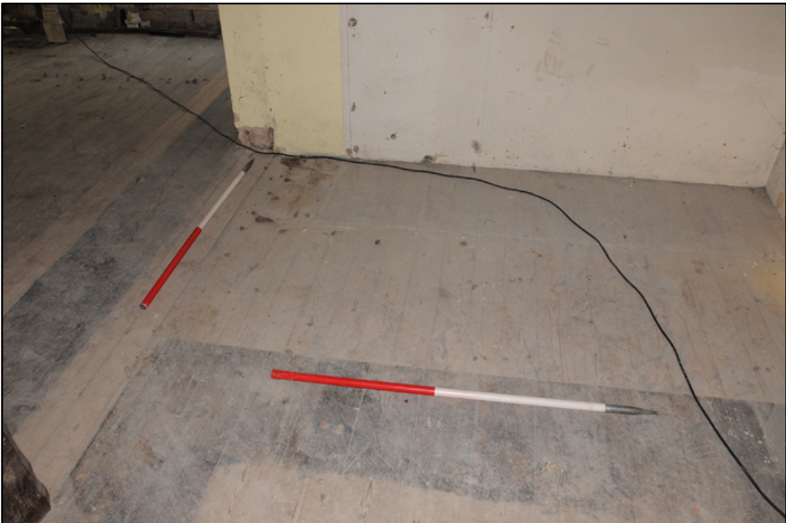
Appendix 5.45: Detail of floor staining in F6, and scar for removed (phase 9) open-well staircase (2m scale)
