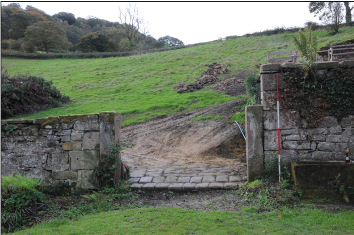
Appendix 5.53: General view of gateway (altered) to south field (2m scale)
