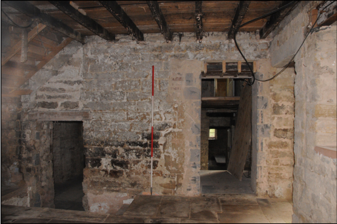
Appendix 5.28: General view of east wall of G3; note altered openings and possible earlier staircase above lintel (2m scale)
