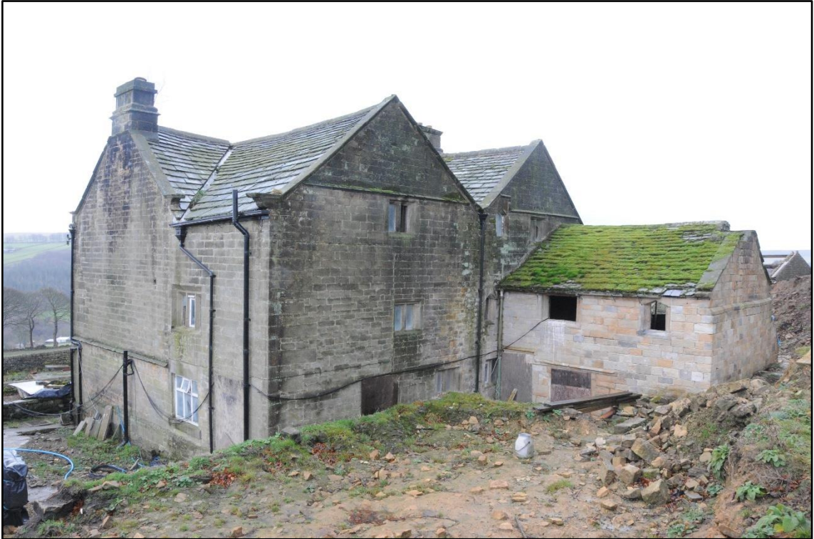
Appendix 2.3: View of the Woodseats Farmhouse (Building 1), looking south
