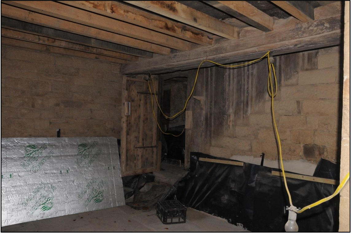
Appendix 2.7: View of rear pantry (Building 1)
