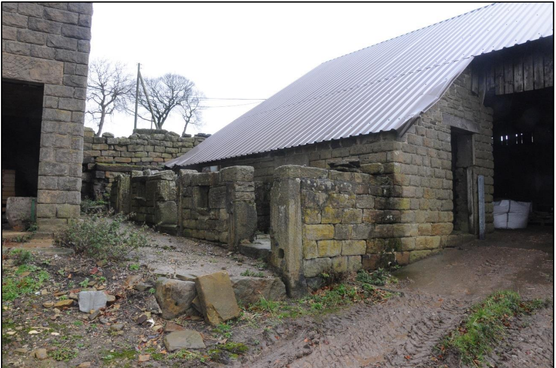
Appendix 2.22: View of pigsty built against west wall of Building 5
