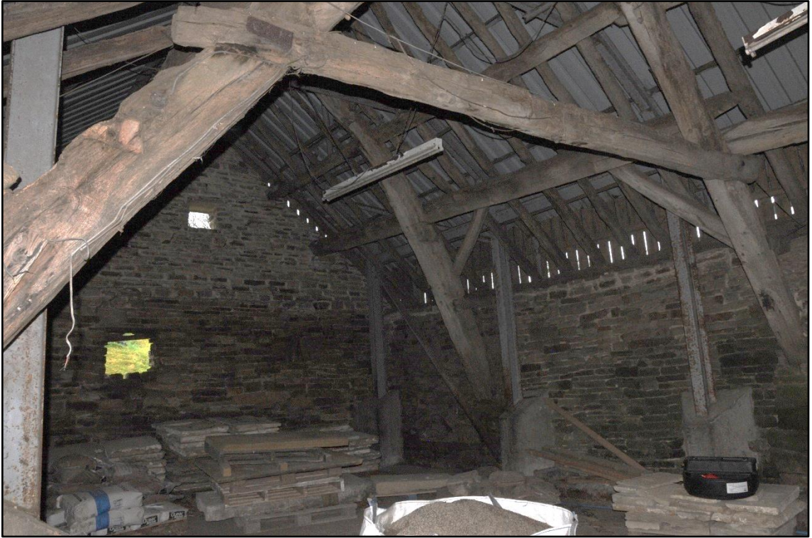
Appendix 2.21: View of interior of Building 5, looking southeast
