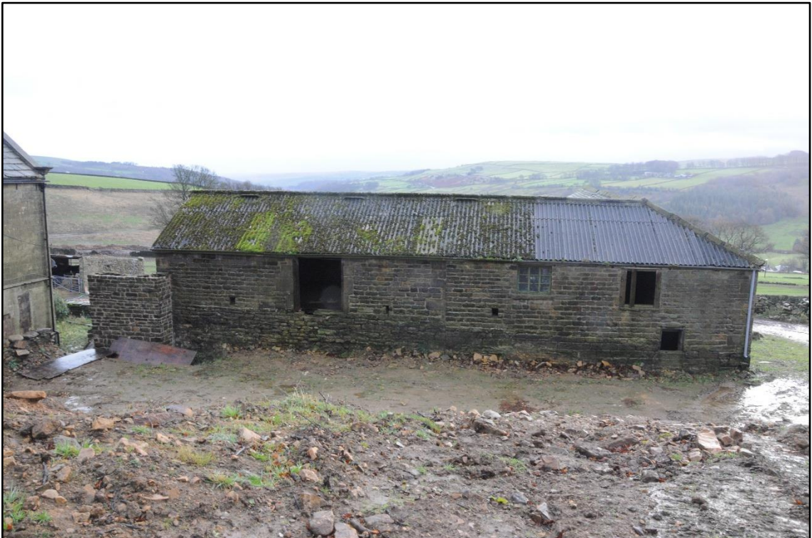
Appendix 2.12: View of Building 2, looking southeast
