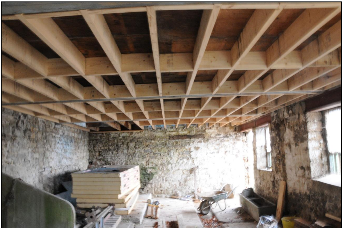
Appendix 2.18: View of interior of Building 4, looking northeast
