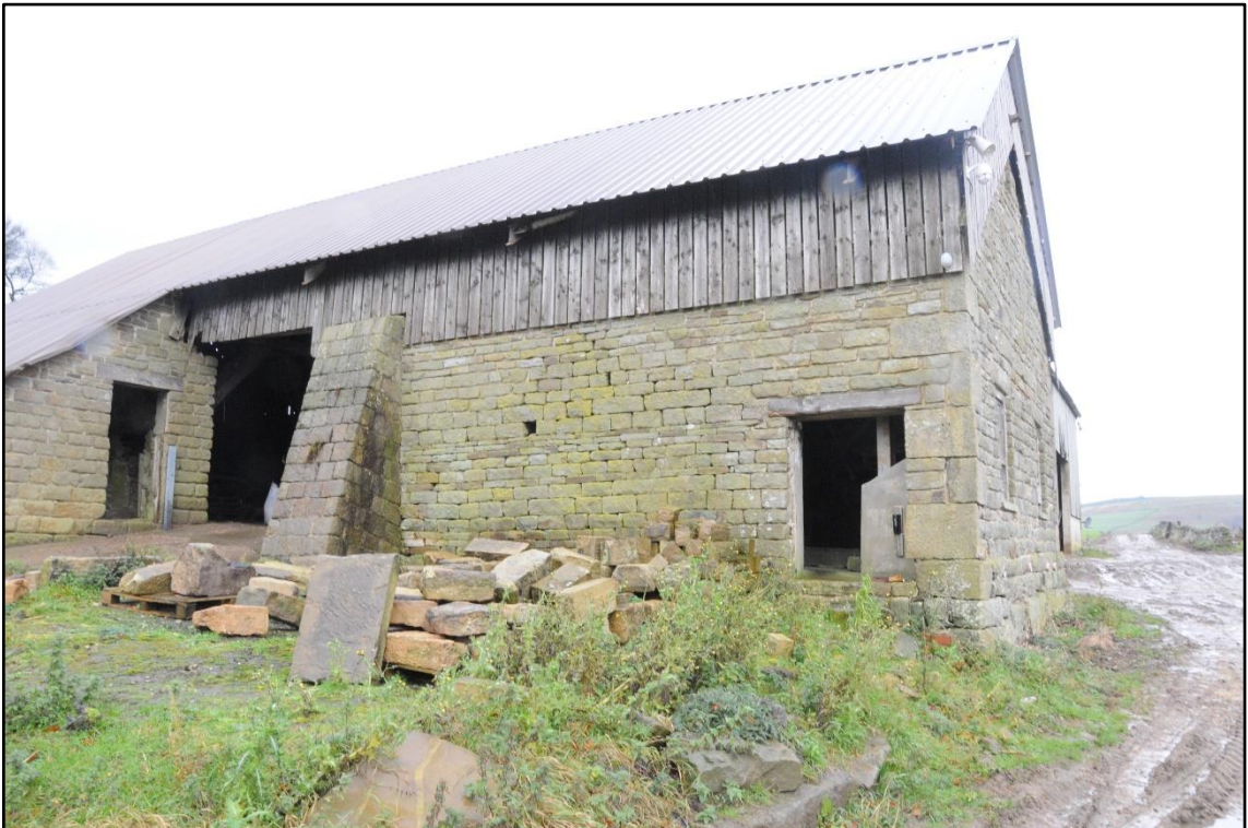
Appendix 2.20: View of Building 5, looking north
