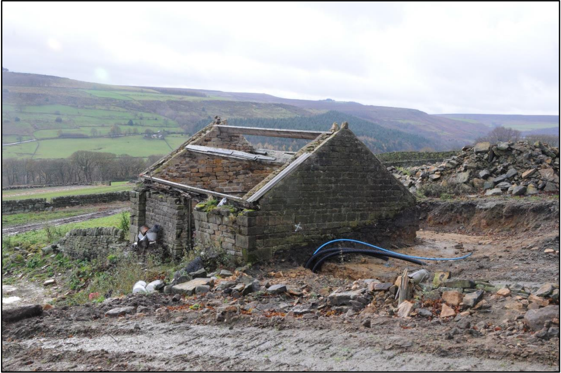
Appendix 2.15: View of Building 3, looking south
