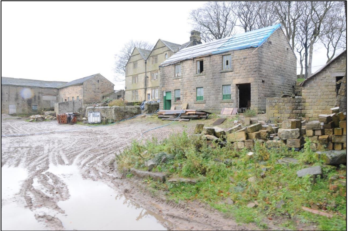
Appendix 2.1: View of woodseats Farm, looking southwest
