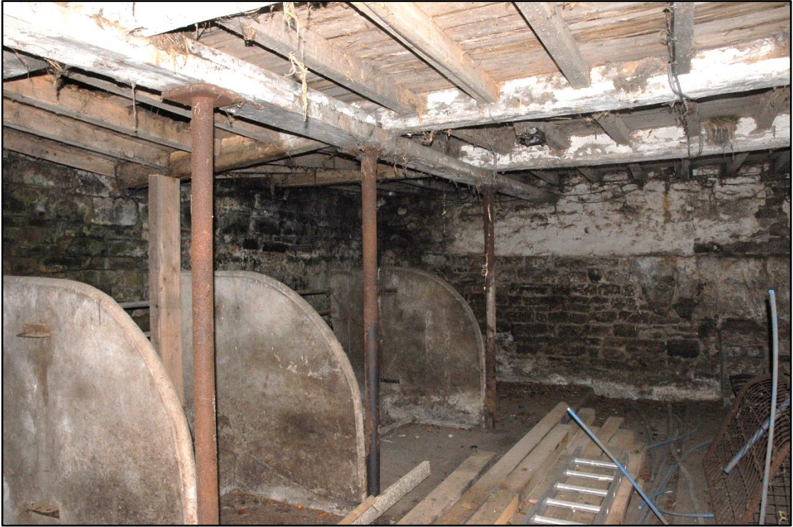
Appendix 2.13: View of interior of northeast-southwest range of Building 2, looking northeast
