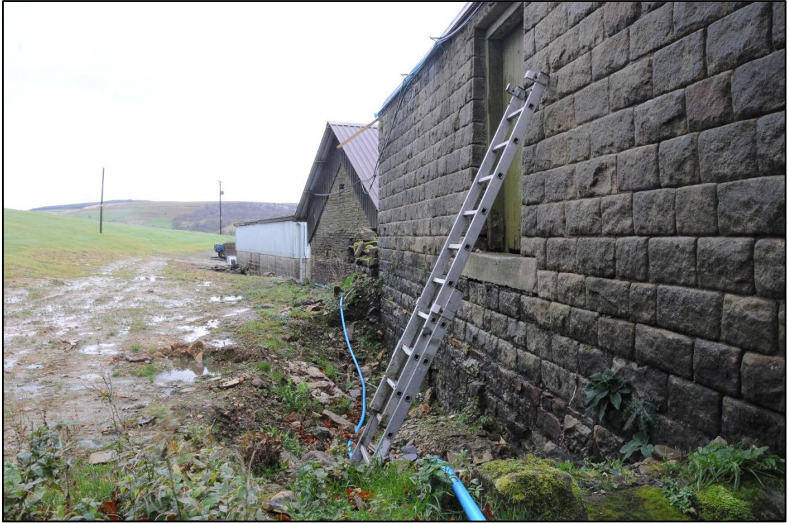
Appendix 2.17: View of north elevation of Building 4, looking northeast
