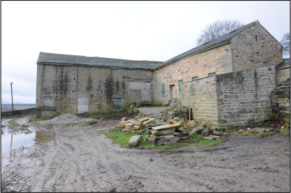
Appendix 2.11: View of Building 2, looking southwest
