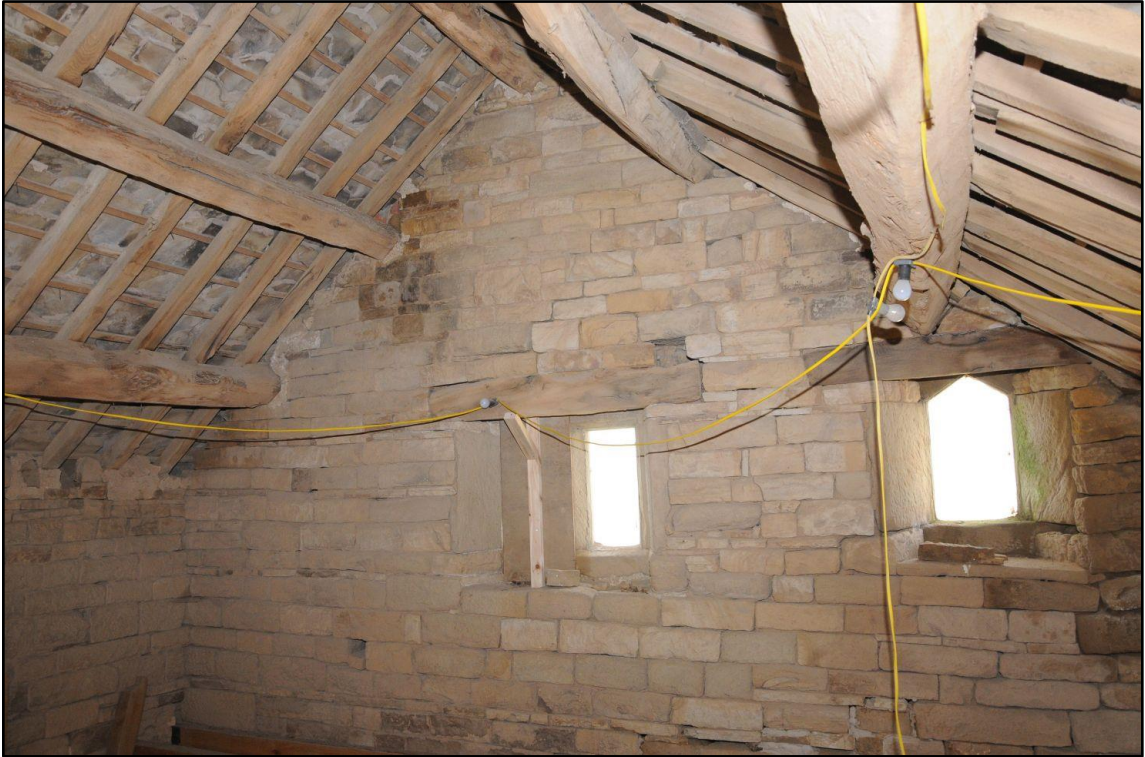
Appendix 2.37: General view of S3, looking northwest
