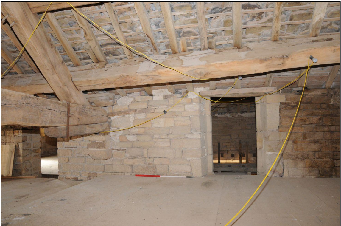
Appendix 2.42: General view of SI, looking southwest (1 m scale)
