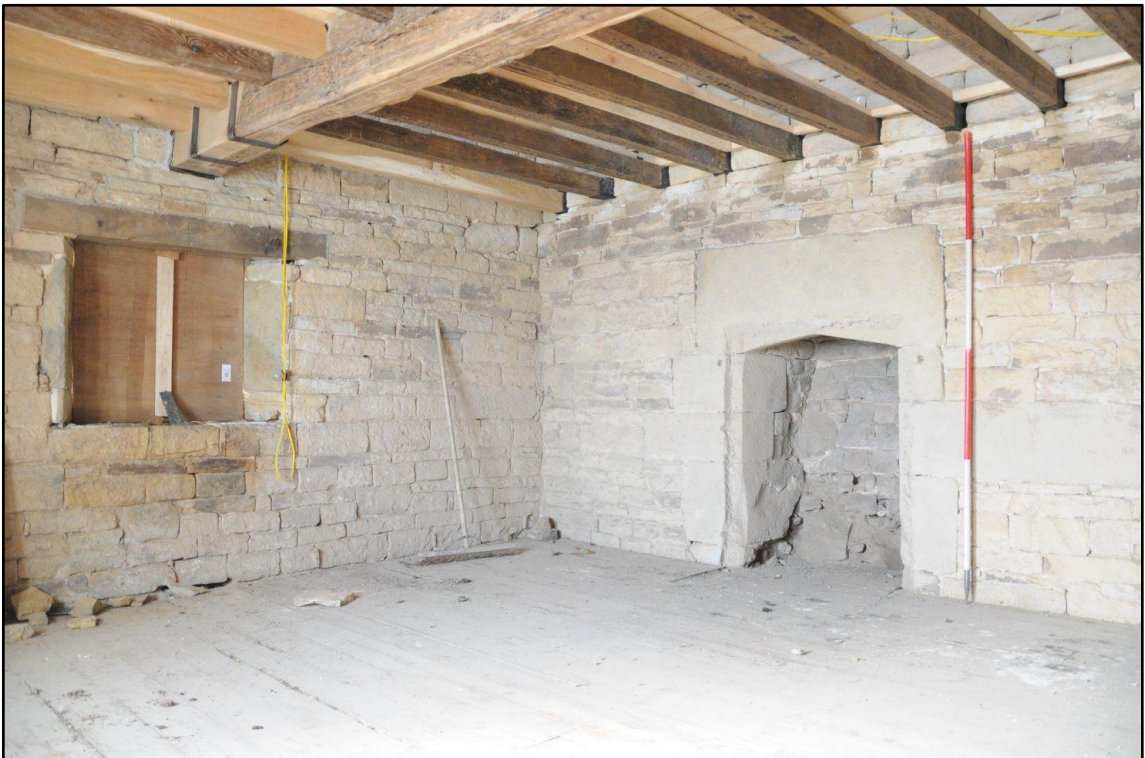
Appendix 2.36: General view of F4, looking west (2m scale)
