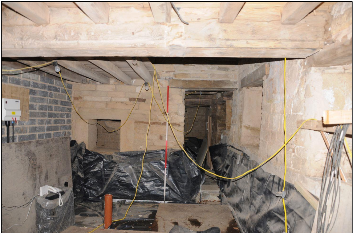
Appendix 2.24: General view of G2
