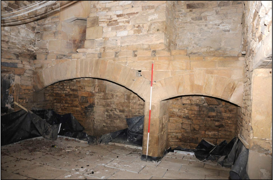
Appendix 2.25: General view of G6/F6, looking north (2m scale)
