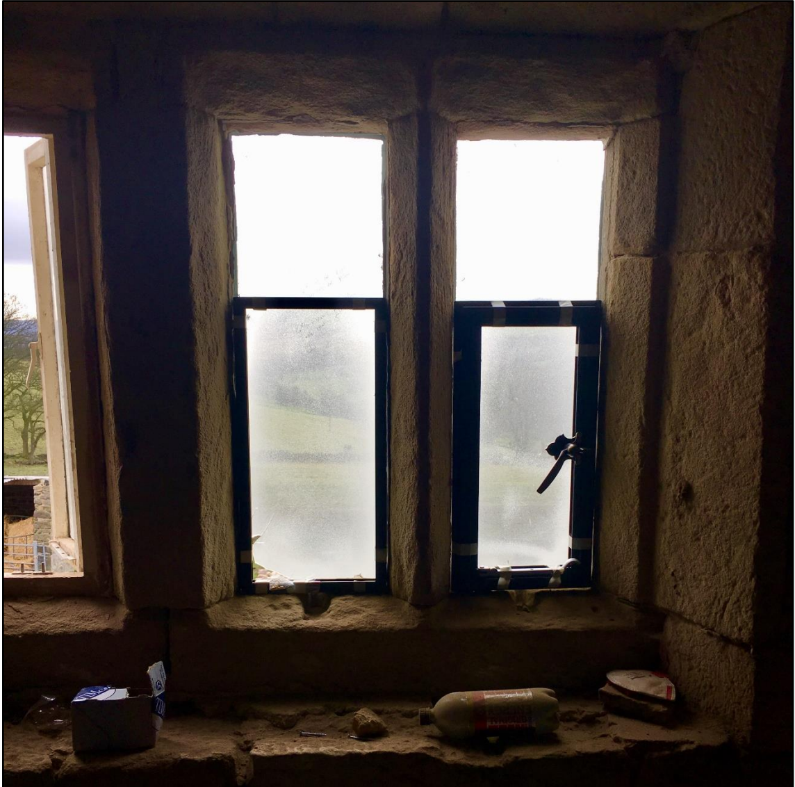
Appendix 2.45: Example of proposed glazing, showing fixed light (left) and casement (right)
