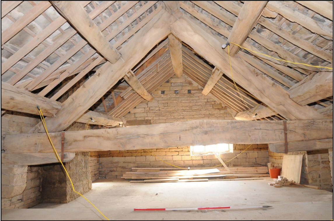
Appendix 2.39: General view of SI, looking southeast (2m scale)
