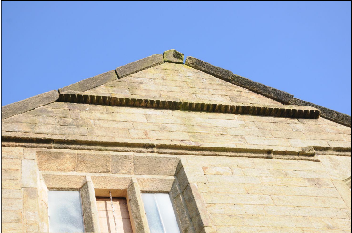
Appendix 2.5: Landing ledge on south elevation of Building I
