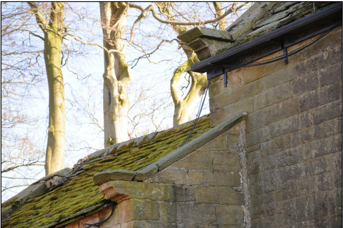
Appendix 2.6: Detail of kneelers, northwest corner of Building I, looking northeast
