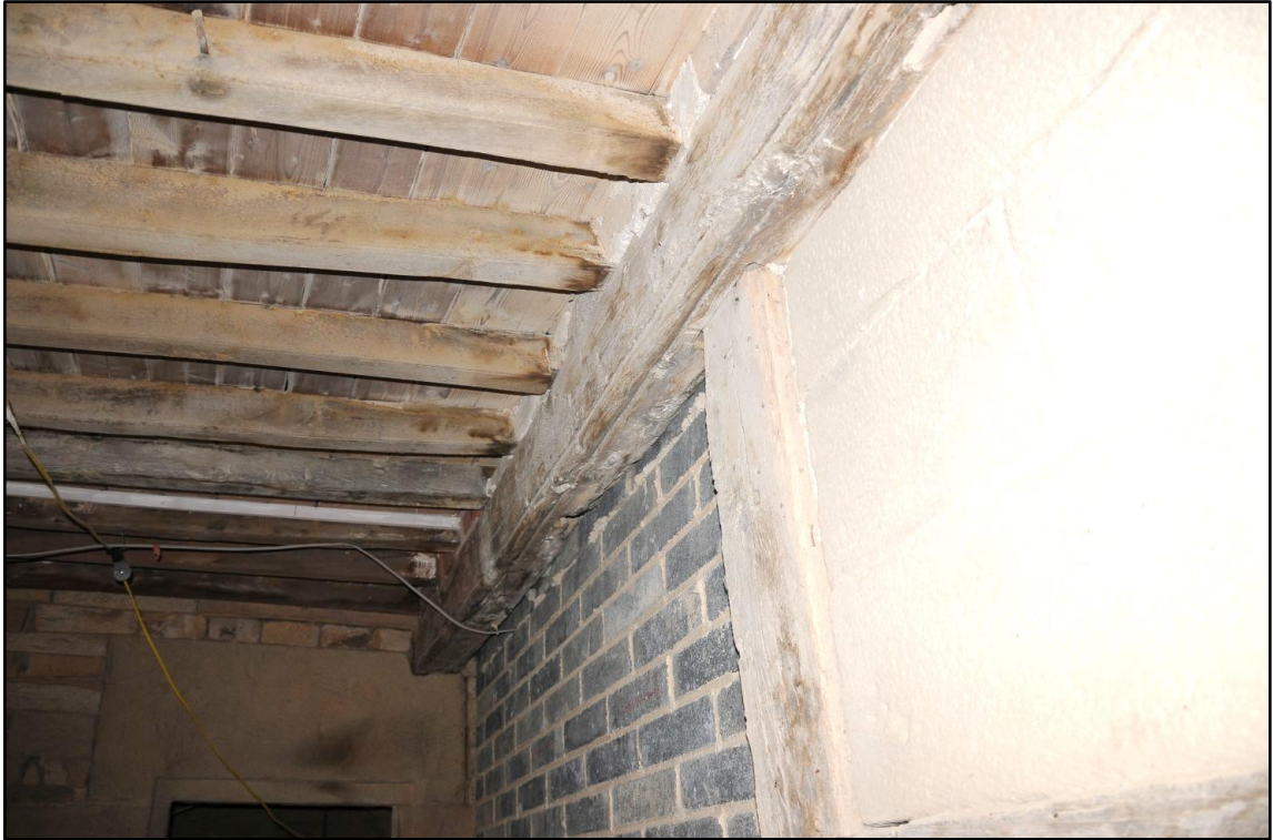
Appendix 2.17: Detail of beam above north wall of G1 , looking southwest
