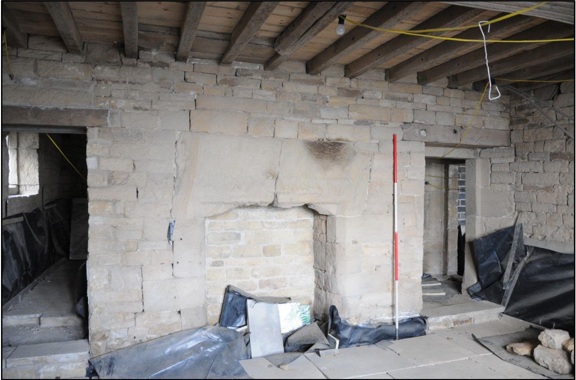
Appendix 2.21: General view of G4, looking north (2m scale)
