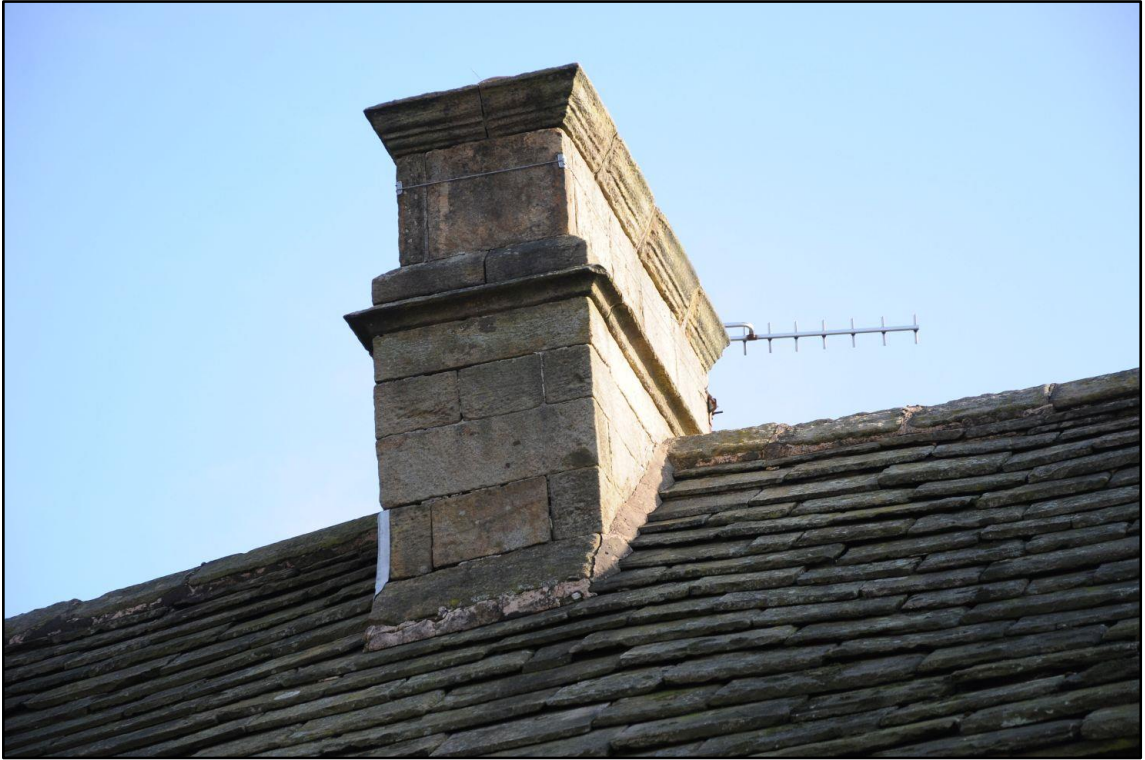
Appendix 2.7: West chimney stack of Building I, looking northeast
