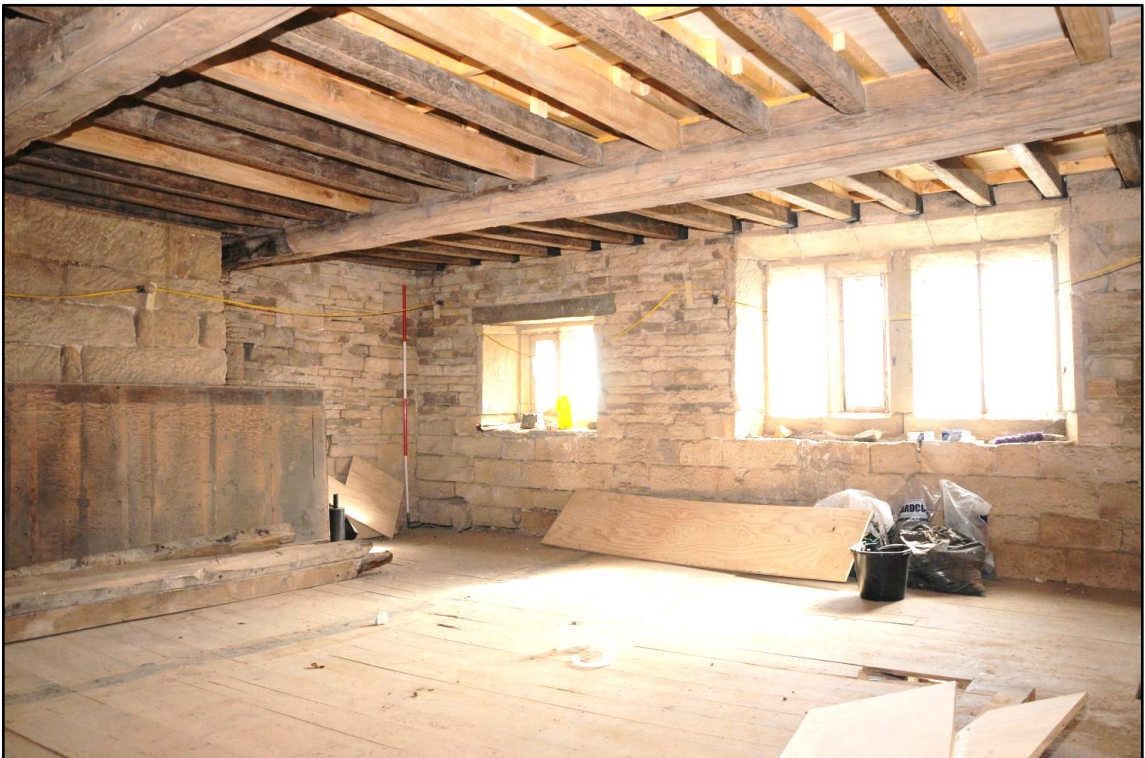
Appendix 2.32: General view of F1, looking east (2m scale)
