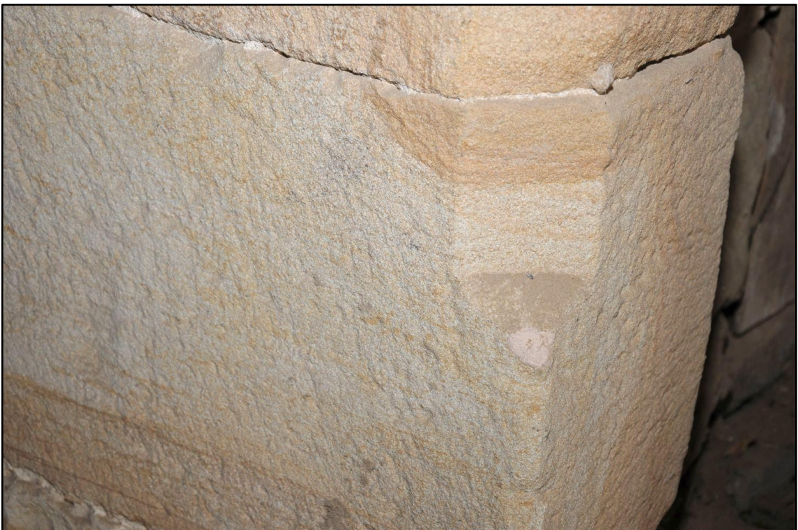
Appendix 2.30: Detail of stop to chamfer on surround to doorway between F3 and F1 , looking northeast
