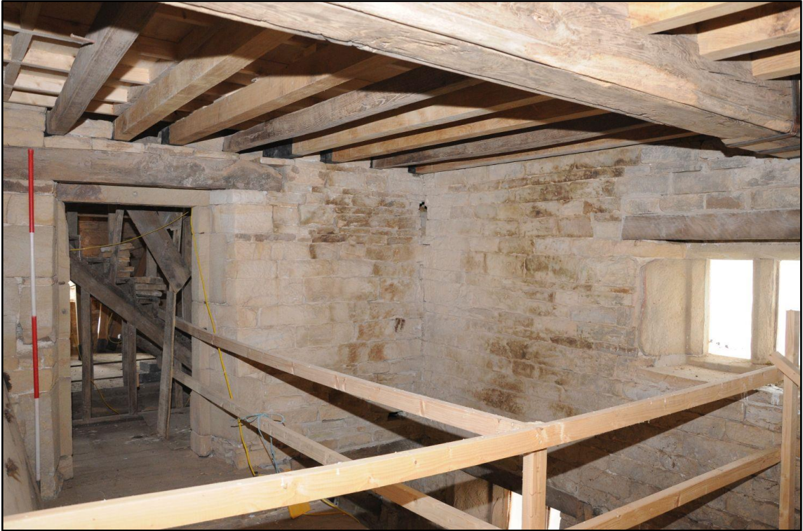
Appendix 2.35: General view of F2, looking west (2m scale)
