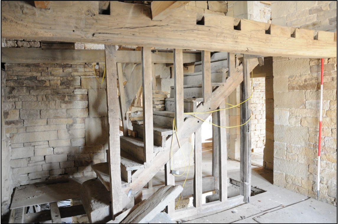
Appendix 2.31: General view of F5, looking east (2m scale)
