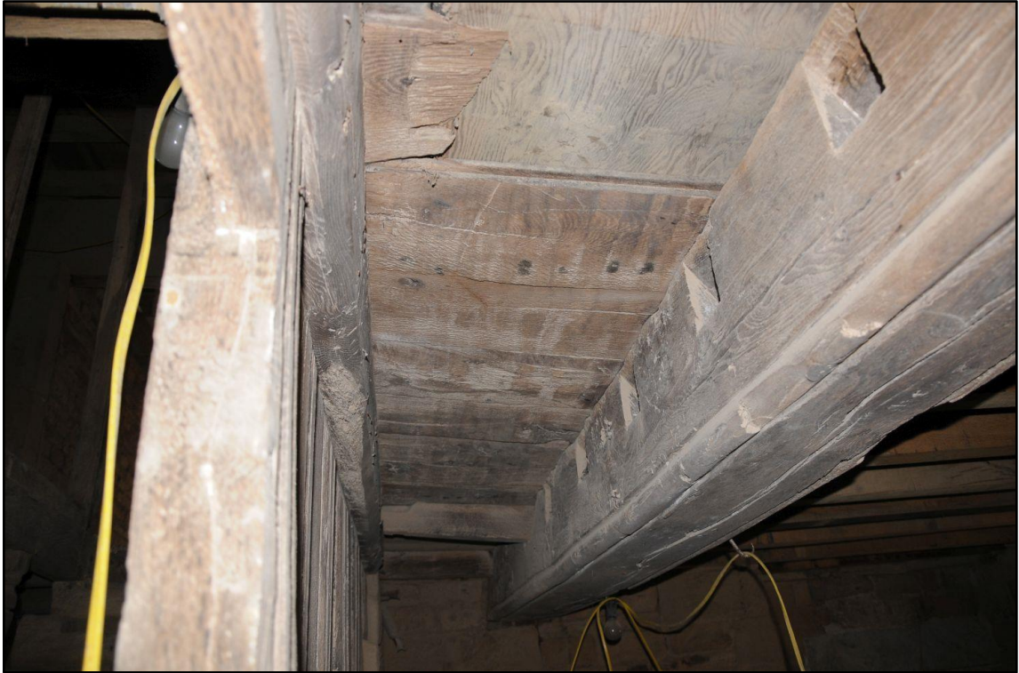
Appendix 2.23: Detail of joist in G5 showing empty mortices, looking southeast
