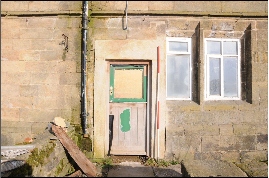
Appendix 2.9: Inserted door in south elevation of Building I (2m scale)
