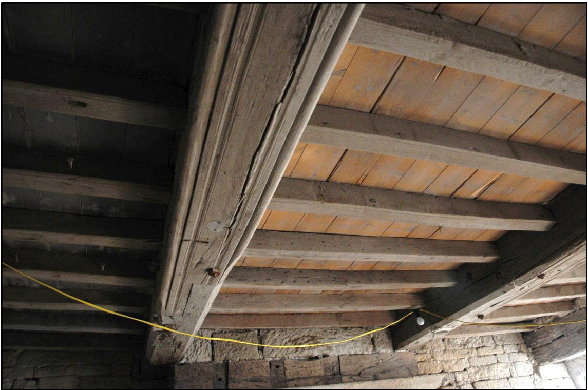
Appendix 2.16: Detail of joists in GI, looking northeast
