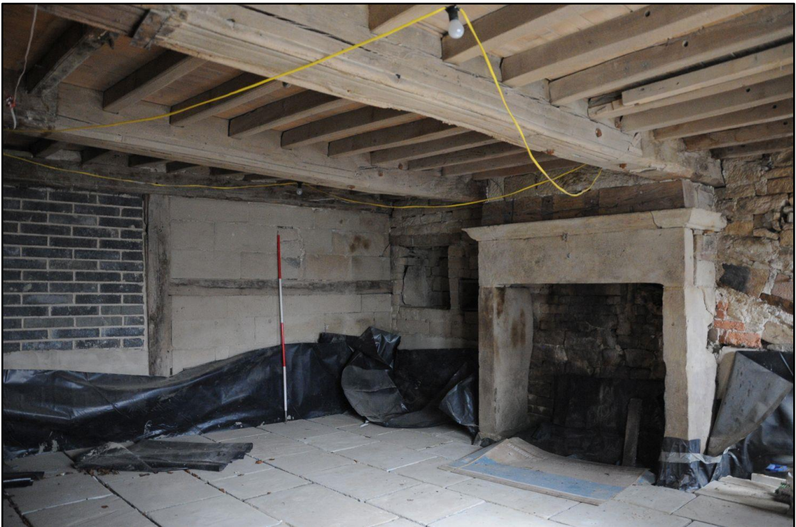
Appendix 2.14: General view of Room GI, looking north (2m scale)
