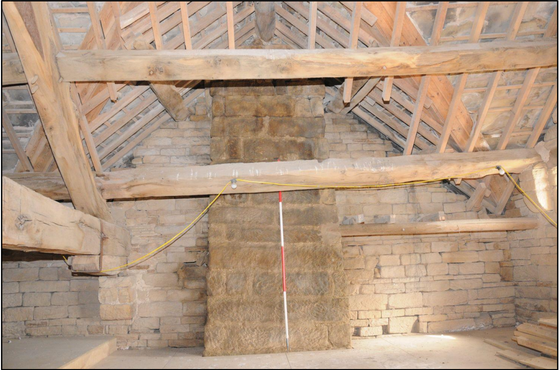
Appendix 2.43: Detail of chimney in S1, looking northeast (2m scale)
