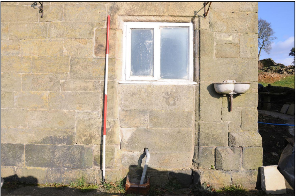
Appendix 2.8: Blocked door in south elevation of Building I (2m scale)
