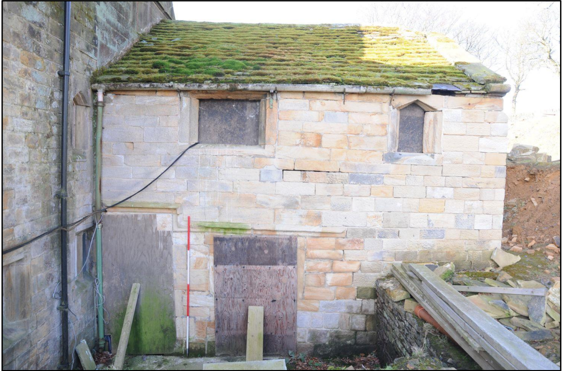
Appendix 2.11: East elevation of north wing of Building I (2m scale)
