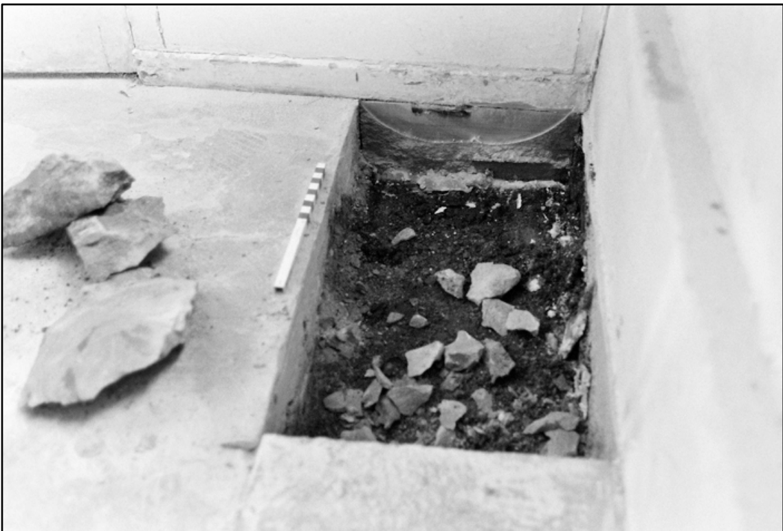
Appendix I.25: Detail of excavated trial hole 2, following removal of slab (20cm scale). Film I.35
