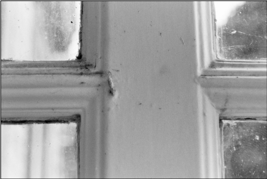
Appendix I.20: Detail of internal joinery, looking south. Film I.32.
