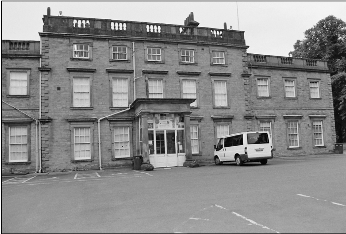
Appendix I.1: General view of Porch and north elevation of Hall, looking south. Film I.03.
