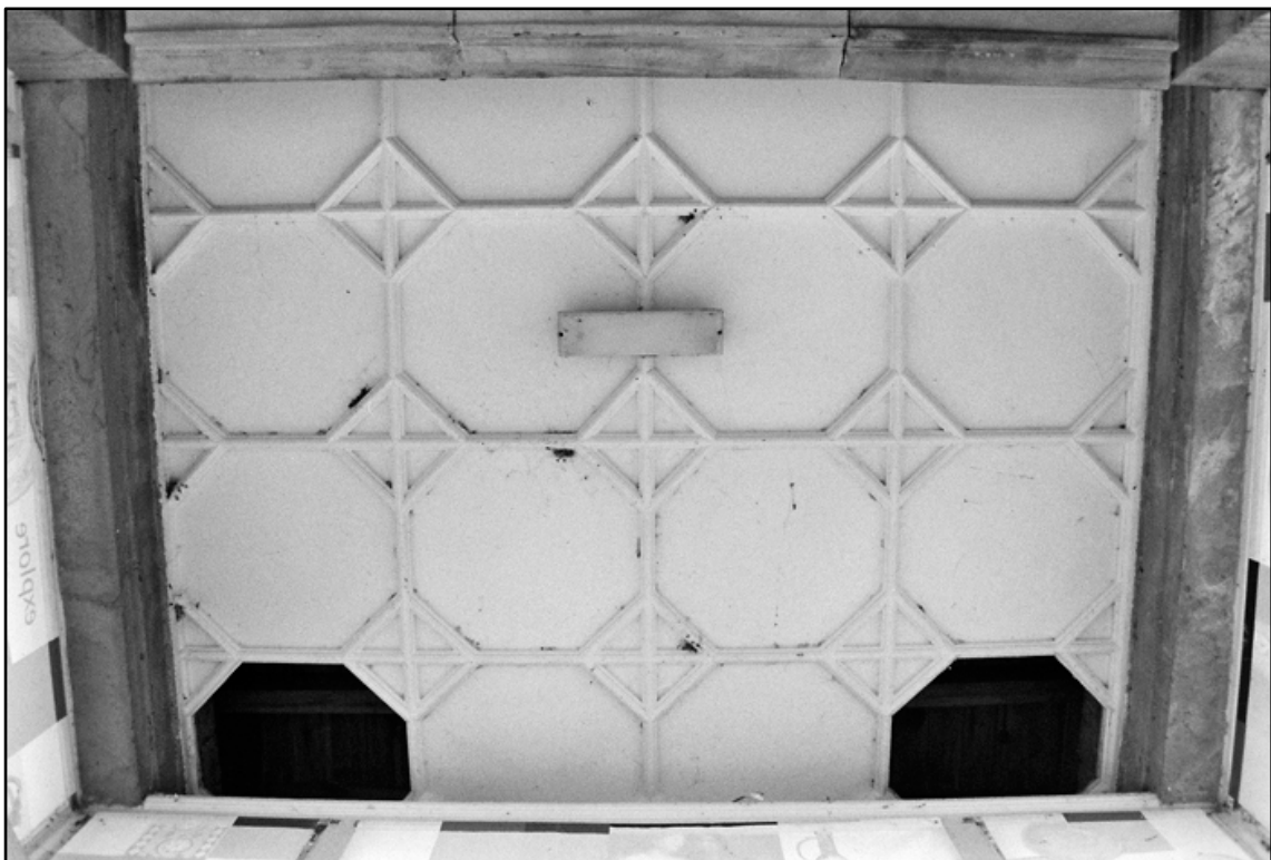
Appendix I.19: Detail of ceiling from below above porch. Film I.31.
