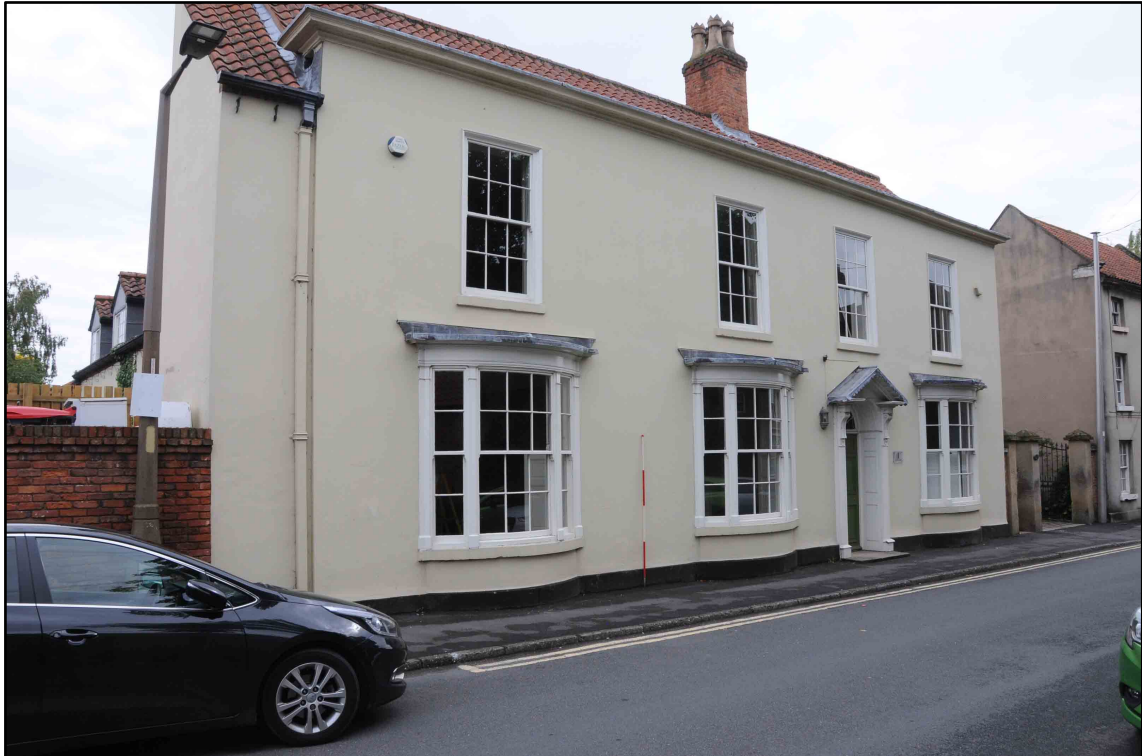
Appendix I.1: General view of front elevation of Grove House looking east (2m scale).
