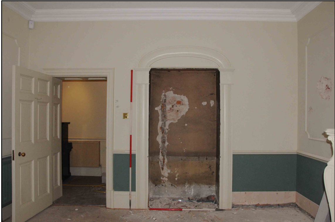
Appendix I.9: General view of north wall in G2 (1m/2m scale).
