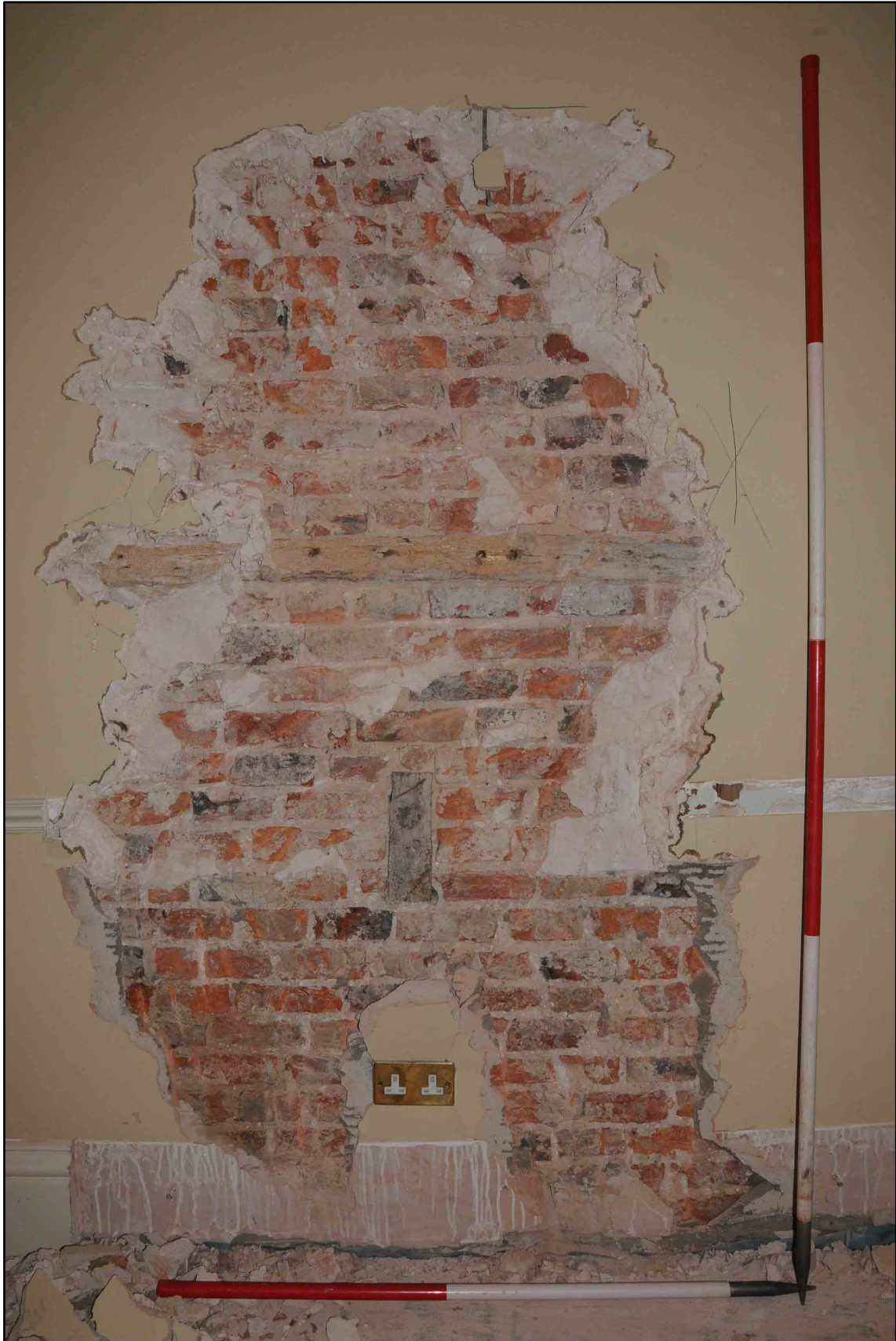
Appendix I.15: General view of north wall in G7, note inset timbers (1m/2m scale).
