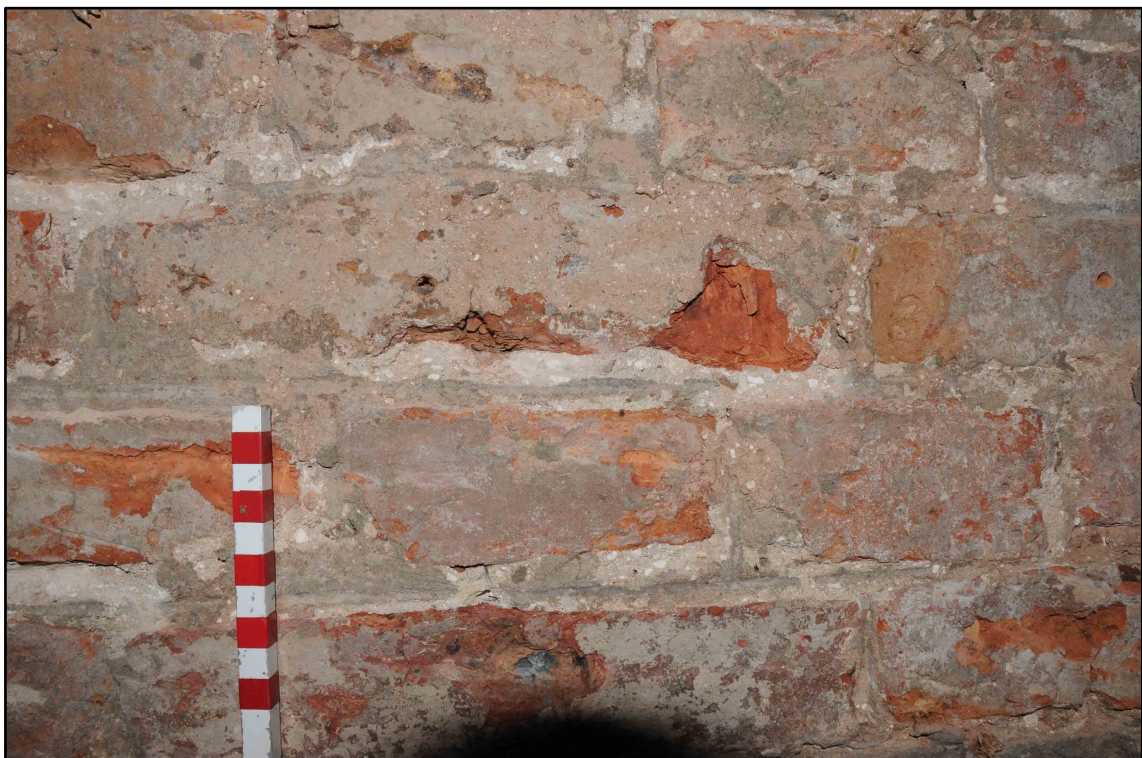
Appendix I.8: Detail of south wall of G4 ; note struck pointing suggestive of being external (10cm scale).
