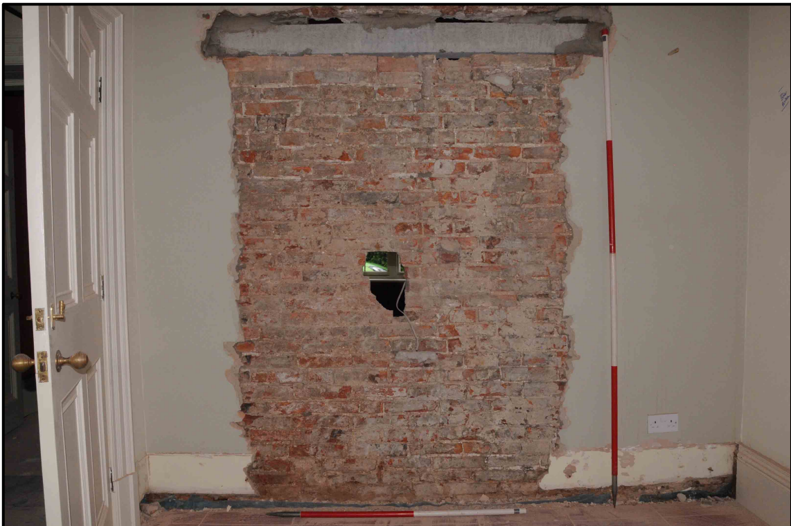
Appendix I.6: Detail of south wall of G4 with plaster removed (1 m/2m scale).
