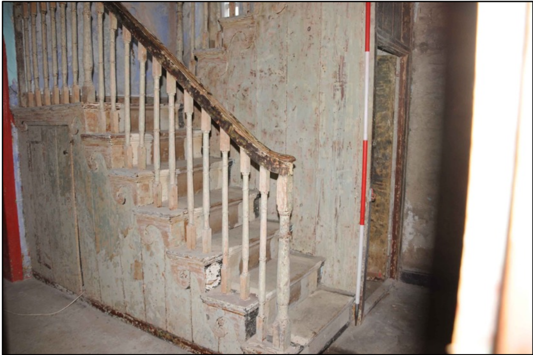
Appendix 2.15: Detail of staircase in G9, looking north (2m scale)
