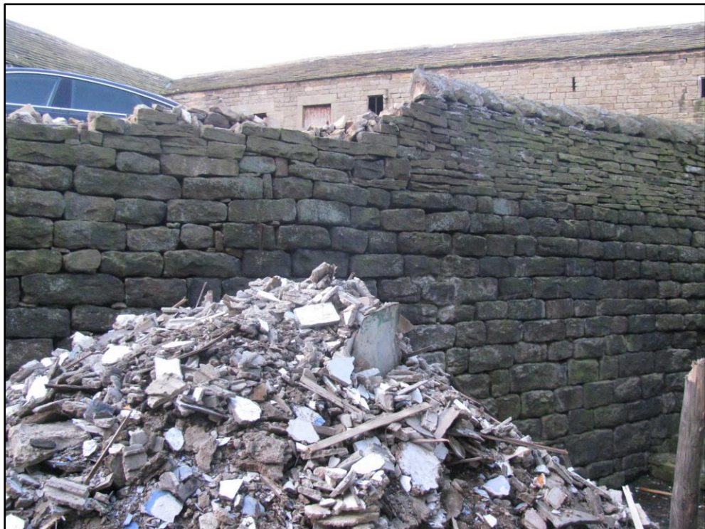
Appendix I.9: Detail of rear boundary wall c. 2016; note change in construction style © PDNPA.
