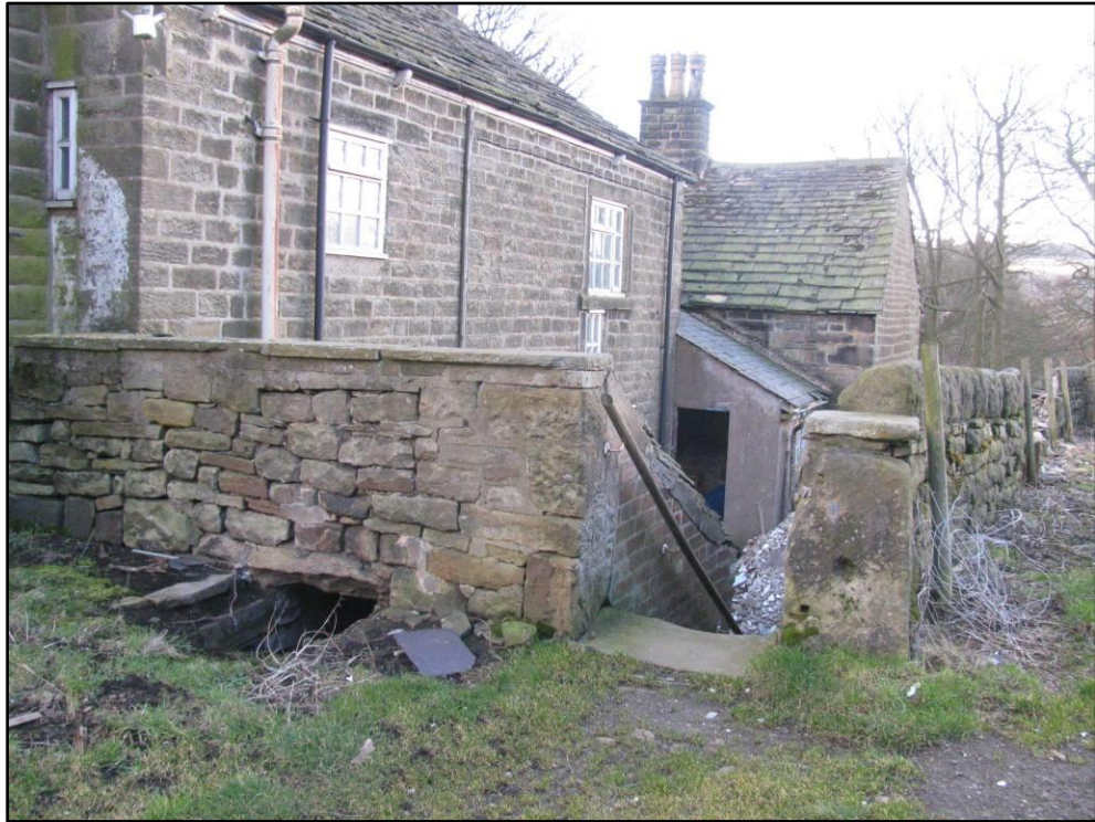
Appendix I.8: View looking northwest along rear boundary wall c. 2016 © PDNPA
