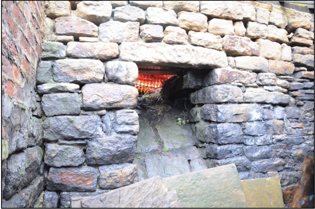
Appendix 2.9: Detail of coal chute in addition to rear of farmhouse
