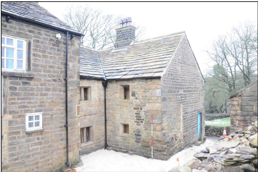
Appendix 2.4: Detail of northeast corner of cottage from the rear, looking southwest (2m scale)
