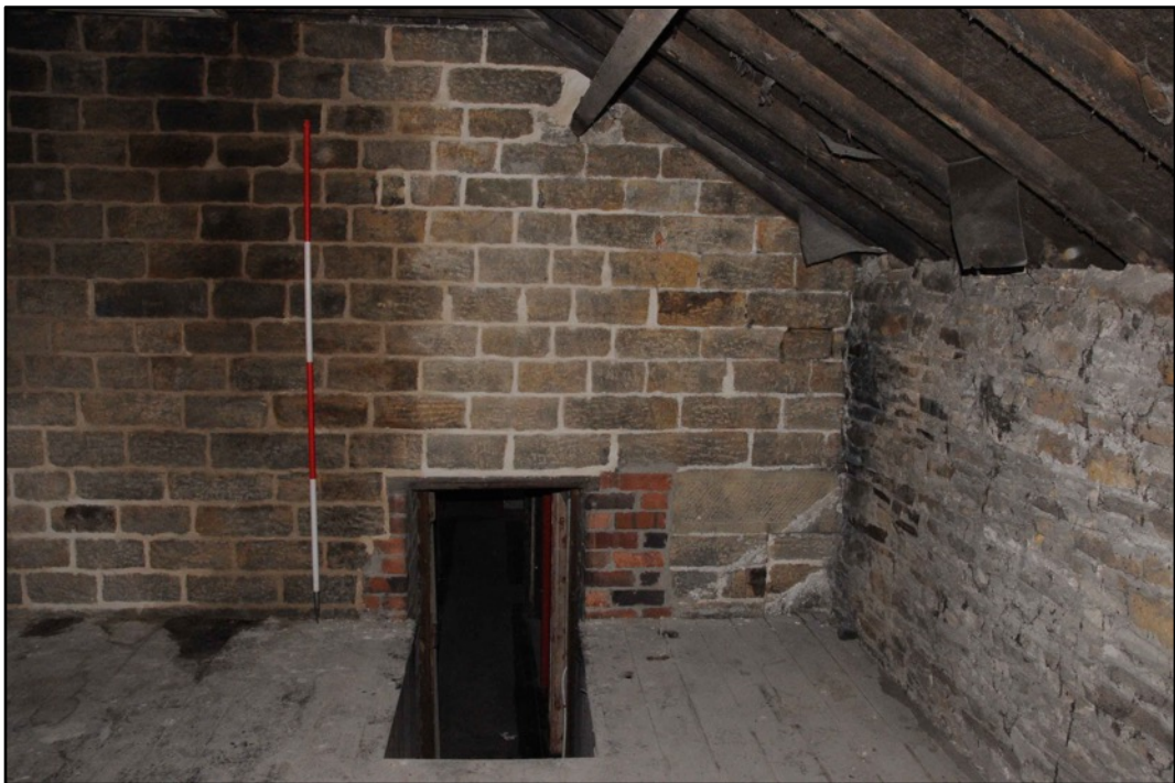
Appendix 2.26: General view of northeast corner of F10; note inserted doorway (2m scale)
