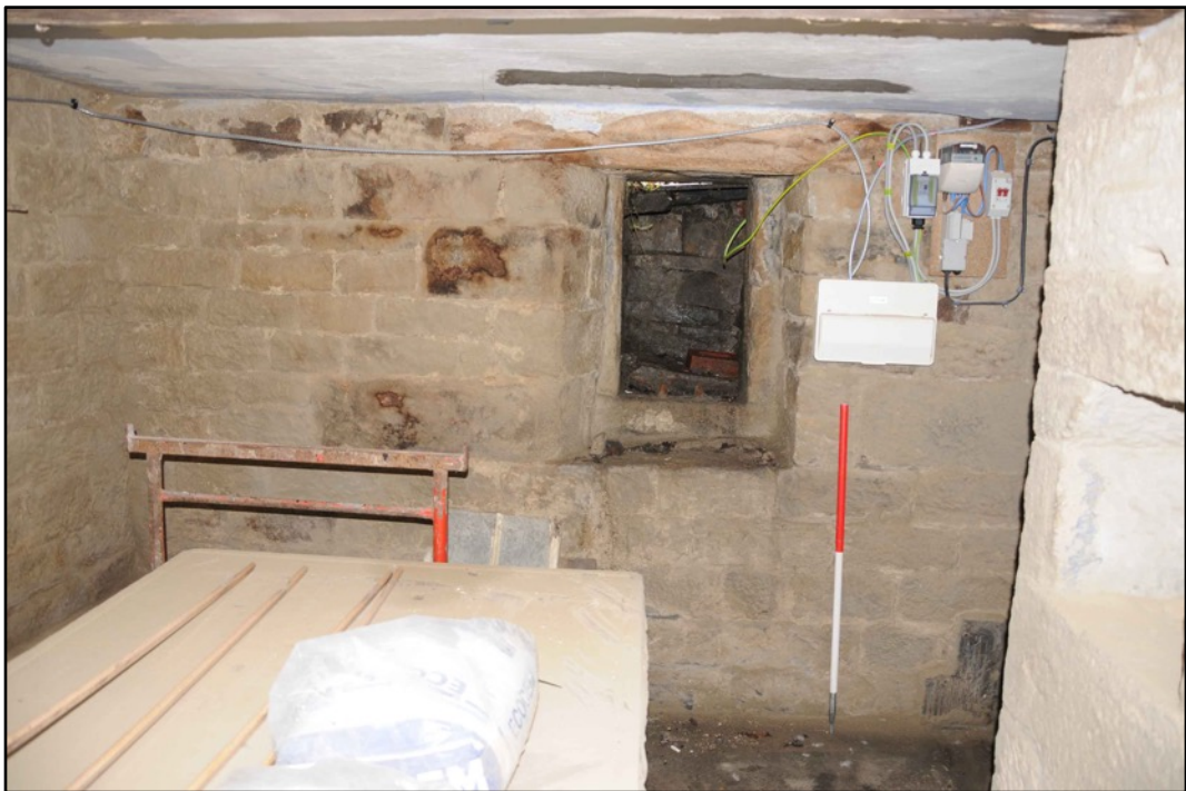
Appendix 2.38: General view of CI, looking southwest towards lightwell (1m scale)
