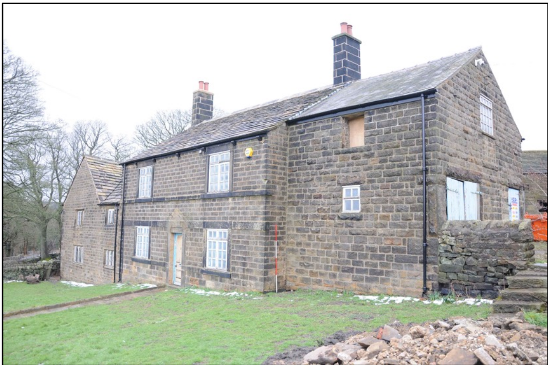
Appendix 2.2: View of south elevation, looking northwest (2m scale)
