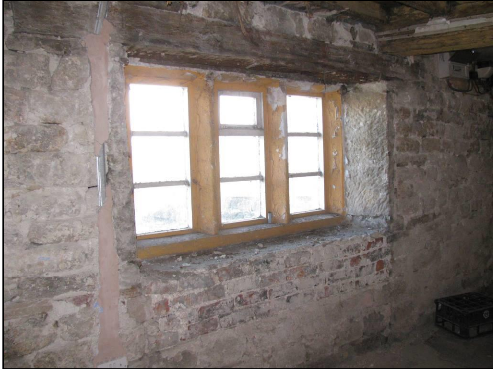
Appendix I.10: View of south window in GI ; note secondary infilling of brick below sill © PDNPA
