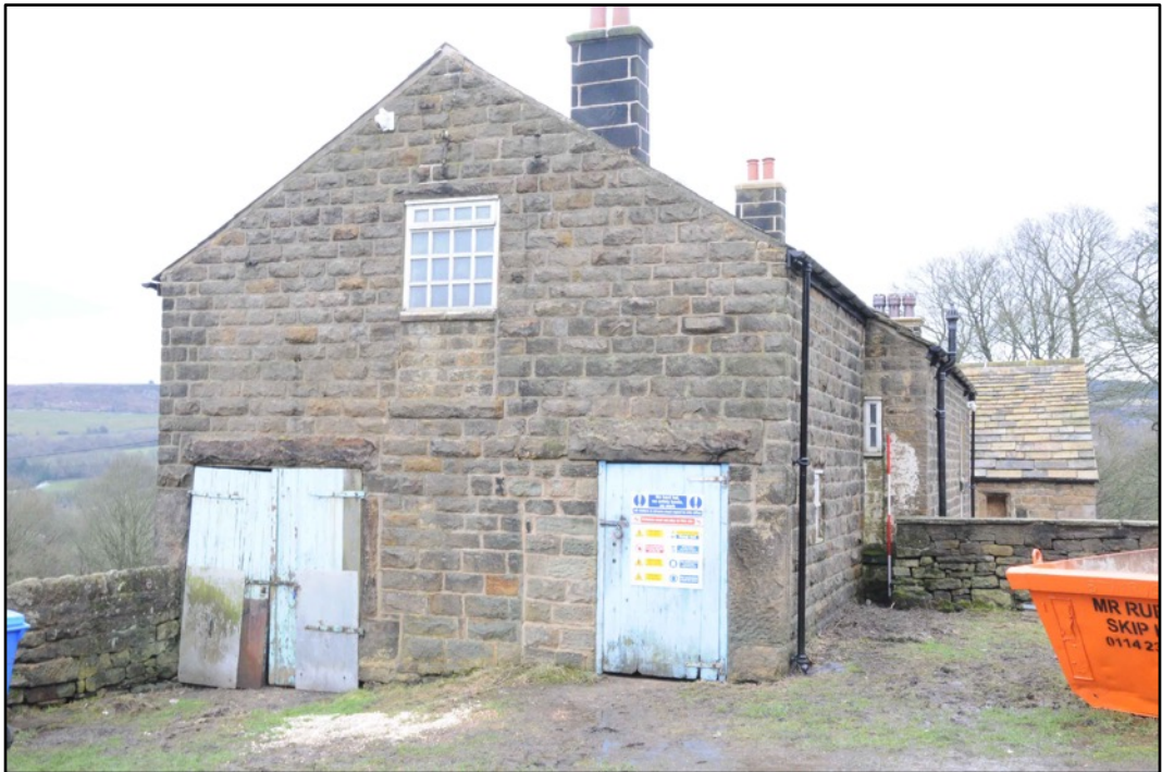
Appendix 2.10: East elevation of 20 th century addition to farmhouse (2m scale)
