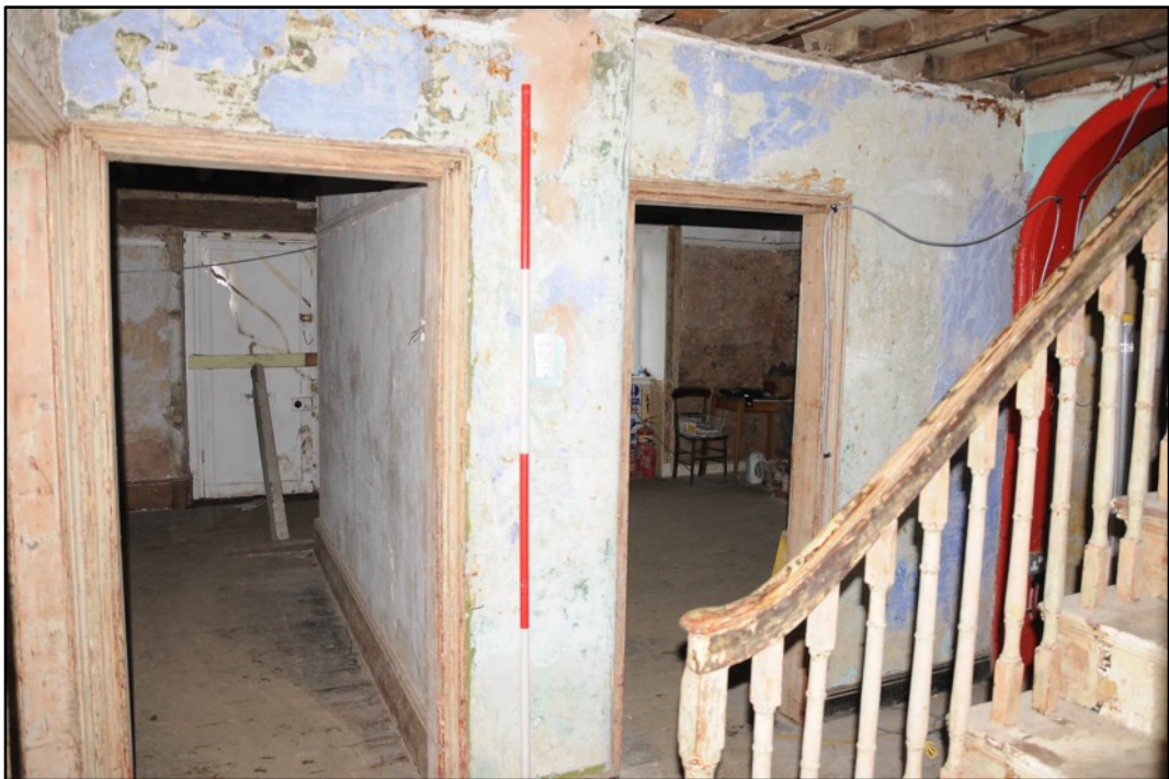
Appendix 2.16: General view of G8, looking south (2m scale)
