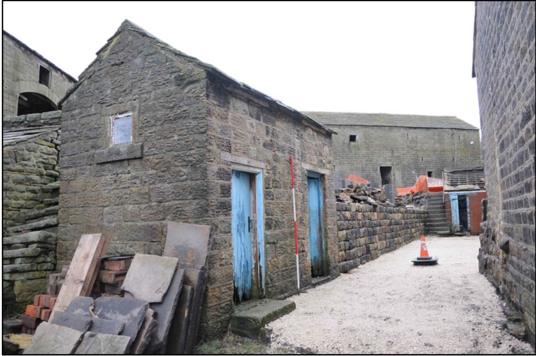
Appendix 2.5: View looking into rear yard from the northwest (2m scale)
