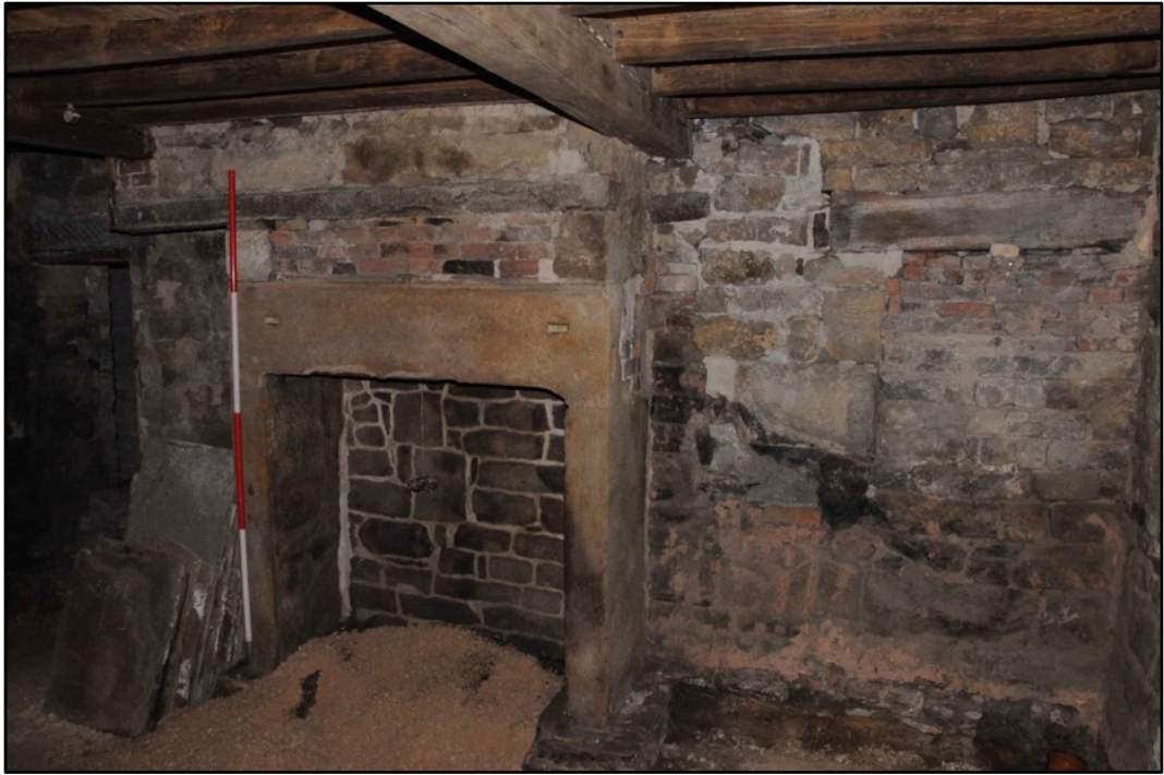
Appendix 2.27: General view of fireplace in G2, looking southeast; note blockings (2m scale)
