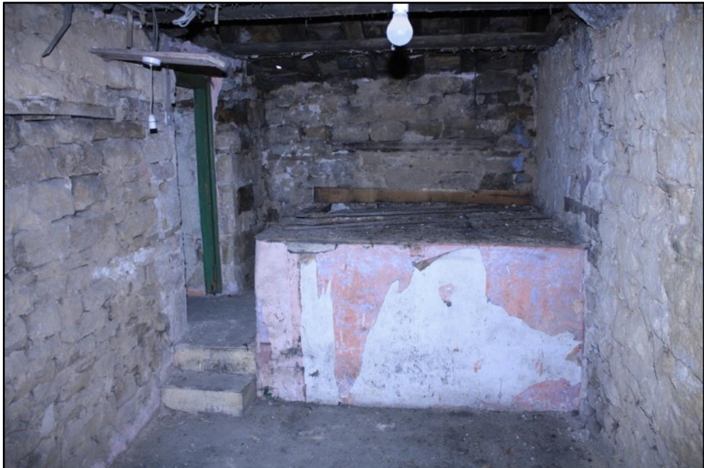
Appendix I.11: View looking north of in F3 ; note raised platform dating to Phase 5 alterations © PDNPA
