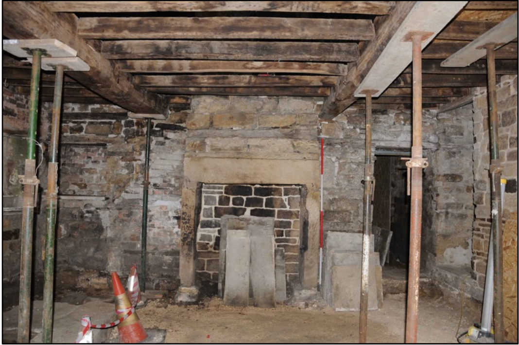
Appendix 2.31: General view of GI looking north (2m scale)
