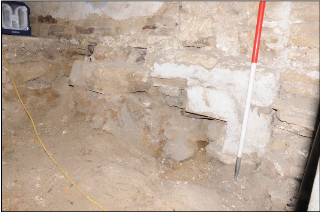
Appendix 2.19: Detail of scar from removed steps in G3, looking south (0.5m scale division)
