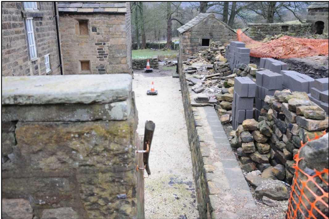
Appendix 2.6: View looking northwest along boundry wall of rear yard
