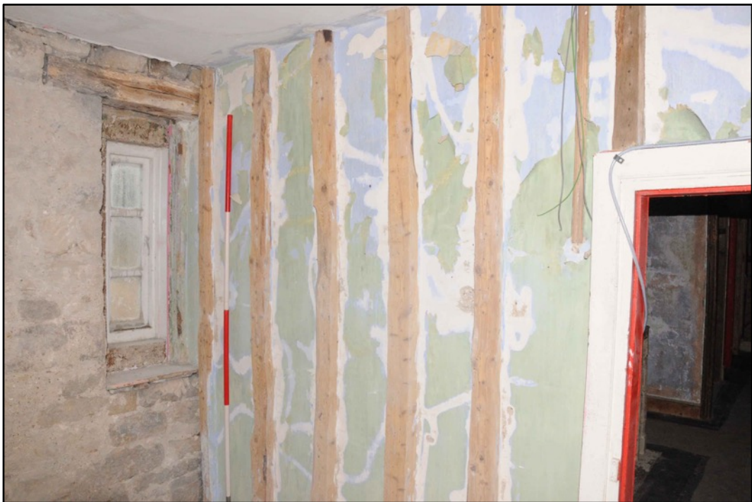
Appendix 2.22: Detail of inserted stud wall in F6, looking east (2m scale)
