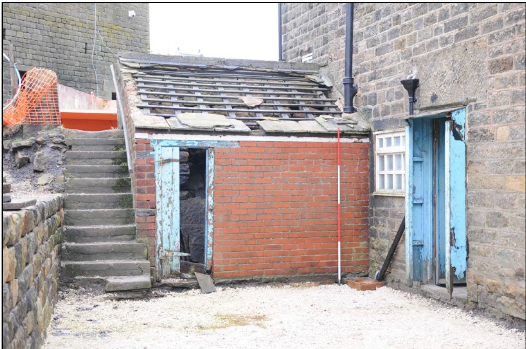
Appendix 2.8: Detail of brick built addition to rear of farmhouse of storage of coal (2m scale)
