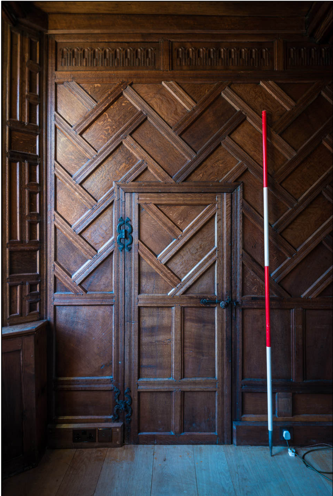
Appendix 5.35: Detail of former doorway in southwest corner of G4 (2m scale) (Photo 152)
