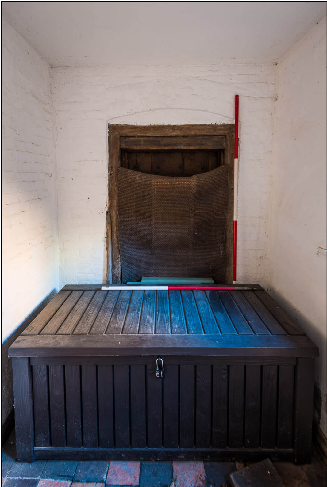
Appendix 5.44: Blocked external doorway into southeast corner of G2 (2m scale) (Photo 38)
