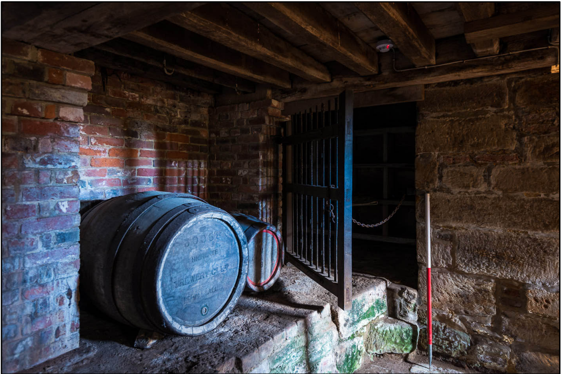
Appendix 5.88: View of southeast corner of BI (1m scale) (Photo 91)
