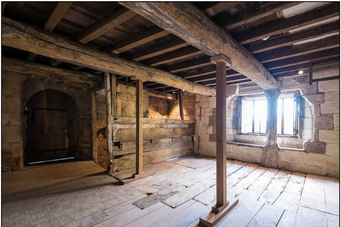
Appendix 5.101: General view of G10, looking southwest (2m scale) (Photo 78)
