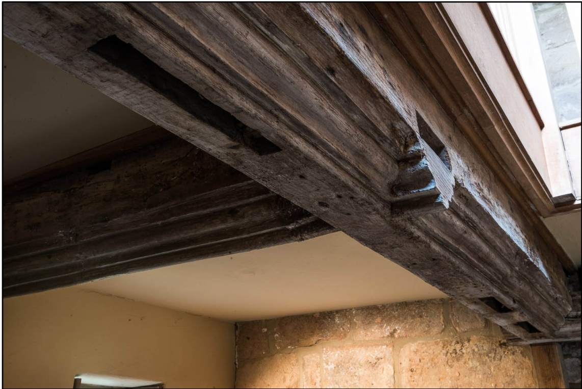
Appendix 5.97: Detail of re-used beams in first floor of G9 (Photo 73)
