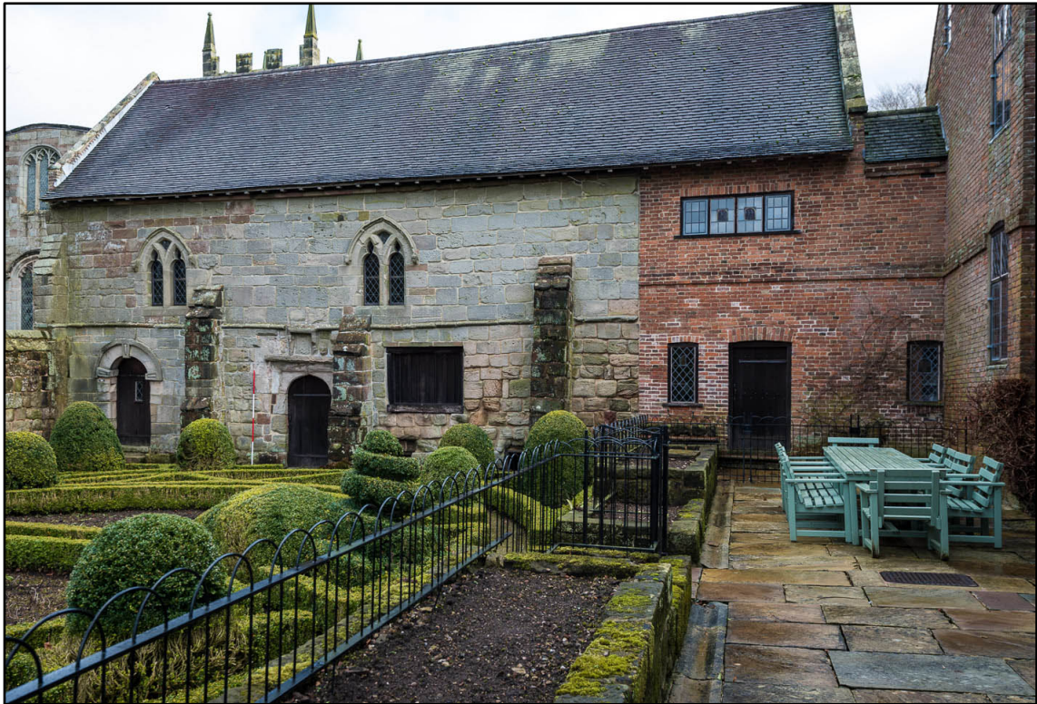
Appendix 5.77: General view of west elevation of Building 2 (2m scale) (Photo 29)
