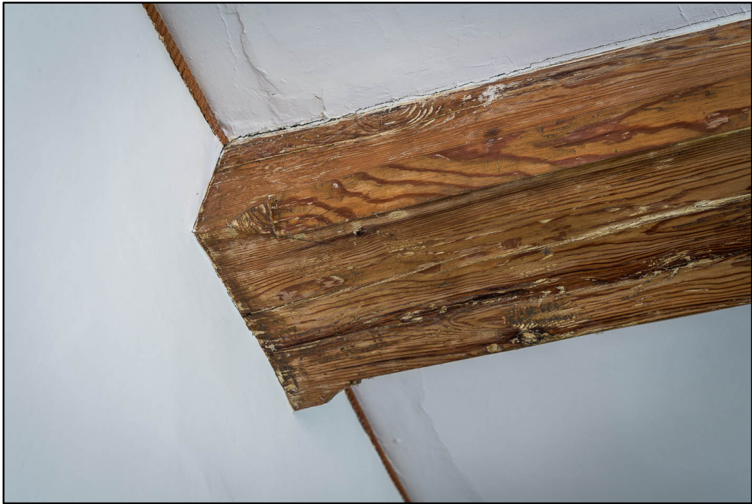
Appendix 5.49: Detail of ceiling beam in F2; note runout stops (Photo 113)
