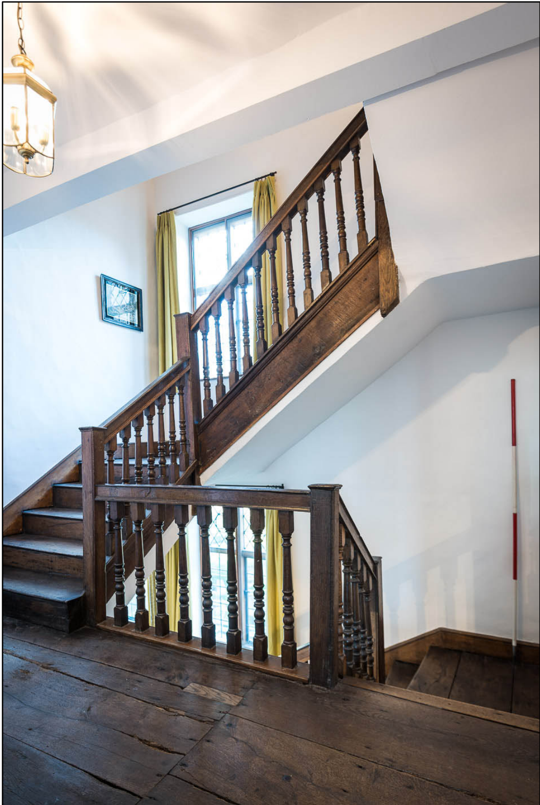
Appendix 5.54: General view of staircase FI, looking northwest (2m scale) (Photo 115)
