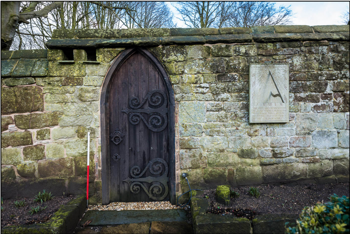
Appendix 5.21: Detail of false doorway in north garden wal, looking north (1m scale) (Photo 18)
