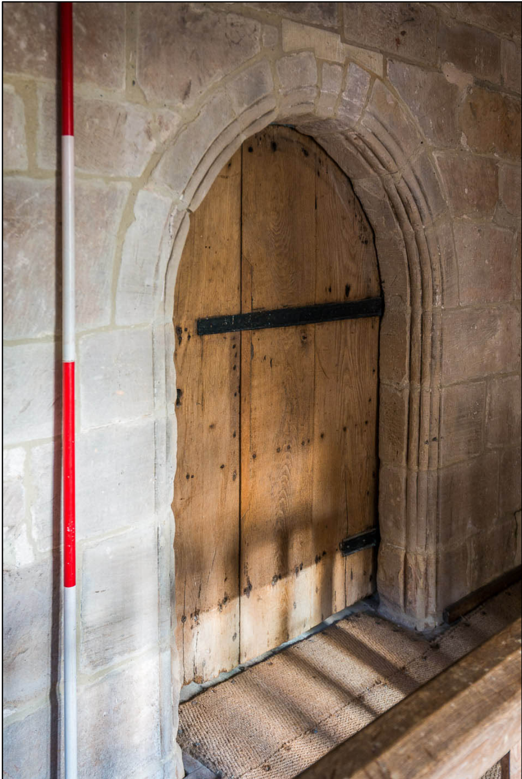
Appendix 5.120: Detail of doorway between F12 and F13 (2m scale) (Photo 56)
