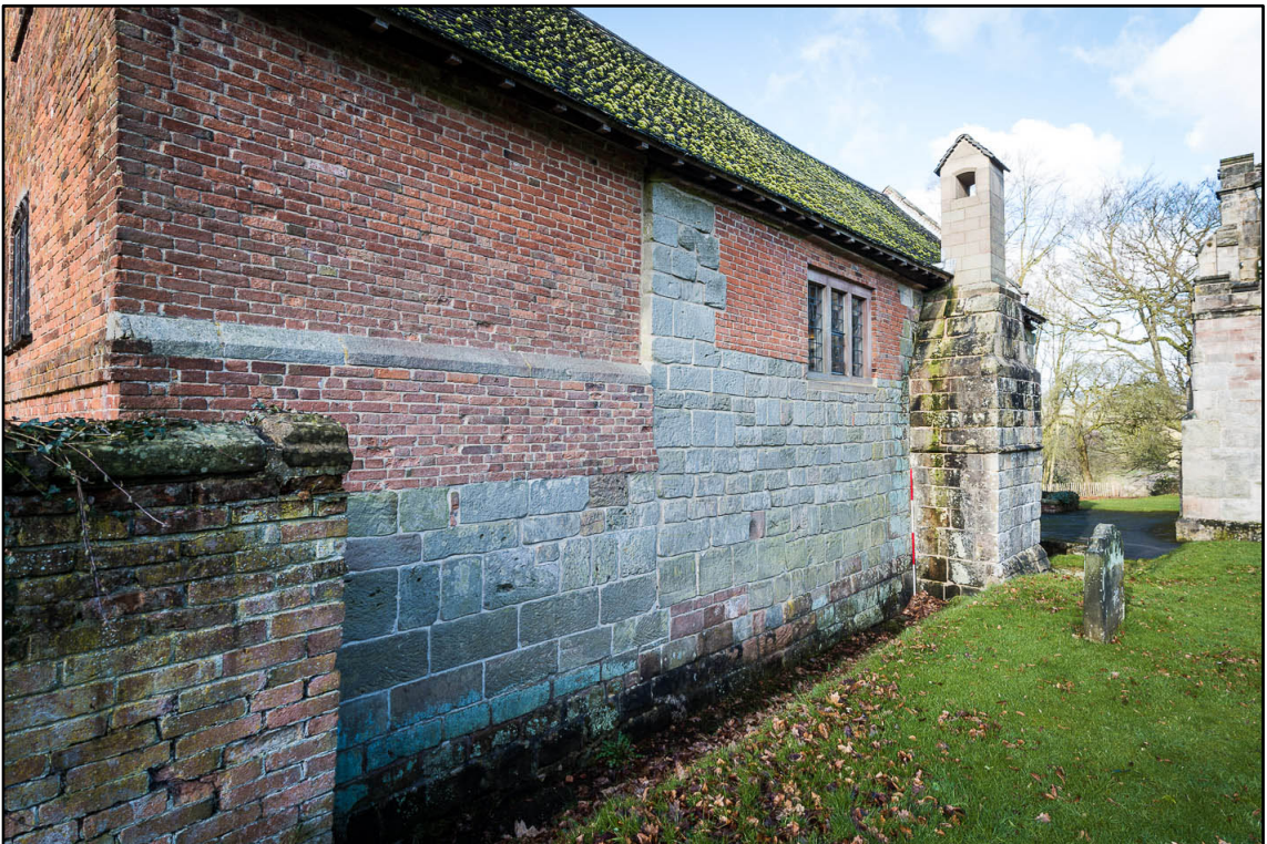
Appendix 5.84: East elevation of Building 2, looking northwest (2m scale) (Photo 48)
