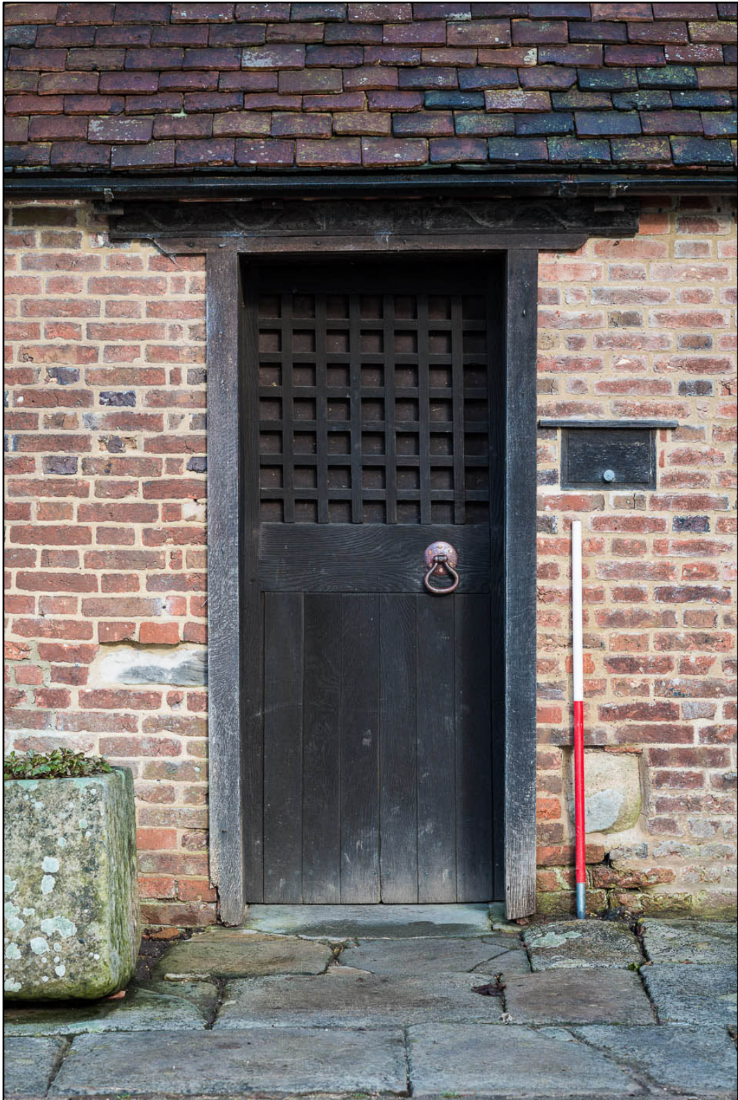
Appendix 5.20: Detail of inserted doorway to east courtyard (1 m scale) (Photo 33)
