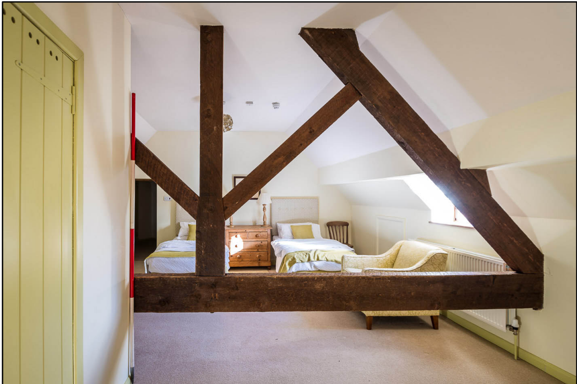
Appendix 5.72: General view of S5, looking east (2m scale) (Photo 103)
