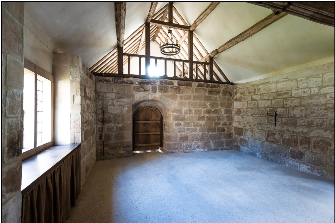
Appendix 5.129: General view of south wall in F13 (2m scale) (Photo 61)
