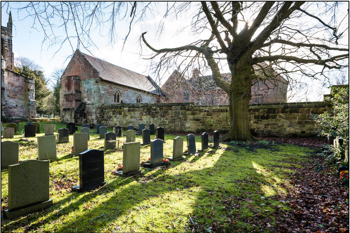
Appendix 5.7: View of Old Hall (Building 2), looking southeast (2m scale) (Photo 42)
