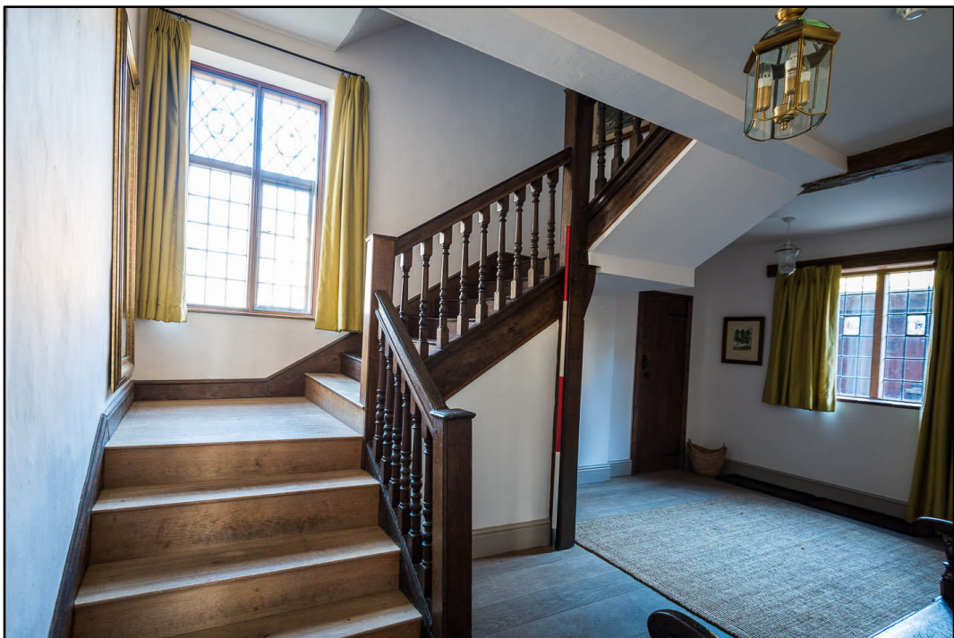
Appendix 5.41: Detail of staircase in GI looking northeast (2m scale) (Photo 137)
