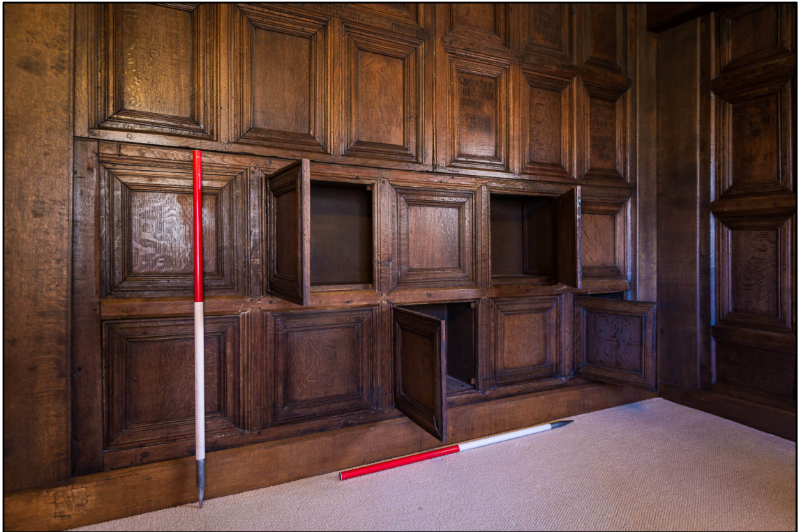
Appendix 5.66: Hidden cupboards in F8, looking southwest (1m scale) (Photo 133)
