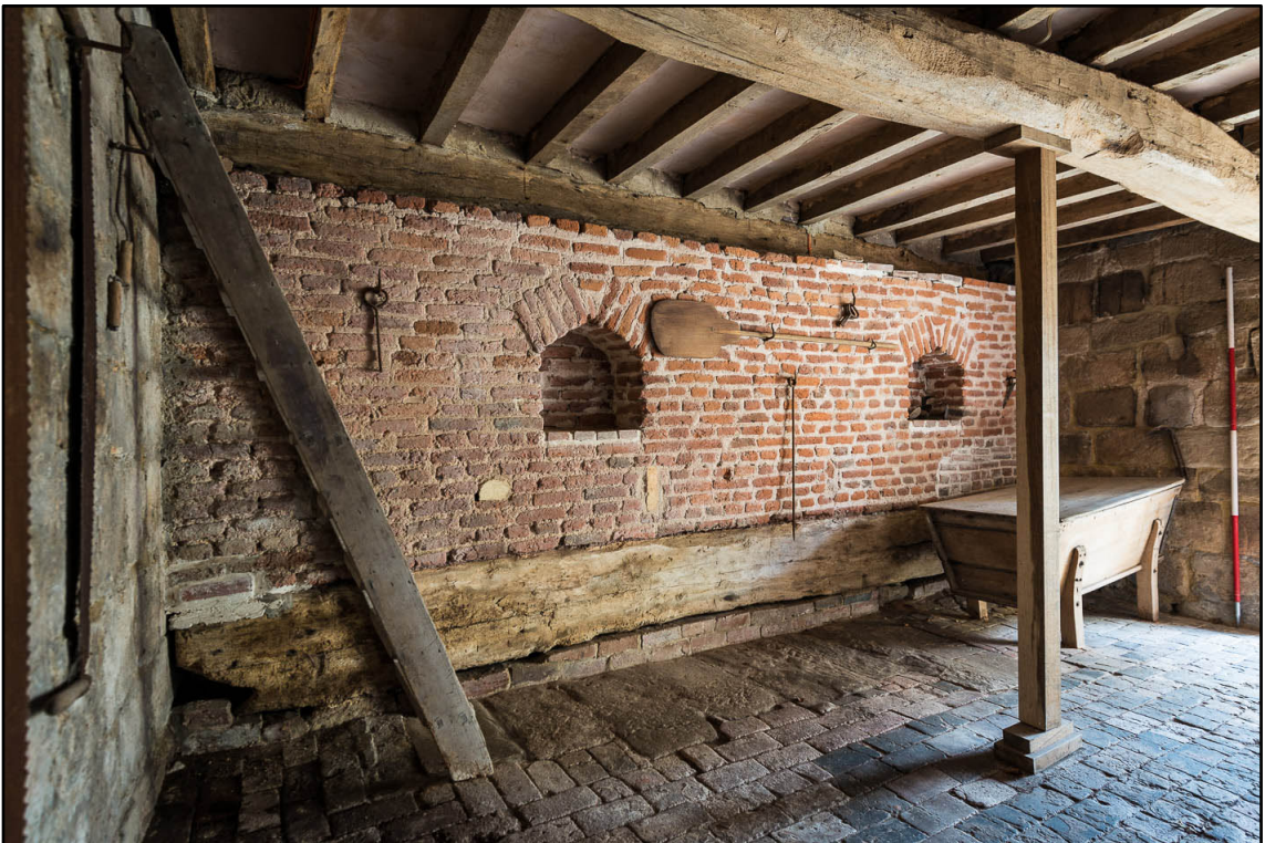
Appendix 5.113: General view of G12, looking southwest (2m scale) (Photo 96)
