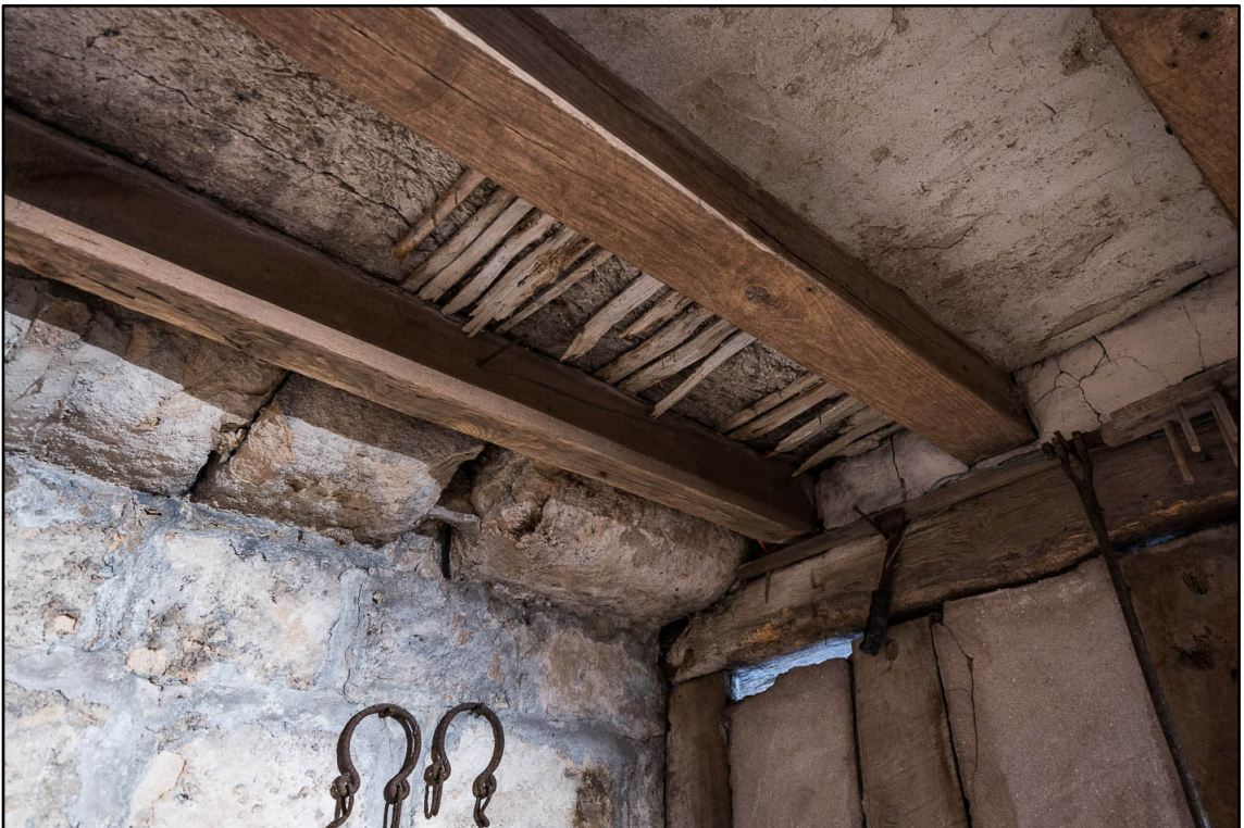
Appendix 5.II1: Detail of exposed ceiling laths in G11; note hearthstone corbels (Photo 85)
