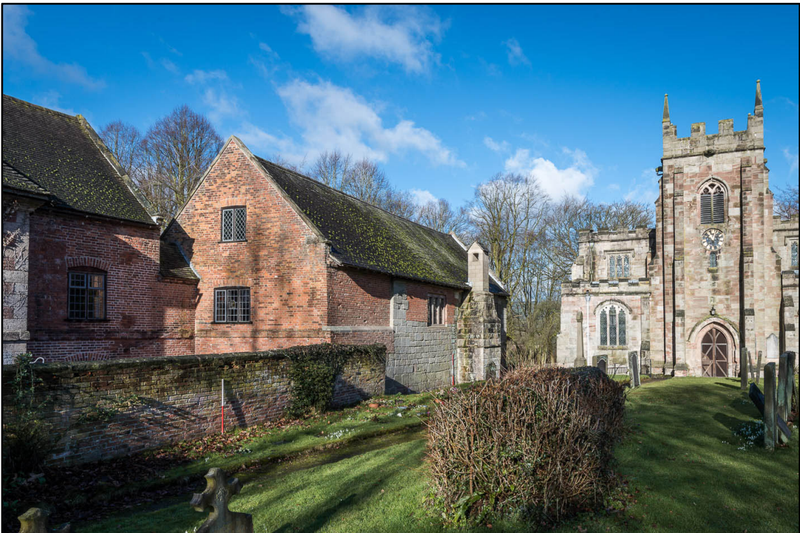
Appendix 5.6: View of Old Hall (Building 2), looking northwest (2m scale) (Photo 40)
