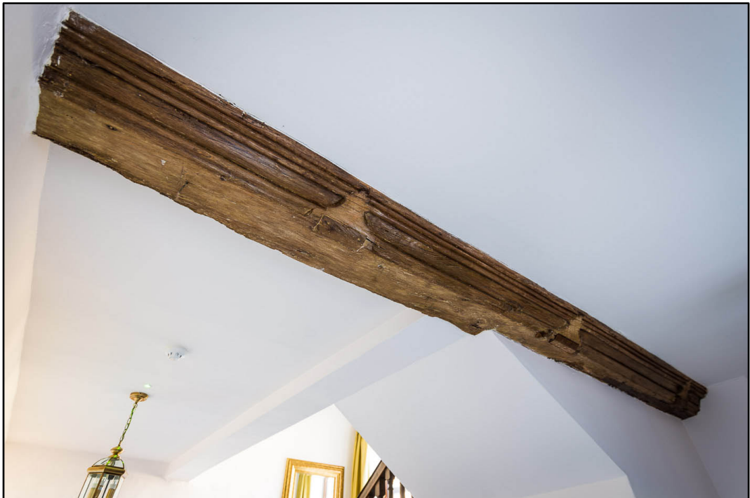
Appendix 5.38: Detail of re-used beam in G1 (Photo I36)
