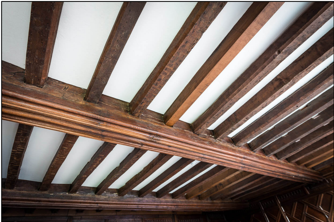
Appendix 5.34: Detail of ceiling joists in G4; note moulded beams (Photo 157)
