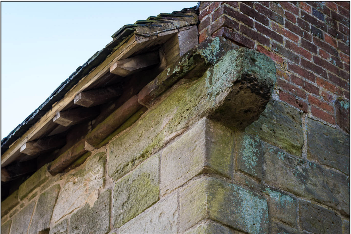
Appendix 5.83: Detail of northeast corner of Building 2; note projecting corbel (Photo 46)
