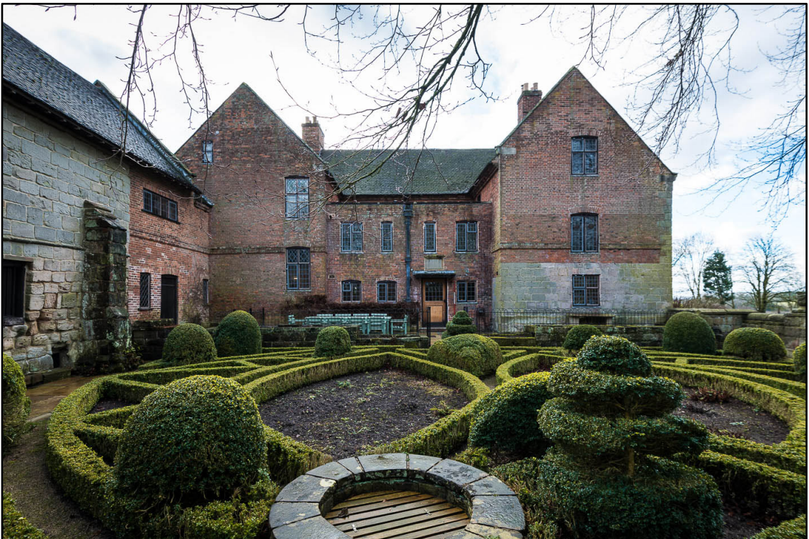
Appendix 5.22: View of north elevation of (Building 1) (2m scale) (Photo 25)
