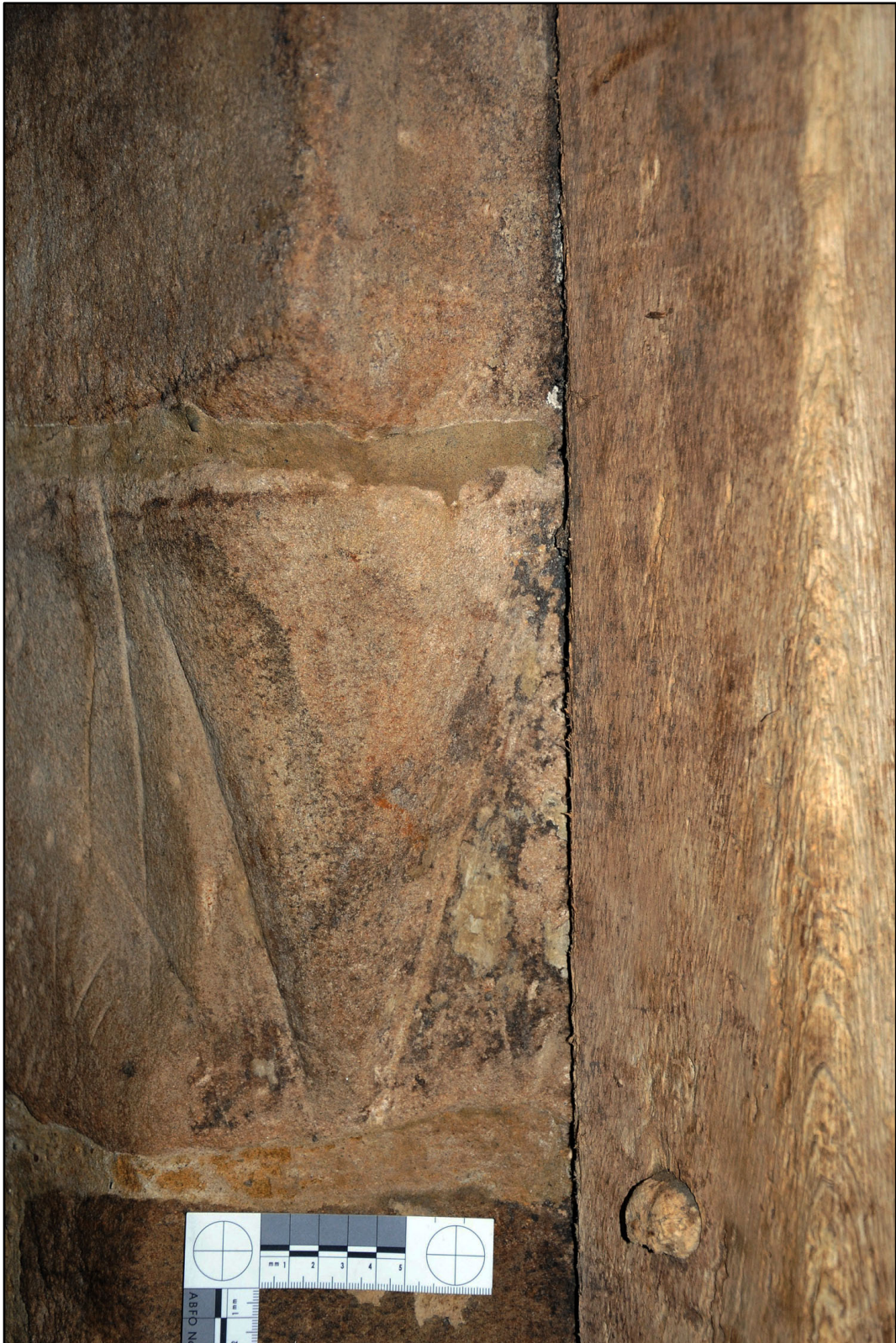
Appendix 5.99: Detail of moulding on door reveal in south wall of G10 (20cm) (Photo 176)
