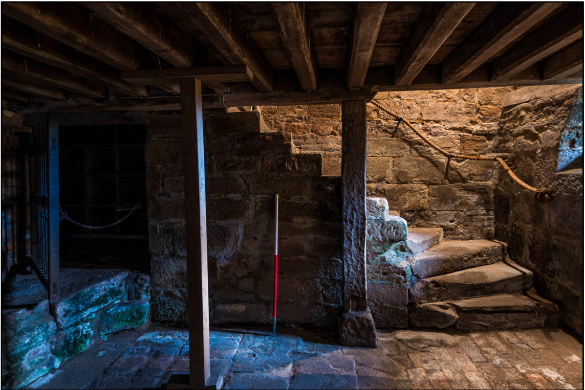
Appendix 5.86: View of south wall of BI (1m scale) (Photo 90)
