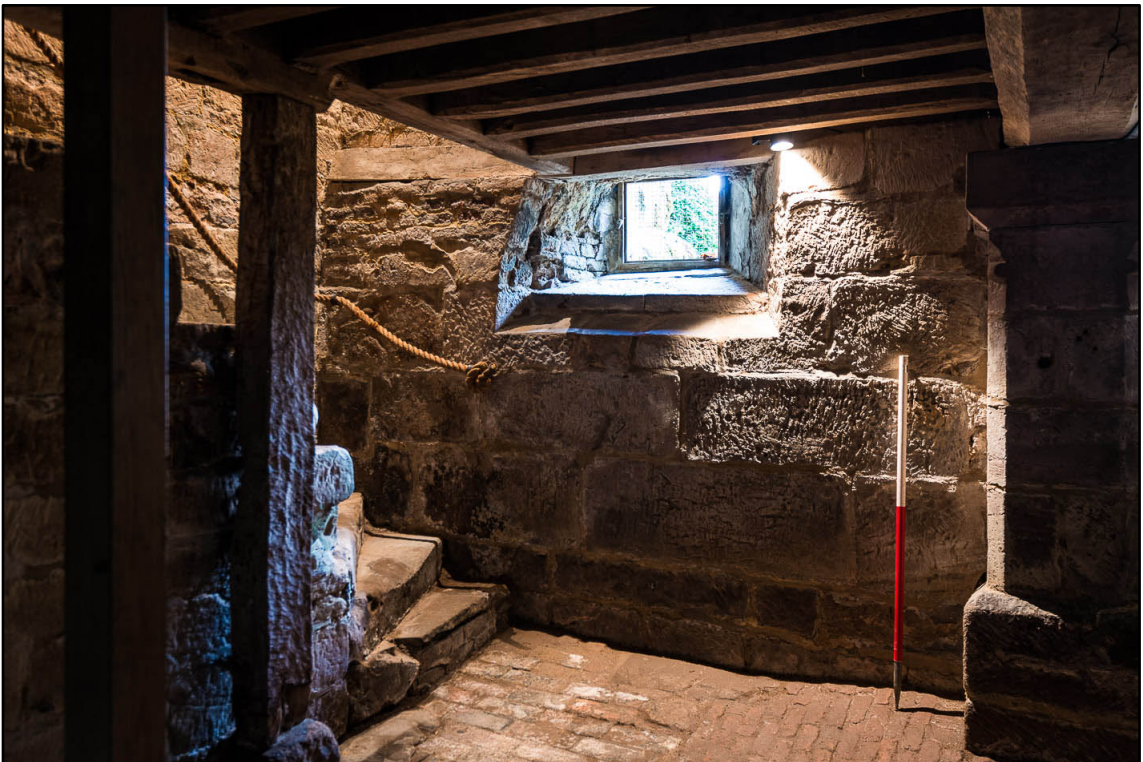
Appendix 5.87: View of southwest wall of BI (1m scale) (Photo 89)
