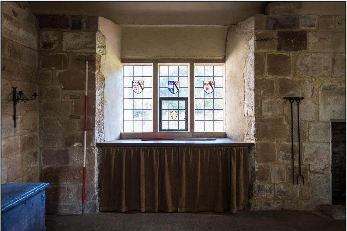
Appendix 5.132: Detail of inserted window in northeast wall of F13 (2m scale) (Photo 69)
