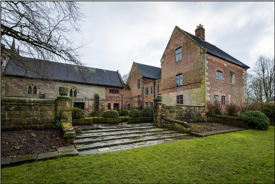
Appendix 5.9: View of Old Hall (Building 2), looking southeast (Photo 14)
