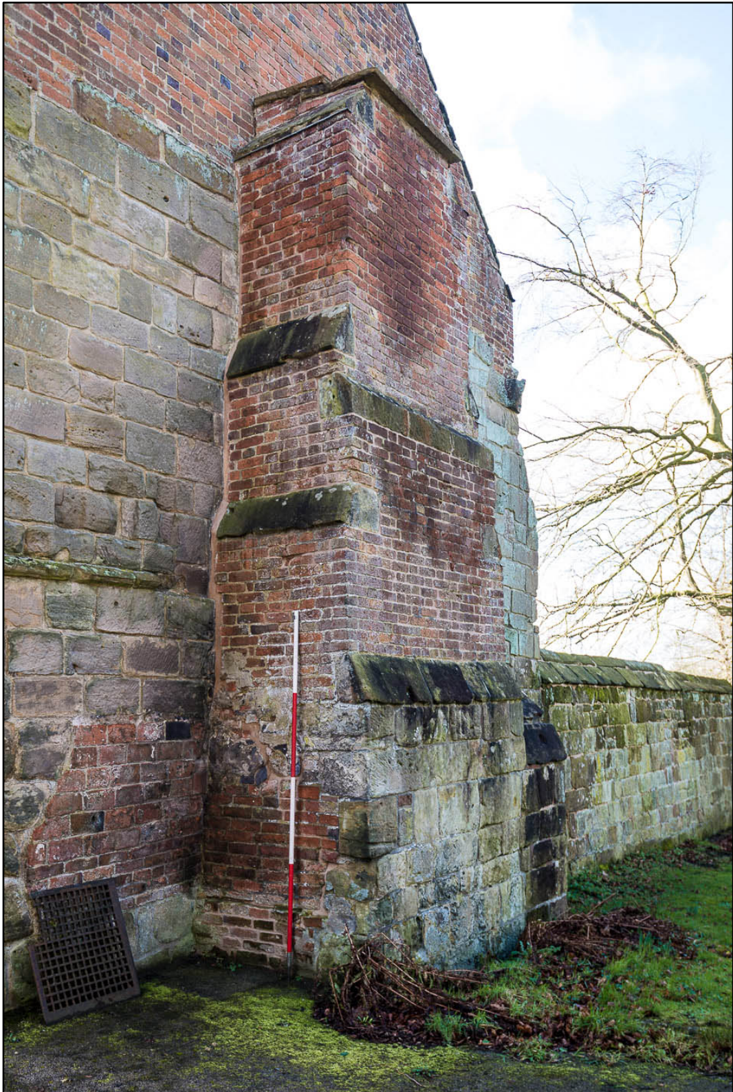
Appendix 5.82: North gable of Building 2, looking southwest (2m scale) (Photo 45)
