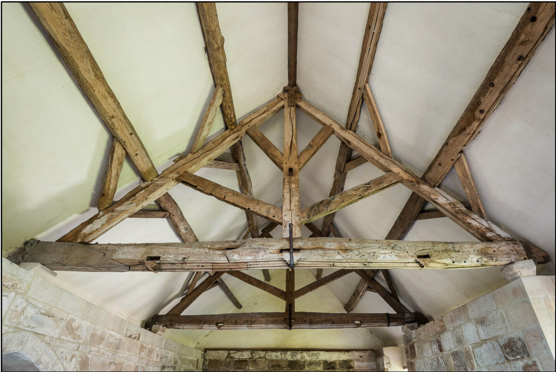
Appendix 5.124: Detail of roof trusses in F13, looking north (Photo 60)
