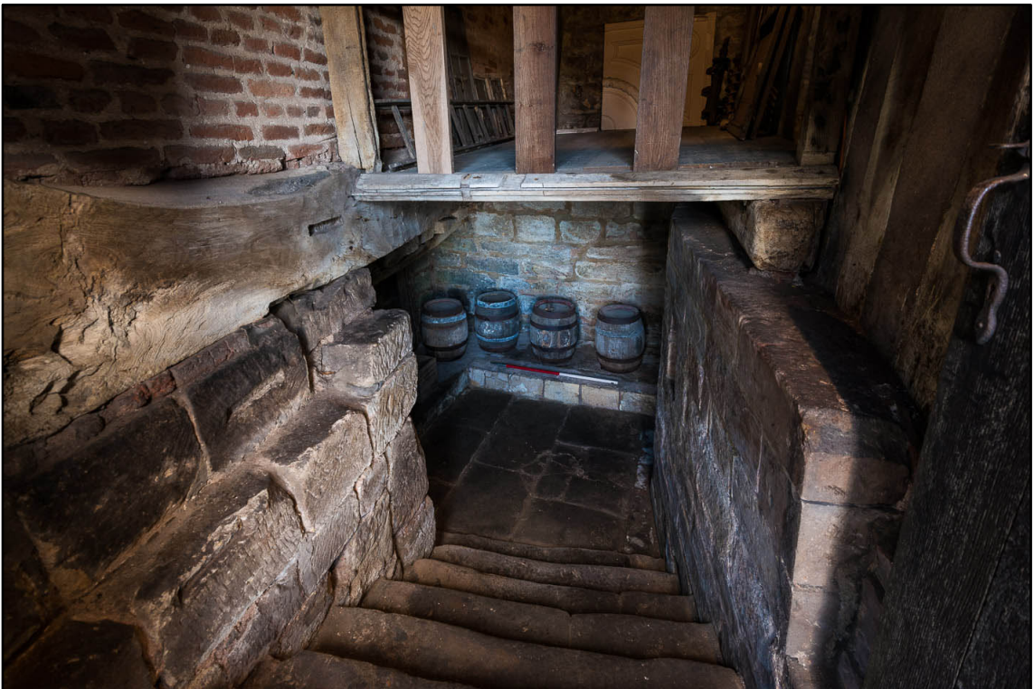
Appendix 5.91: Detail looking down steps into B2 (1 m scale) (Photo 92)
