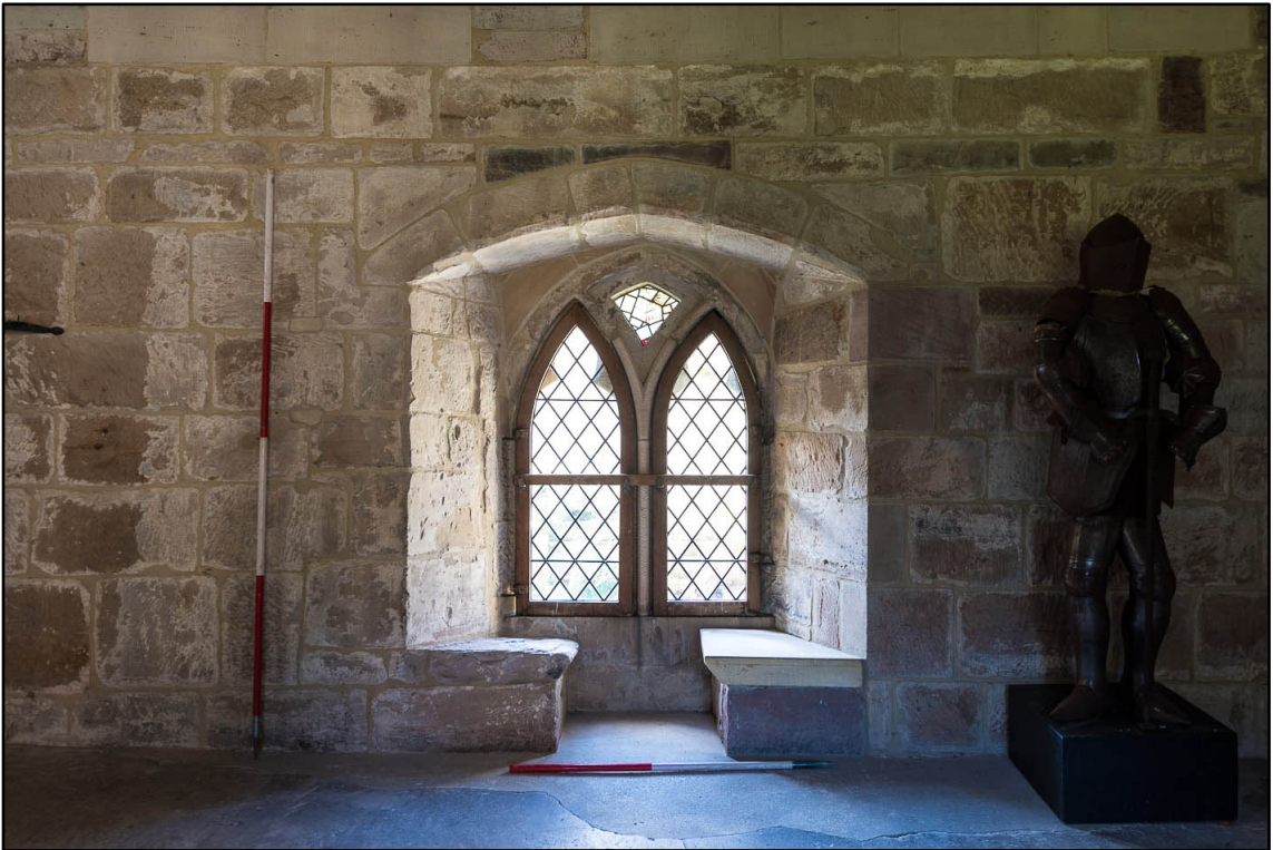
Appendix 5.130: Detail of northwest window in F13 (1m/2m scale) (Photo 67)
