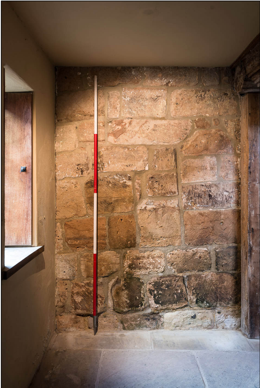
Appendix 5.96: Detail of blocked window in south wall of G9 (2m scale) (Photo 72)
