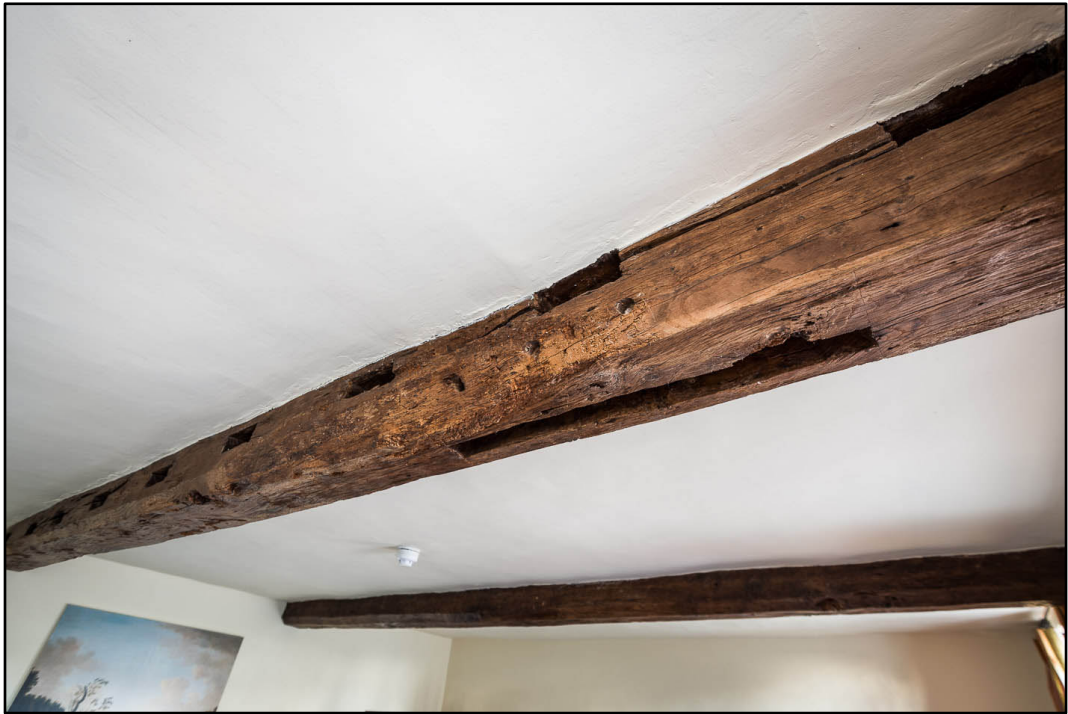
Appendix 5.37: Detail of ceiling beam in G3; note redundant mortices (Photo I47)
