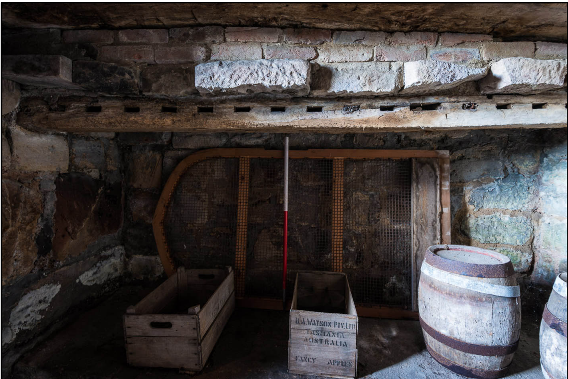
Appendix 5.93: General view of north wall of B2 (1m scale) (Photo 93)
