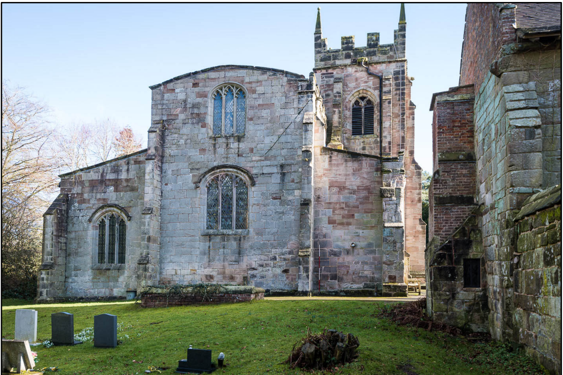
Appendix 5.8: General view of west gable of Church (2m scale) (Photo 44)
