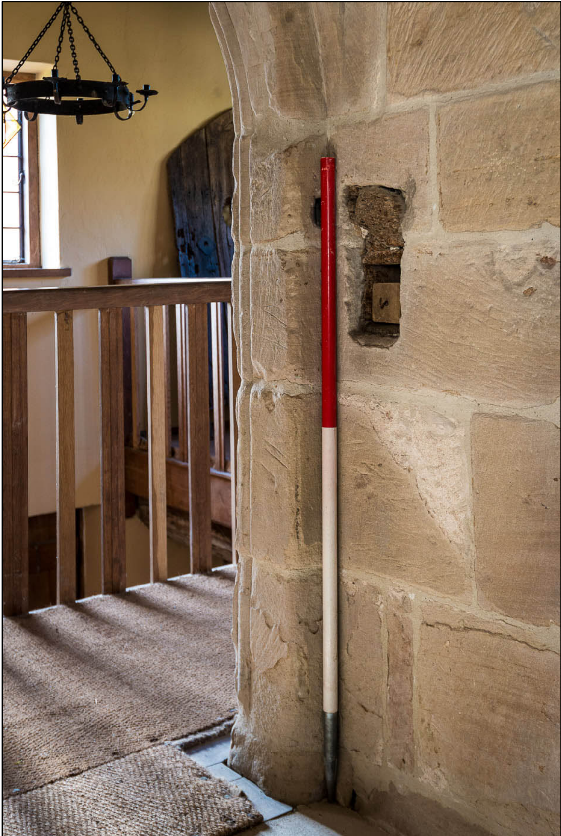
Appendix 5.121: Detail of doorway between F13 and F12 (1m scale) (Photo 57)
