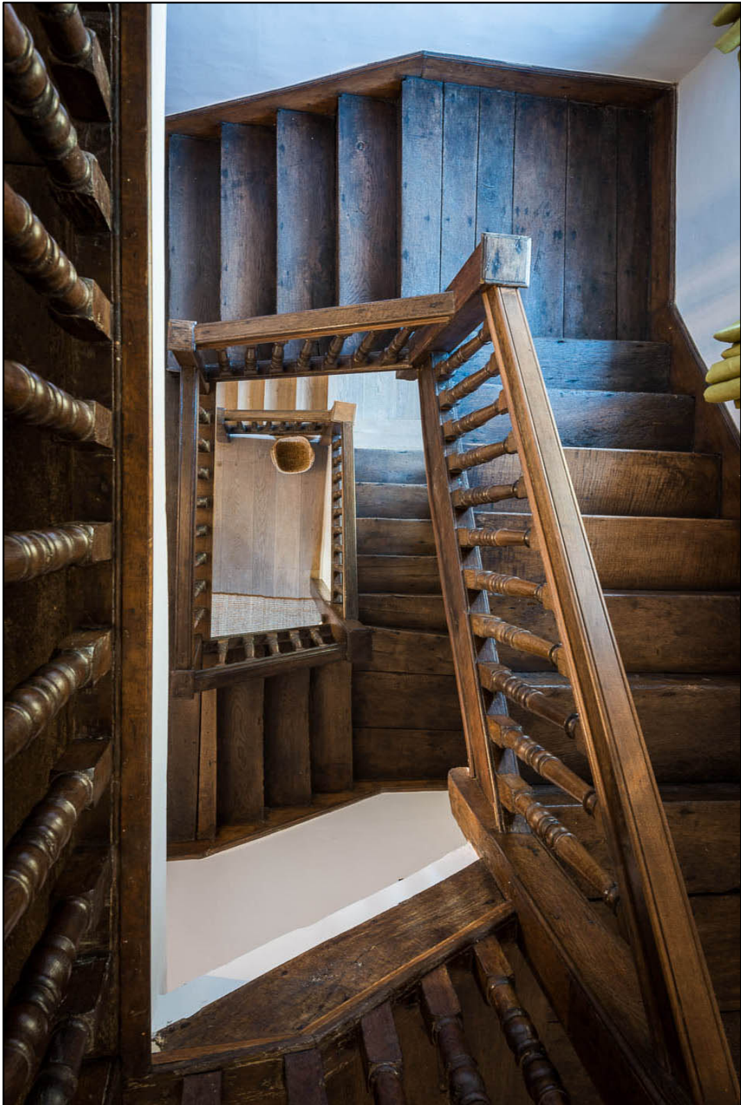
Appendix 5.68: View looking down staircase S1 (Photo 118)
