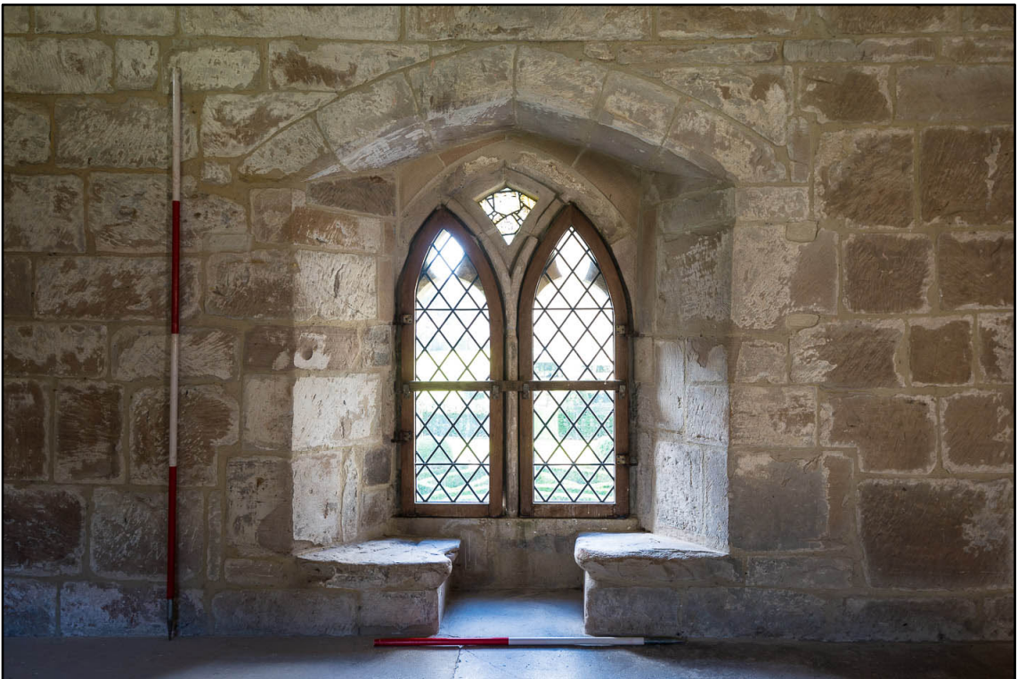
Appendix 5.131: Detail of northeast window in F13 (1m/2m scale) (Photo 63)
