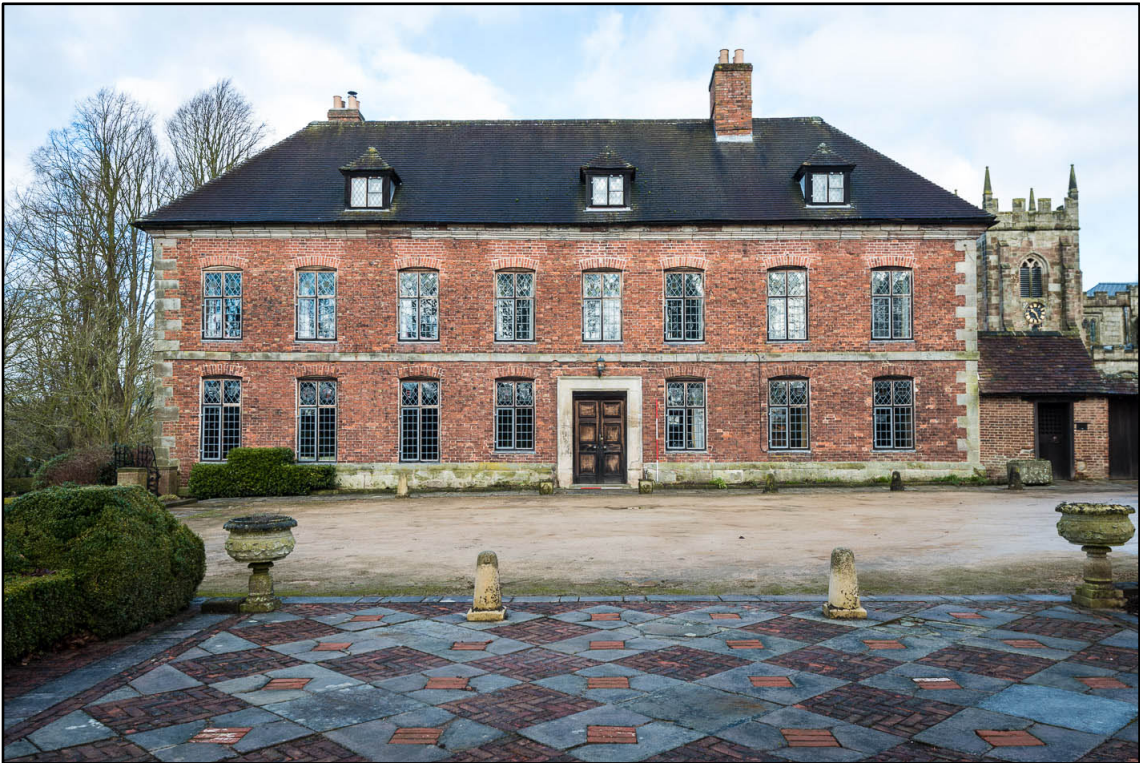
Appendix 5.16: Detail of façade of Building I, looking north (1m/2m scale) (Photo 1)
