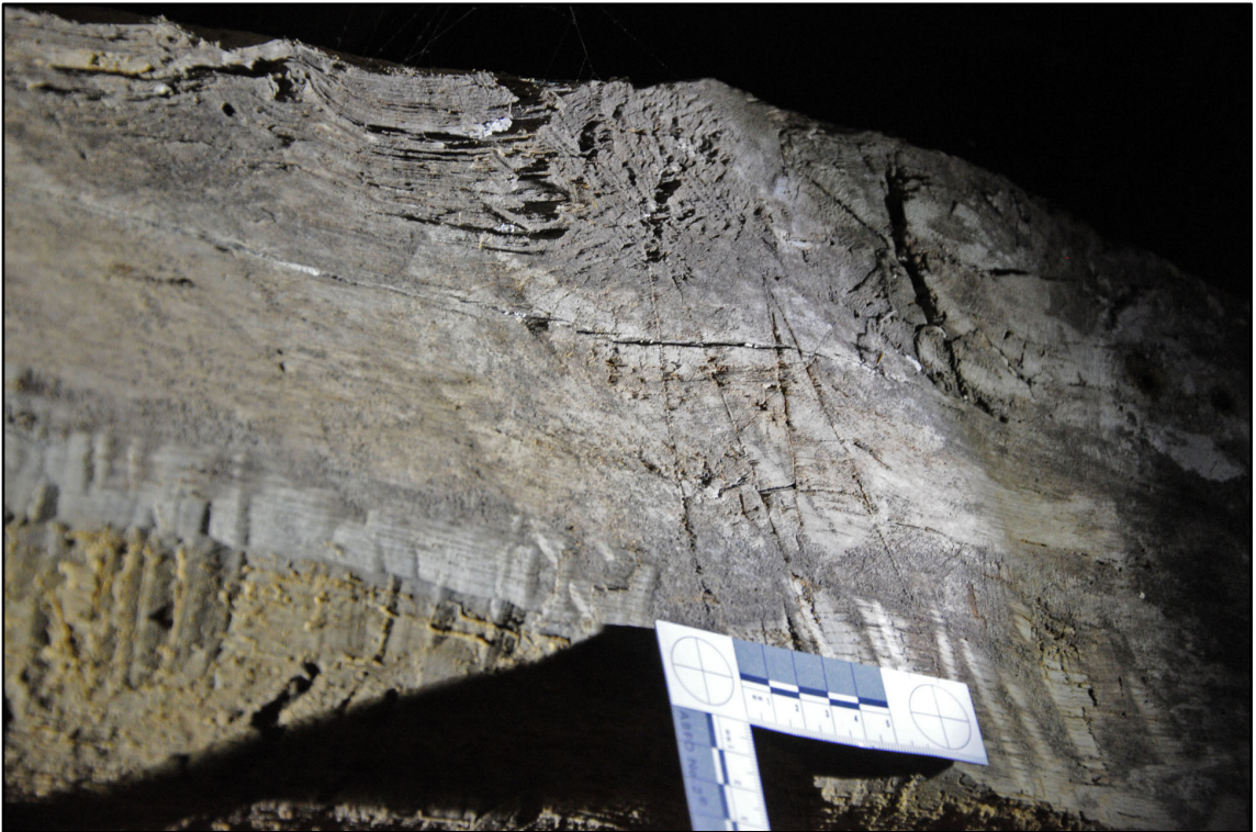
Appendix 5.108: Carpentry mark on timber above doorway in to G10 (5cm scale) (Photo 177)
