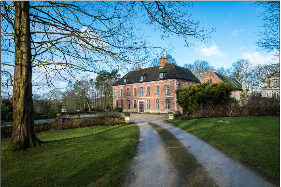
Appendix 5.1: General view of Norbury Manor (Building I), looking northwest (Photo 4)
