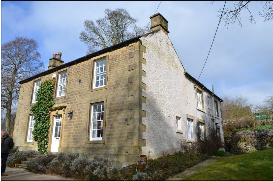
Appendix 2.1: South Elevation of Brough House, looking northwest
