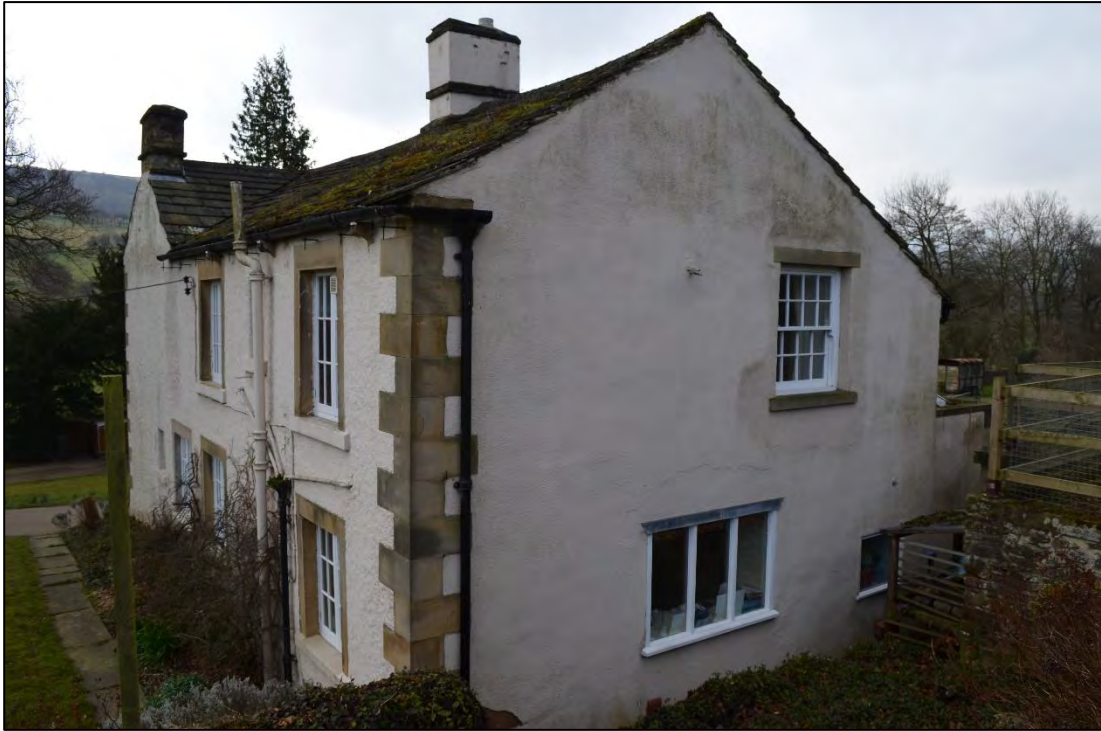
Appendix 2.5: North Elevation of Brough House looking southwest
