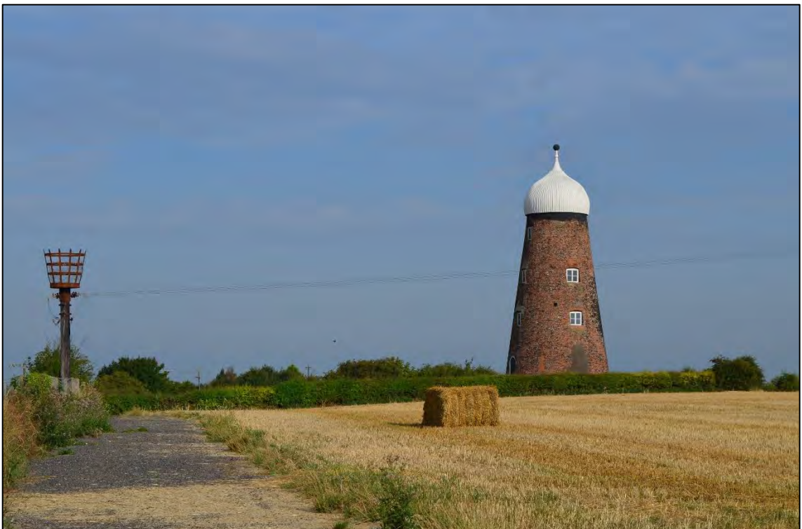
Appendix 2.4: View of Grade II Listed Maw's Mill to the northwest of the site
