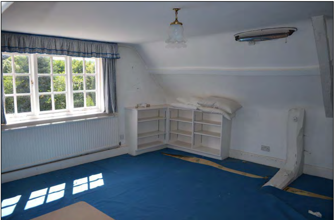
Appendix 2.20: General view of S2 looking south-east
