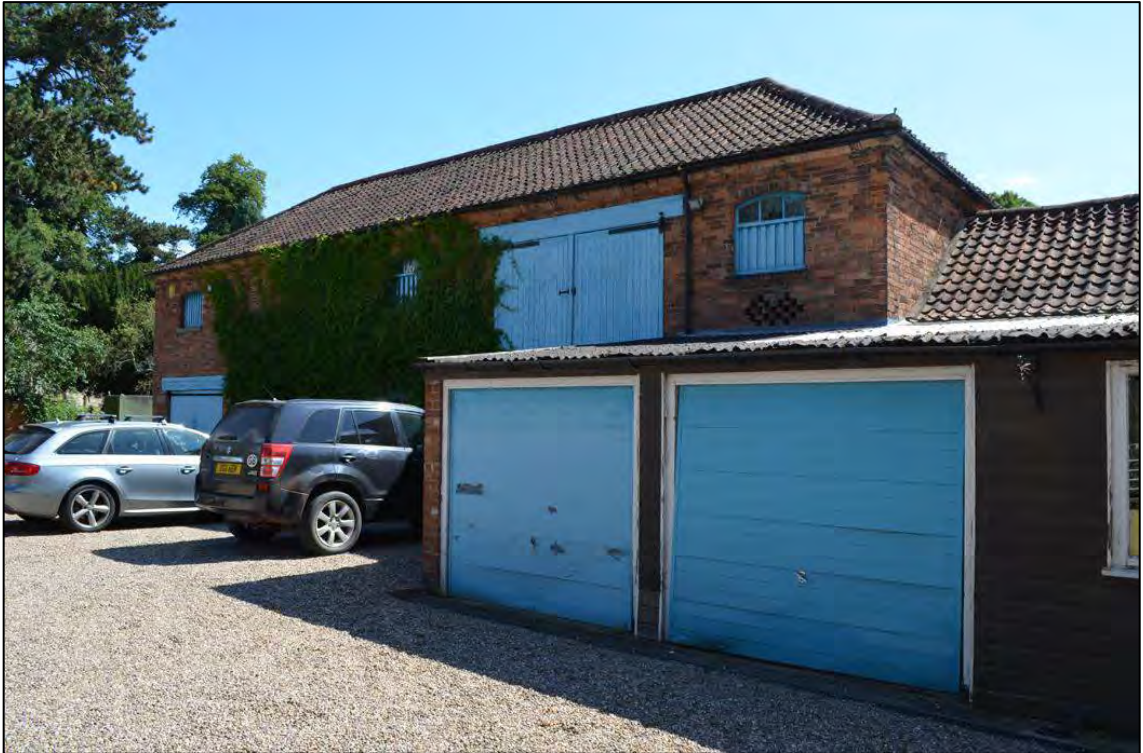
Appendix 2.29: General view of Building 4, looking south-west
