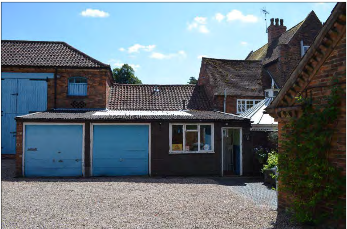
Appendix 2.24: General view of Buildings 2 and 3, looking east, noting modern garage in front
