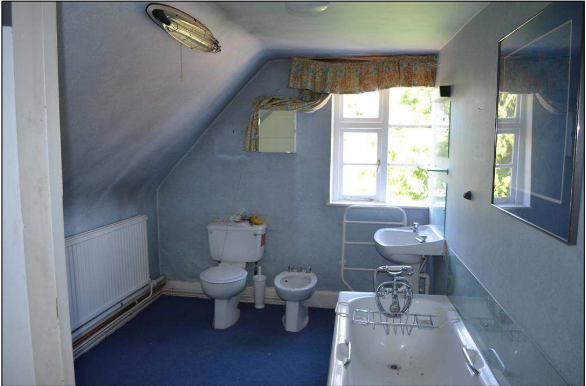
Appendix 2.21: General view of S3 in Building 1, looking west
