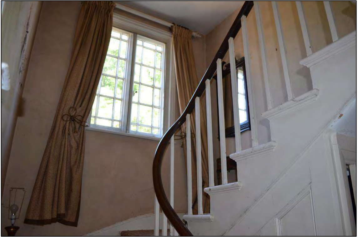
Appendix 2.15: General view of staircase in GI in Building I, looking north-west
