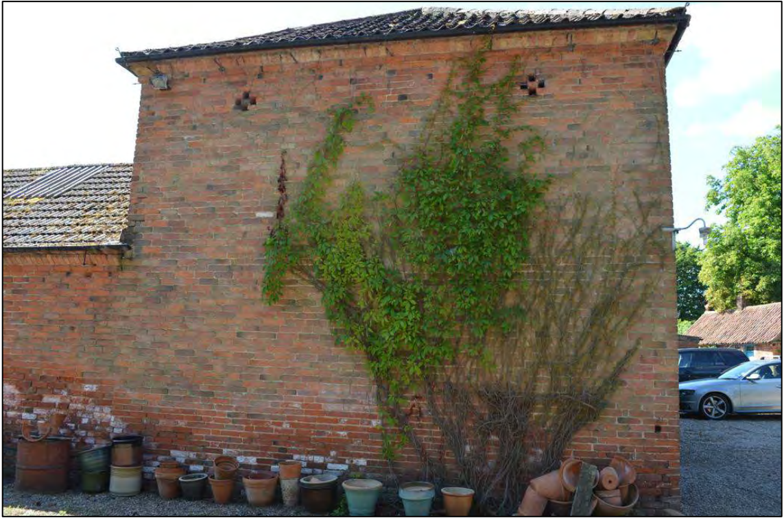
Appendix 2.31: Detail of north elevation of Building 4
