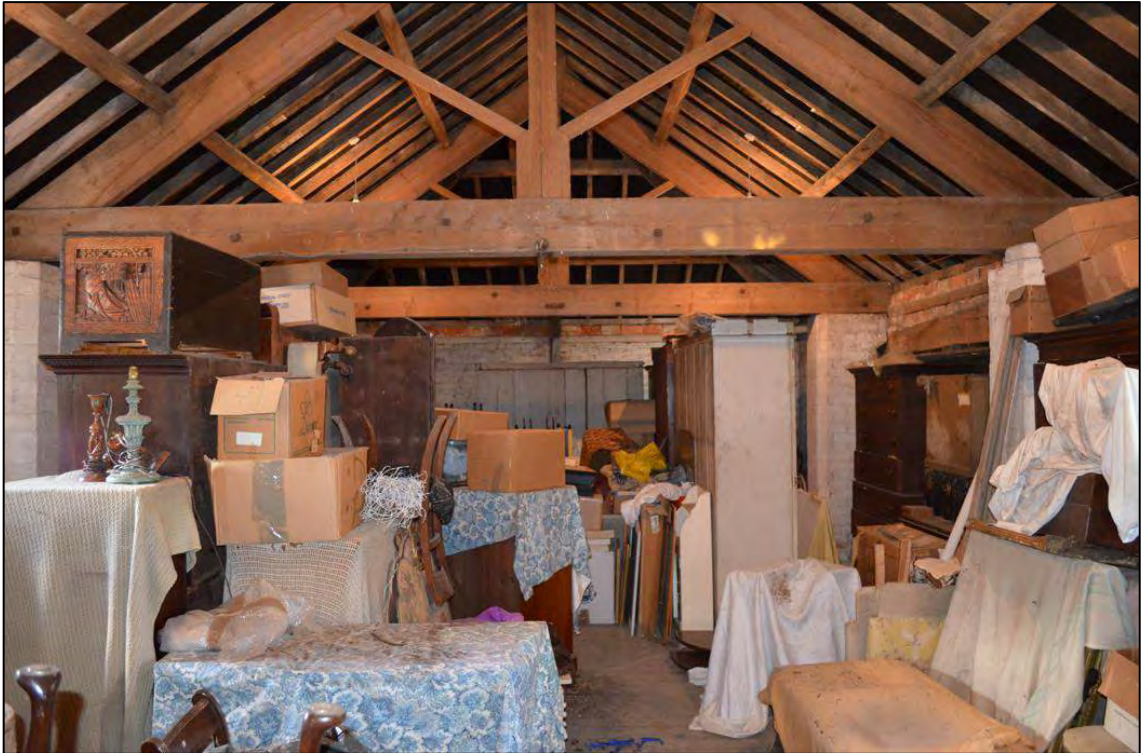
Appendix 2.35: General view of interior of F8 in Building 4, looking south
