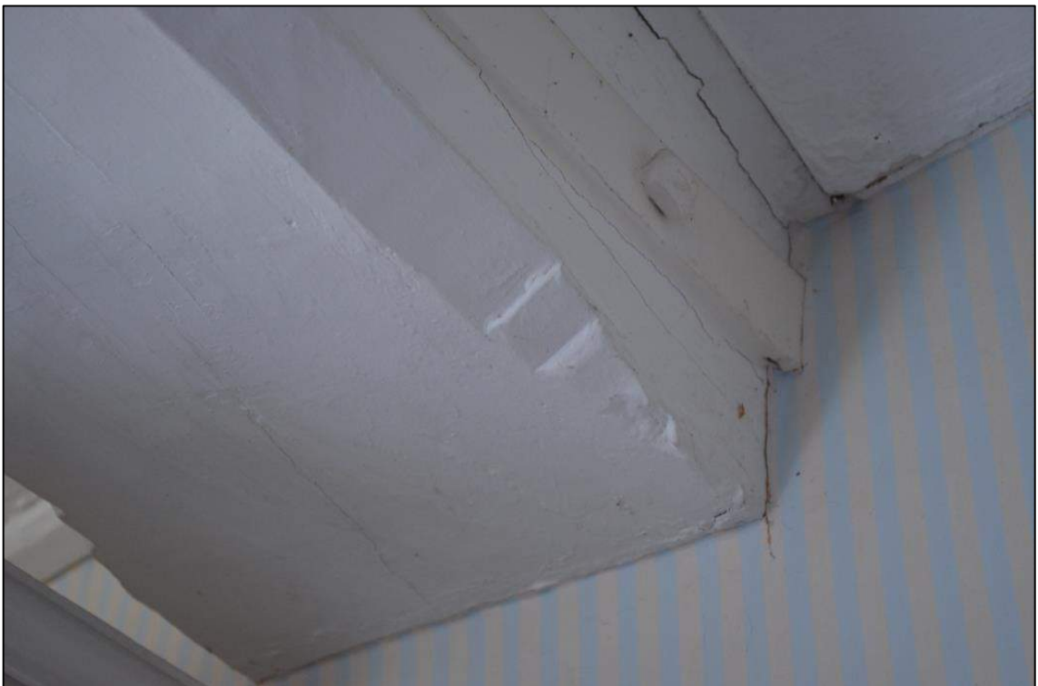
Appendix 2.18: Detail of scroll and notch stop on chamfered beam in F3
