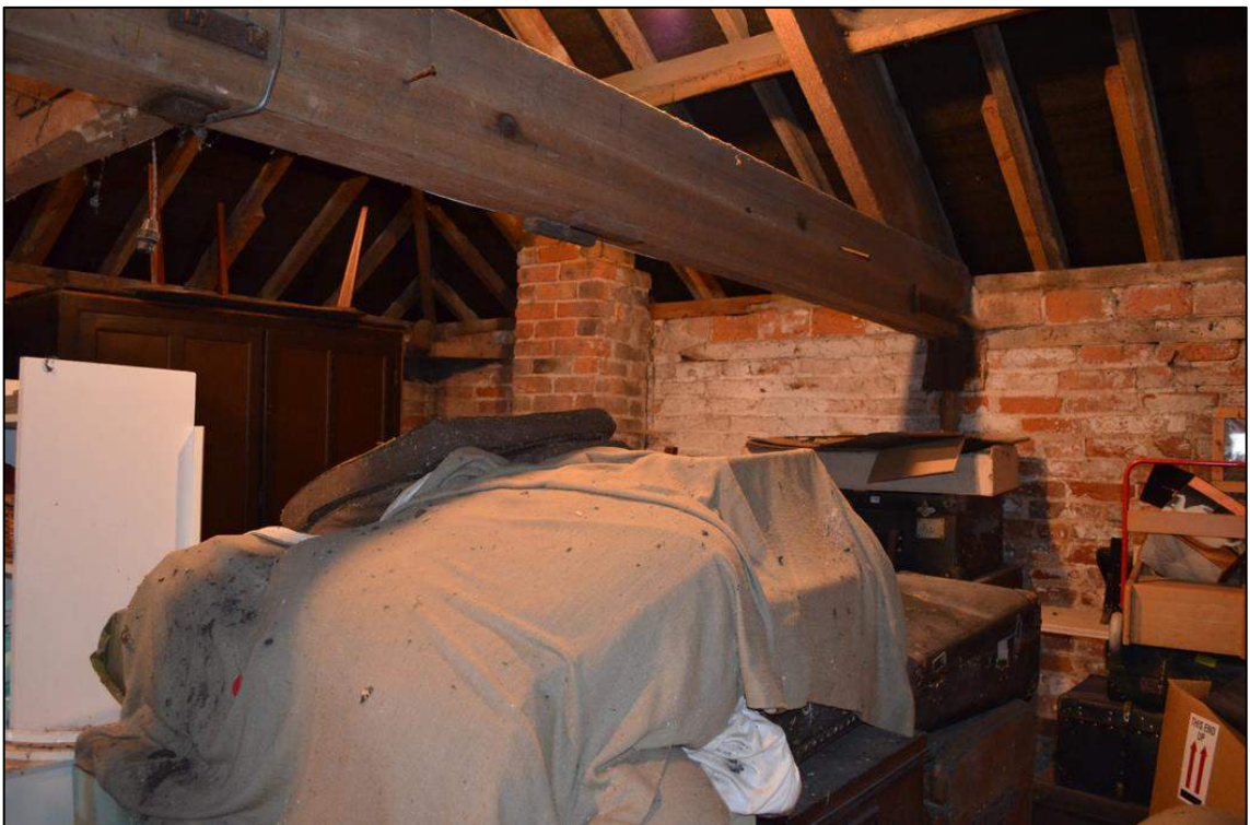
Appendix 2.38: General view of interior of F9 in Building 4, looking northwest
