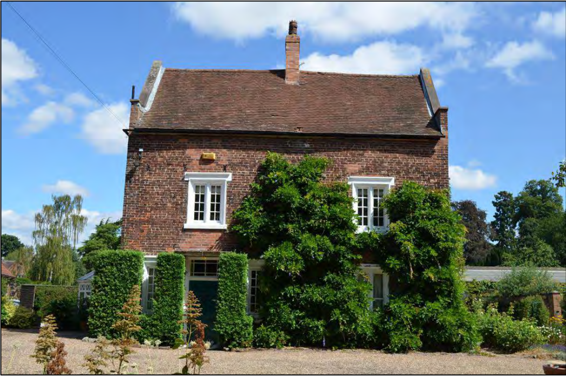
Appendix 2.9: South elevation of Building I
