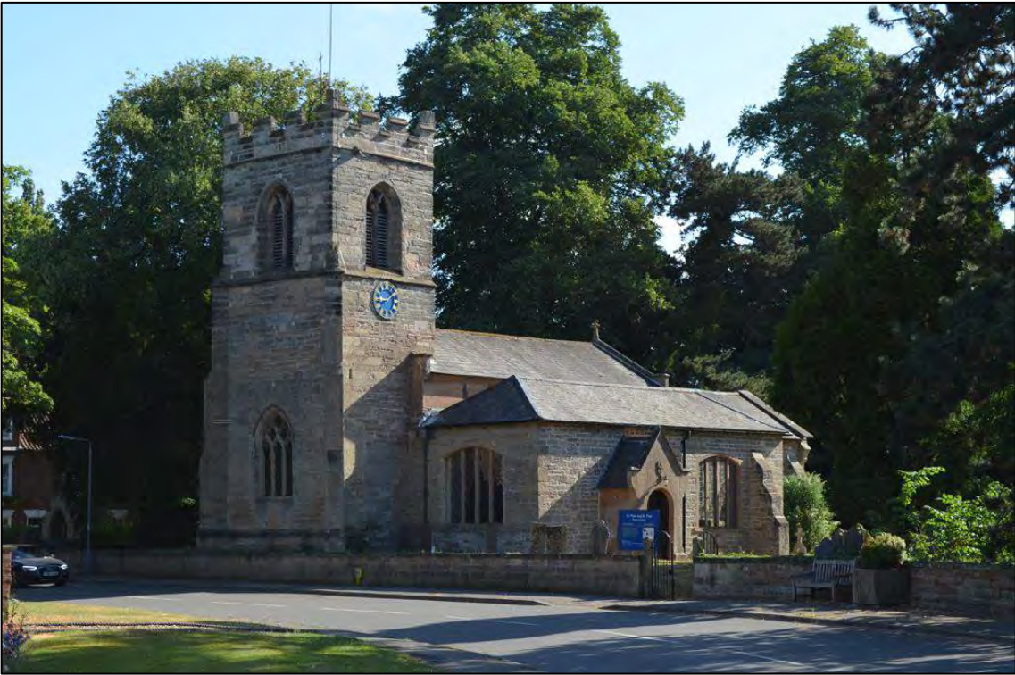
Appendix 2.4: Church of St Peter and St Paul, looking north-east
