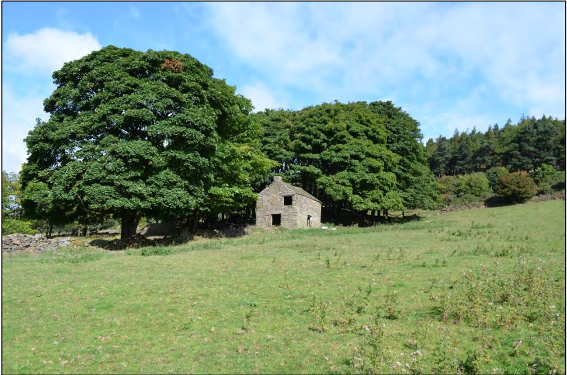
Appendix 2.1: General view of the site, looking north-west (scale: 2m)
