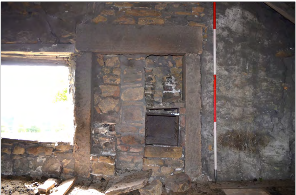
Appendix 2.12: Detail of fire place in FI (scales: 2m & 10cm)
