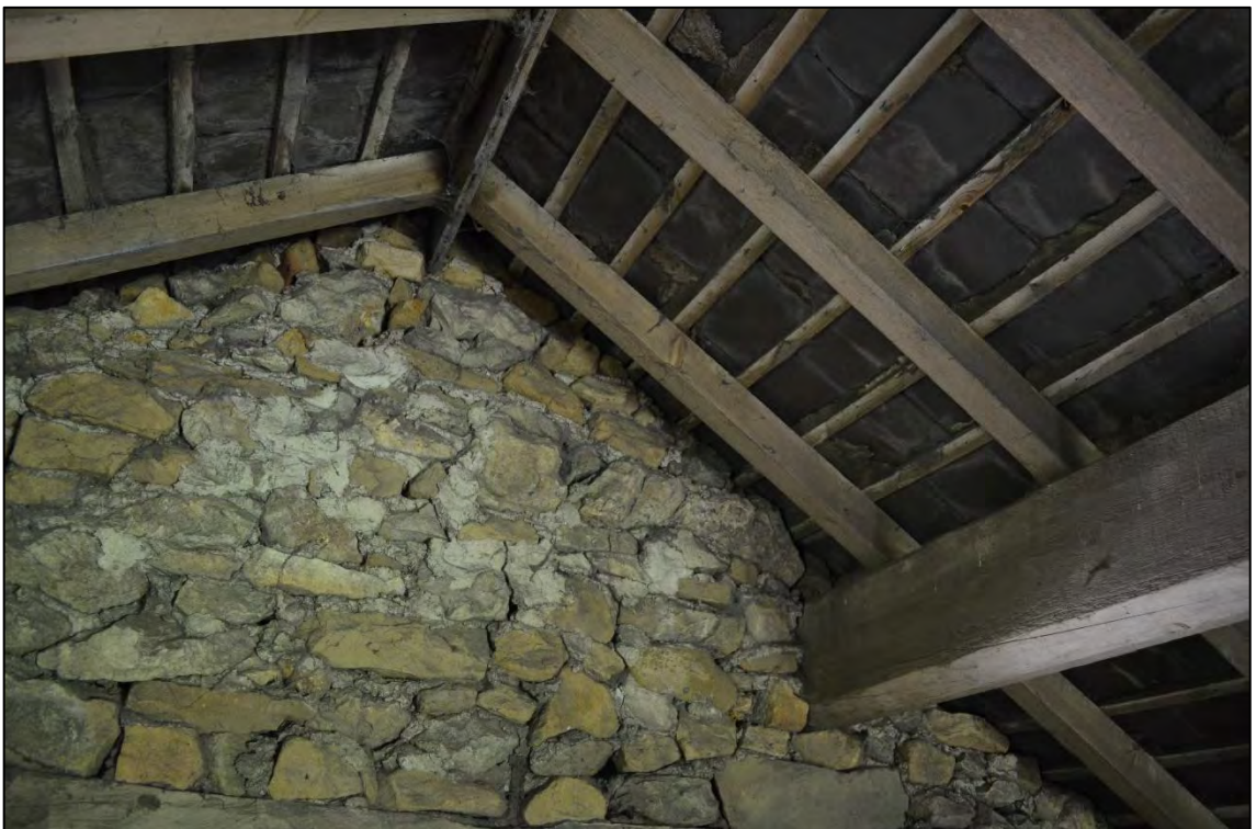
Appendix 2.14: Detail of replaced roof structure above FI
