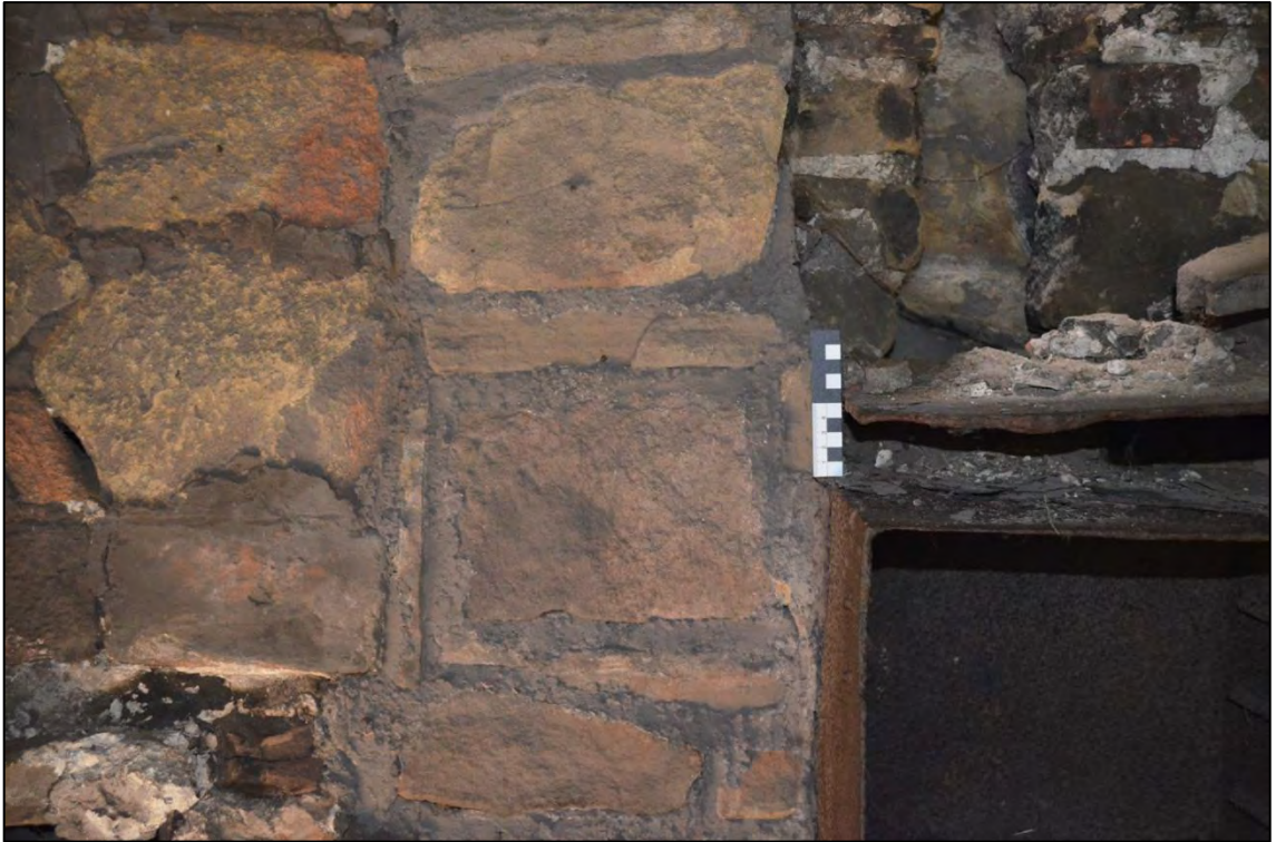
Appendix 2.13: Detail of blocking in back of fireplace (scale: 10cm)
