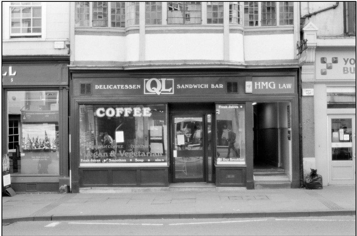
Appendix 2.2: Detail of shopfront, looking south (2m scale; Film 1.04)
