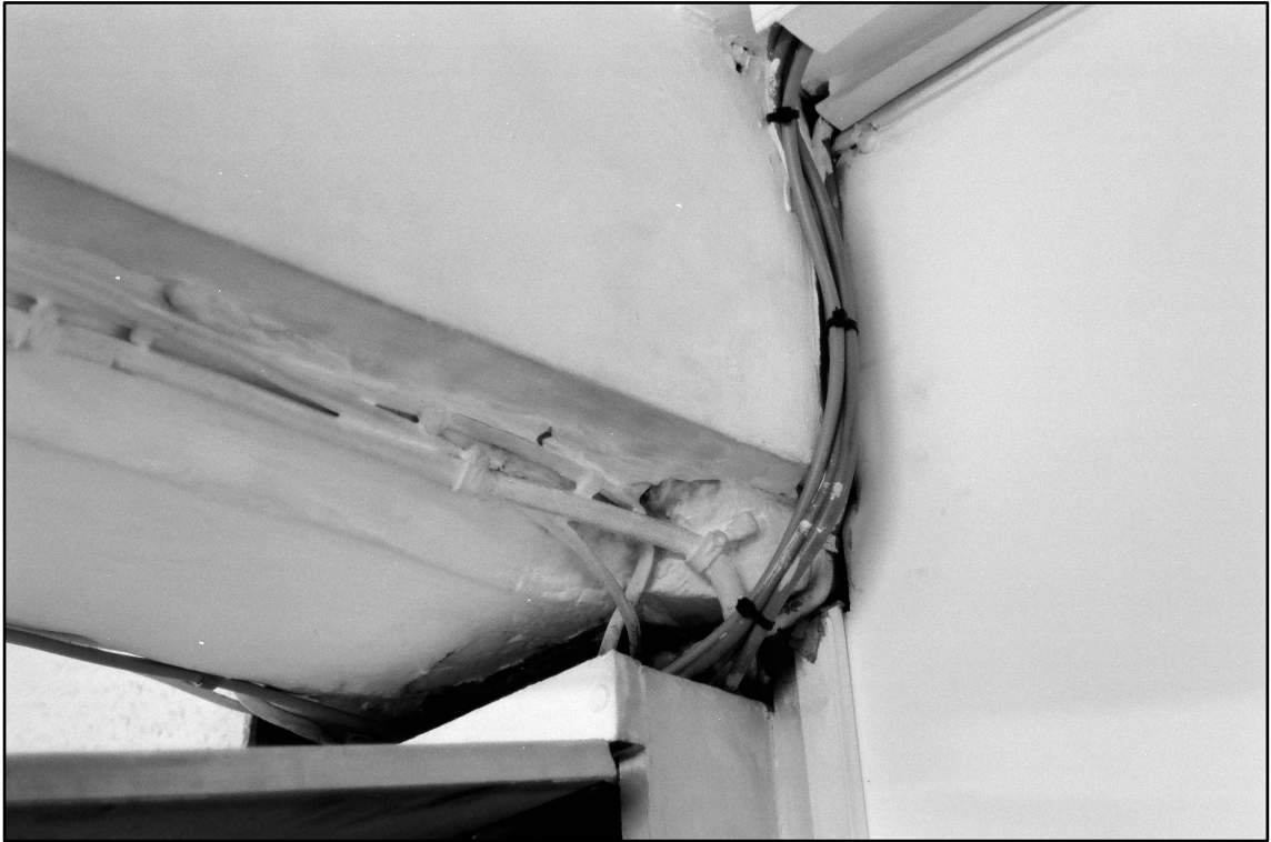
Appendix 2.15: Detail of beam stop in CI, looking north-west (Film 1.33)
