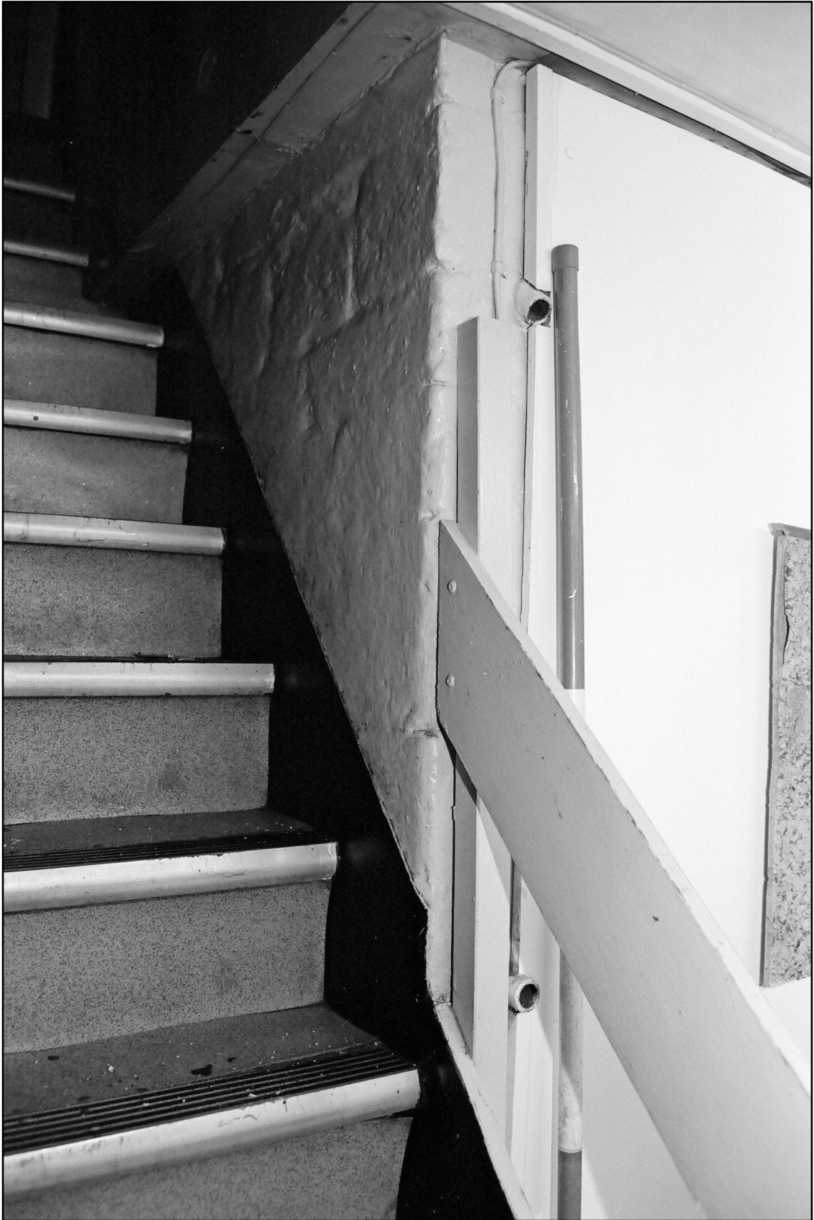
Appendix 2.10: Detail looking up the stairs in CI (2m scale; Fim 1.25)
