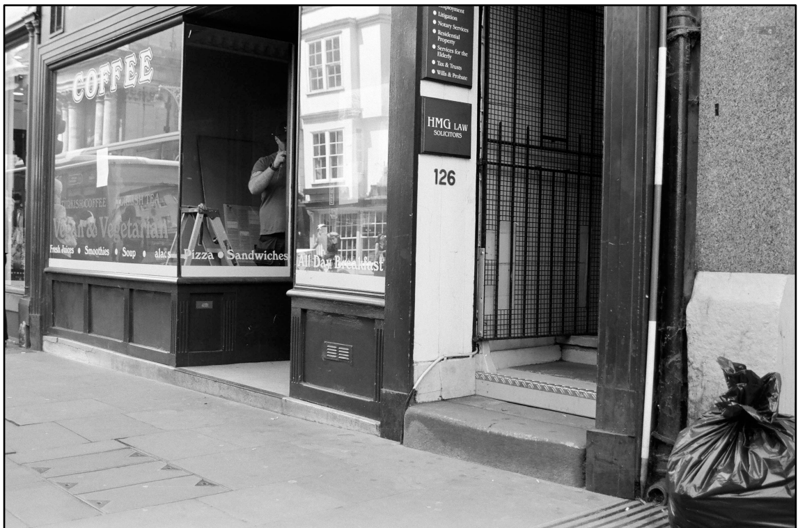
Appendix 2.3: Detail of shopfront, looking south-east (2m scale; Film 1.08)
