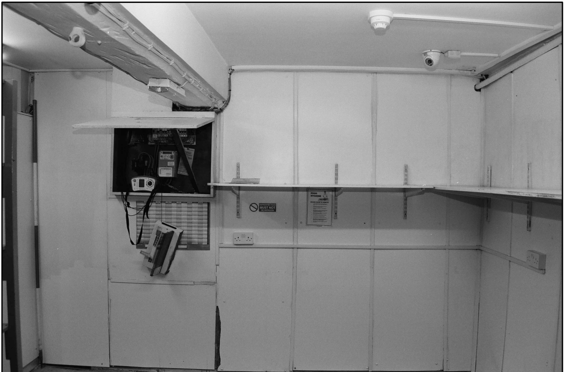
Appendix 2.9: General view of C1, looking north-west (1m scale; Film 1.23)
