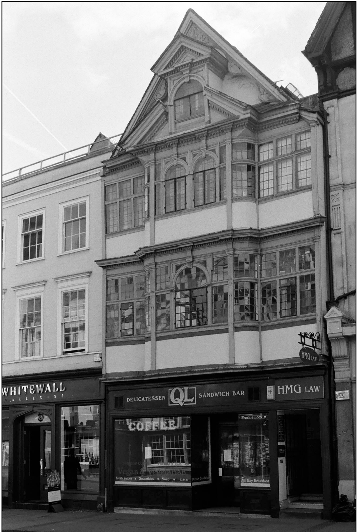
Appendix 2.1: General view of main façade, looking south (2m scale; Film 1.02)
