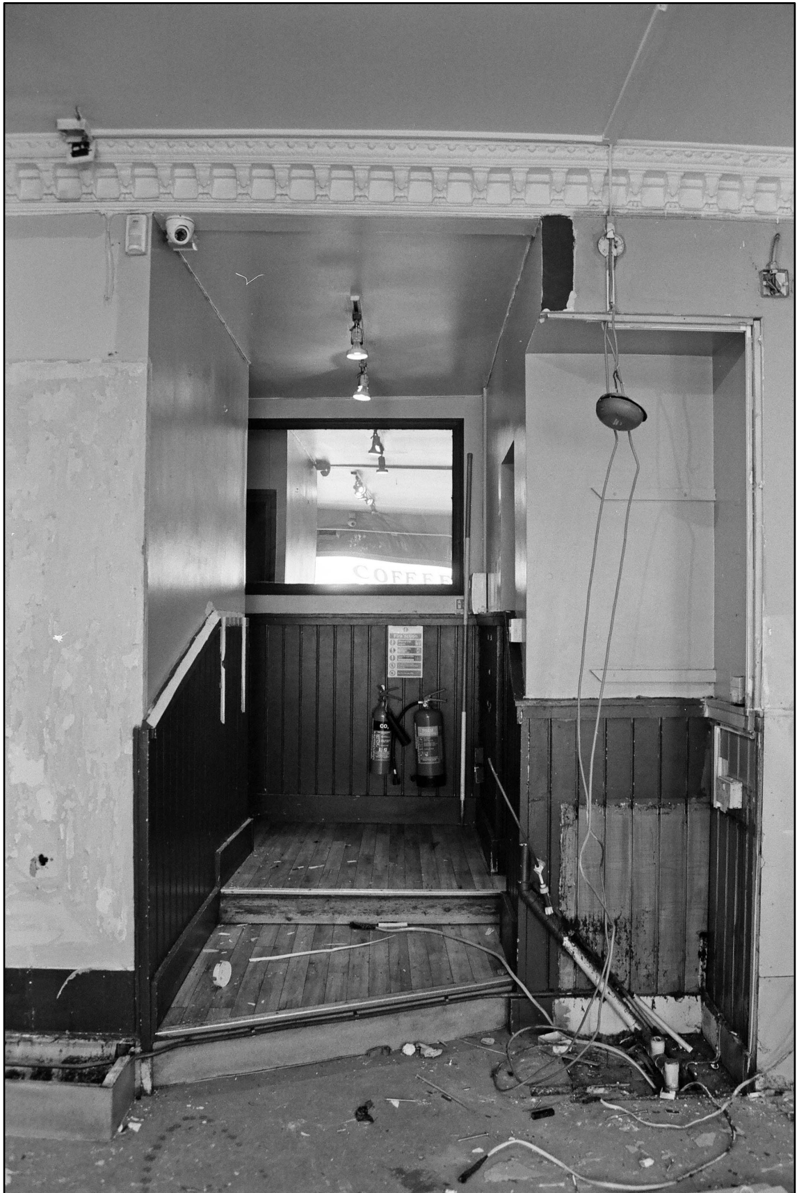
Appendix 2.6: Detail looking into G2, looking south (2m scale; Film 16)
