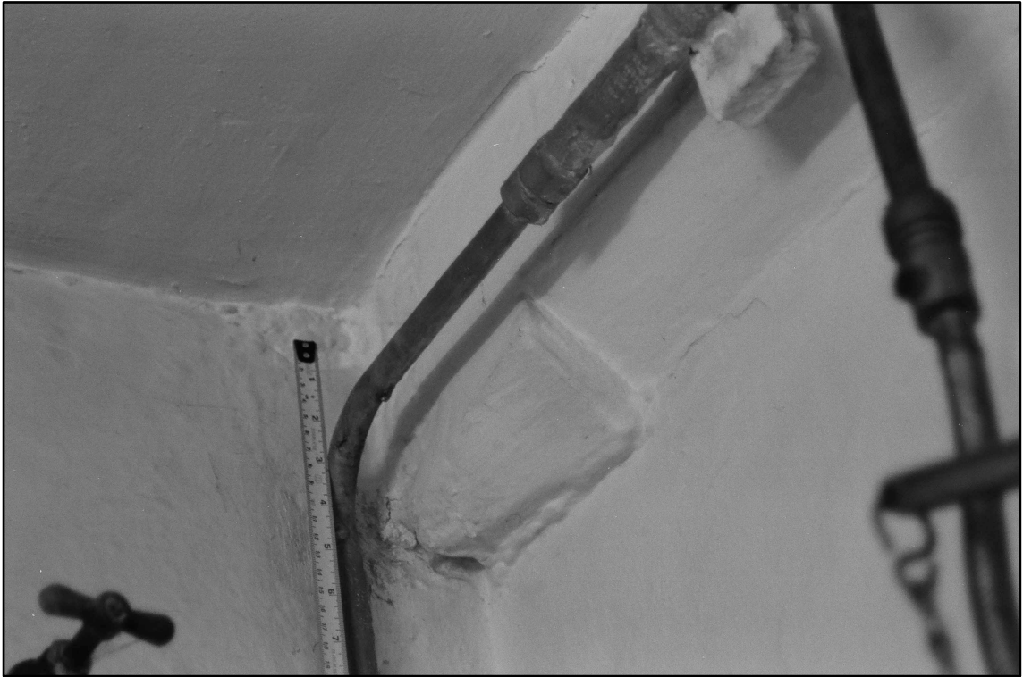
Appendix 2.13: Detail of beam stop in C4 , looking south-west (Film 1.31)
