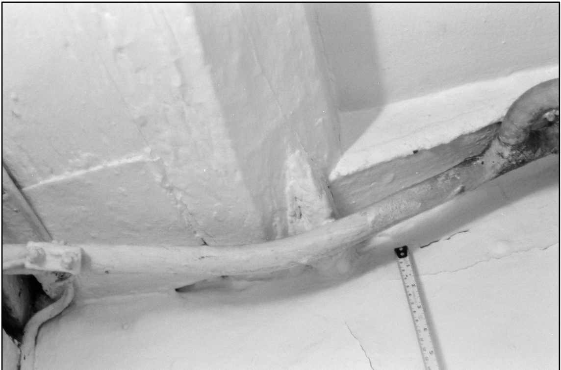
Appendix 2.14: Detail of beam stop in C4 , looking south-east (Film 1.32)
