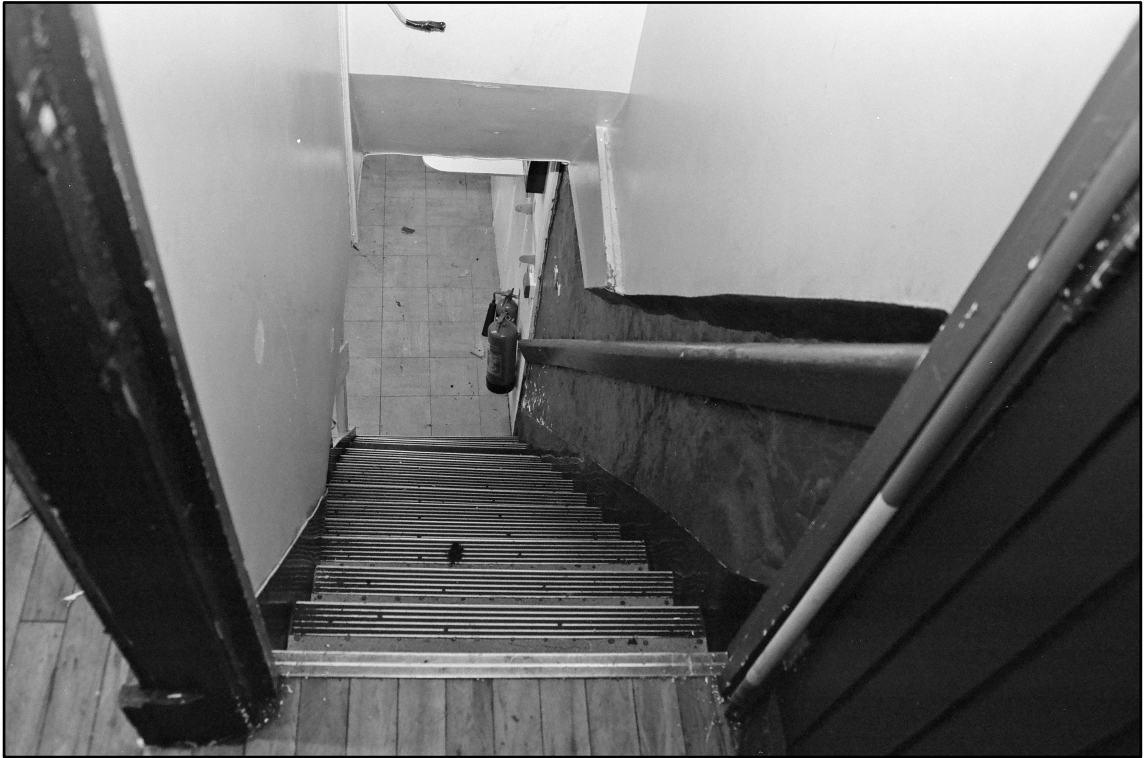
Appendix 2.8: General view looking down the stairs in G2 (1m scale; Film 1.20)
