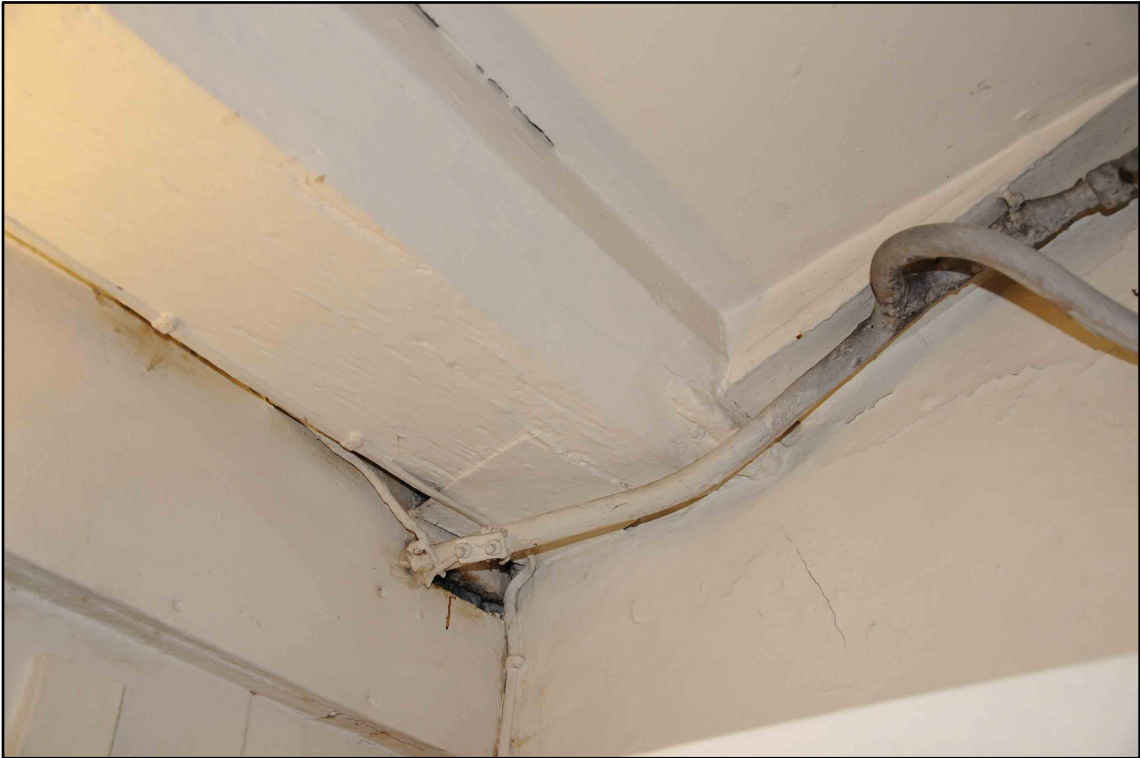
Appendix I.12: Detail of carved chamfer stop at south-east end of ceiling beam in room C4
