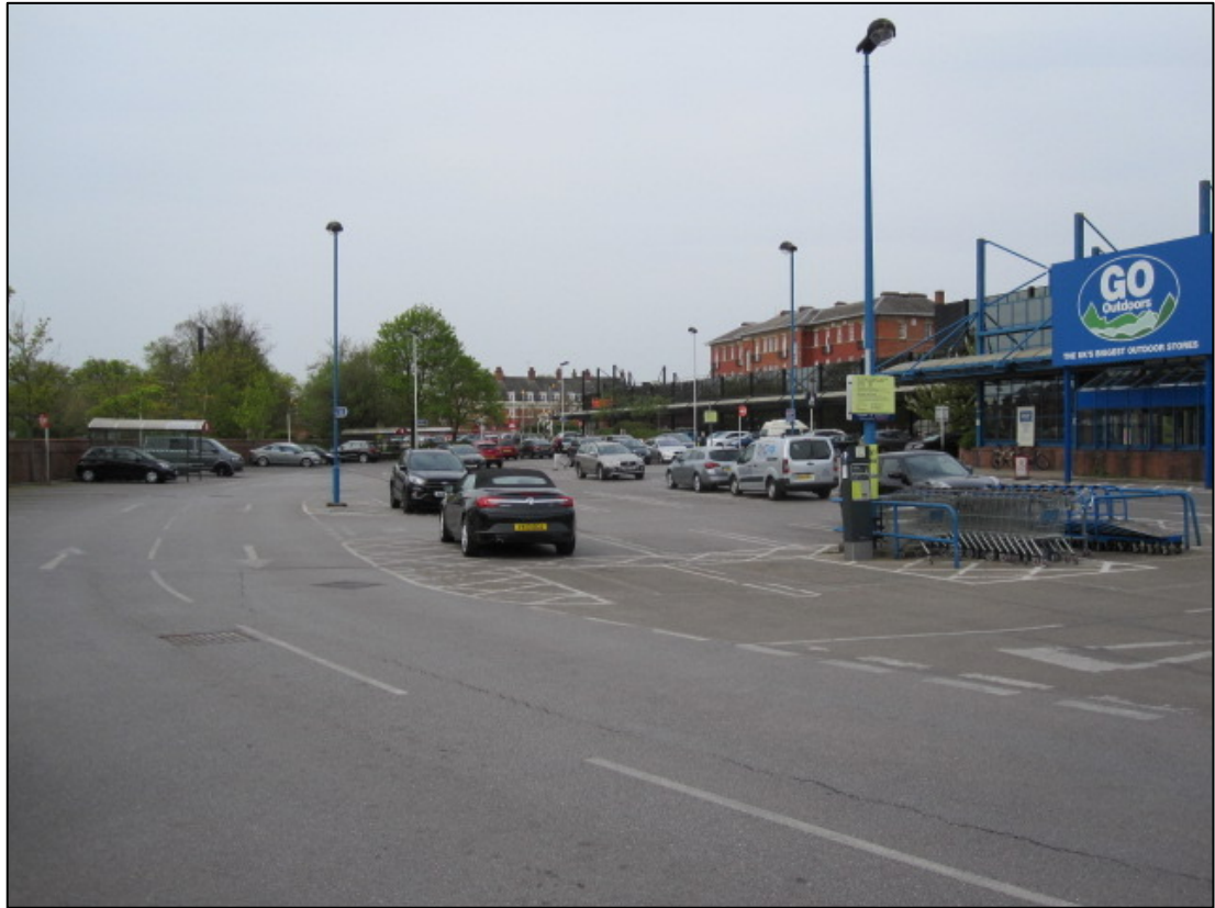
Appendix 2.1: View looking south-west across the car park within the site
