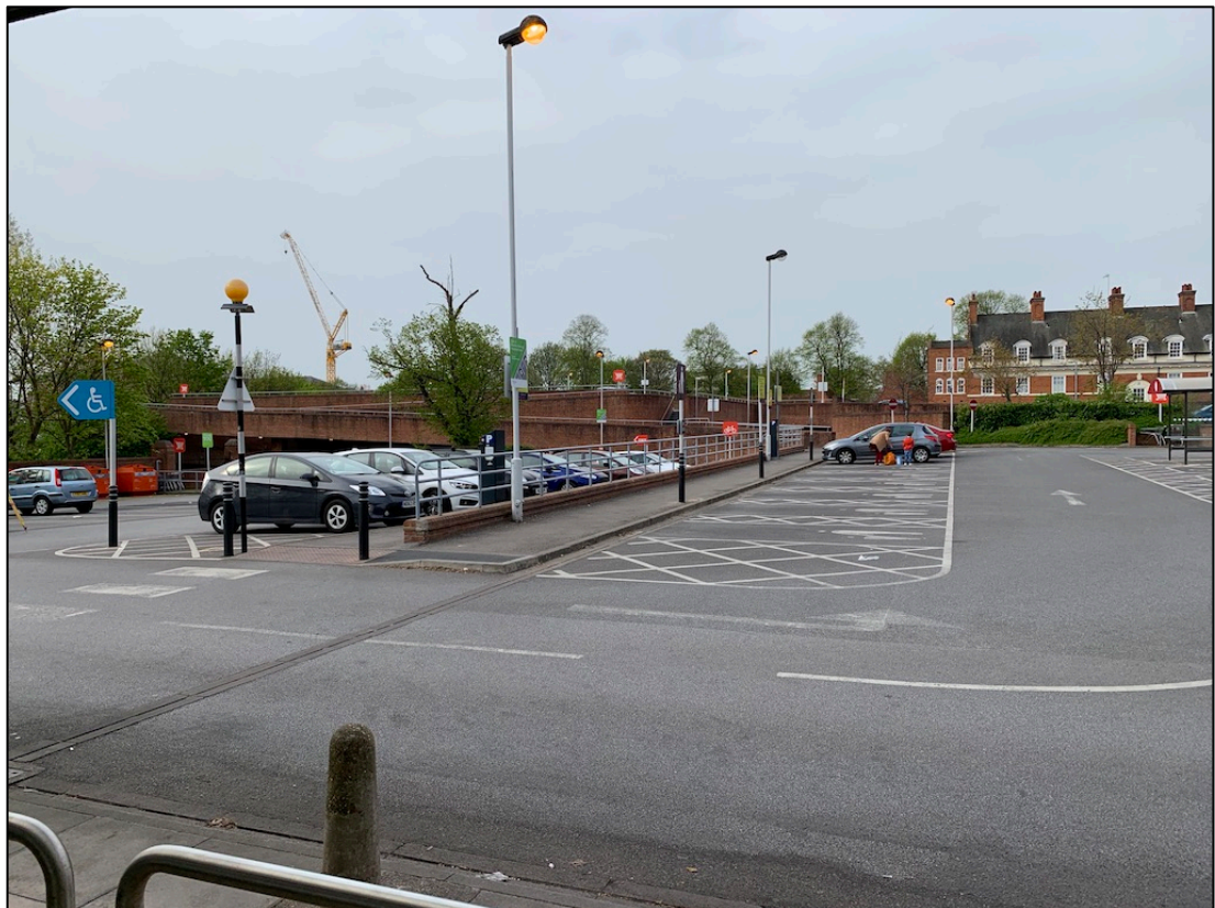
Appendix 2.2: View looking south across the multi-storey car park
