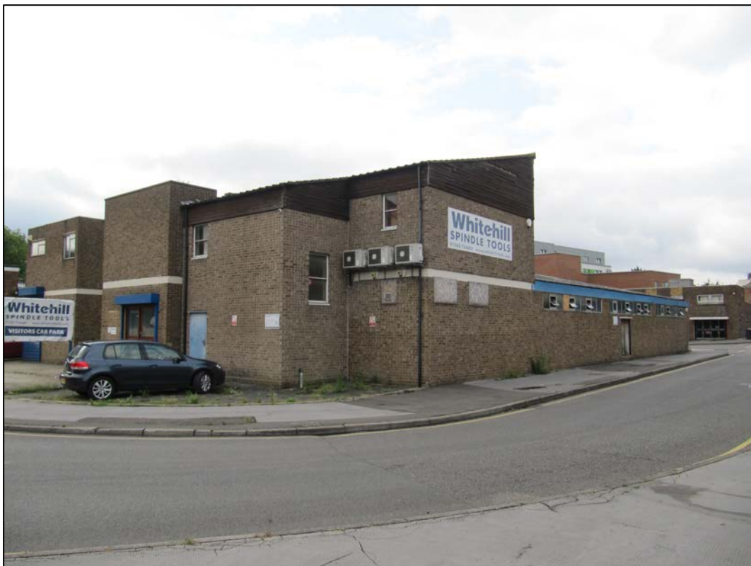
Appendix 2.2: General view of northeast and northwest elevations of Whitehill Spindle Tool Works from Bolton Road
