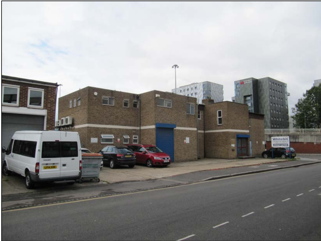
Appendix 2.1: General view of northeast elevation of Whitehill Spindle Tool Works from Bolton Road
