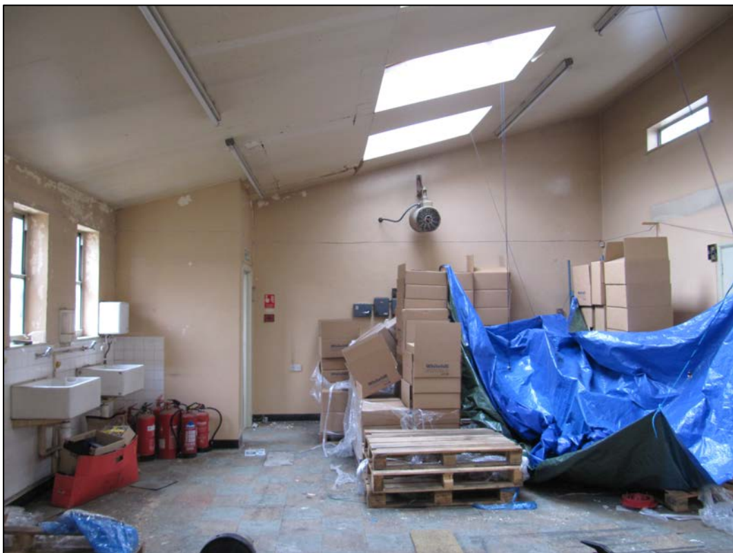
Appendix 2.8: General view of Whitehill Spindle Tool Works first floor interior
