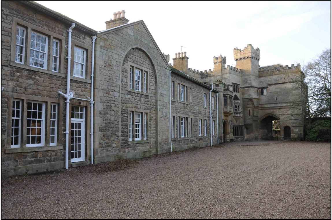
Appendix 2.1: General view of north elevation of the Library Flat and adjacent building
