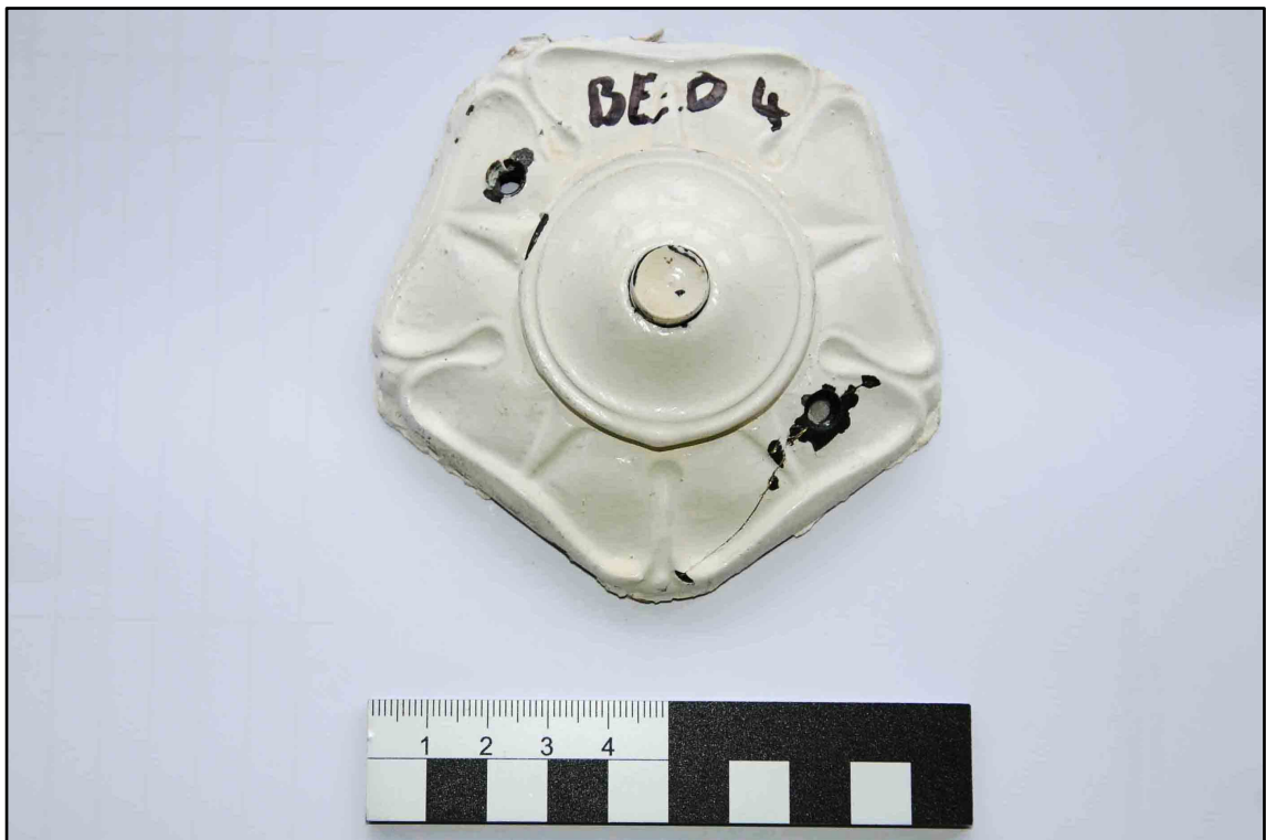
Appendix 2.8: Detail of push switch cover in west wall in Bedroom 4 (10cm scale; b/w Film I.15)
