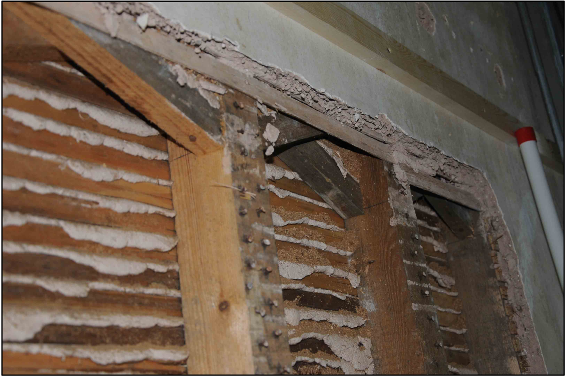
Appendix 2.17: Detail of timber noggin in Bedroom 4 following removal of laths (b/w Film 1.33)
