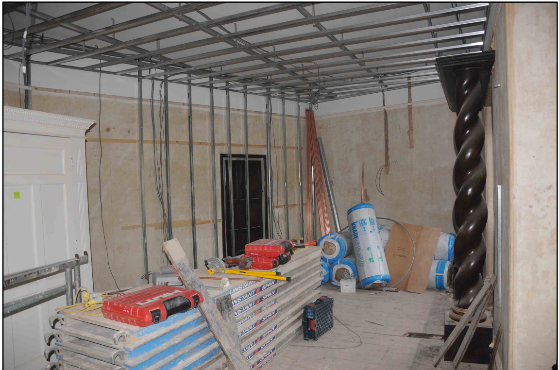
Appendix 2.3: General view of Bedroom 4 looking west (b/w Film 1.2)
