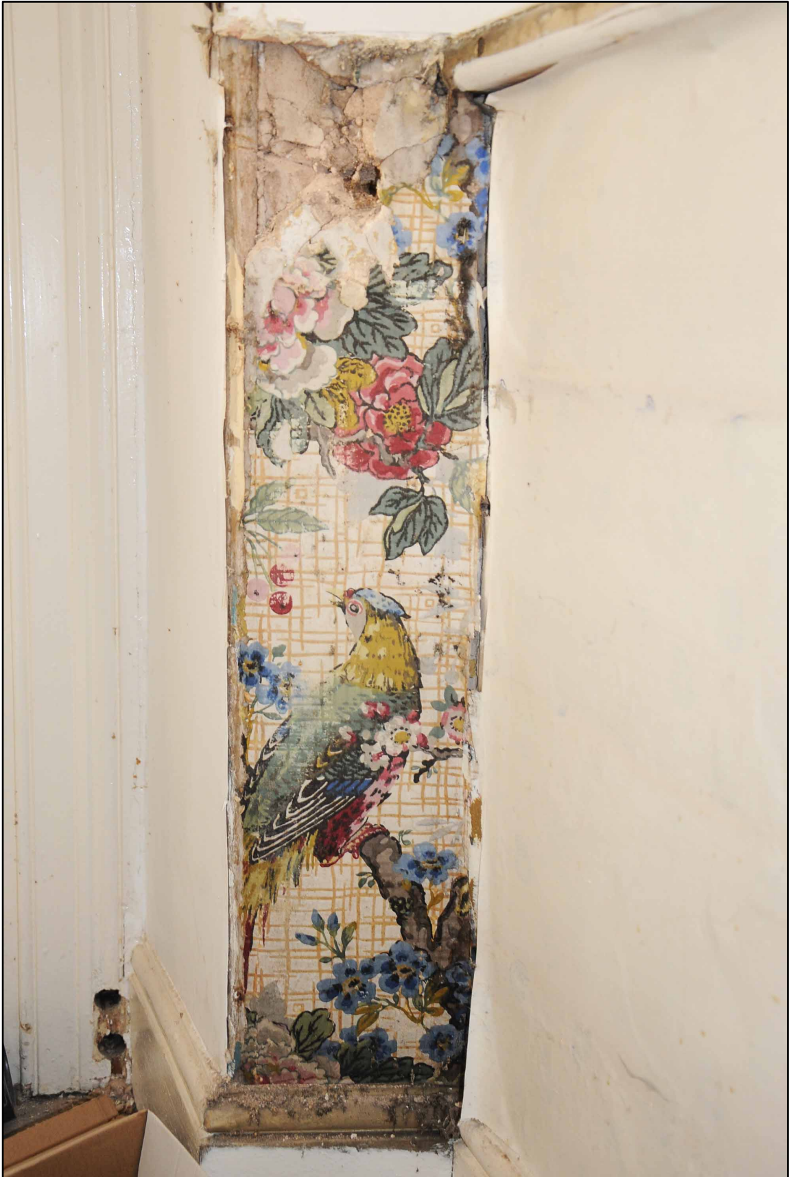
Appendix 2.23: Detail of wallpaper in window reveal in room to the north-west of the staircase
