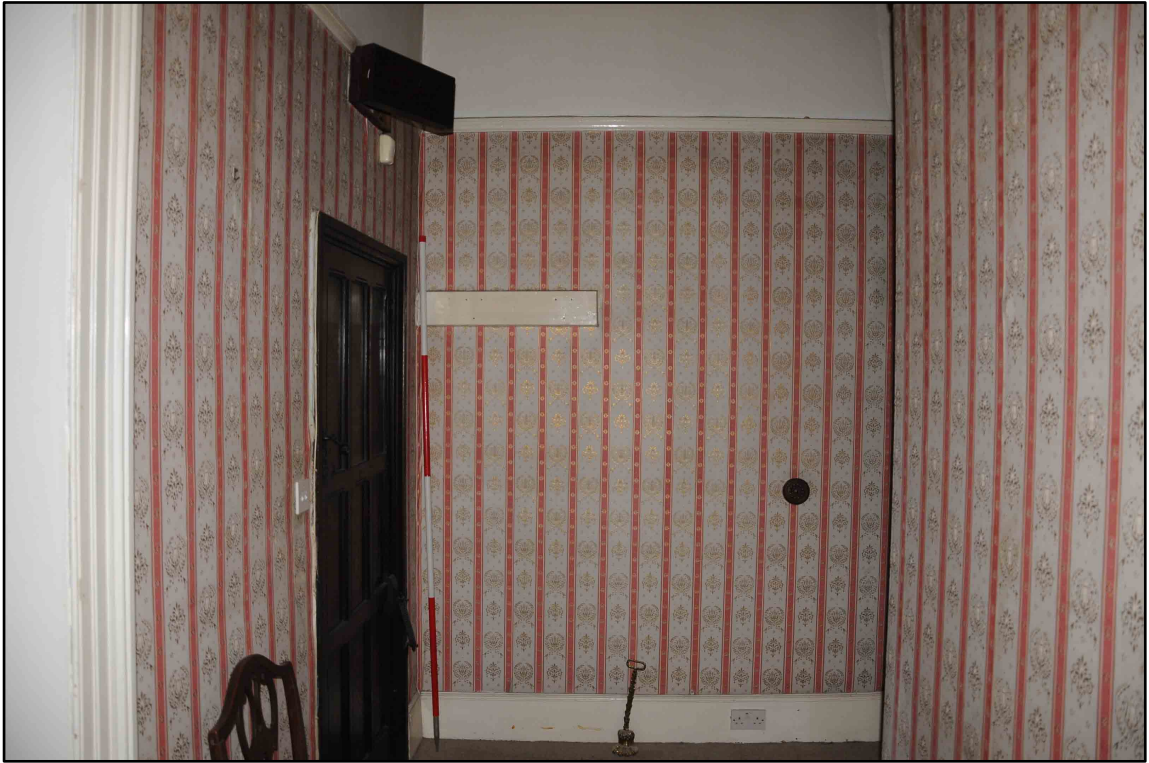
Appendix 2.19: View of position of new door in Corridor 2 (2m scale; b/w Film 1.16)
