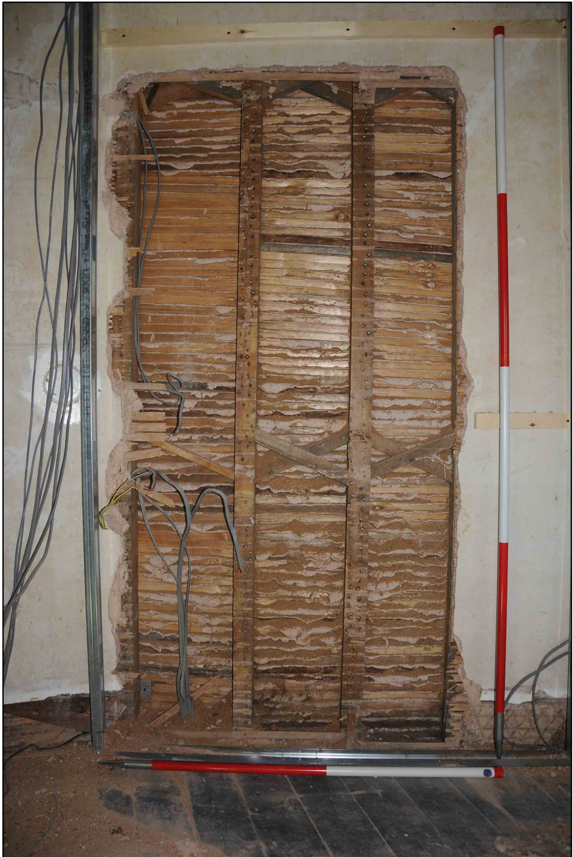
Appendix 2.16: West wall of Bedroom 4 following lath removal (1m/2m scale; b/w Film 1.30)
