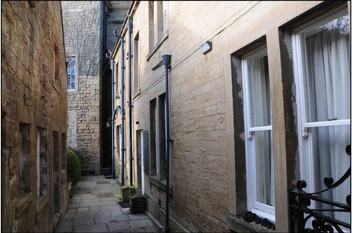
Appendix 2.2: General view of south elevation of the Library Flat, looking north-west
