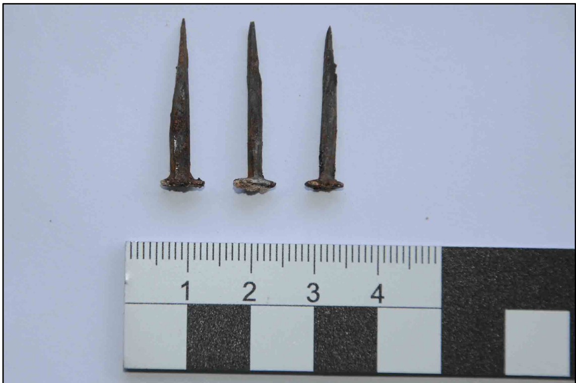
Appendix 2.11: Detail of nails used to secure laths for wall plaster (5cm scale)
