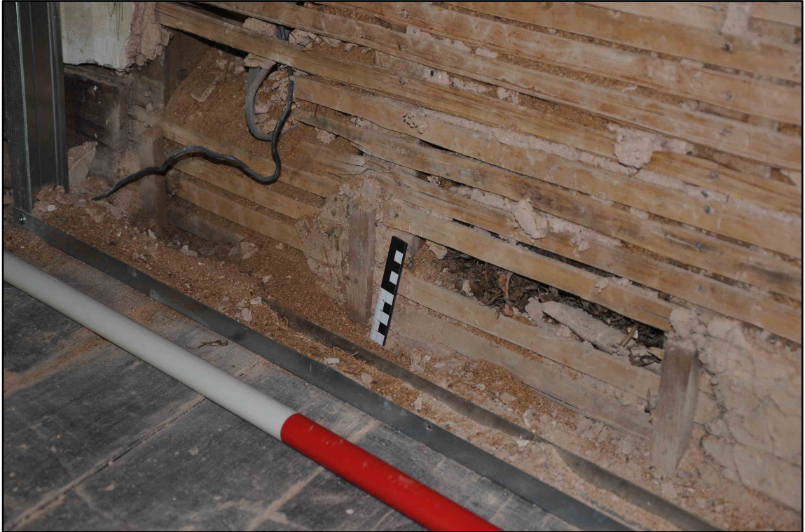
Appendix 2.13: Detail of batons to secure skirting in west wall (10cm scale; b/w Film 1.26)
