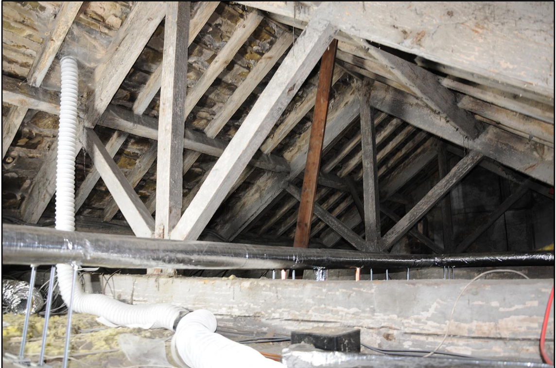
Appendix 2.22: Detail of roof structure above Hall Cottages , looking south-east
