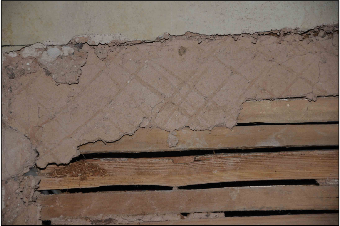
Appendix 2.12: Detail of scratch coat plaster in west wall of Bedroom 4 (b/w Film 1.23)
