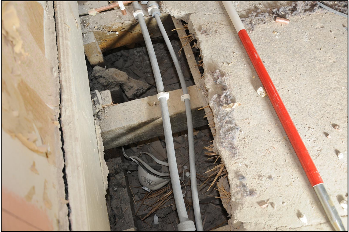
Appendix 2.21: Lime-ash floor in adjacent room to the south-east of Bedroom 4 (0.5m scale)
