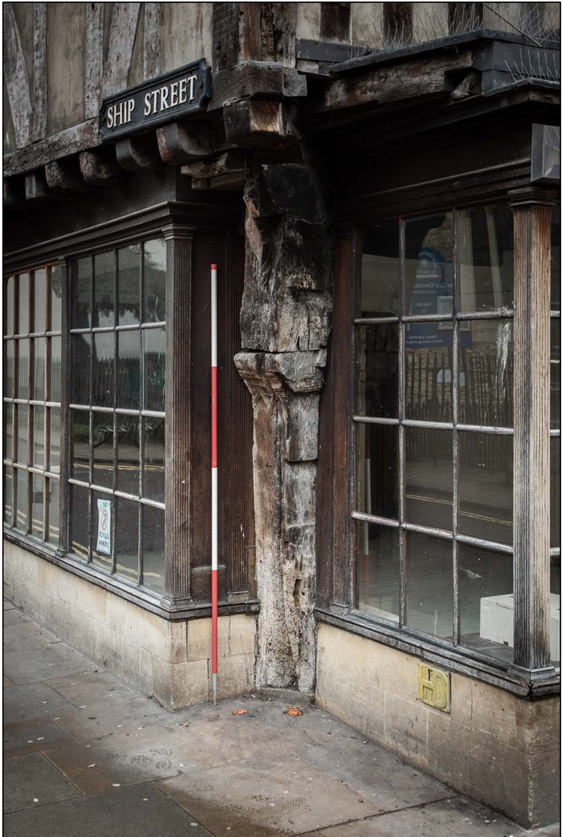
Appendix 3.9: Detail of carved corner post, looking east (2m scale; b/w *Film I.14)
