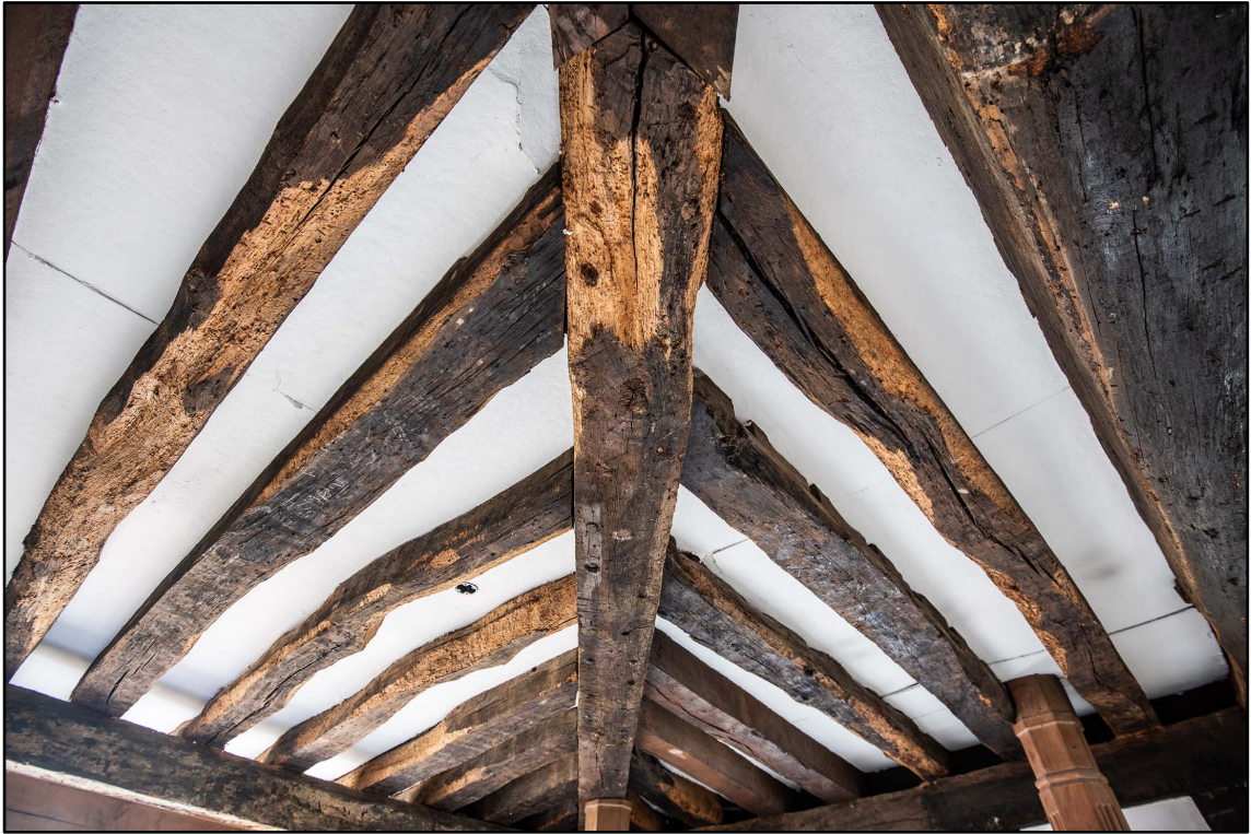
Appendix 3.25: Detail of ceiling beams in F1, looking north-west (b/w *Film 4.10)
