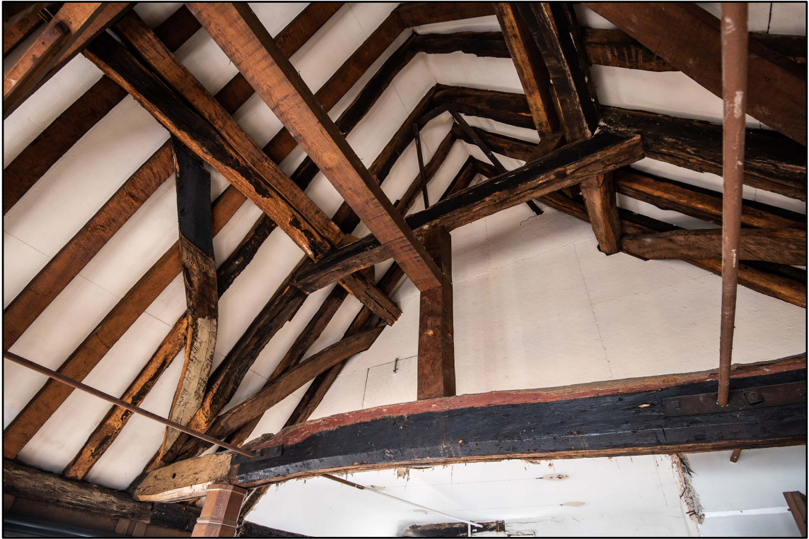
Appendix 3.30: Detail of replaced kingpost in SI, looking east (b/w *Film 5.11)
