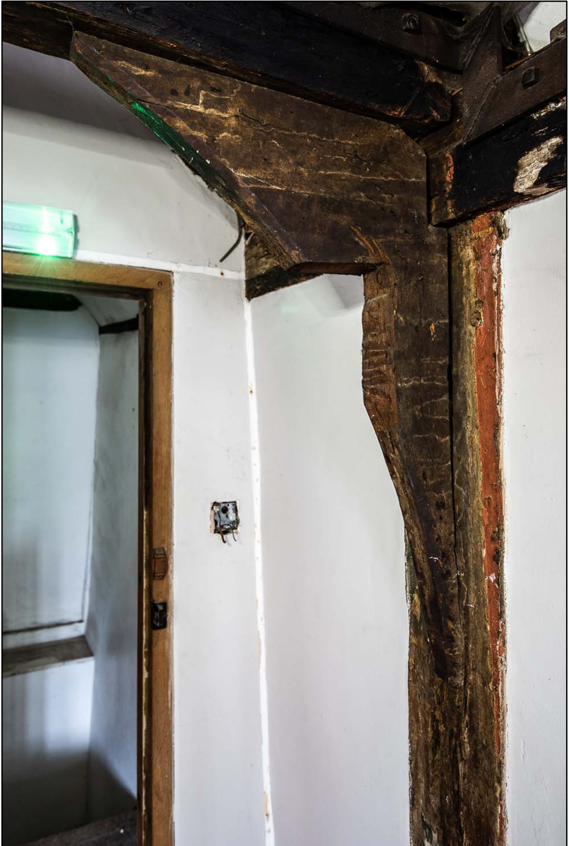
Appendix 3.34: Detail of jowl post with cut for a secondary doorway in S1; note lambs tongue stops on tie-beam (b/w *Film 5.15)
