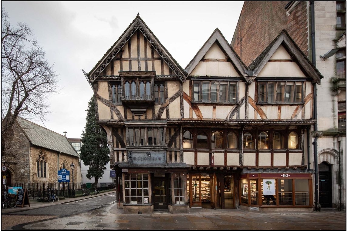
Appendix 3.1: General view of the Cornmarket elevation of No.s. 26-28 (2m scale)
