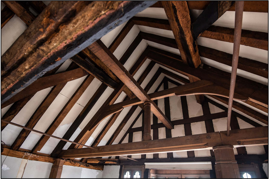
Appendix 3.35: General view of roof in SI, looking west; note replaced timbers (b/w *Film 5.9)
