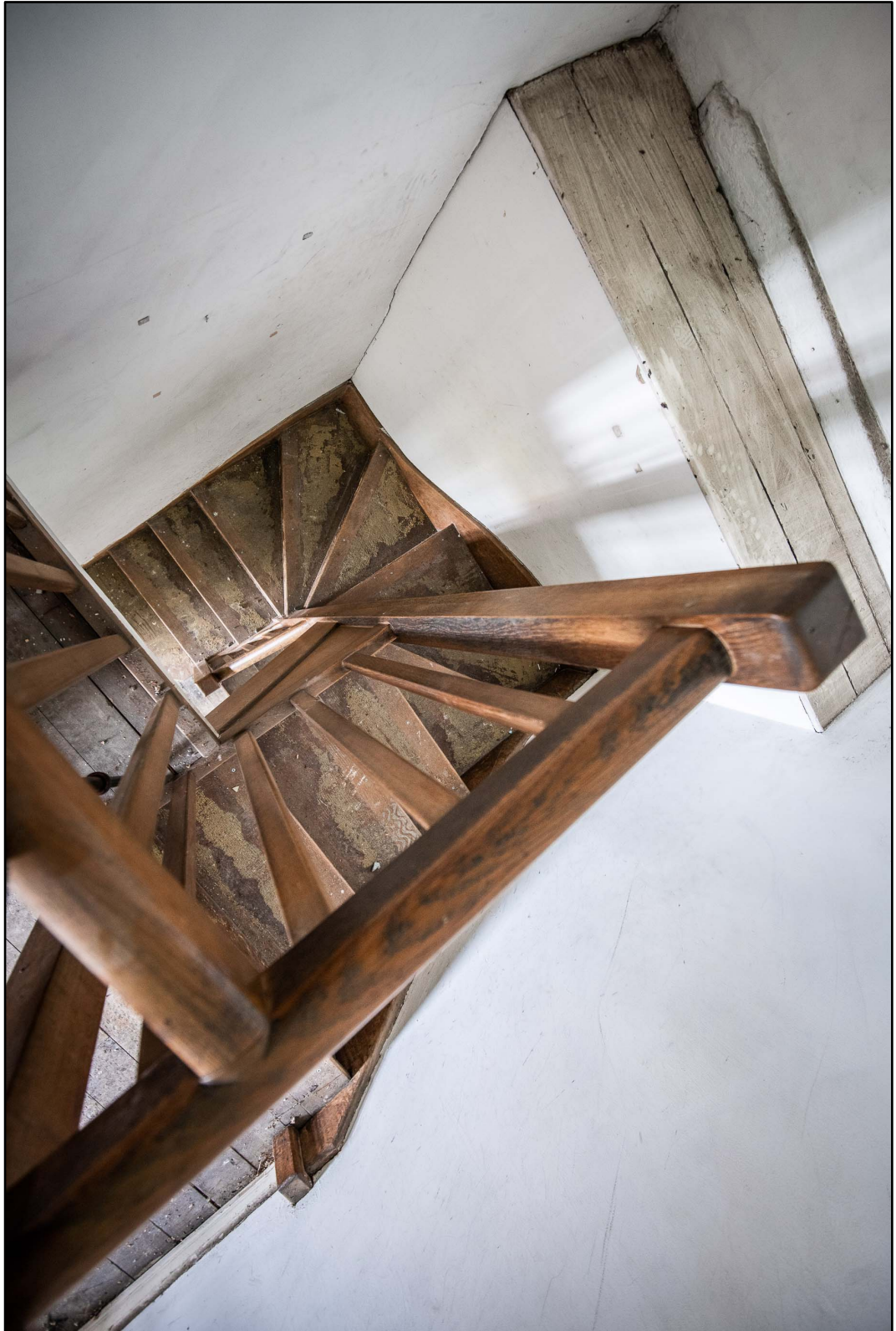
Appendix 3.28: General view looking down staircase in S2 (b/w *Film 4.14)
