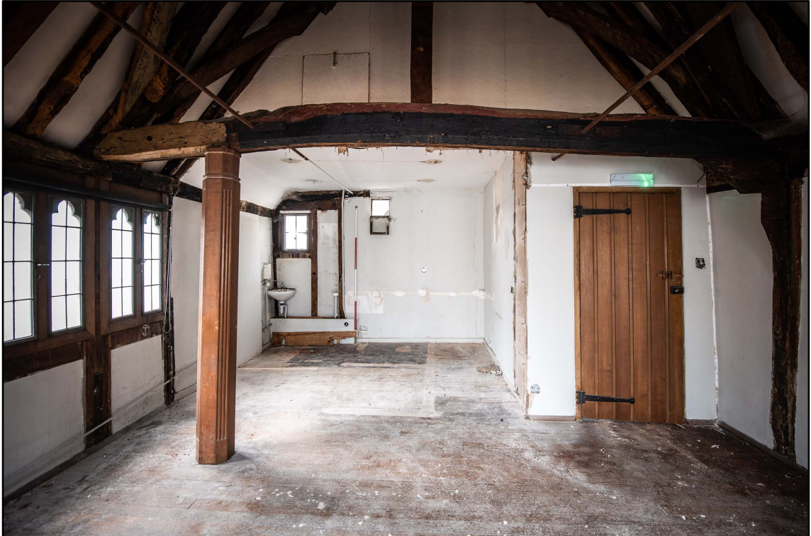
Appendix 3.31: General view of SI, looking east; note 1951 column (2m scale; b/w *Film 5.3)
