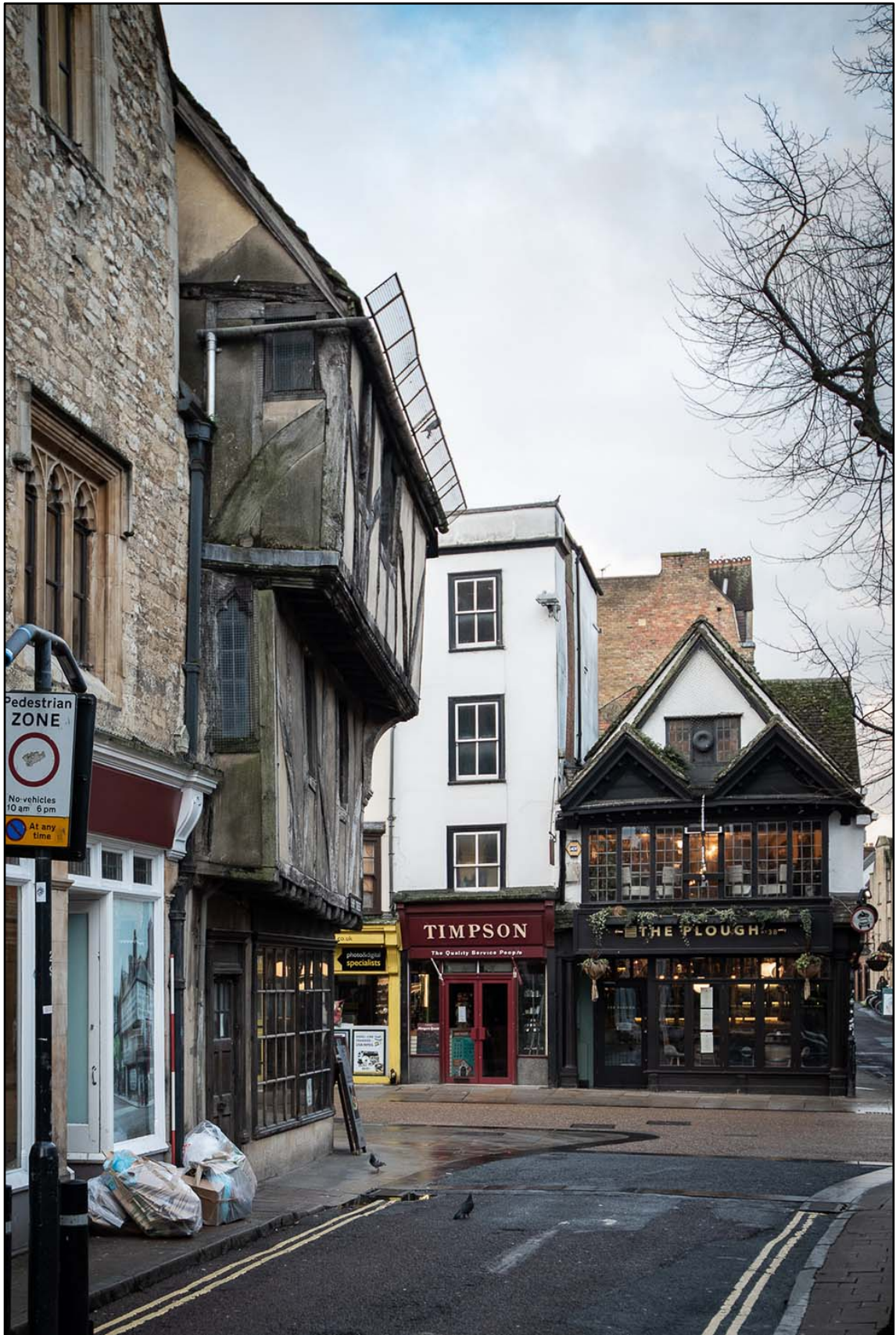
Appendix 3.8: General view looking west along Ship Street (2m scale; b/w *Film 1.2)
