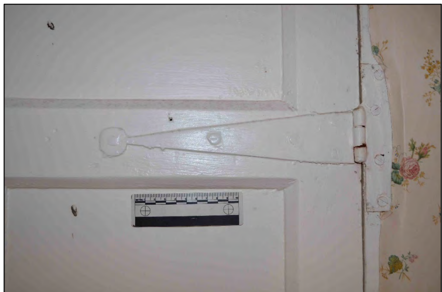
Appendix 2.27: Detail of hinge to door in F2
