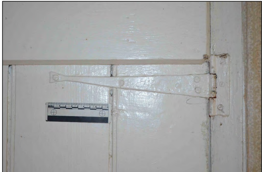
Appendix 2.26: Detail of hinge to door in B1F5
