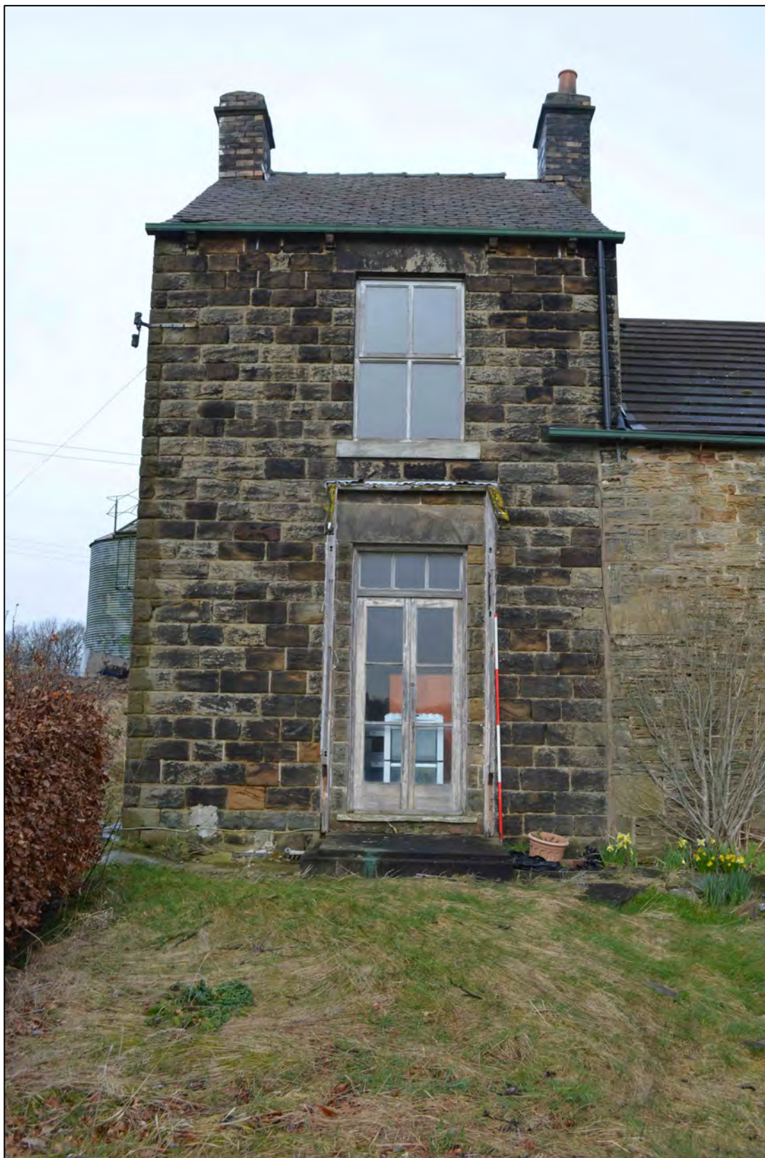
Appendix 2.28: View of Building 2, looking north
