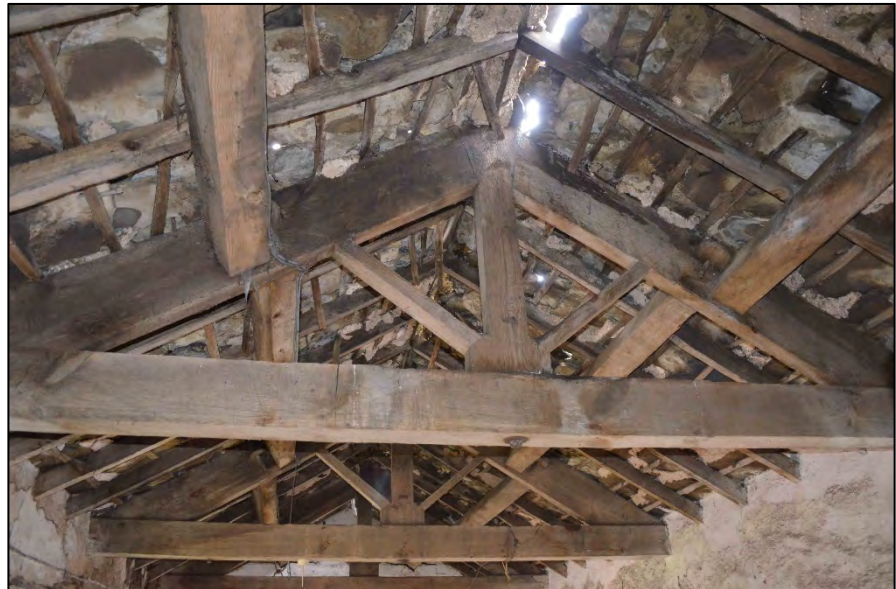
Appendix 2.52: Detail of truss in B3F1, looking south
