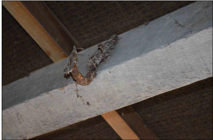
Appendix 2.53: Detail of hook on north purlin above B2F2
