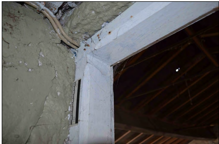
Appendix 2.52: Detail of chamfered timber doorcase between rooms B2F1 and B2F2, looking north-east
