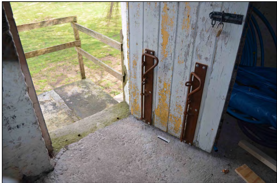
Appendix 2.48: Detail of vertical draw bolts to door in B2F1
