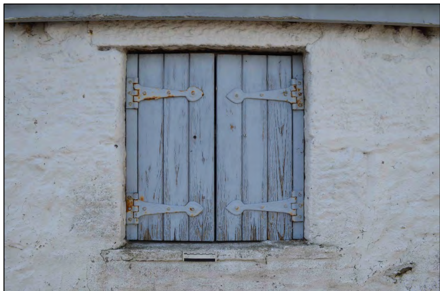
Appendix 2.16: Detail of external shutter to northern window in east elevation of Building 1
