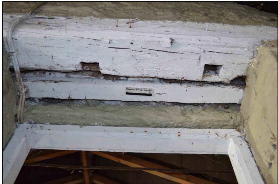
Appendix 2.51: Detail of soffit of reused timber lintel between rooms B2F1 and B2F2
