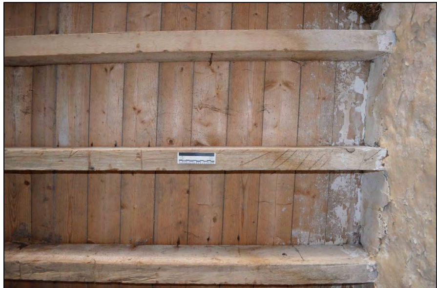
Appendix 2.45: Detail of Baltic timber mark on floor joist above B2G2
