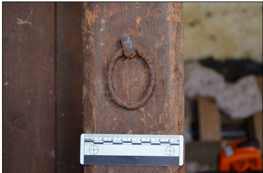
Appendix 2.40: Detail of tethering ring on north side of the western post of the stall in B2G1
