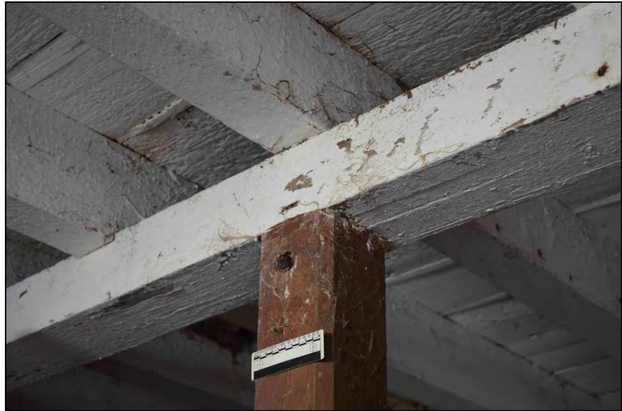
Appendix 2.38: Detail of junction between post and soffit of stall and floor joists above in B2G1
