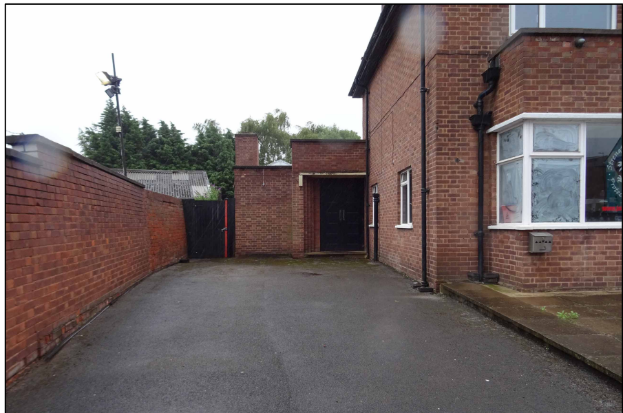
Appendix 2.2: Detail of building looking south-east showing north-east elevation.
