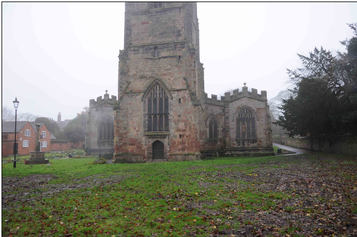
Appendix 2.24: General view of St Helens Church
