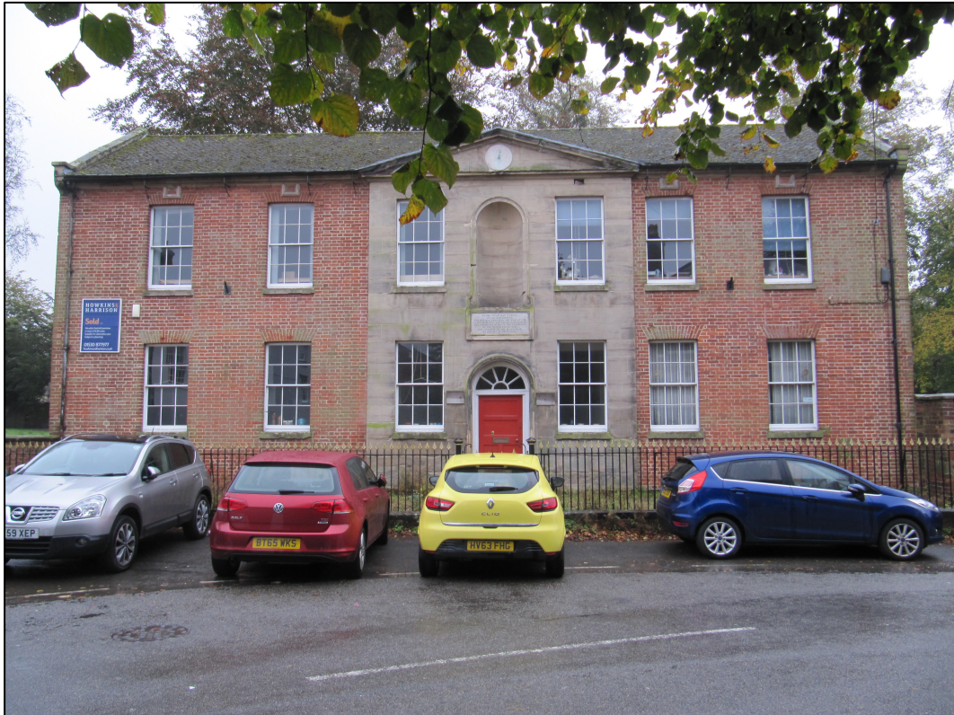
Appendix 2.1: General view of north elevation of the former Ashby Grammar School
