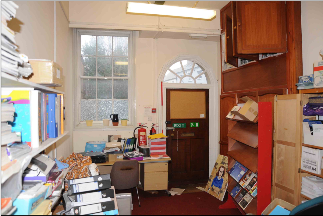
Appendix 2.17: General view of G8 looking north; note former entrance door (2m scale)
