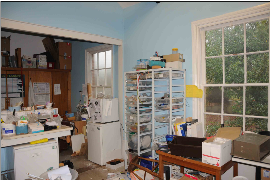
Appendix 2.22: General view of F2 looking south-east; note hung-sash windows (2m scale)
