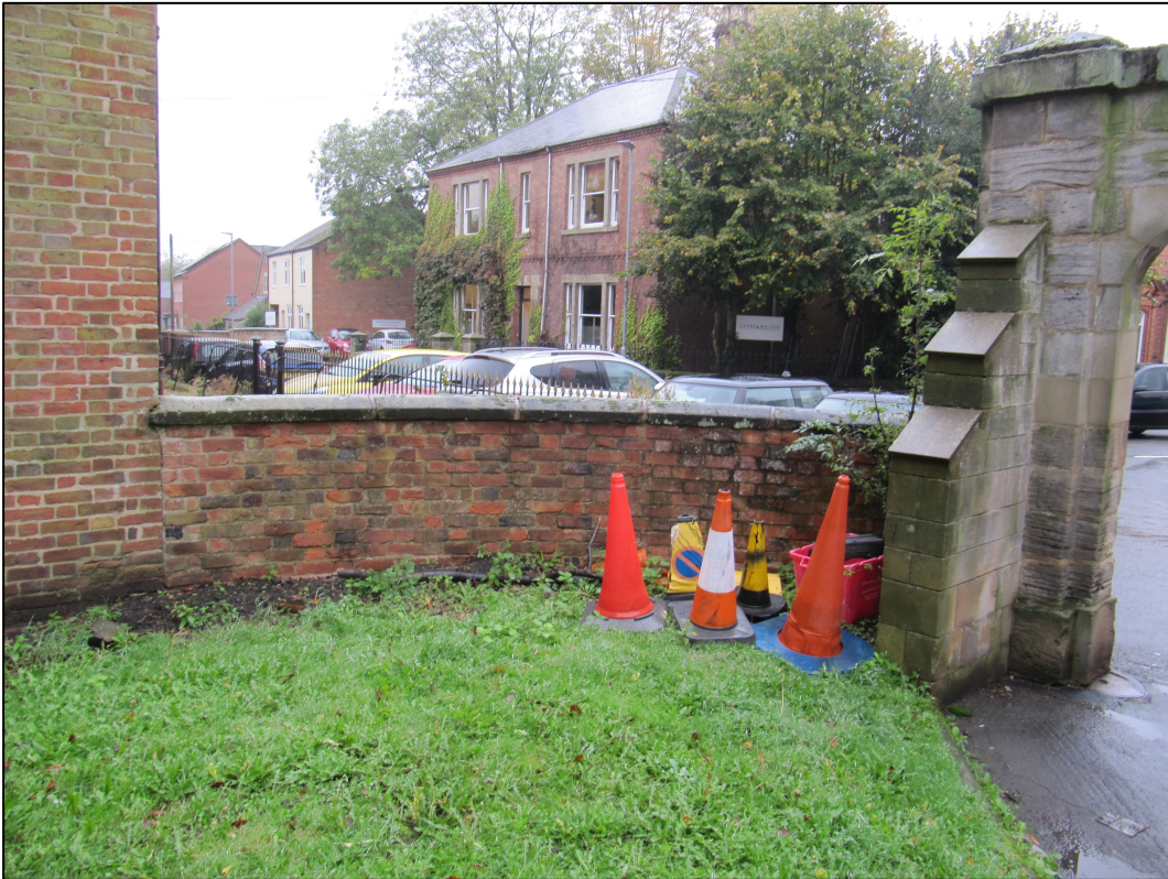
Appendix 2.9: Curvilinear wall forming boundary between churchyard and former school
