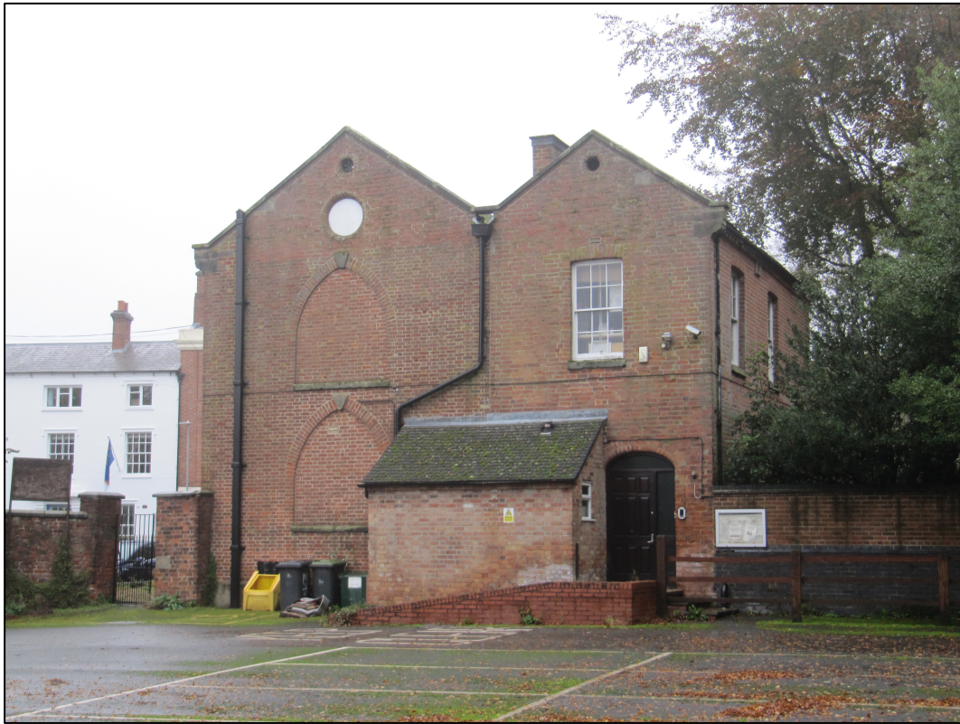
Appendix 2.7: General view of the west elevation of the former school
