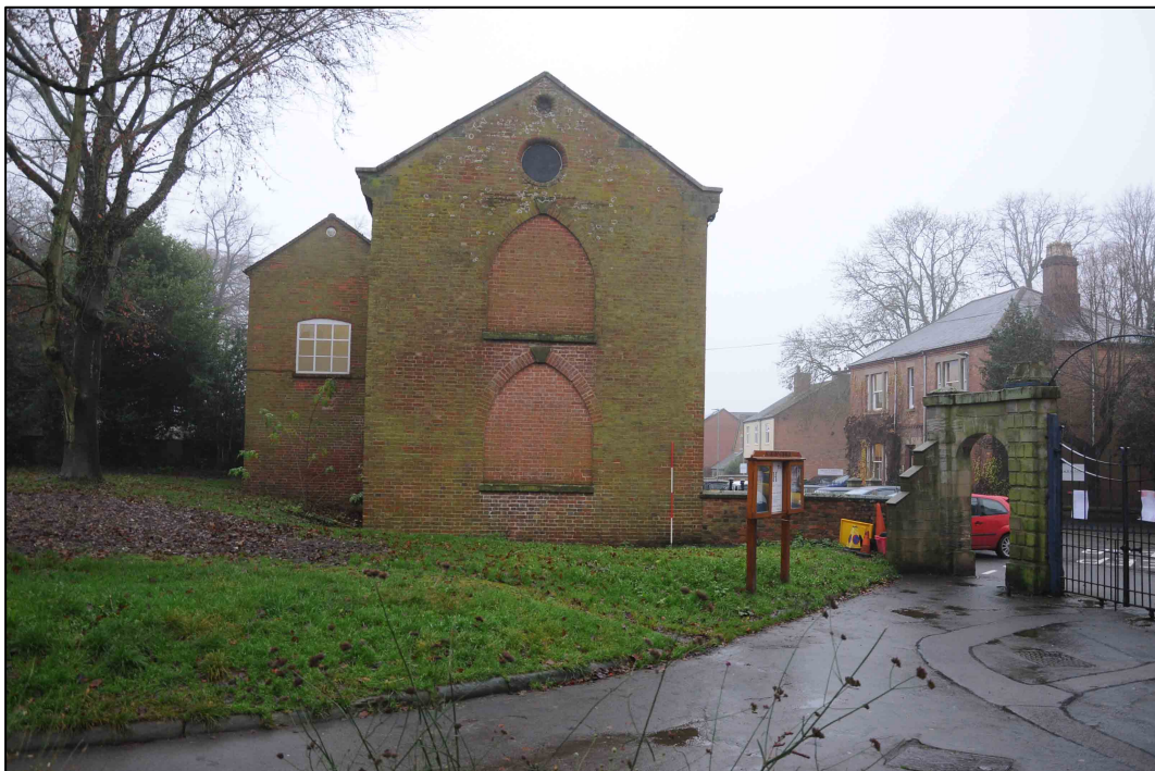
Appendix 2.4: General view of the east elevation of the former school
