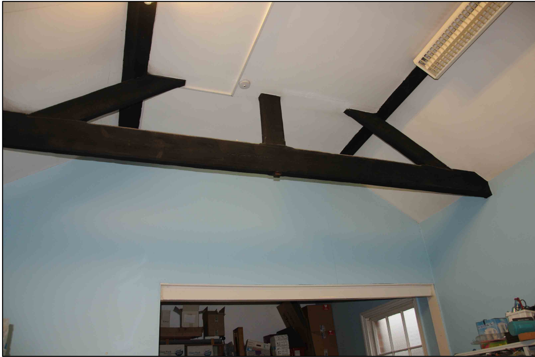
Appendix 2.23: Detail of exposed kingpost truss in F2 looking east
