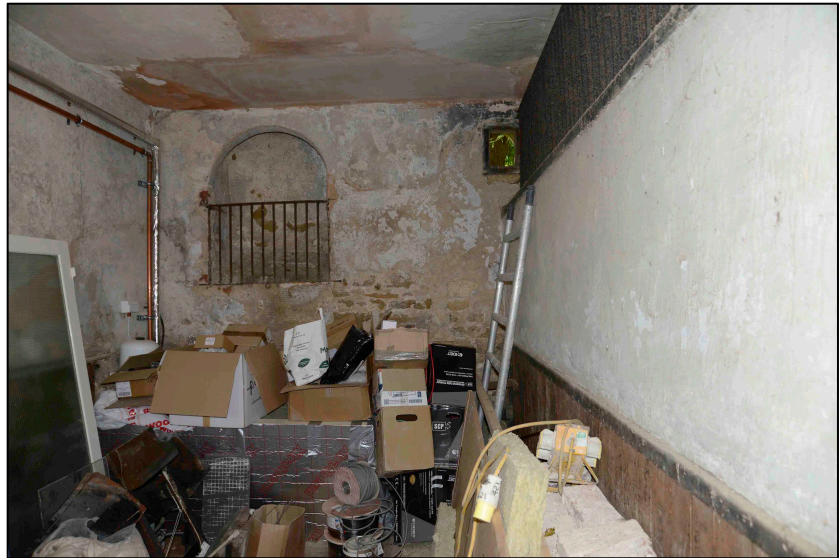
Appendix 2.20: General view of GI looking west
