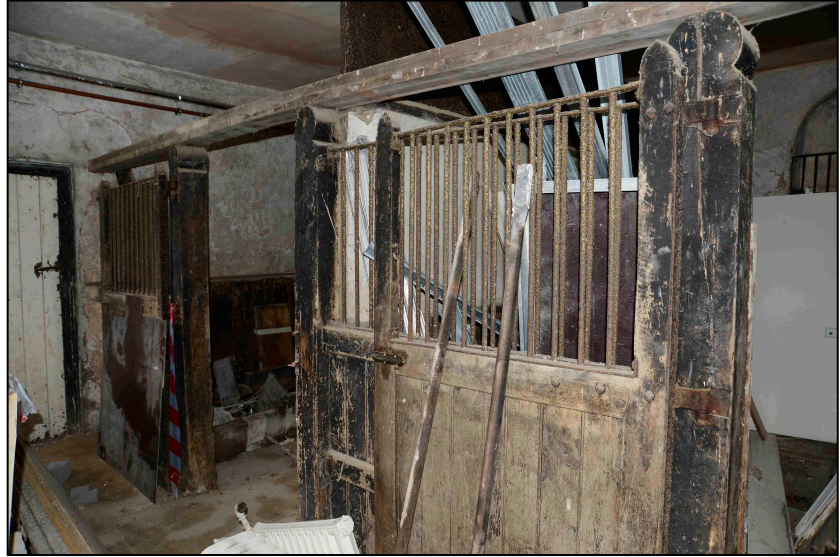
Appendix 2.19: Detail of stall partitions in GI looking south-west
