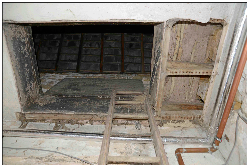
Appendix 2.21: Detail of loft hatch in GI
