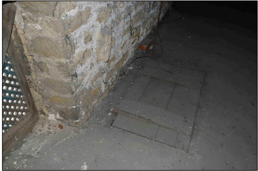
Appendix 2.28: Detail of floor hatch in FI
