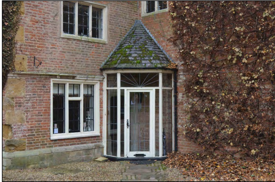
Appendix 2.8: View of porch to west entrance
