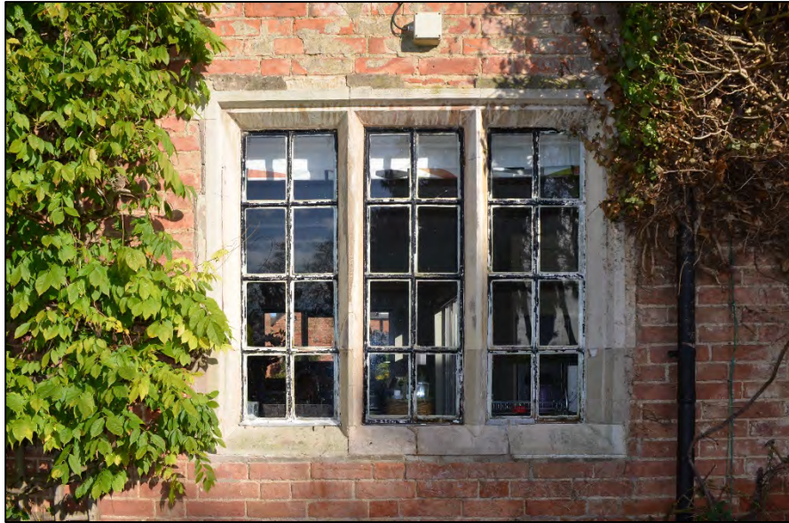
Appendix 2.5: Detail of window into Room G4
