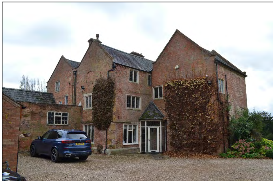
Appendix 2.2: View of north elevations of the Hall
