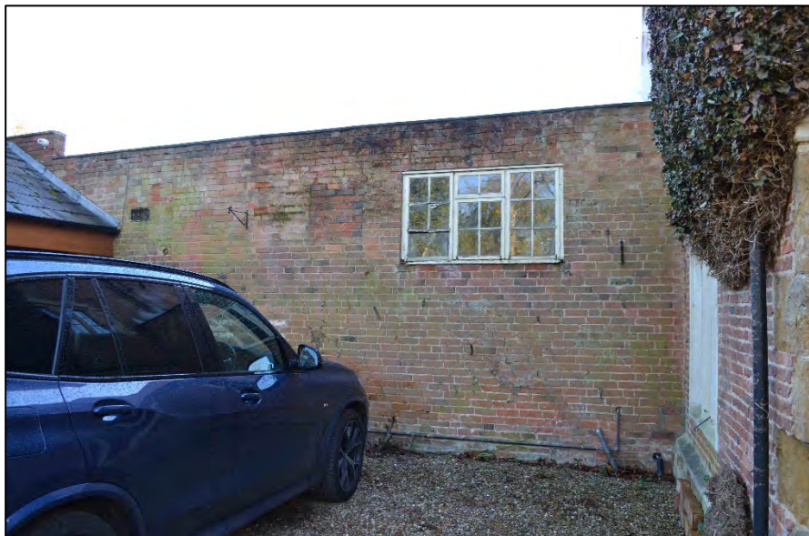
Appendix 2.27: View of the west elevation of the Outbuildings
