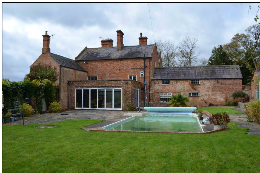
Appendix 2.3: View of the east elevations of the Hall
