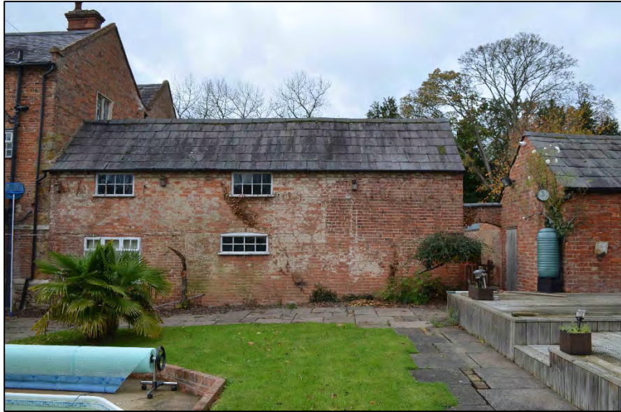
Appendix 2.26: View of east elevation of the Outbuildings
