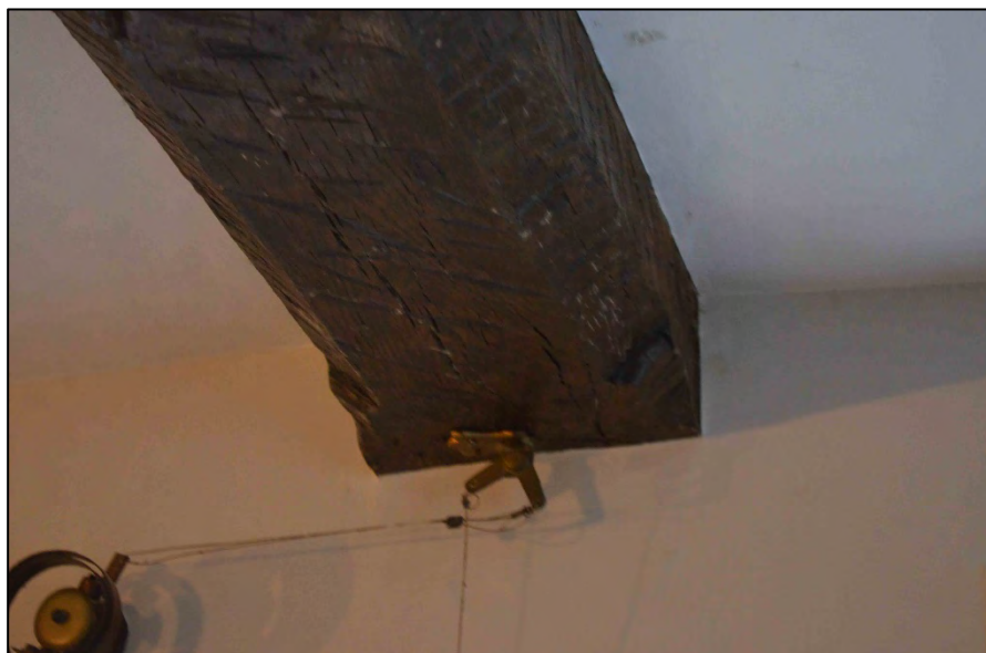
Appendix 2.13: Detail of chamfered stop to beam in Room G1
