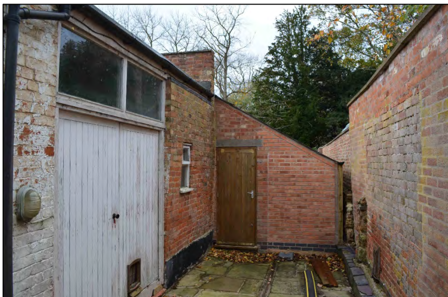
Appendix 2.28: View of the north elevation of the Outbuildings, lookgin west
