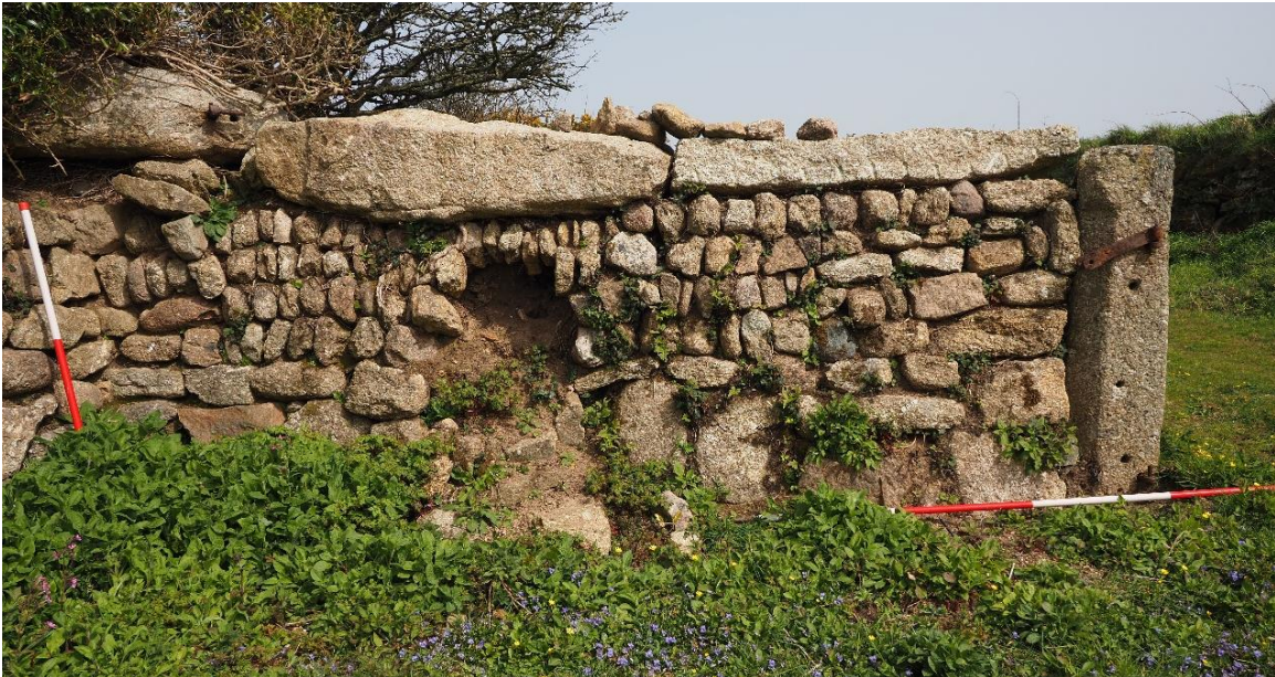
Figure 60: Cornish hedge north of barn, incorporating reused C17 probable fireplace lintel
