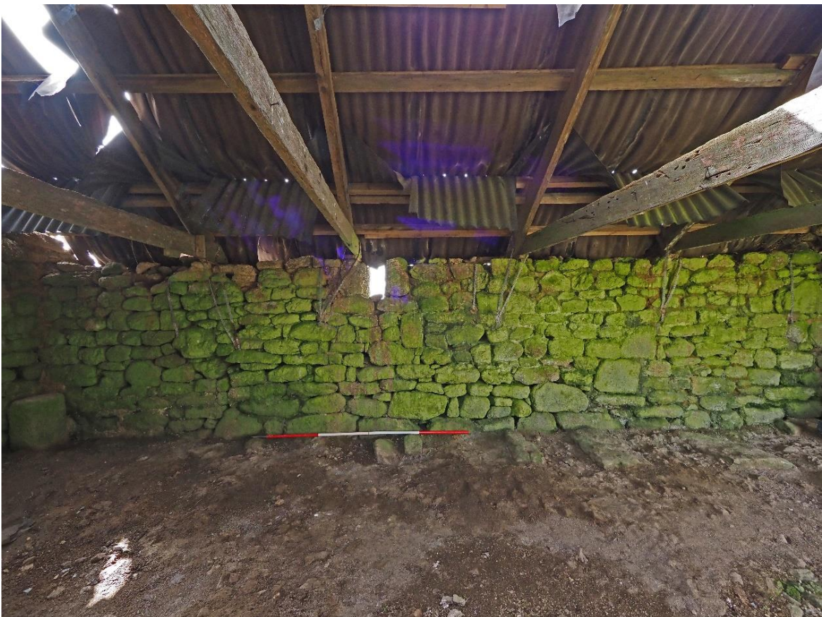
Figure 45: Cartshed SW wall
