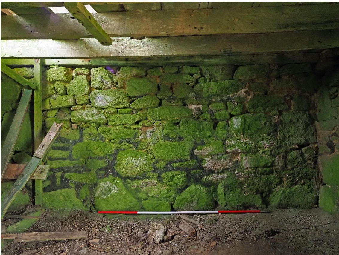
Figure 33: Barn ground floor south end
