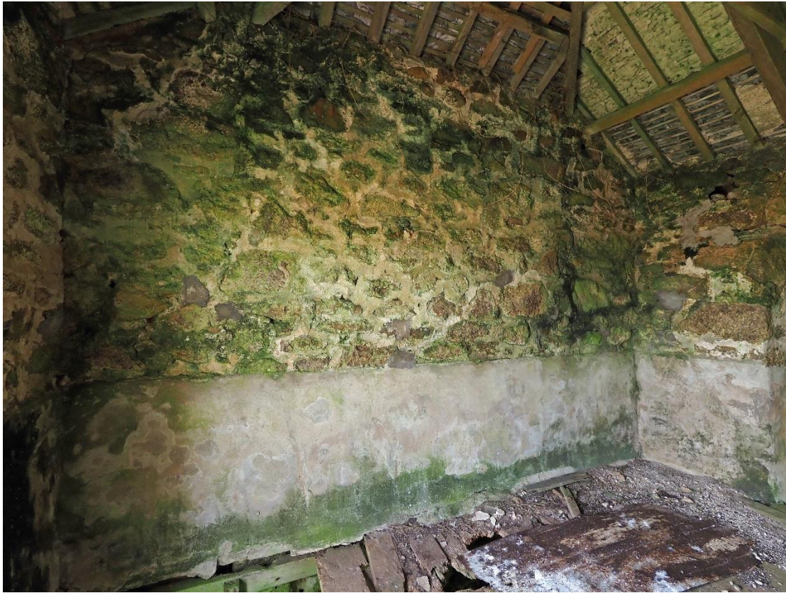
Figure 38: Barn loft south wall from NE
