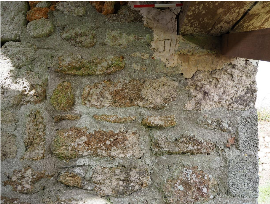
Figure 51: Cartshed: rebuilt masonry to NW side of doorway inscribed: SJH 8:5:1986
