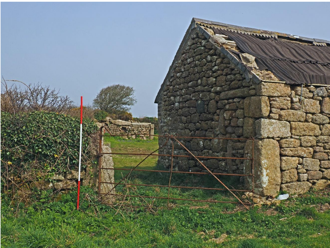
Figure 65: Gateway adjoining Cartshed including rare C19 wrought-iron field gate
