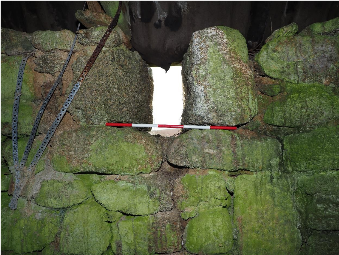
Figure 56: Cartshed: vent central to SW wall
