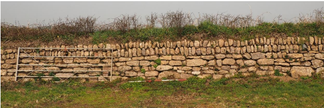
Figure 59: Cornish hedge to north side of farmyard built replacing rear wall of former farmhouse
