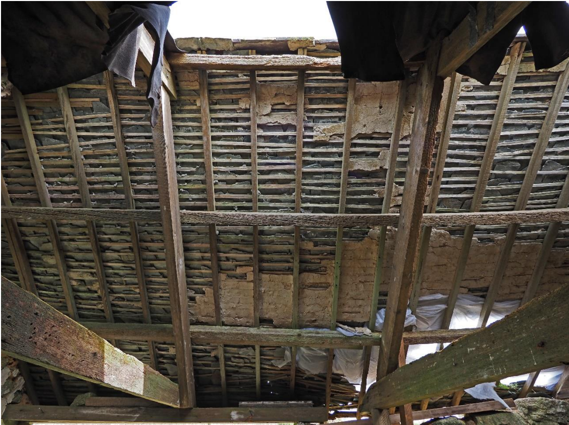
Figure 50: Cartshed roof (NE side)
