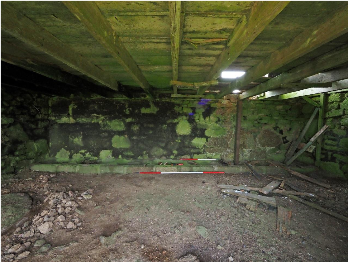
Figure 32: Barn ground floor east wall
