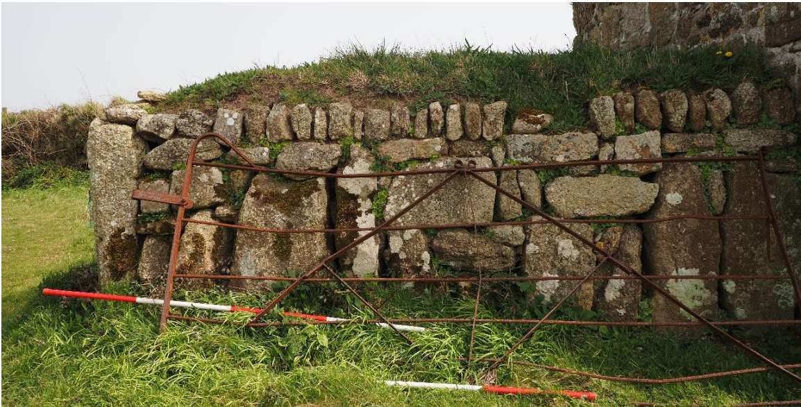
Figure 61: Cornish hedge adjoining north side of barn with reused probable jamb-stone (left), plus C19 wrought-iron field gate
