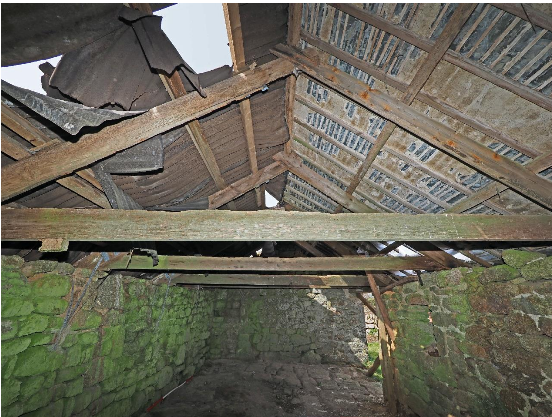
Figure 49: Cartshed roof from SE
