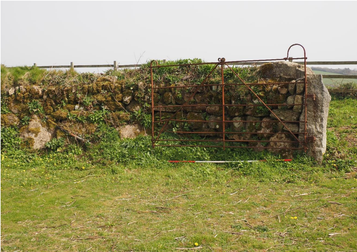
Figure 64: Context Cornish hedge south of Barn, with rare C19 wrought-iron field gate
