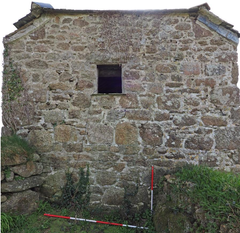
Fig 30: Barn north end
