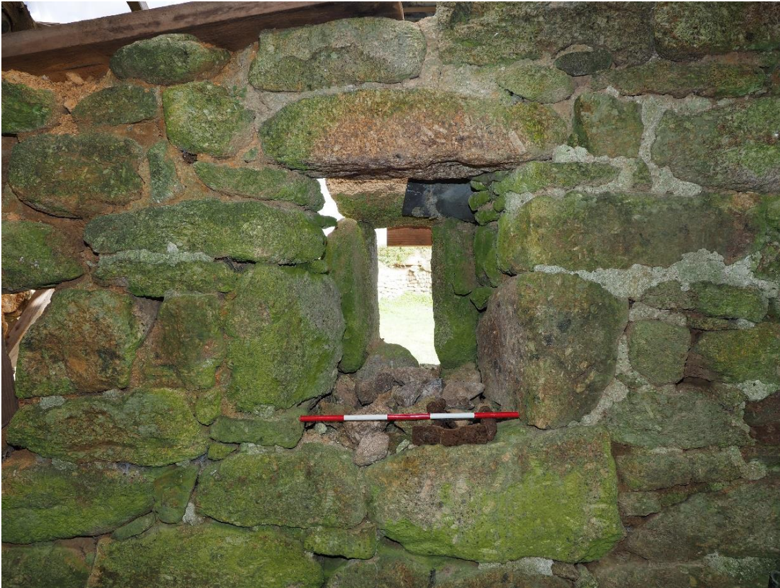
Figure 54: Cartshed: vent to centre of NE wall
