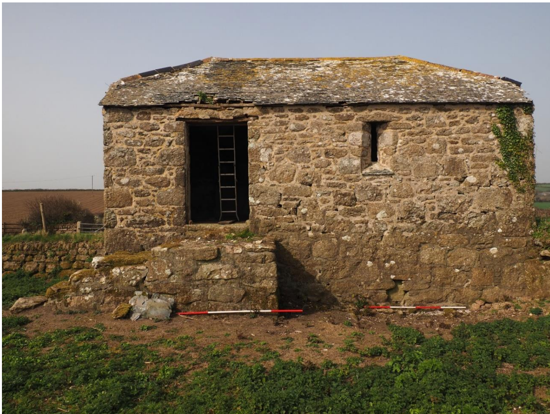
Figure 27: Barn east side
