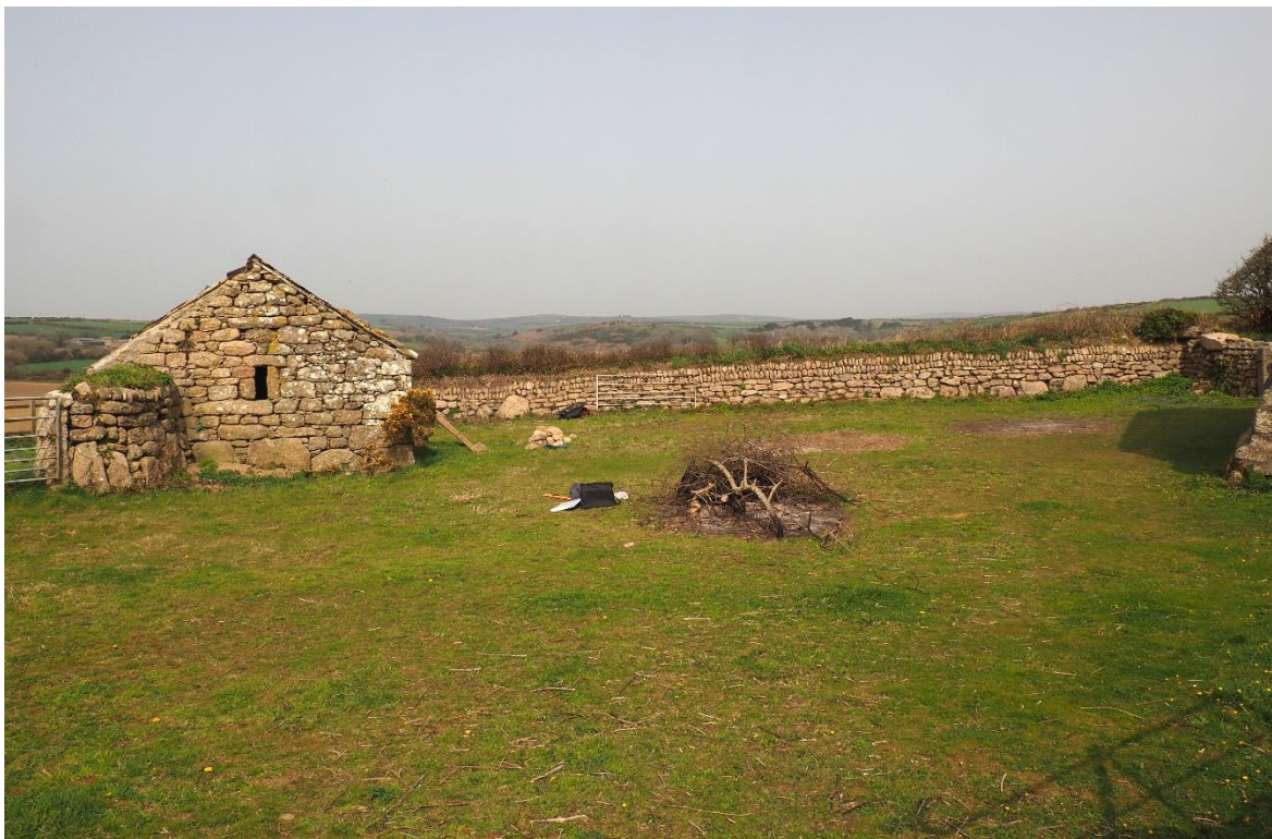
Figure 67: Context: Farmstead from SE: Cartshed, left, boundary hedge of farmyard beyond, located on site of probable former farmhouse
