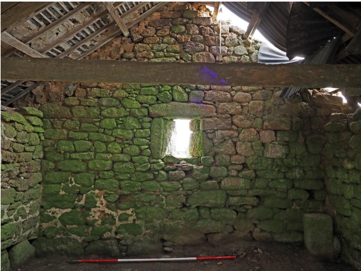
Figure 47: Cartshed SE wall
