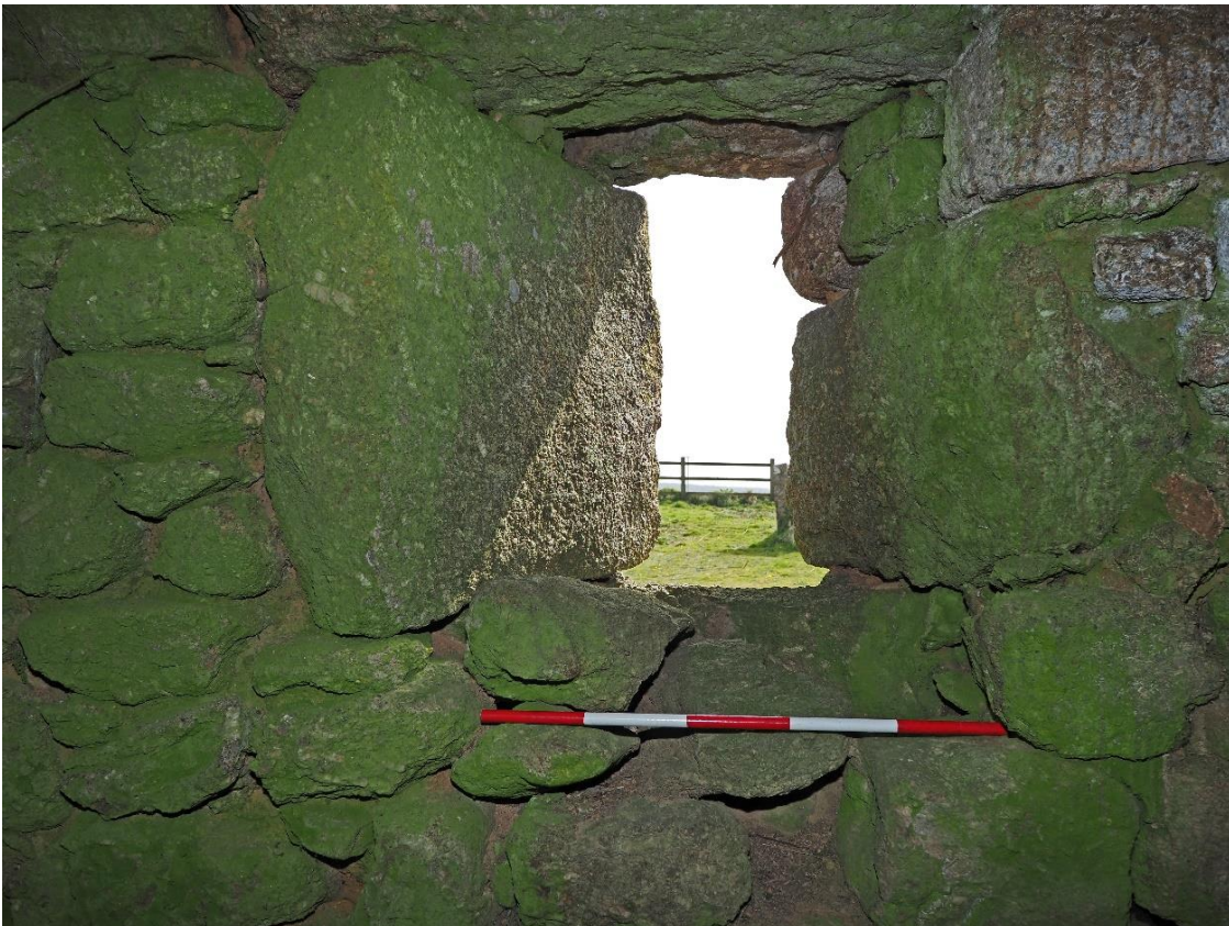
Figure 55: Cartshed: vent to SE gable end
